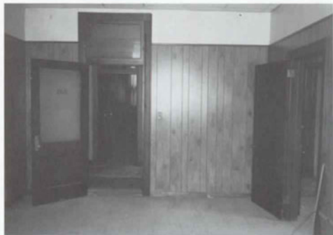
Fig. 53. Room 216 (Investigator's Office), West Wall [1988].
