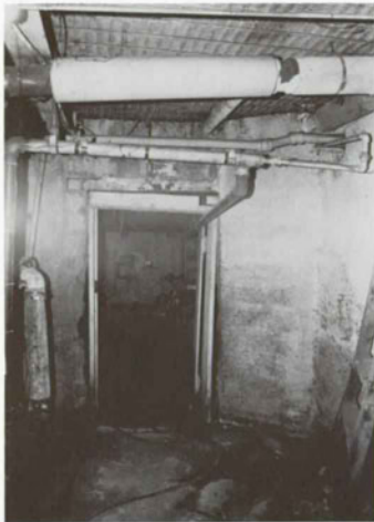
Fig. 22. Boiler Room, South Wall, Looking Toward Meter Room [1988].
