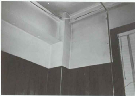
Fig. 49. Room 209 (Booking Room), Ceiling Detail at Southwest Corner [1988].
