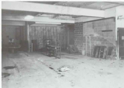
Fig. 33. Room 106 (Garage), Looking Southwest [1988].
