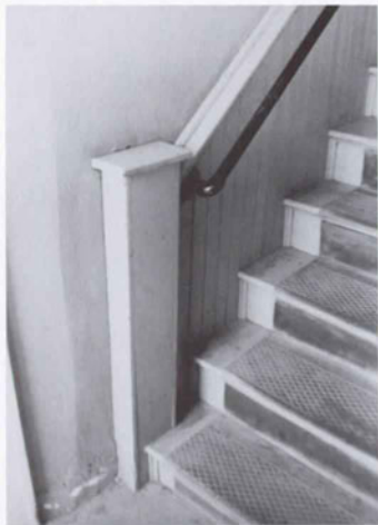
Fig. 24. Room 101 (Main Stairway) [1988].
