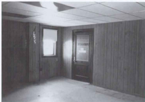
Fig. 42. Room 203 (Police Locker Room), Southeast Corner [1988].
