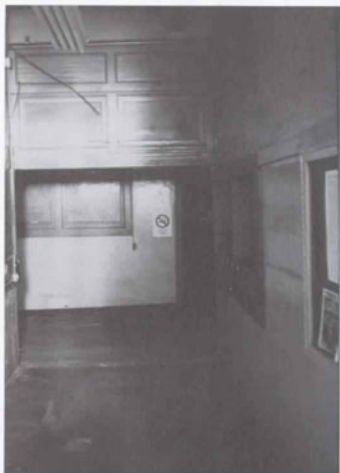
Fig. 43. Room 204 (Dispatcher Room), Looking North [1988].
