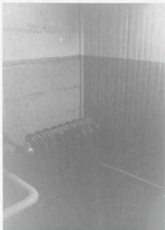
Fig. 36. Room 108 (Toilet), Northeast Corner [1988].
