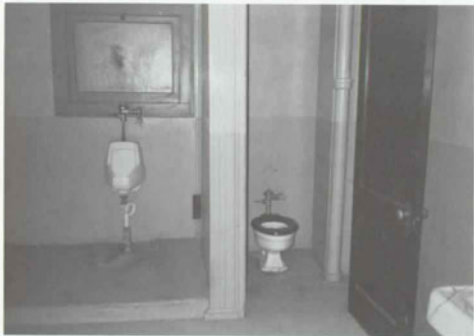
Fig. 54. Room 219 (Men's Bathroom), North Wall [1988].
