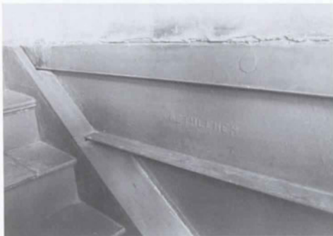
Fig. 41. Room 201 (Main Stairway) [1988].
