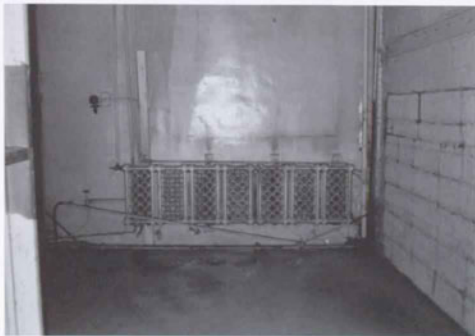
Fig. 38. Room 109 (Water Department), Northwest Corner [1988].
