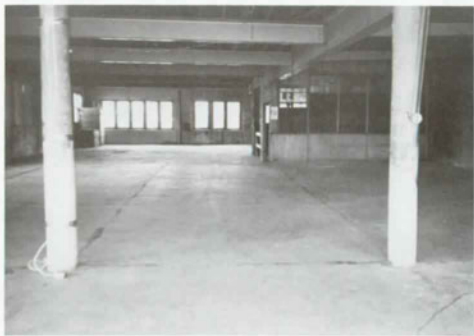
Fig. 56. Third Floor, Looking North [1988].
