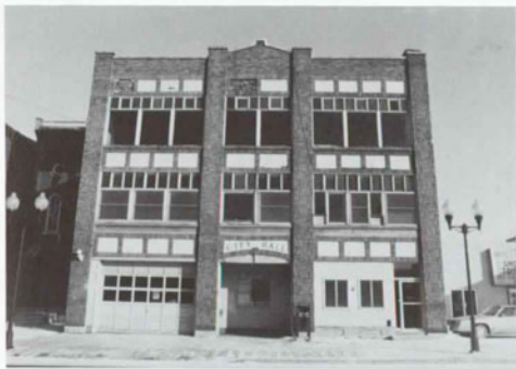
Fig. 13. Exterior South Facade [1988].
