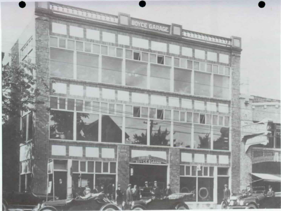
Fig. 4. Boyce Garage, South Facade [ca. 1916].
