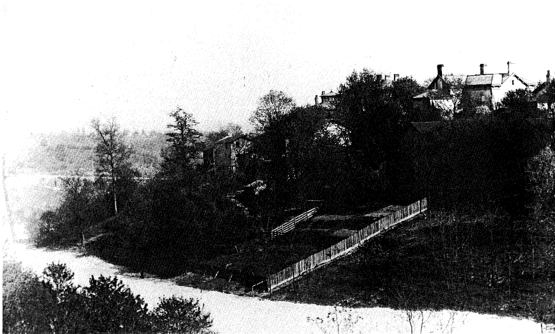
FIGURE A.11: A c. 1885-90 view of Mount Auburn back yards - It is clear from this photograph that homeowners in the Mount Auburn area maintained agrarian activities in the rear of their properties. Typical farm board fences are apparent, gardens, pasture land, fruit trees and vine culture can be detected. Source: Cincinnati Historical Society.
