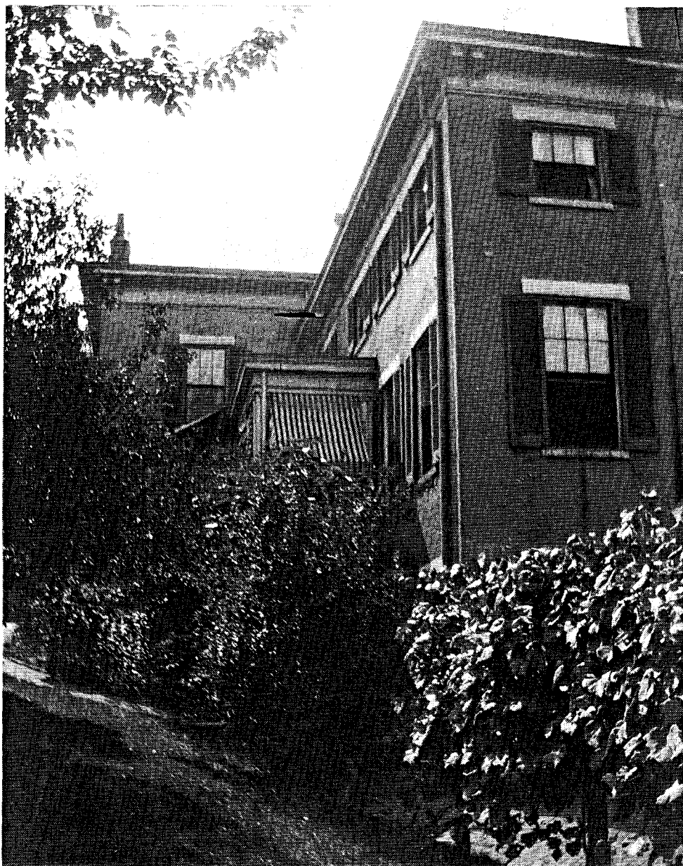
FIGURE A.5: A c. 1910 view of the southeast corner of the house, showing a healthy grape vine, its arbor and a brick path which allegedly led to the privy shown at right. A 1991 view of the scene shown at left. Source: Cincinnati Historical Society (right); The Westerly Group, Inc. (left).
