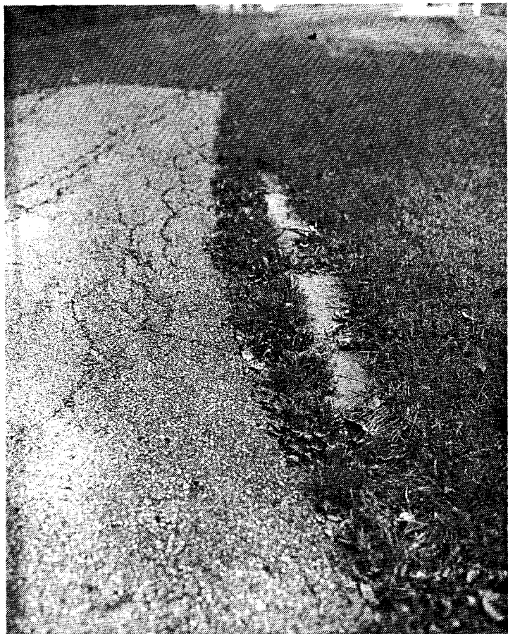
FIGURE A.18: A c.1955-60 view, looking at the southeast corner of the house, of a masonry curb, or possibly the top of a retaining wall shown at right. A 1991 view of this feature, of unknown origin, can be seen in the south drive today, shown at left. Sources: William Howard Taft National Historic Site Archives (right); The Westerly Group, Inc. (left).
