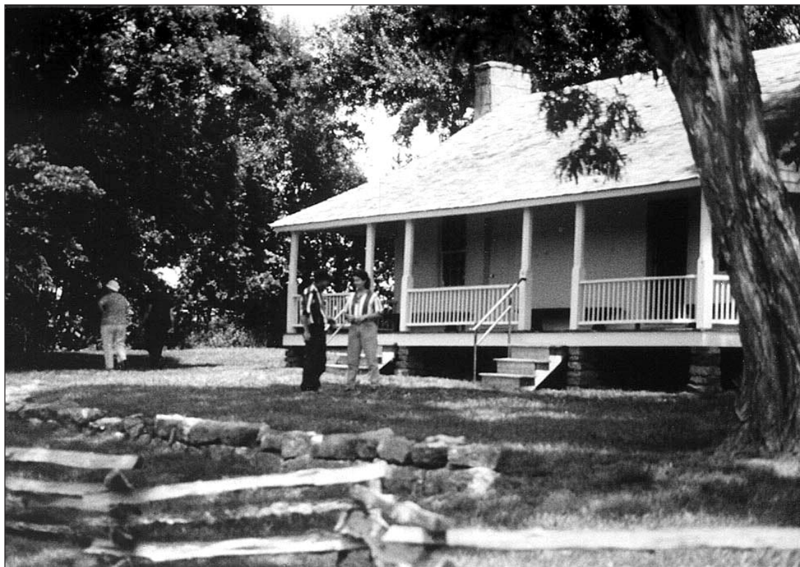
Figure 6. The Ray house is the only structure still standing from the Civil War era.
