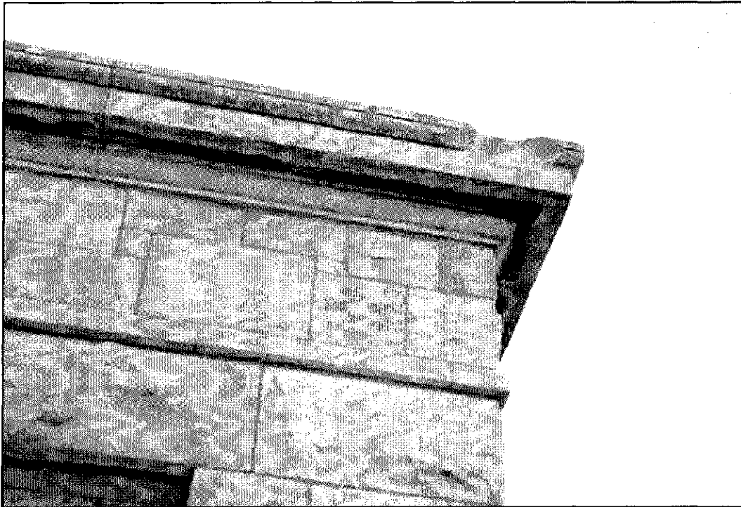
Figure 5.4: Monument Lodge, east façade, old damage at northeast corner of cornice.
