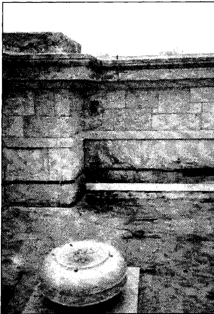
Figure 4.17: Monument Lodge, concession addition roof, southwest downspout from lodge roof.
