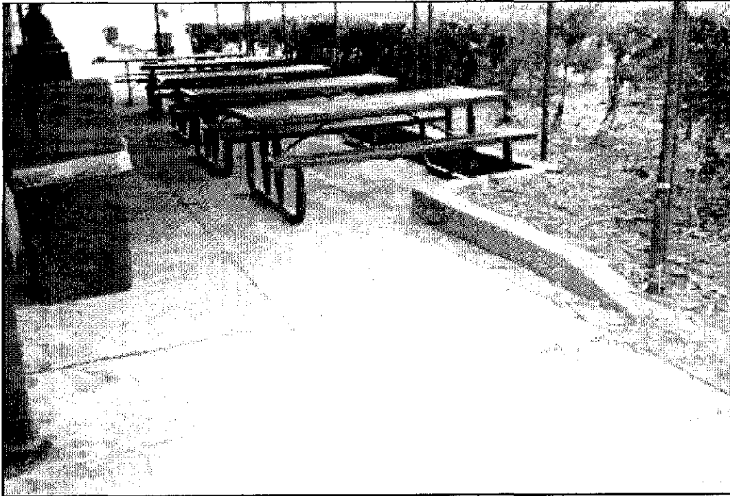
Figure 4.4: Monument Lodge, site, west façade, paving at porch.
