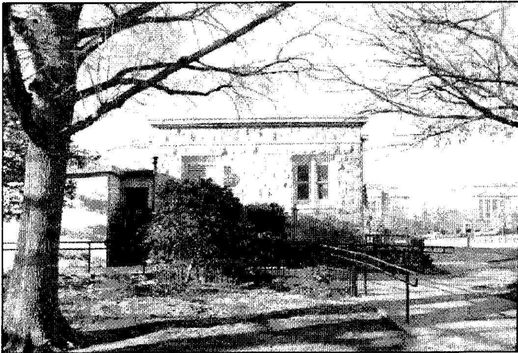
Figure 4.11: Monument Lodge, south façade.
