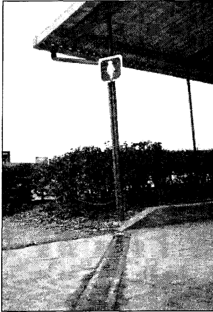
Figure 4.28: Monument Lodge, Concession Addition, southwest corner, downspout and drain.
