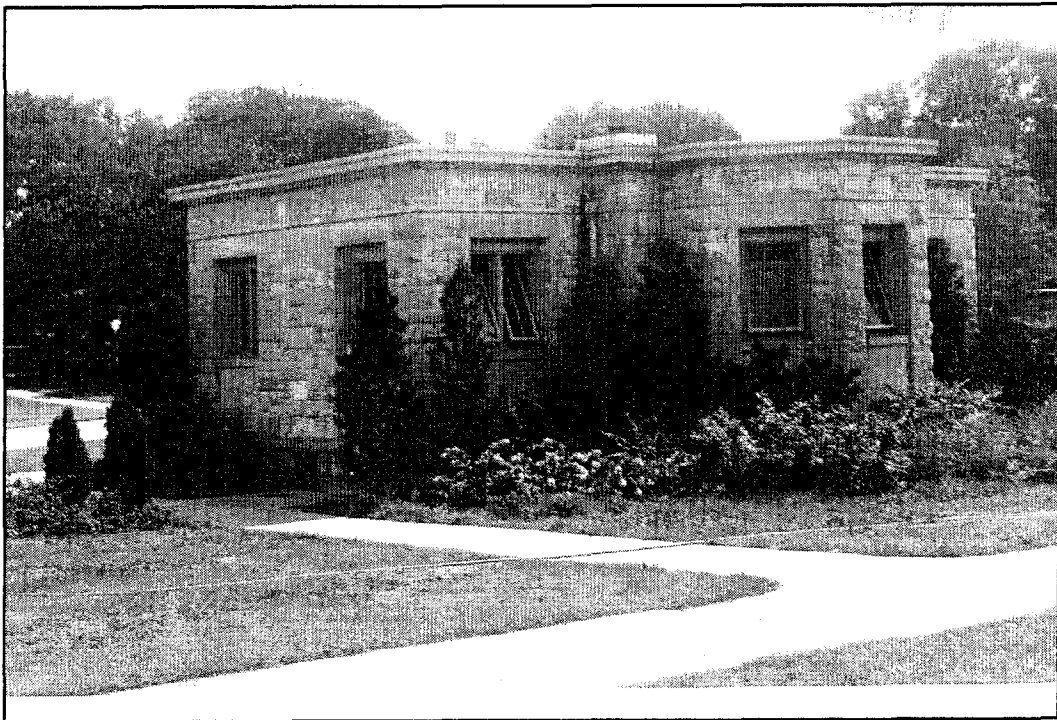
Figure 2.14: View of northeast corner of the Monument Lodge, 1 September 1932 ([Photograph] 1 September 1932; NPS-NCR Collection).
