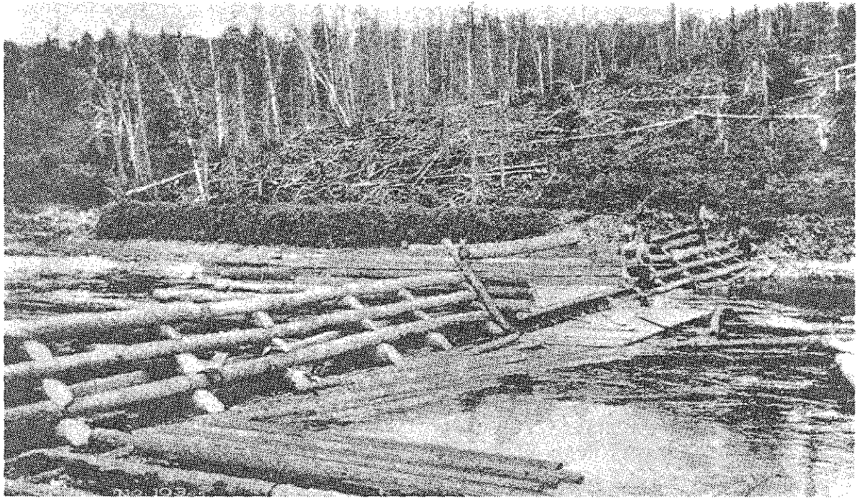
Figure 23: Damming a stream to raise water for floating logs, c. 1928 (Minnesota Historical Society).
