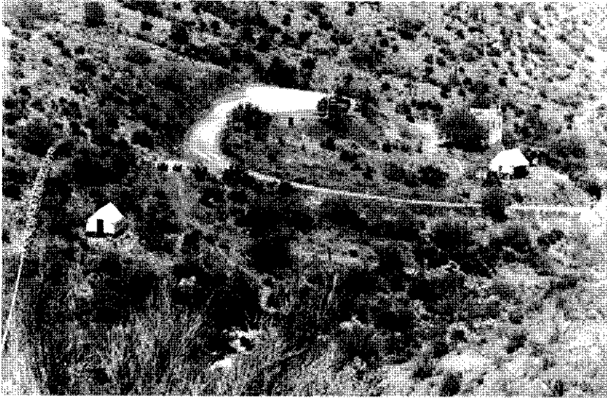
Figure 32: Tonto National Monument parking area and ranger housing, 1941
