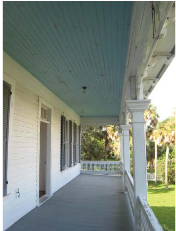
Figure 21 , Original beaded board ceiling and modern flooring of the second-floor porch.
