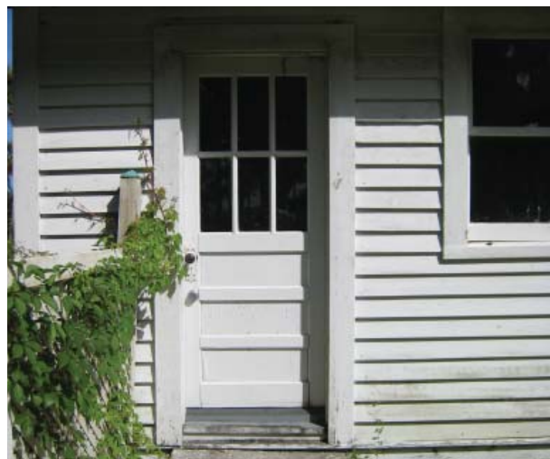
Figure 36, At the northernmost doorway of west elevation of Rear Shed, an early twentieth-century sash door.
