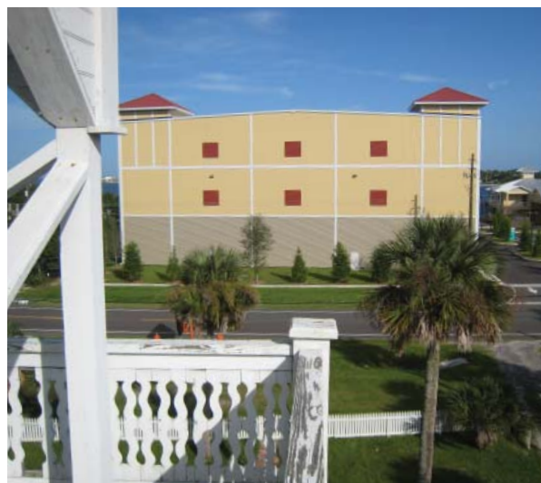
Figure 28 , View from cupola blocked by 2008 boat storage facility. (Oppermann, 2009)
