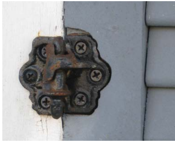
Figure 29 , Inaccurate replacement shutter hinges on shutters of the east elevation of the Main Block.
