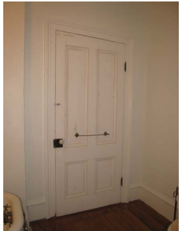
Figure 63, Room 105-Bathroom door at east wall to Room 101-Reception Room.
