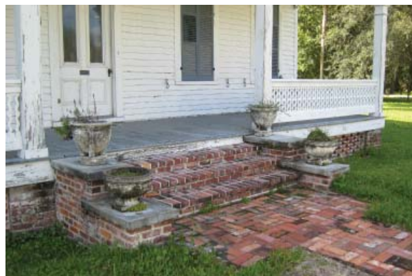
Figure 24 , Brick steps of east elevation.
