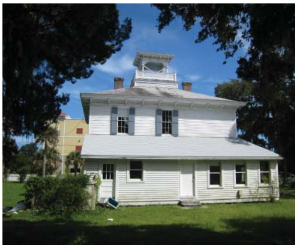
Figure 24. Back of house showing replacement windows and weatherboard siding added 1996-2003. (Oppermann, 2009)
