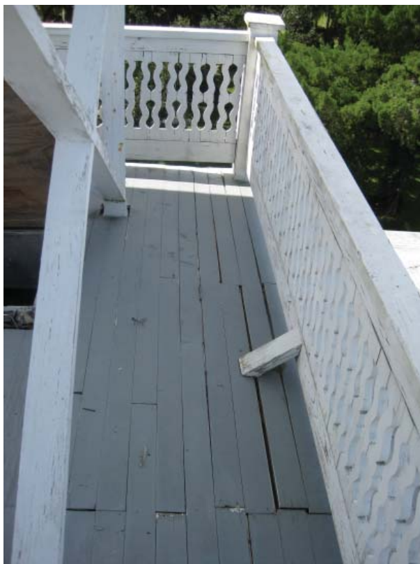
Figure 23 , Modern flooring, X-bracing, and balustrade of the widow's walk and cupola.
