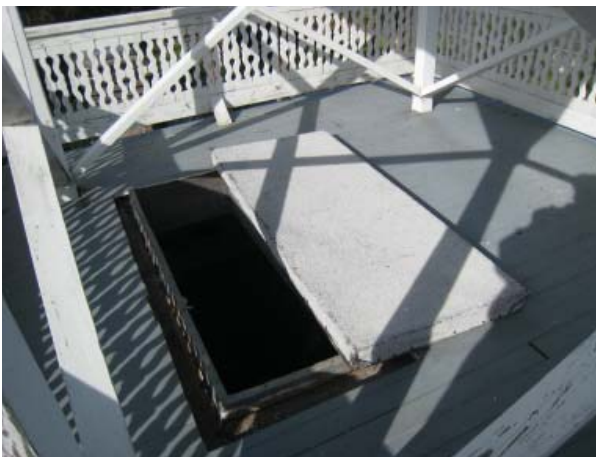
Figure 101, Hatch providing access to the widow's walk and cupola.
