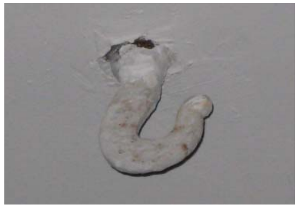
Figure 58, Room 103-Northeast Office ceiling hook.
