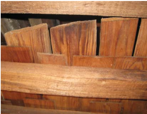
Figure 18, Early wood shingles beneath the deck of the widow's walk.
