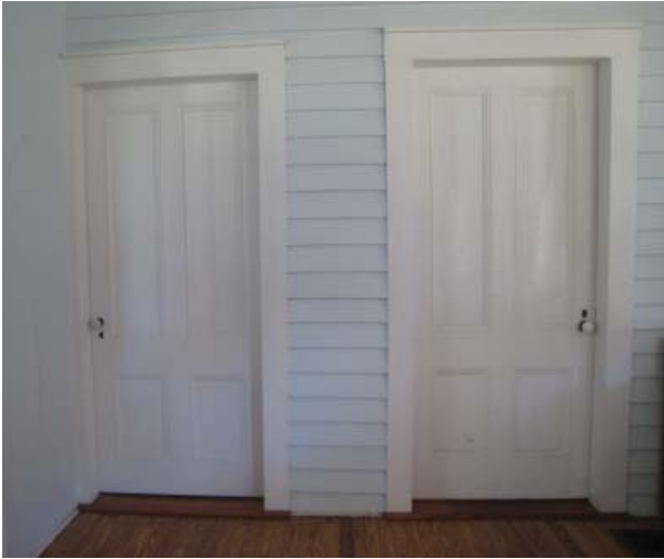
Figure 75 , Doorways on the east wall of Room 108-Conference Room lead to Room 104-Northwest Office (left) and Room 102-Center Hall (right). Both doorways have flush board casing with a drip edge.
