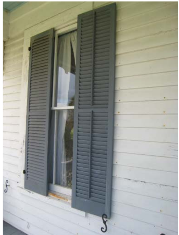
Figure 27 , Second-floor east elevation reproduction louvered shutters based on salvaged shutter.
