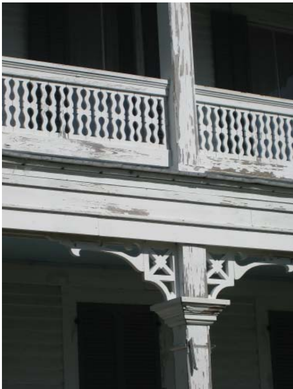
Figure 20 , Sawn trim and balustrades of the east-elevation porches.
