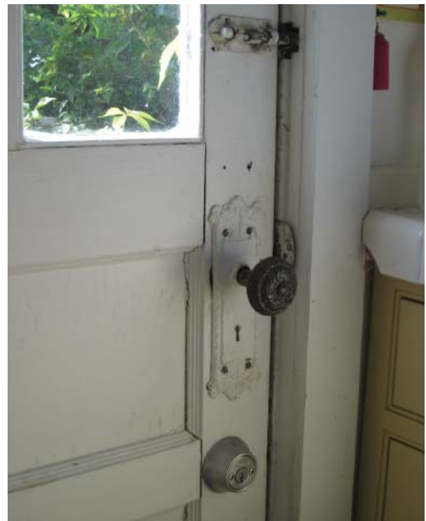
Figure 72 , Room 107-Kitchen door to exterior with embossed, pressed escutcheon, embossed doorknob, barrel lock, and modern dead bolt.
