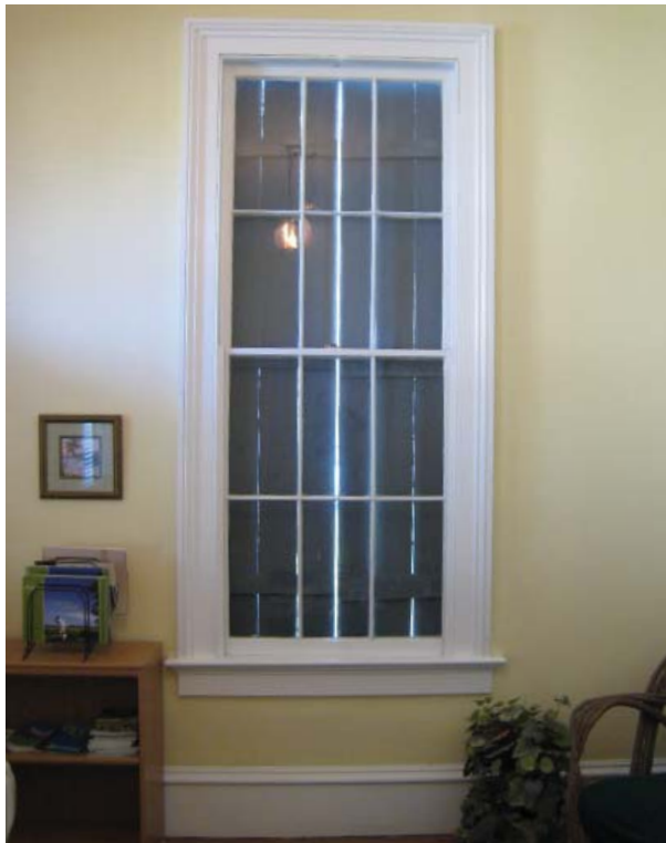
Figure 40 , Typical six-over-six double-hung sash window of north, south and west elevation of Main Block.
