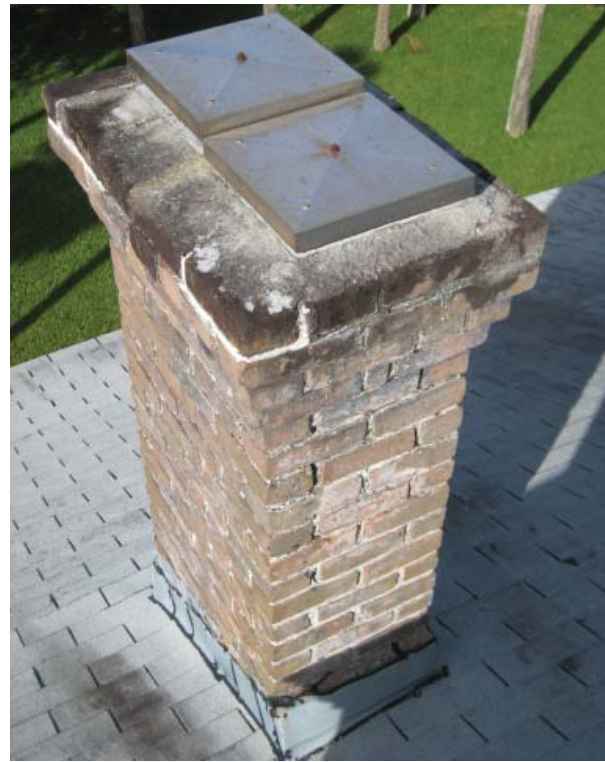
Figure 19, Chimney at north roof hip.
