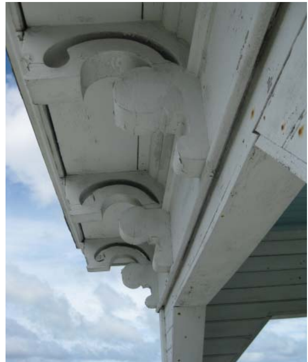
Figure 23, Cornice brackets of cupola
