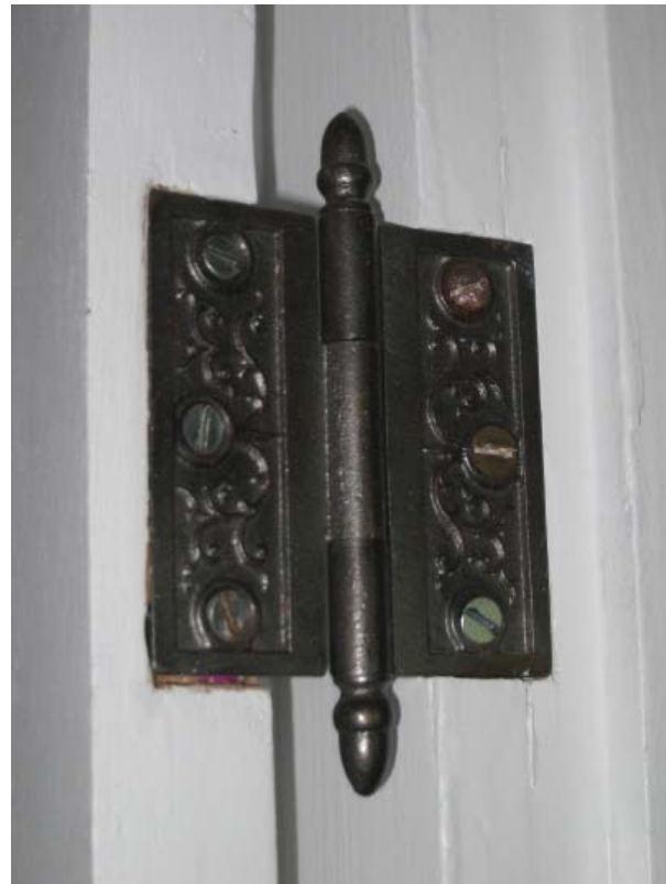
Figure 42 , Reproduction hinge with acorn pin is a common late design element found on doors throughout the house.
