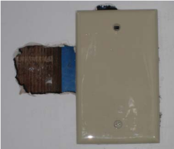
Figure 71 , Area of gypsum board removed to reveal an original stud, which shows lime stains and nail holes. This indicates the wall had plaster on lath at one time, probably originally.
