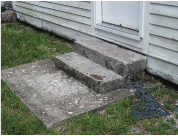
Figure 25 , West elevation poured-in-place concrete pad and cement stucco over brick steps at center doorway.
