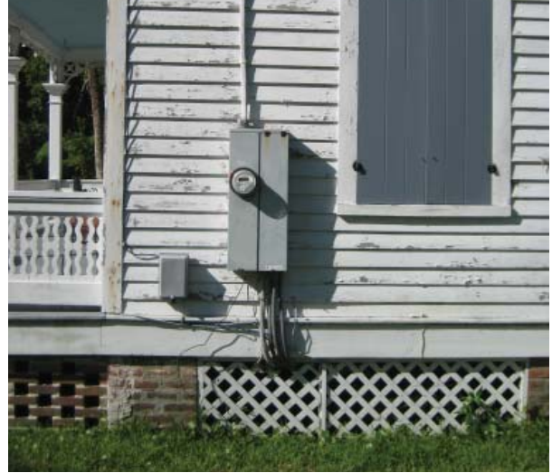
Figure 17 , Distribution panel and meter on the east end of the north elevation.
