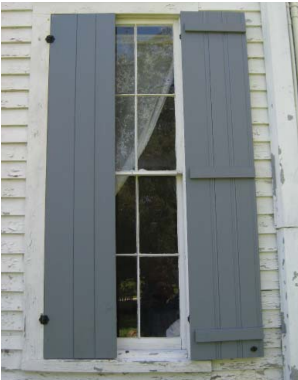
Figure 31 , Typical board-and-batten shutters as occurring on the north, west, and south elevations of the Main Block.
