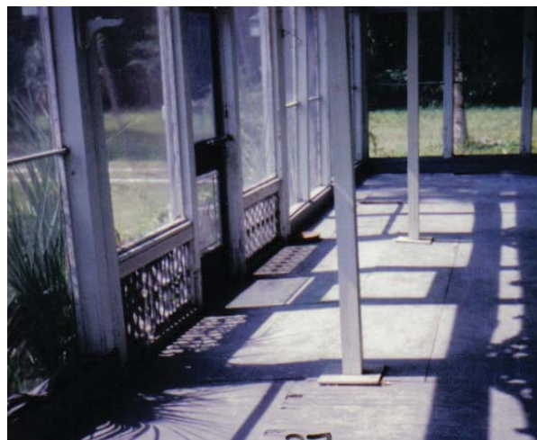
Figure 17, Interior of the screened porch in 1996 showing 4-by-4s supporting second-floor porch. (Zillgitt)
