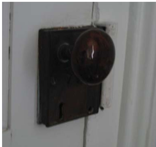
Figure 79, Room 201-Southeast Office door to Room 202-Center Hall, hardware.
