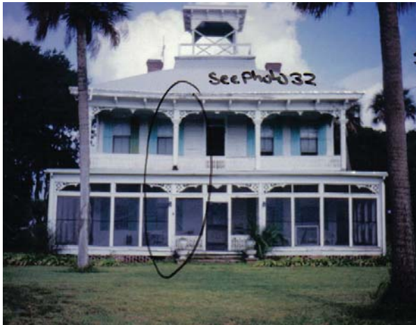
Figure 22, Porches in 1996 showing sagging roof. (Zillgitt)
