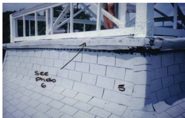
Figure 18, Cupola railing, floor, and shingled base in 1996. (Zillgitt)
