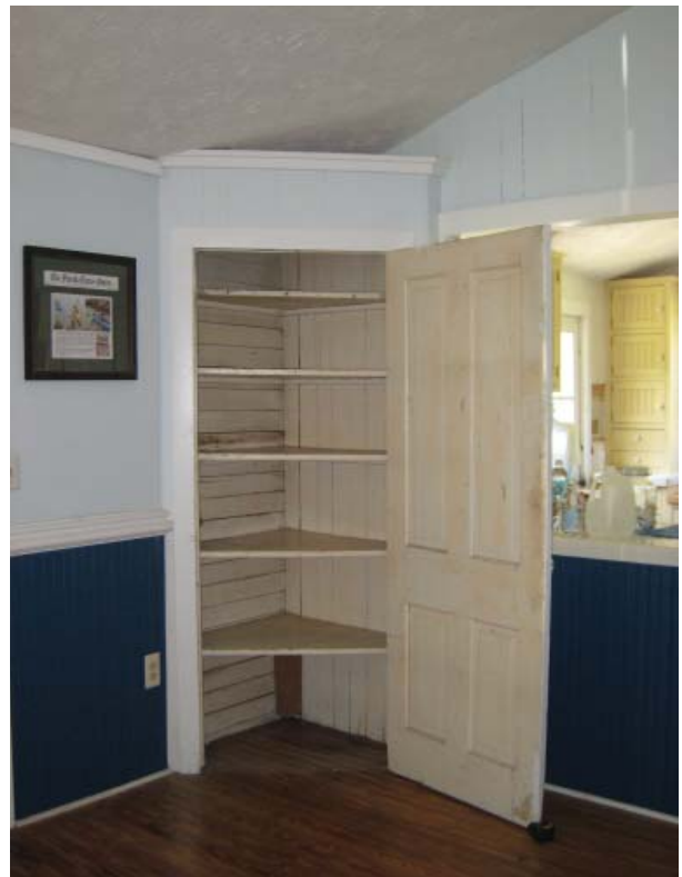
Figure 76 , Room 108-Conference Room closet at northwest corner.
