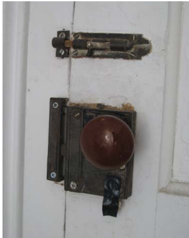
Figure 84, Room 202-Center Hall door to east porch, hardware.
