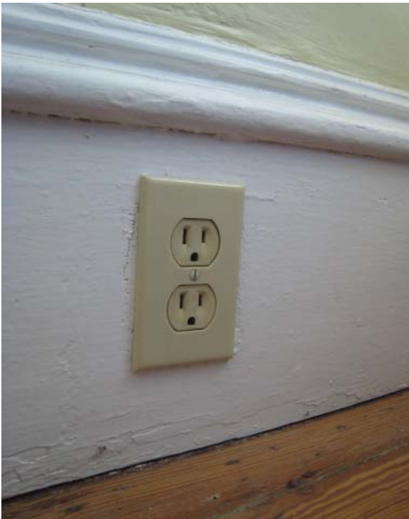
Figure 43 , Modern molded-plastic outlet covers installed in 1996-2003 throughout the house.
