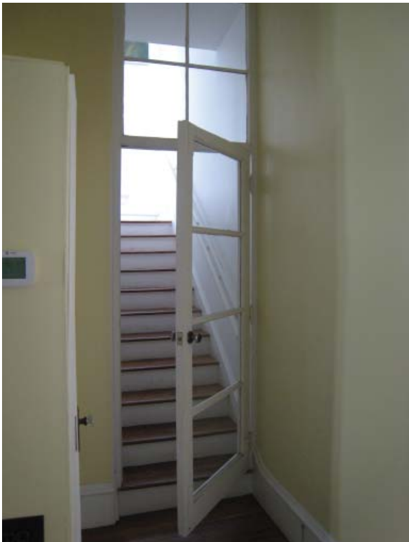
Figure 49, Door to Room 106-Lower Stair Hall from Room 102-Center Hall.
