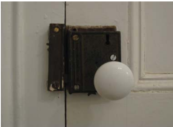
Figure 64, Room 105-Bathroom door to closet, hardware.
