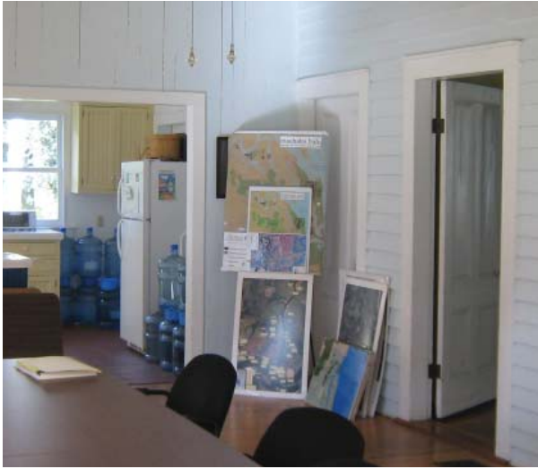
Figure 13. Weatherboards form the east walls of Room 108-Conference Room of the Rear Shed. Exposed vertical boards form the south side of the dividing wall between Room 107-Kitchen and Room 108-Conference Room of the Rear Shed.
