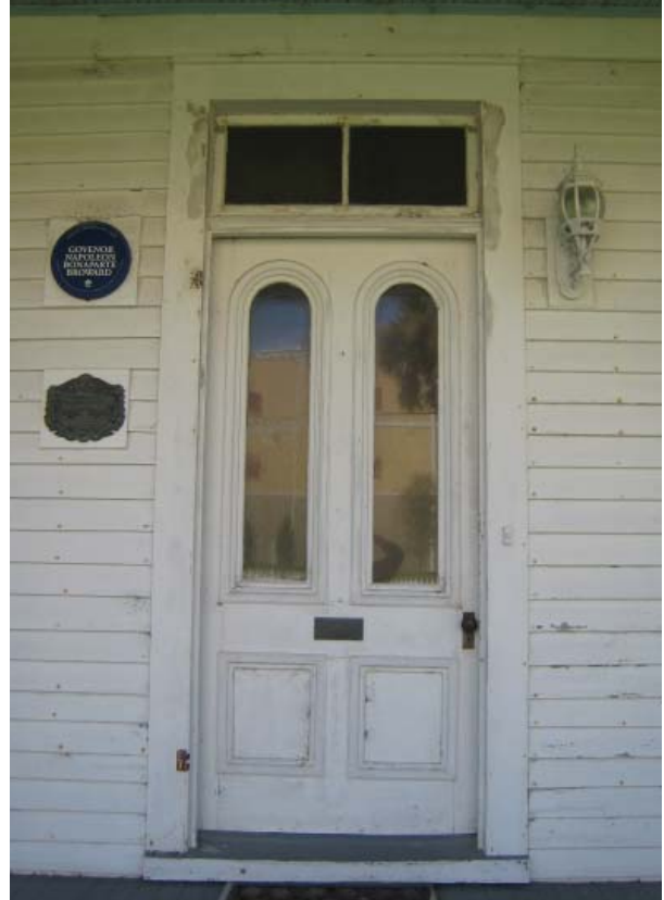
Figure 32 , The front entrance doorway, east elevation.
