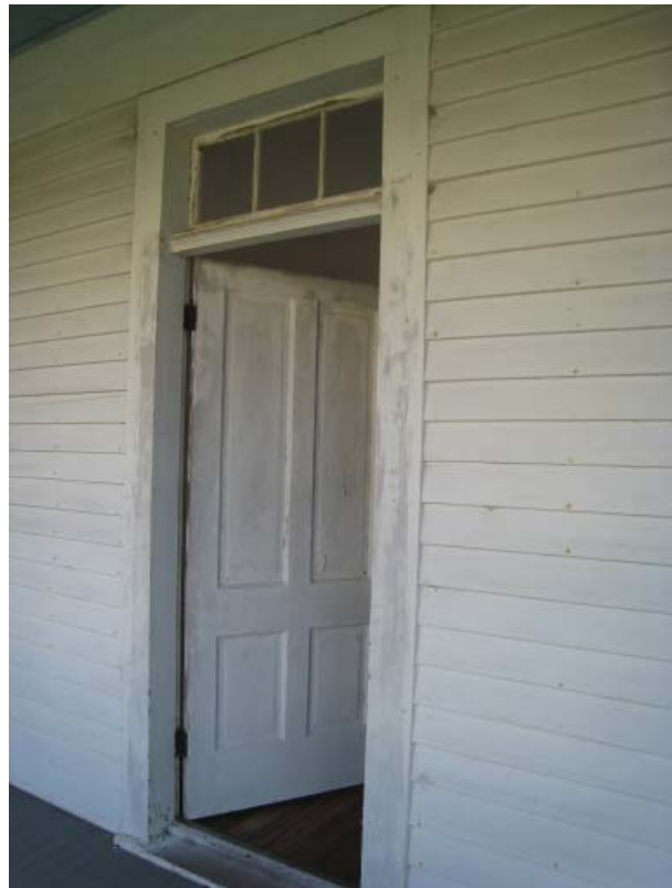
Figure 35, East elevation second-floor doorway.
