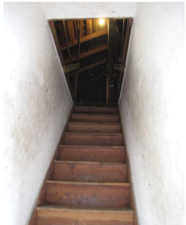
Figure 97, Room 207-Attic Stair Hall facing east.
