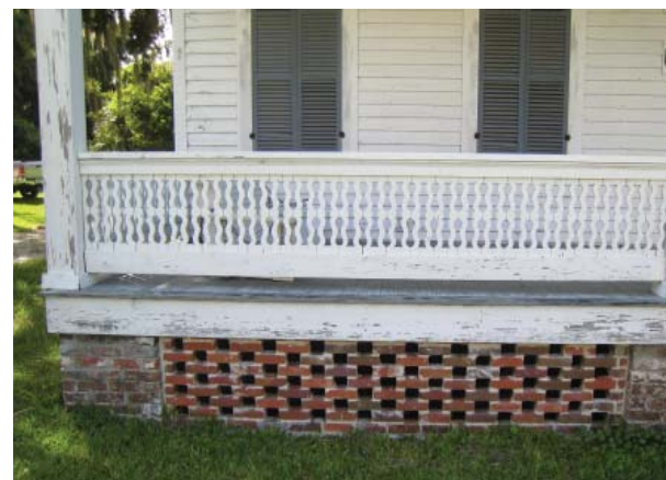
Figure 10, Original brick porch piers on the east elevation with twentieth-century brick lattice infill.
