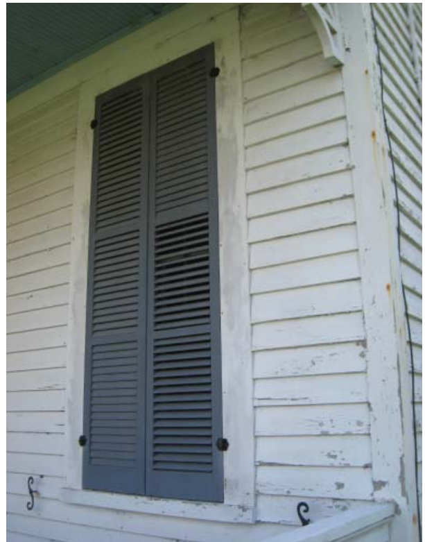
Figure 26 , First-floor east elevation reproduction louvered shutters based on salvaged shutter.
