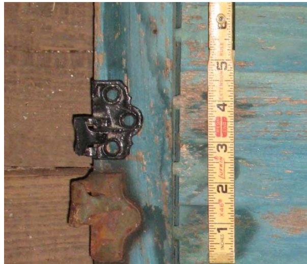
Figure 30 , Salvaged louvered shutter stored in Attic, showing different size of early hinge compared to replacement hinge above (Figure 29).
