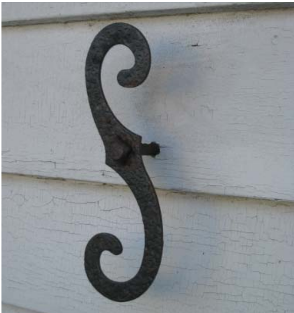
Figure 28 , Typical modern shutter dog added to east-elevation shutters in 1996-2003.
