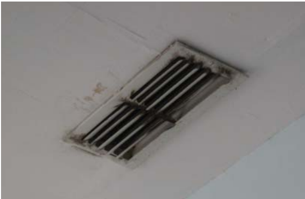
Figure 44 , Modern metal return registers installed in 1996-2003 at second-floor rooms.
