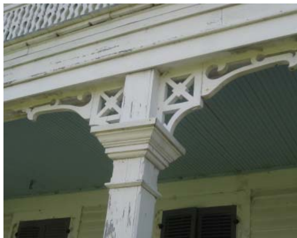
Figure 21, Porch post brackets showing replaced straight “X” pieces and repaired scroll-cut elements.. (Oppermann, 2009)
