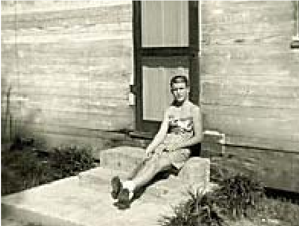
Figure 8 , Back of rear shed in the 1950s showing flush horizontal siding. (courtesy of Broward sisters)
