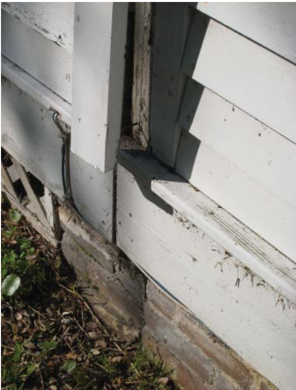
Figure 12. The westernmost pier of the south elevation of the Main Block abutting the easternmost pier of the Rear Shed.
