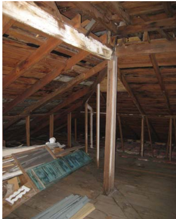
Figure 98, Northwest oblique of the Attic.
