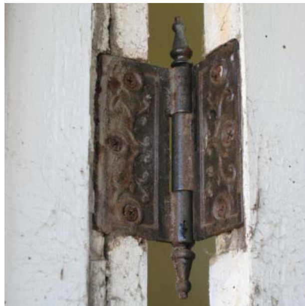
Figure 33 , Salvaged front door hinge, exterior view.
