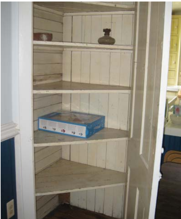
Figure 9 , Corner closet showing the horizontal flush boards of the exterior wall and the corner junction with the vertical flush boards of the interior partition wall between Rooms 107 and 108. (Oppermann, 2009)
