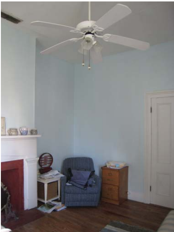
Figure 77, Northwest oblique of Room 201-Southeast Office.
