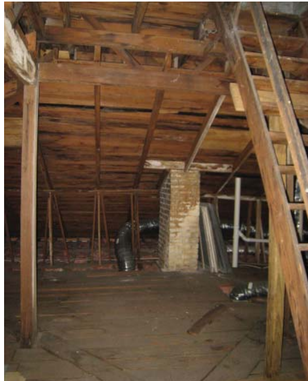
Figure 99, Attic looking south.
