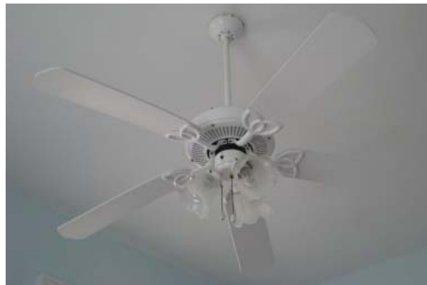
Figure 87, Room 203-Northeast Office modern three-globe ceiling fan/light fixture.
