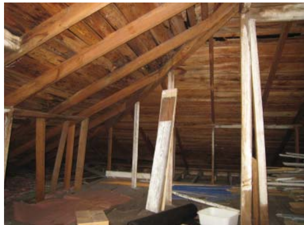
Figure 14. Northwest oblique of Attic framing.
