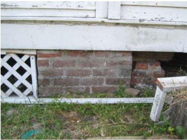
Figure 11. The westernmost pier of the north elevation of the Main Block is also the easternmost pier of the original Kitchen Ell.
