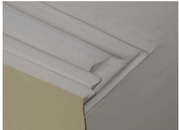
Figure 57, Room 101-Reception Room and Room 103-Northeast Office cornice.
