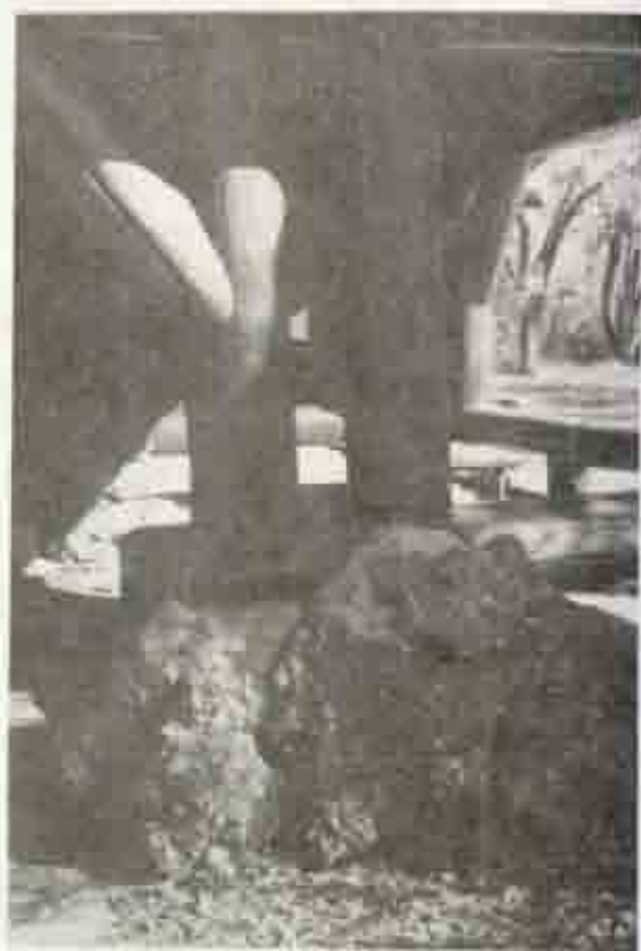
Illus 10. Details of construction, large shelter at Squaw Creek campground (photograph by author, taken October 1977)
