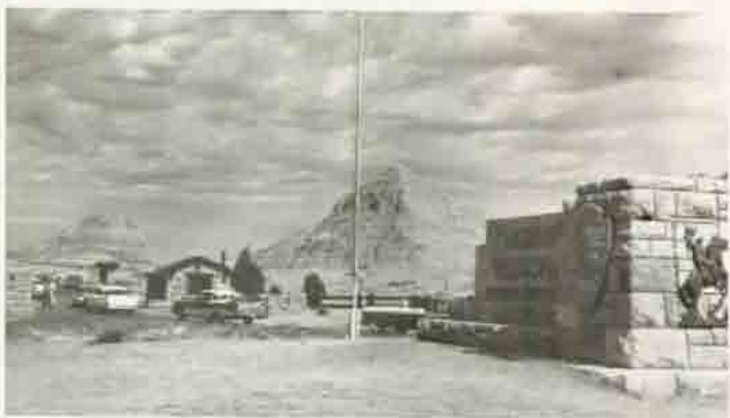
Illus 3. Pylon at east entrance (photograph from park files, taken September 12, 1959)
