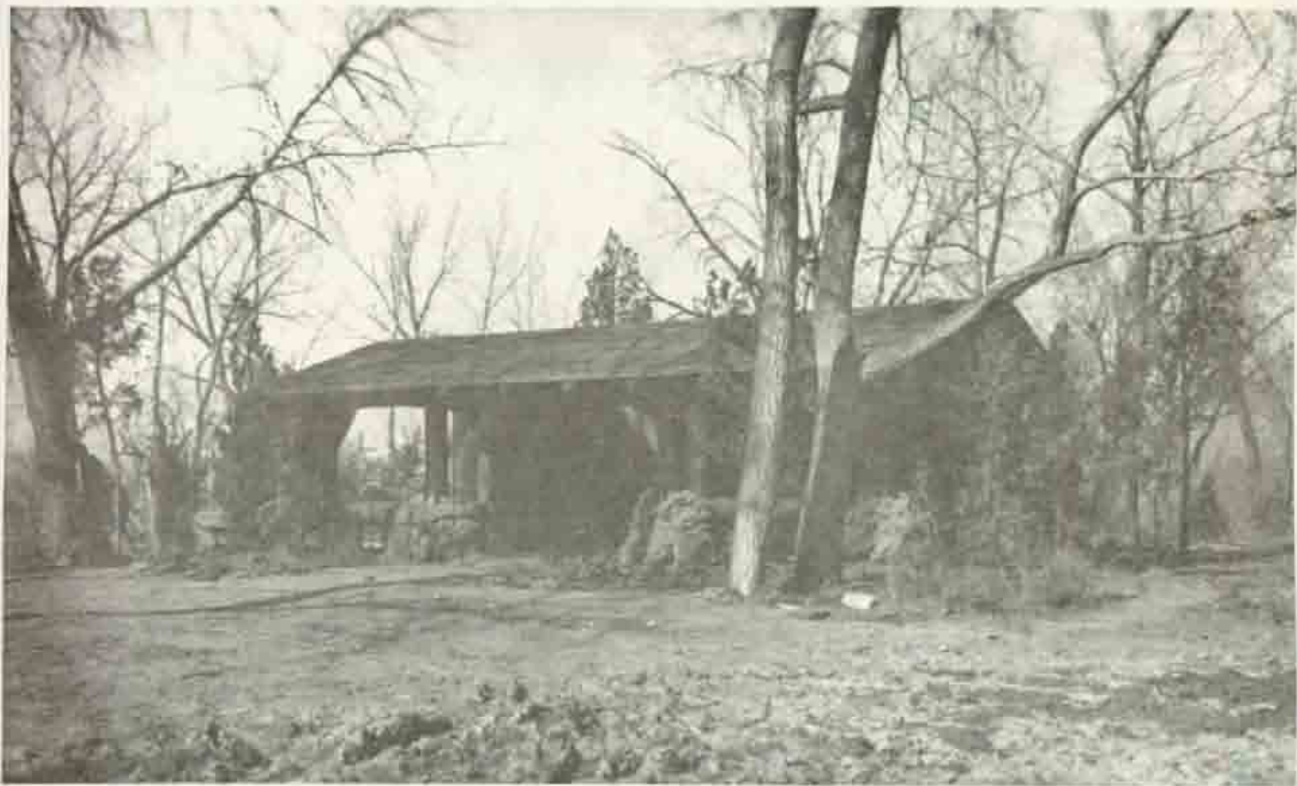
illus 7. Large shelter at Squaw Creek campground, soon after construction (photograph from National Archives, taken ca. 1938)
