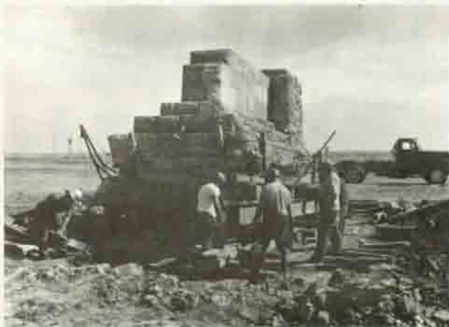
Illus. 4. Pylon being moved from east entrance to Painted Canyon overlook (photograph from park files, taken August 1968)
