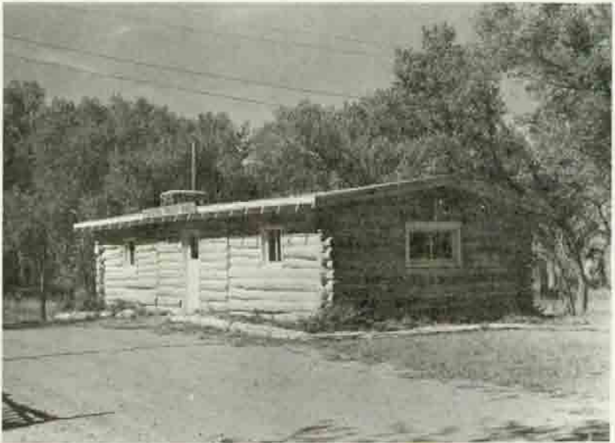
Illus 30. Bunkhouse at Peaceful Valley Ranch (photograph from park files, taken 1947)
