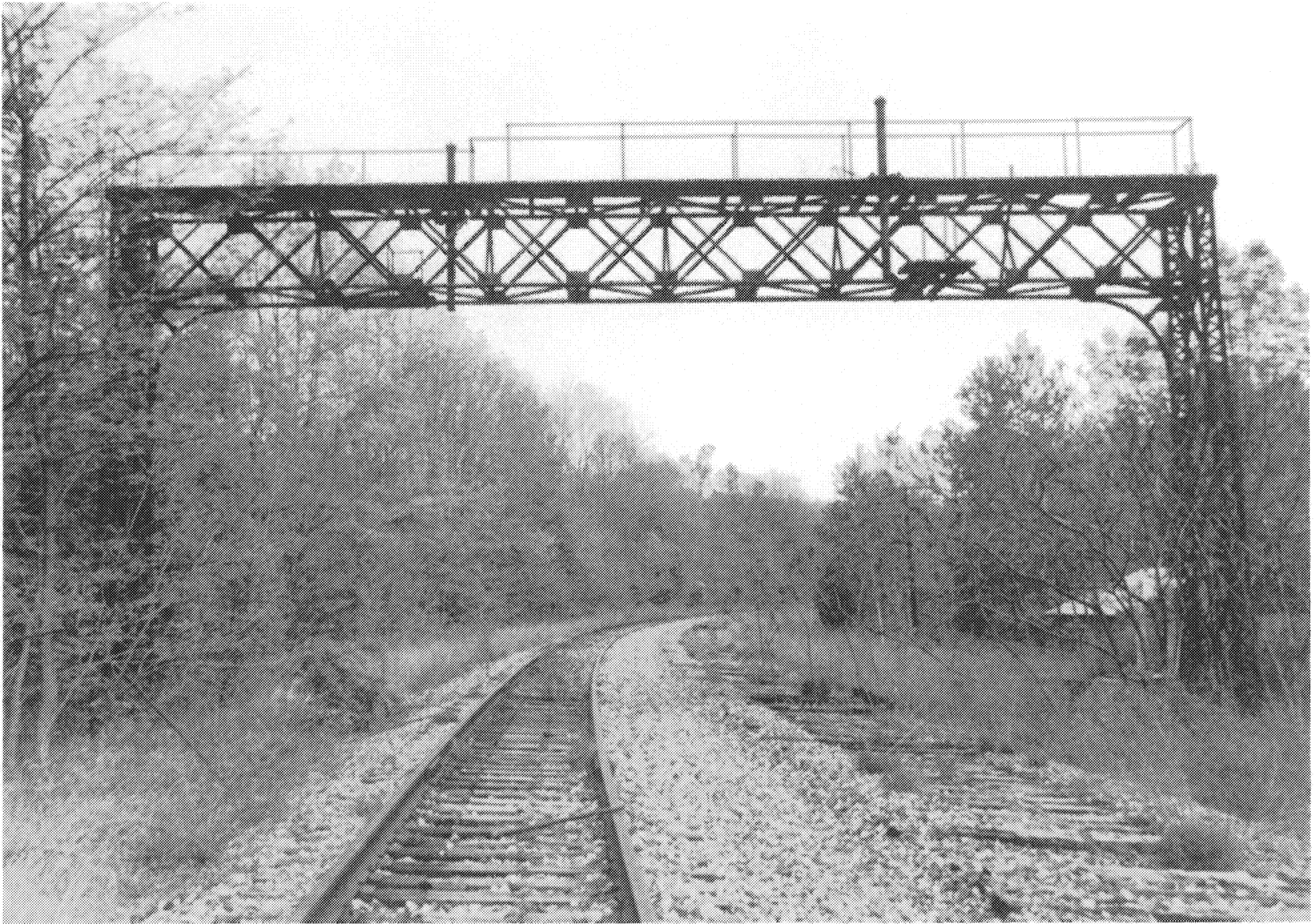
Figure 24 May 1989 Amalomink Signal Bridge
