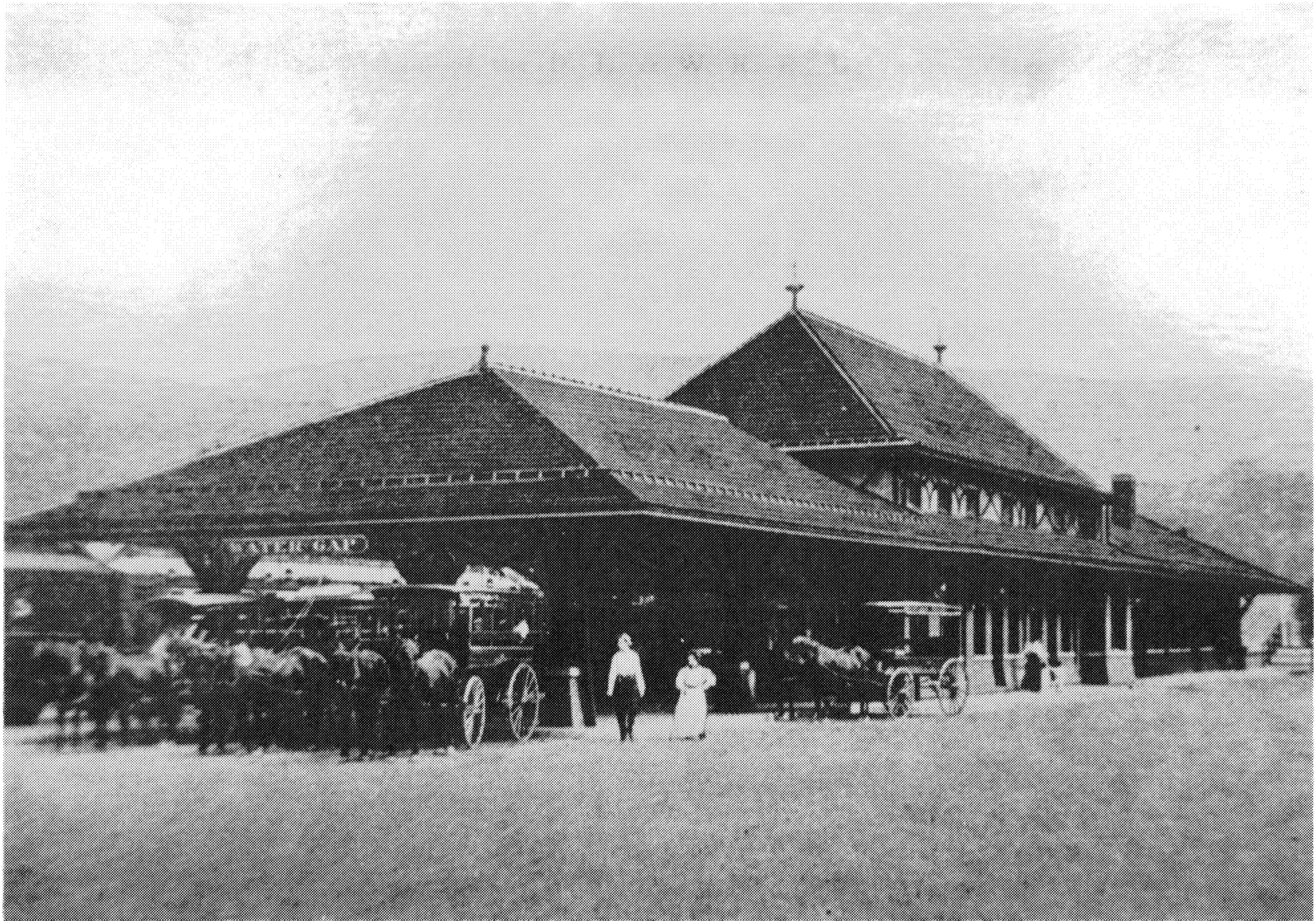
Figure 9 Ca. 1903 Delaware Water Gap Passenger Station Courtesy of the Monroe County Historical Society Stroudsburg, Pennsylvania
