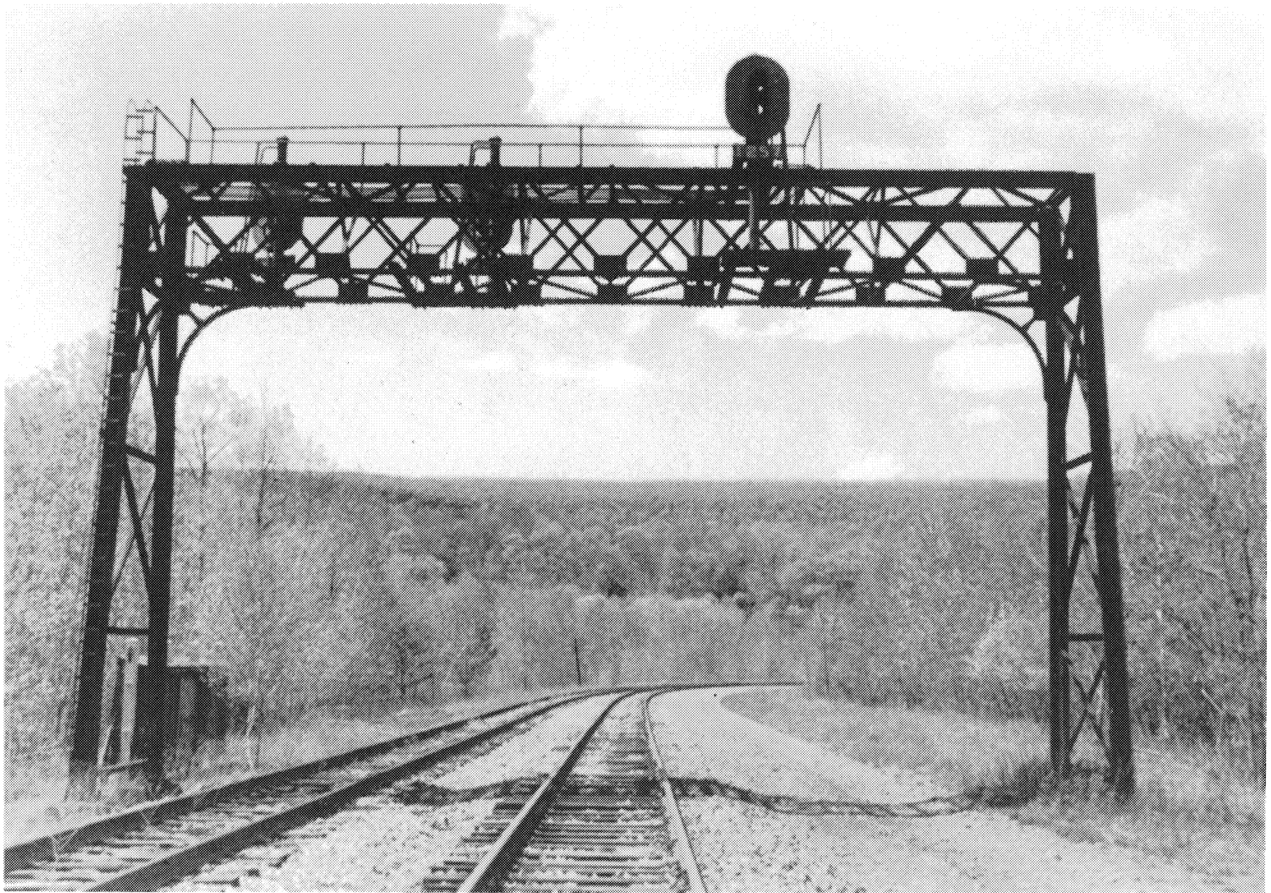
Figure 25 May 1989 Signal Bridge at Mile 125.70
