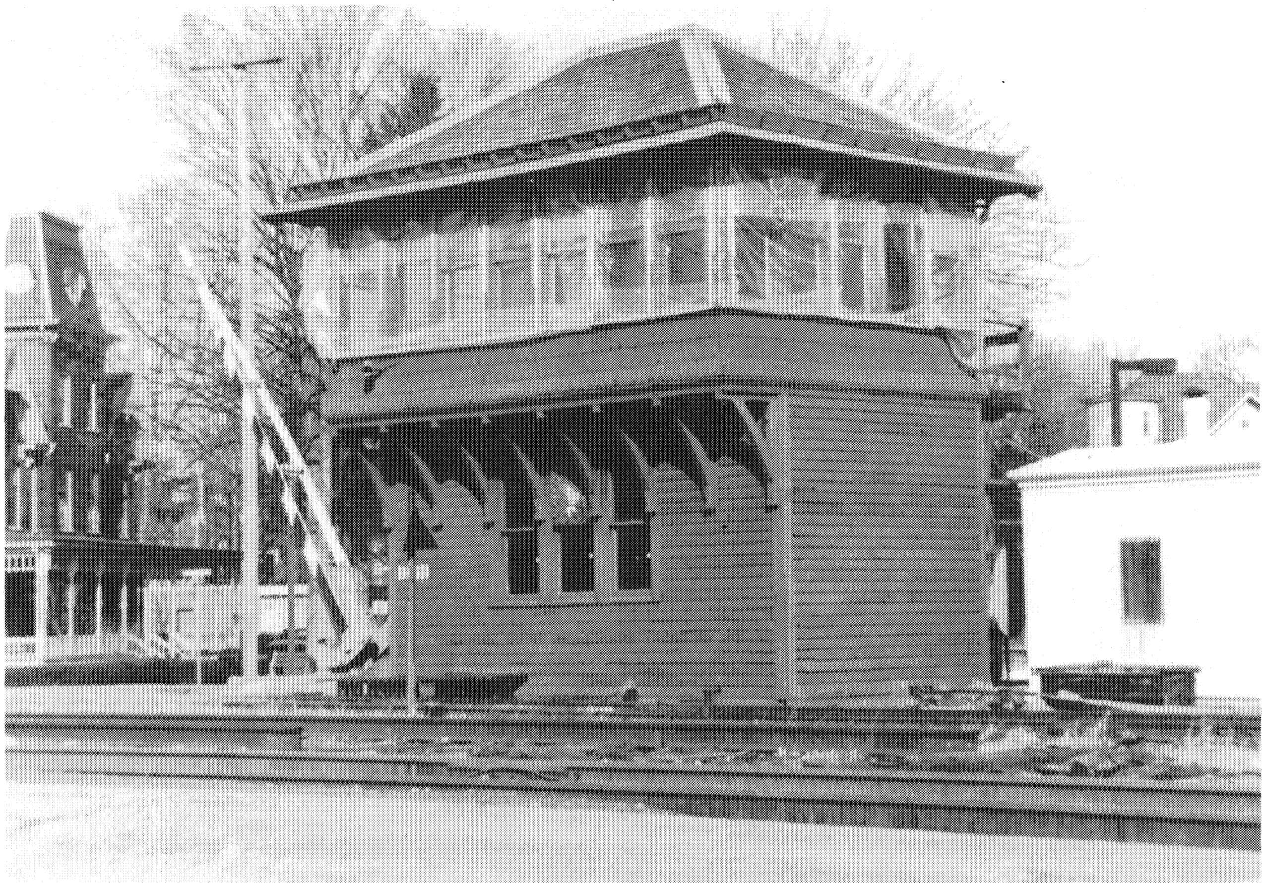
Figure 21 February 1989 East Stroudsburg Interlocking Tower
