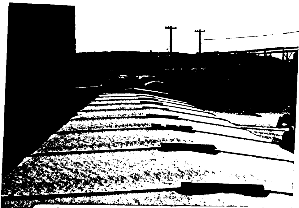
Roof of boxcar showing mounts for roofwalk.
