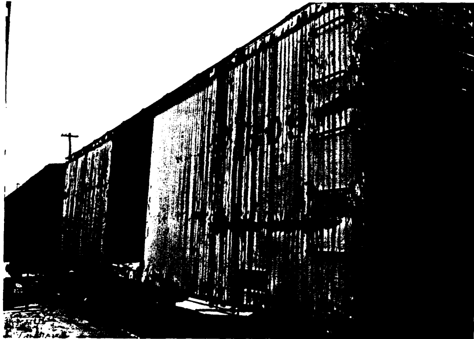
Fig. 17. Right side of boxcar No. 43651, showing the deteriorated condition of the sheathing. Photograph by Mark Morgan.
