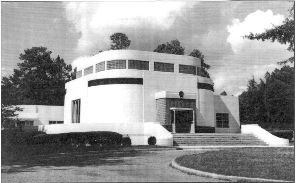
FIGURE 13. The Museum and Administration Building at Ocmulgee National Monument. In October 1968, Director Hartzog authorized the Southeast Archeological Center to assume responsibility for park management under line authority of OAHP. This experimental arrangement was later abandoned. SEAC operated from the basement of this building, whose construction began in 1938. Negative Number 67-OCM-3, no date; NPS Historic Photograph Collection, Harpers Ferry Center
