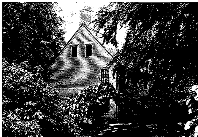
Spencer-Pierce-Little House, Newbury
