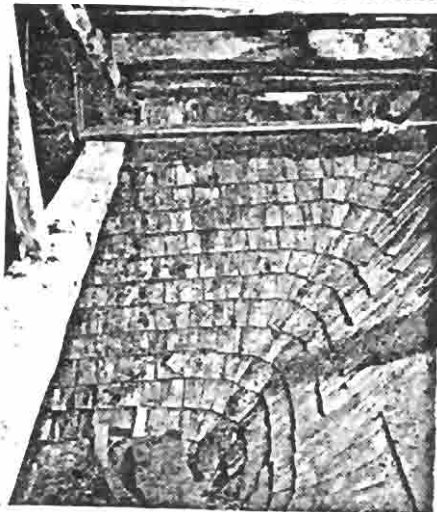
ORIGINAL ROOF CONSTRUCTION (COVERED BY LATER ROOF), ST. MICHAEL'S CHURCH, MARBLEHEAD
