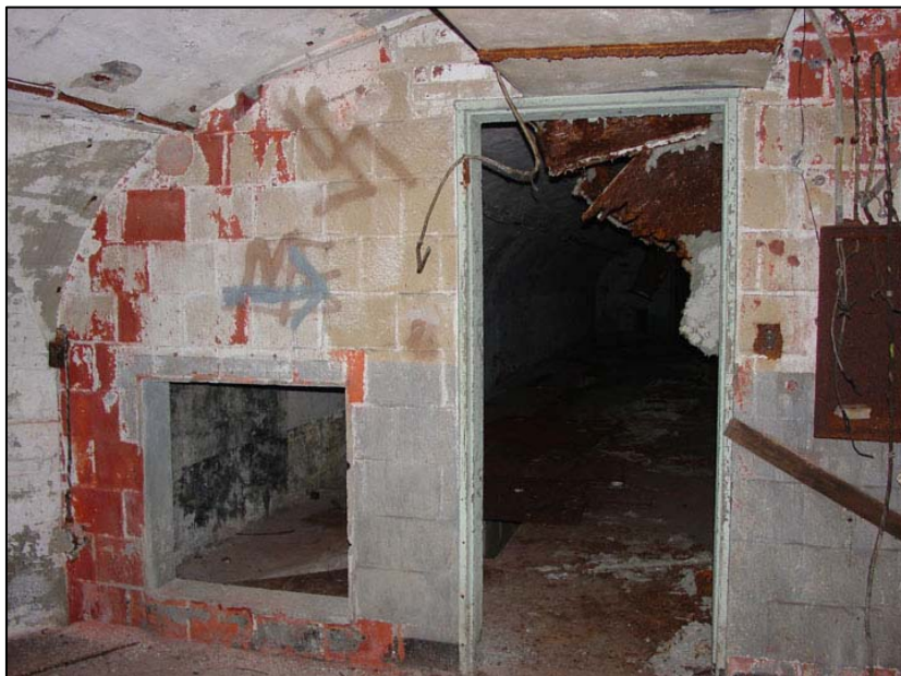
Figure 176. Mortar Battery, within Battery McCook, hollow-tile partition wall at north end of longitudinal gallery (room 112), 2006.
