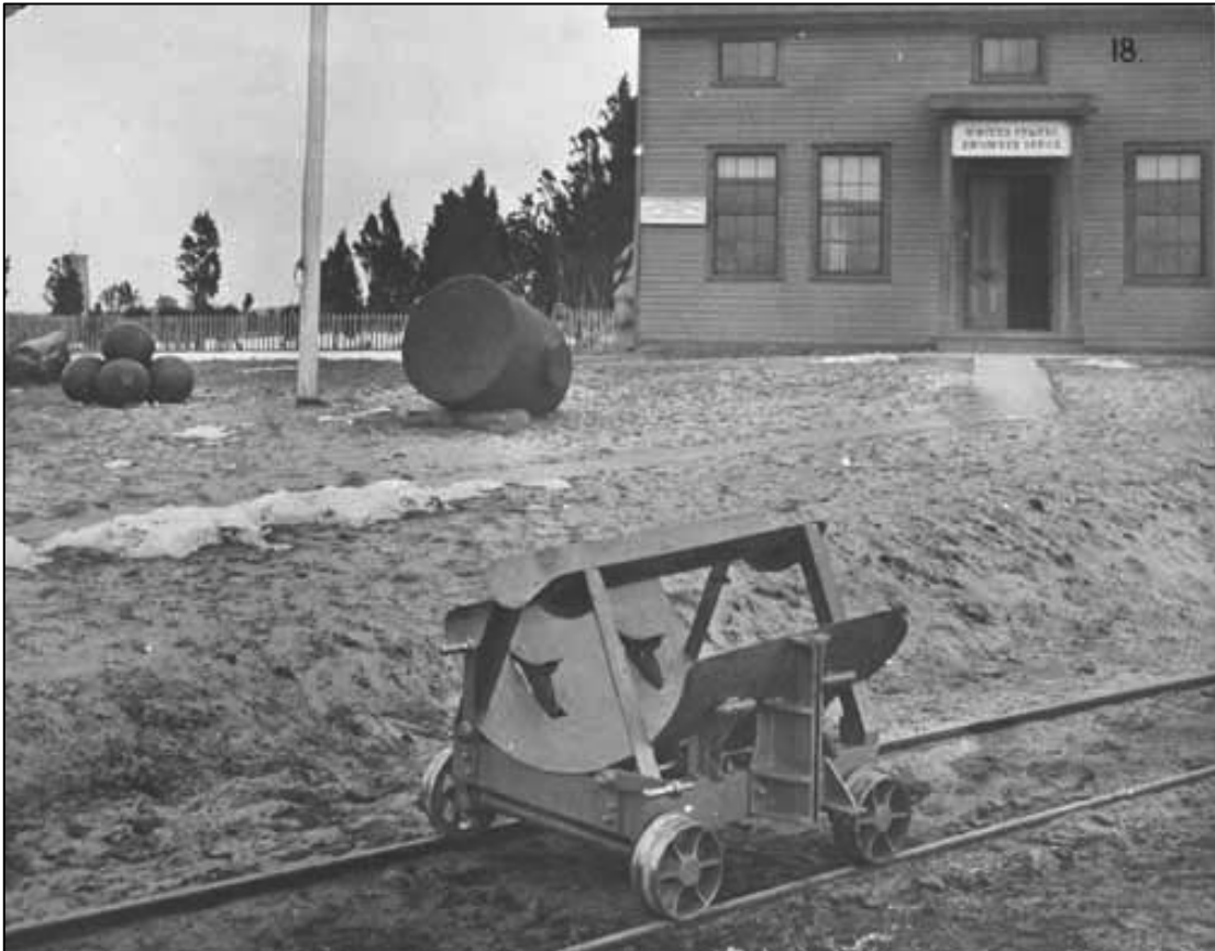
Figure 42. Battery Potter, carriage for ammunition hoist, Feb. 1893. Photograph no. 18 of 39 with F.Y. 1893 Annual Report.
