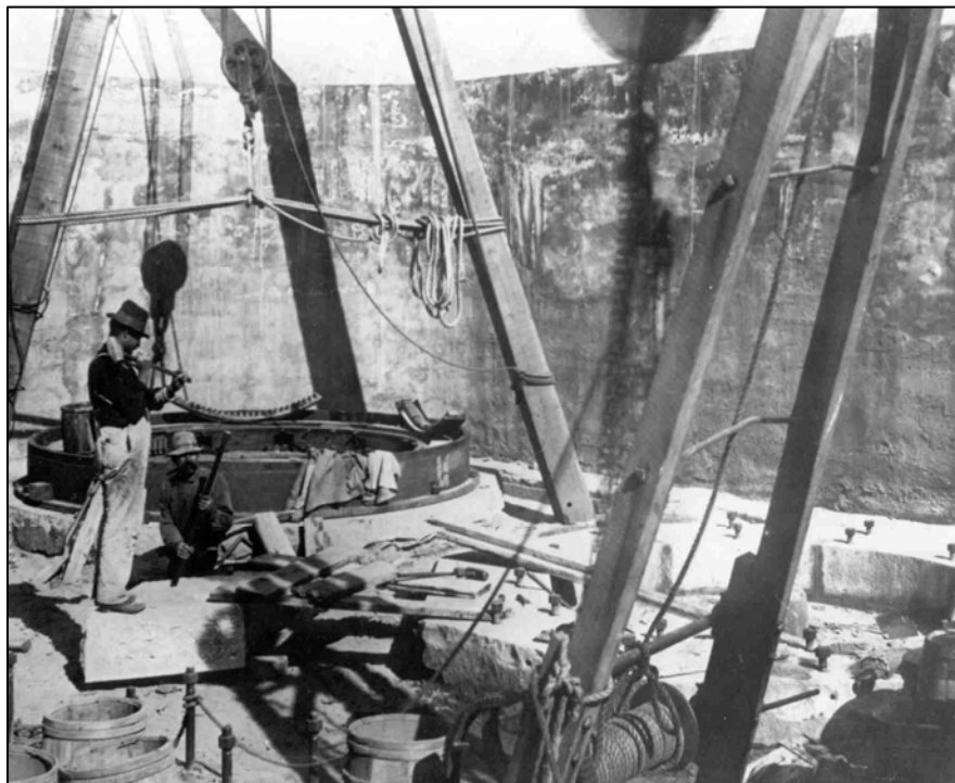
Figure 129. Mortar Battery, construction of mortar platforms; view shows granite base ring and steel roller path.
