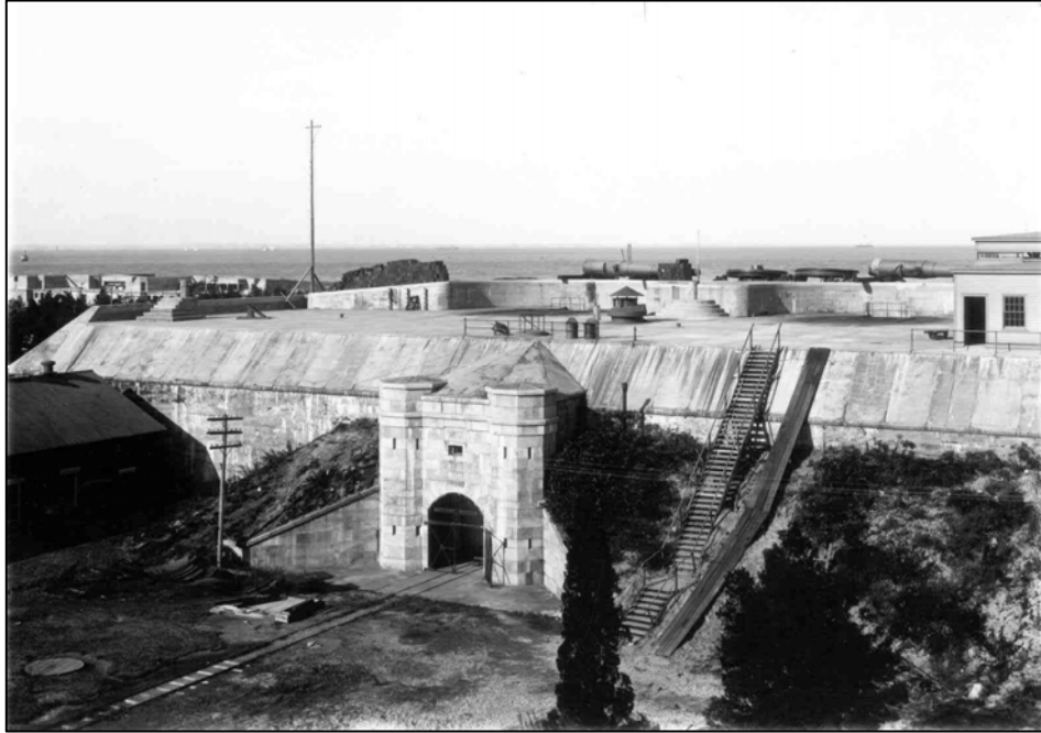
Figure 51. Battery Potter, west elevation and terreplein with 12-inch guns dismantled, circa 1906. Note range-finding platforms at northwest corner and at parapet wall.
