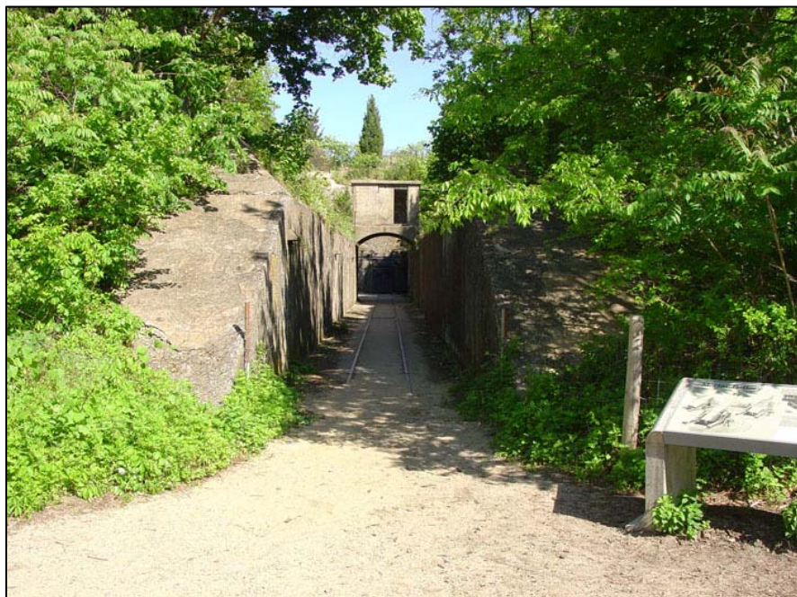
Figure 169. Mortar Battery, entrance gallery to southwest mortar pit, Battery Reynolds, 2006.
