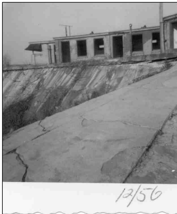
Figure 68. Primary fire-control stations on Battery Potter, Dec. 1956.
