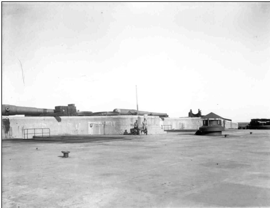
Figure 52. Battery Potter, terreplein with 12-inch guns and carriages dismantled, circa 1906. Note range-finding platform at parapet wall behind soldier on right.
