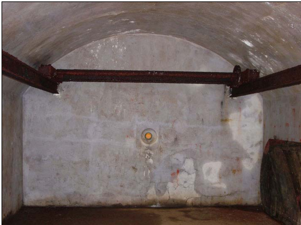
Figure 101. Battery Potter, interior view of north shell magazine (room 114), showing overhead trolley bridge for ammunition-delivery system, 2005.
