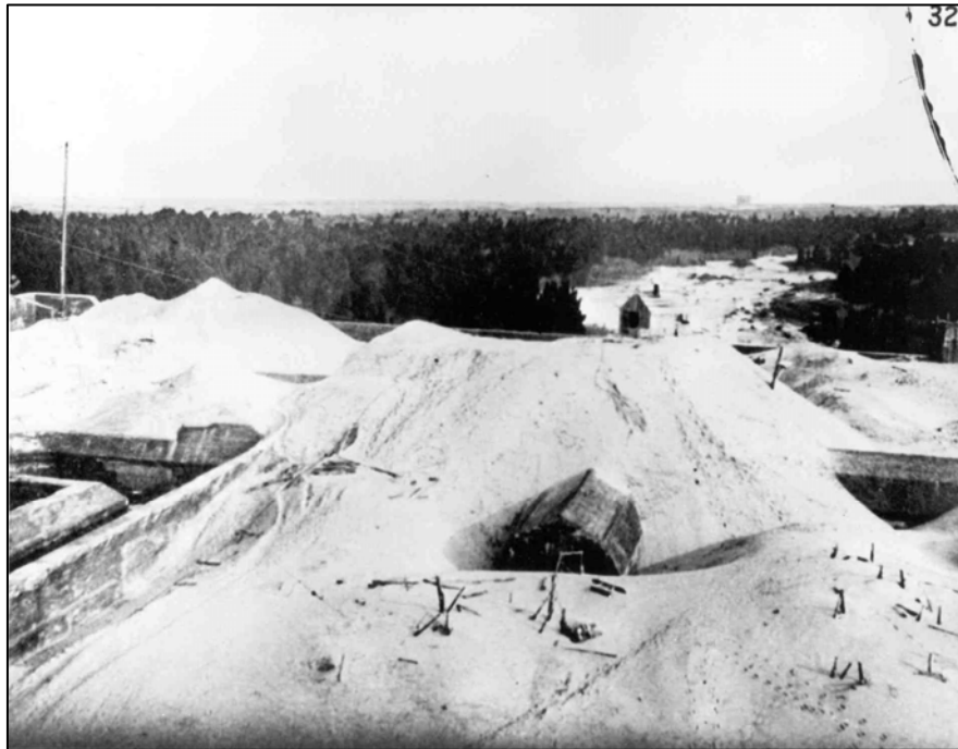
Figure 128. Mortar Battery, as seen from lighthouse, February 8, 1893; view shows covering of battery with sand.
