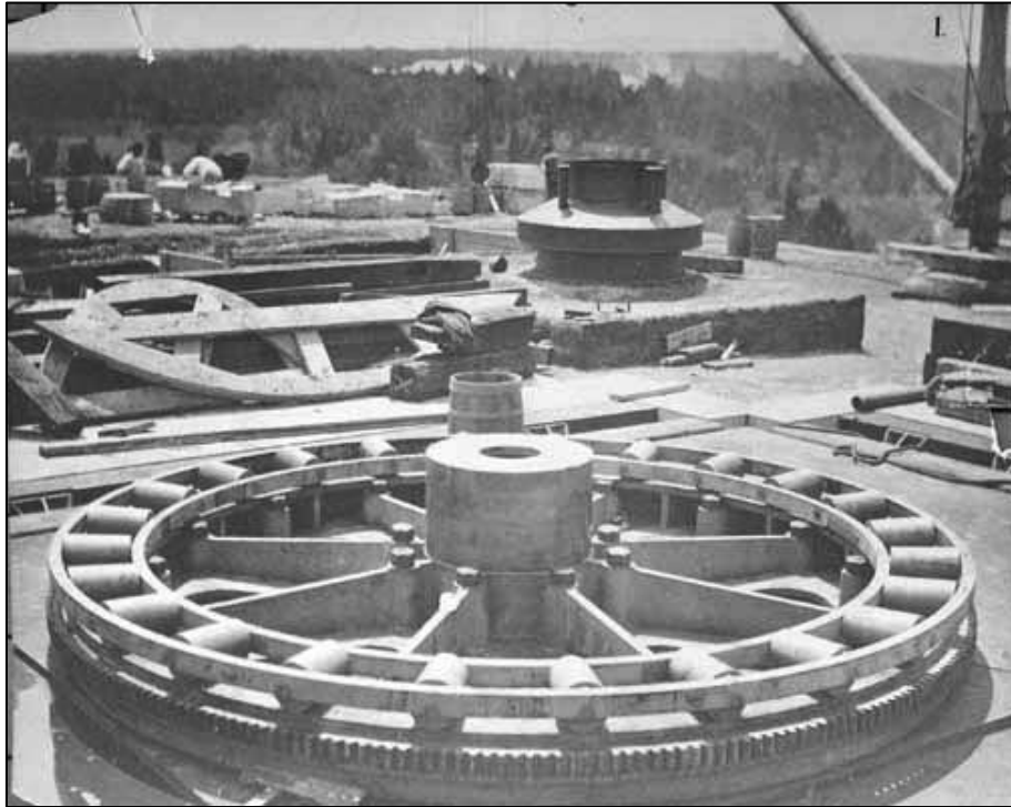
Figure 34. Battery Potter, Schneider & Co. gun carriage, pintle plate, and traversing circle. Photograph no. 1 of 39 with F.Y. 1893 Annual Report.
