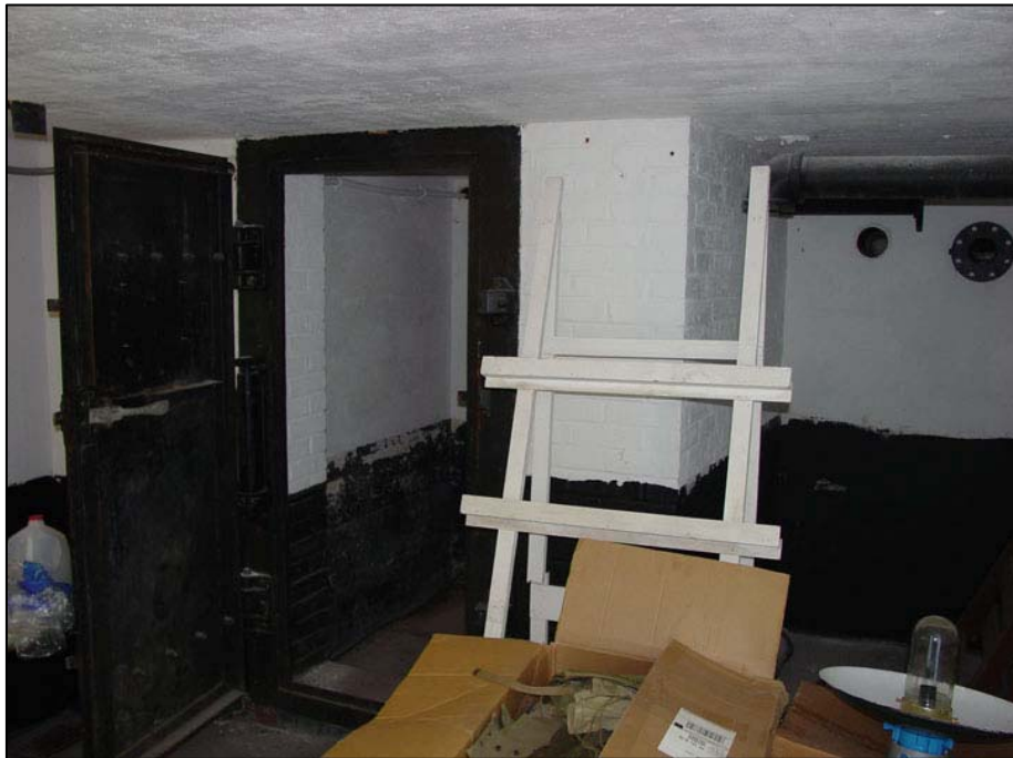
Figure 214. Battery Gunnison, 1943 air lock in storage room (room 101) for chemical-weapons service equipment, 2006.
