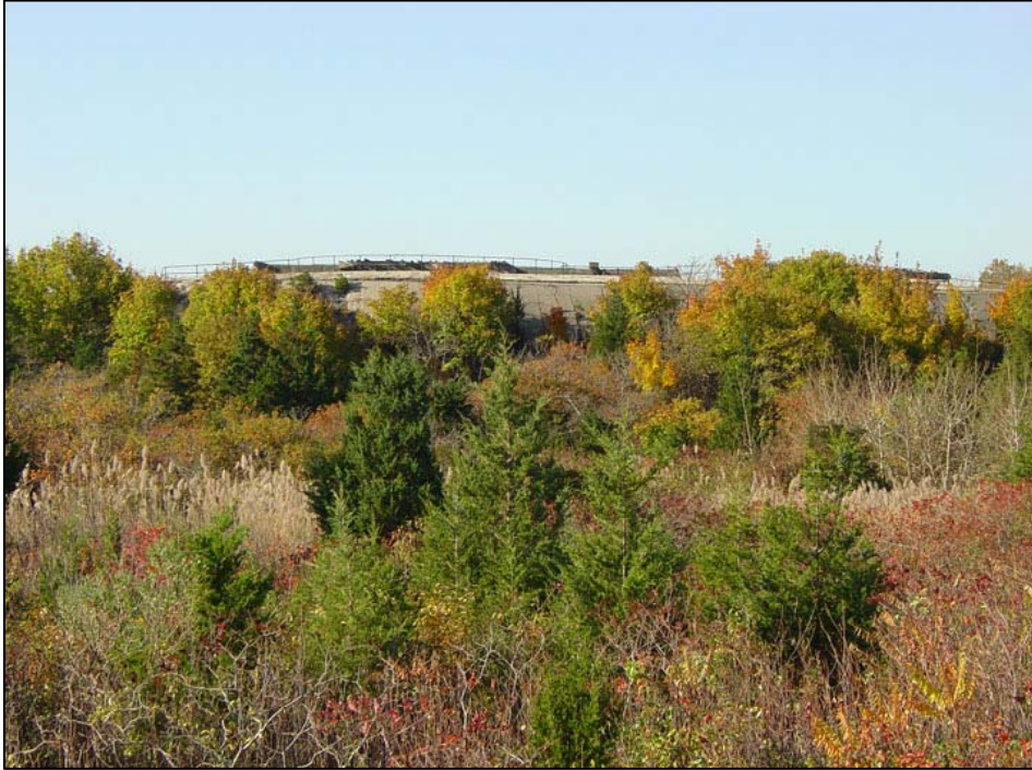
Figure 76. Battery Potter, view of east elevation, 2005.
