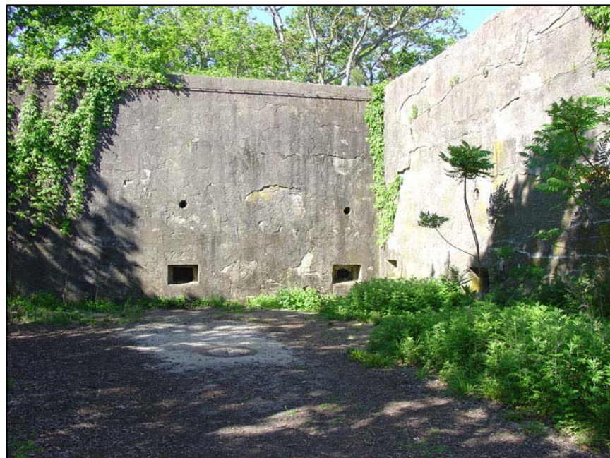
Figure 166. Mortar Battery, view of counterscarp wall interior and southwest counterscarp gallery, 2006.
