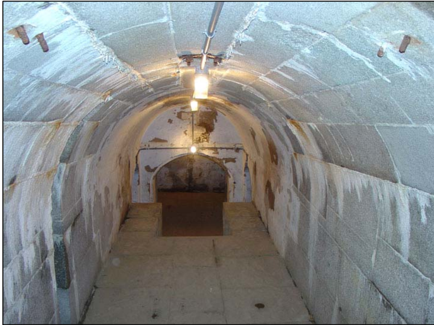
Figure 90. Battery Potter, interior view of north loading gallery (room 209), looking west toward concrete steps, 2006.
