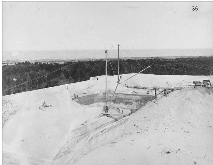
Figure 120. Construction of concrete slopes around the two northern pits, May 1, 1893.
