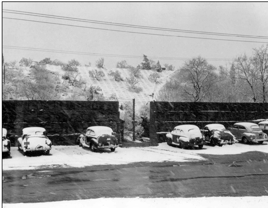
Figure 152. Mortar Battery, opening in countescarp wall, ca. 1944.
