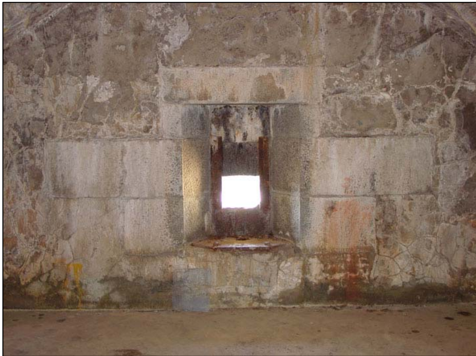
Figure 95. Battery Potter, view of second story of defensible entrance (room 201), gun port in west wall, 2006.
