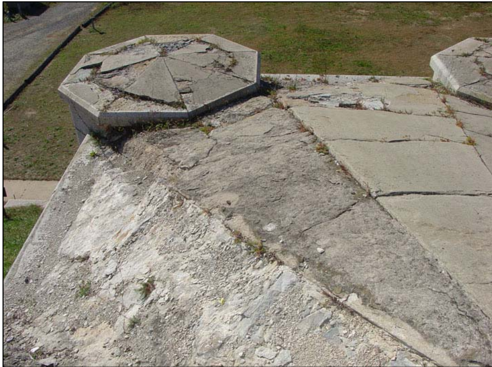
Figure 79. Battery Potter, roof of defensible entrance, 2005.
