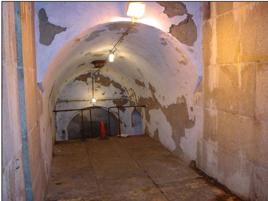
Figure 91. Battery Potter, interior view of south loading gallery (room 213), looking west toward cast-iron ladder, 2006.
