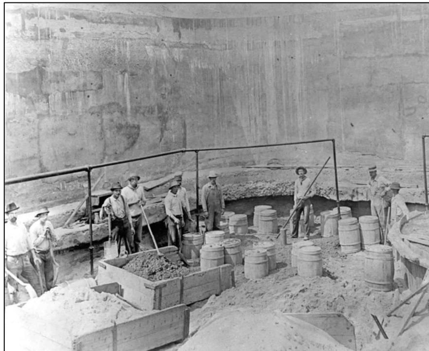
Figure 121. Mortar Battery, excavation and construction of foundations for mortar emplacements; note inverted cement barrels protecting bolt locations.
