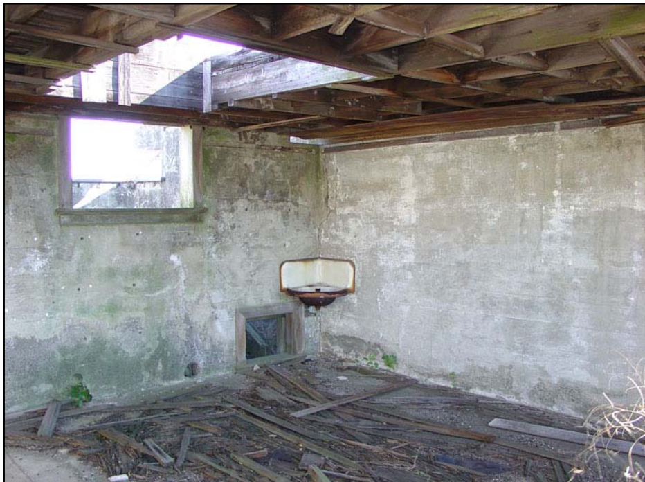
Figure 107. Battery Potter, typical primary fire-control station, showing interior of plotting room and interior partition, 2005.
