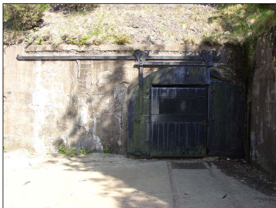
Figure 174. Mortar Battery, doorway and altered steel door from southwest mortar pit to transverse gallery, 2006.
