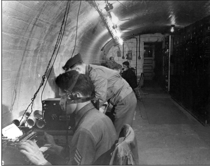
Figure 154. Mortar Battery, switchboard room (room 112), ca. 1941.
