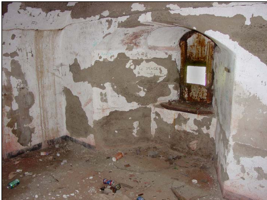
Figure 168. Mortar Battery, interior view of gun port embrasure in southwest counterscarp gallery, 2006.
