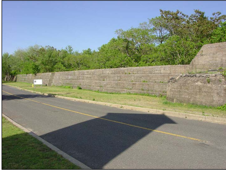
Figure 165. Mortar Battery, exterior view of west side of counterscarp wall, 2006.
