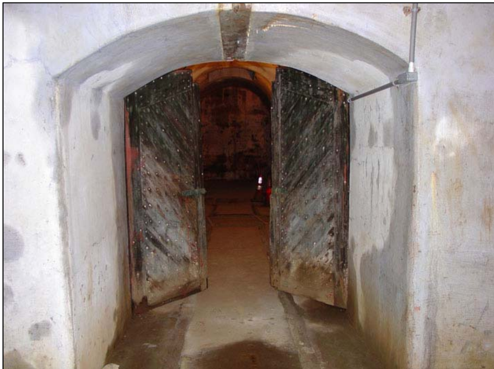
Figure 93. Battery Potter, interior view of doorway to north magazine gallery (room 113), looking east, 2006.
