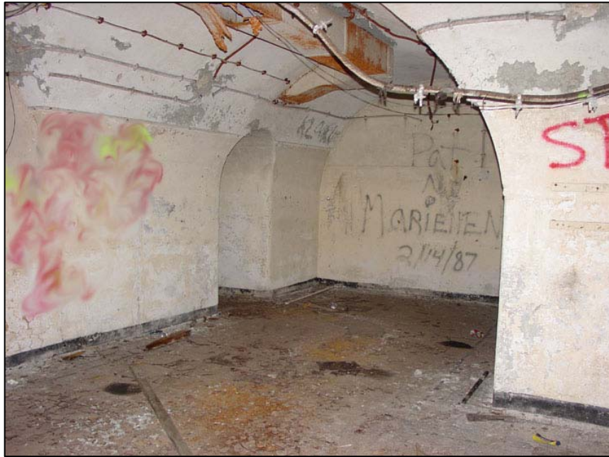
Figure 177. Mortar Battery, within Battery McCook, corridor and storage area (room 113), 2006.
