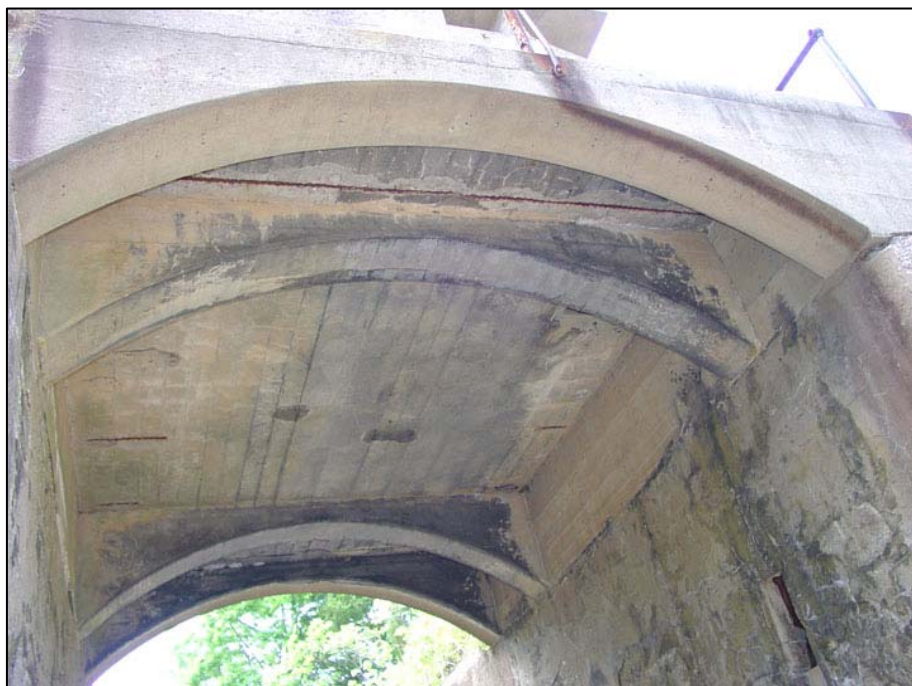
Figure 183. Mortar Battery, supporting arches of telephone booth at southwest mortar pit, Battery Reynolds, 2006.
