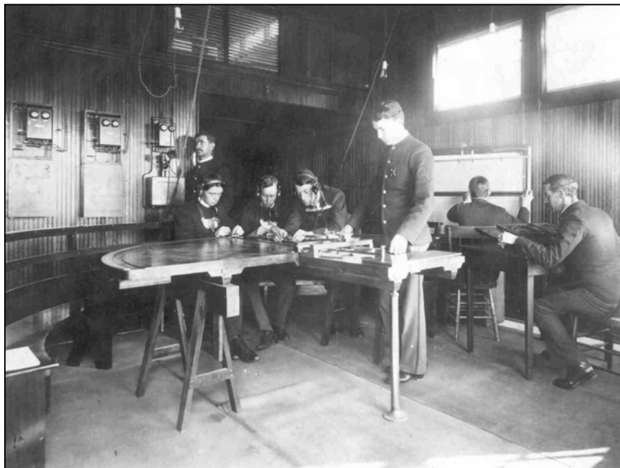
Figure 64. Battery Potter, interior of plotting room of one of two primary fire-control stations for Mortar Battery, circa 1907.
