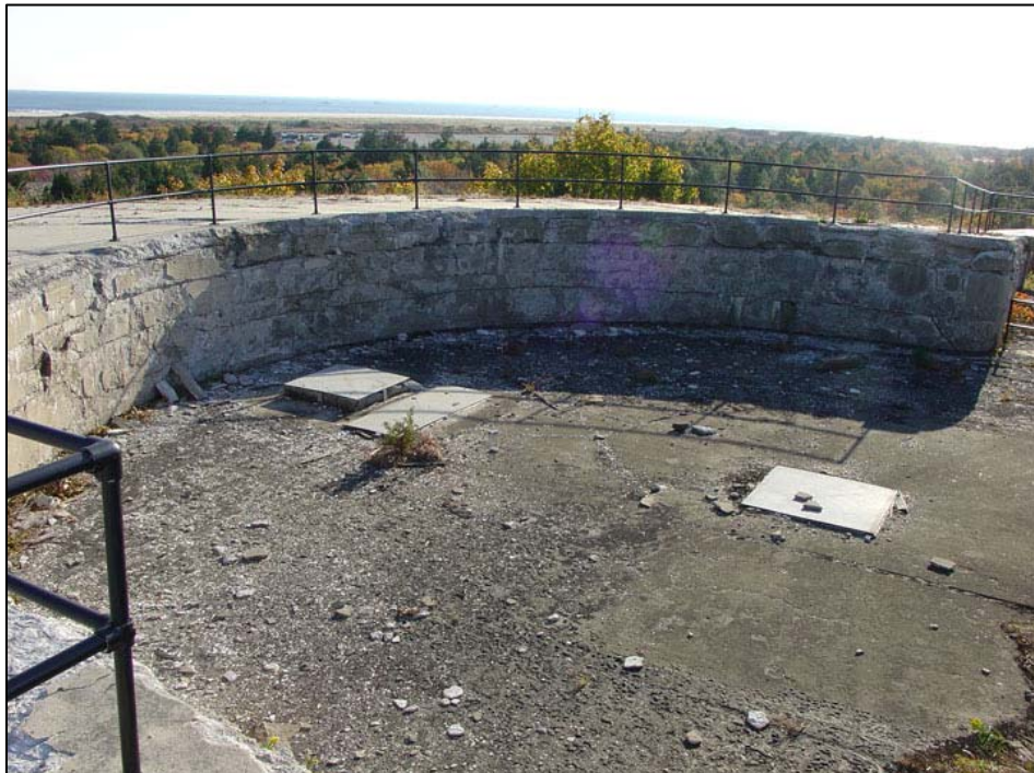
Figure 81. Battery Potter, south gun parapet, 2005.
