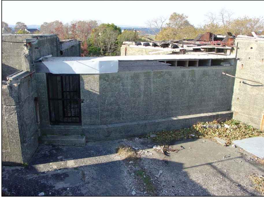
Figure 104. Battery Potter, east elevation of bulkhead (room 315) covering stairway (room 220) that connected second story with terreplein and primary fire-control stations, 2005.
