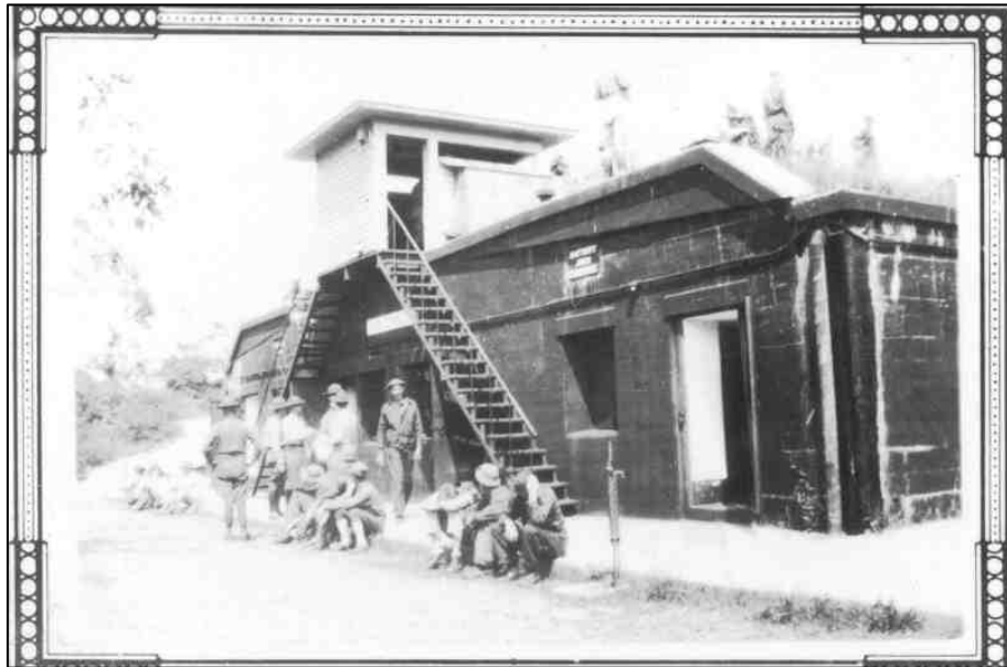
Figure 193. Battery Gunnison, view of west elevation of traverse and battery commander station, ca. 1930.
