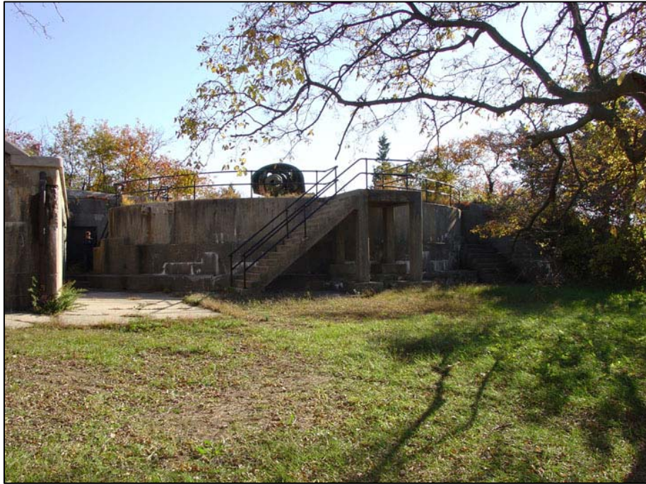
Figure 205. Battery Gunnison, view of south emplacement, looking east, 2006. Note doorway to powder passage, located between traverse (at left) and emplacement (at right).
