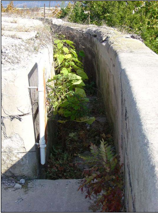
Figure 84. Battery Potter, southeast section of chemin de ronde , 2005.
