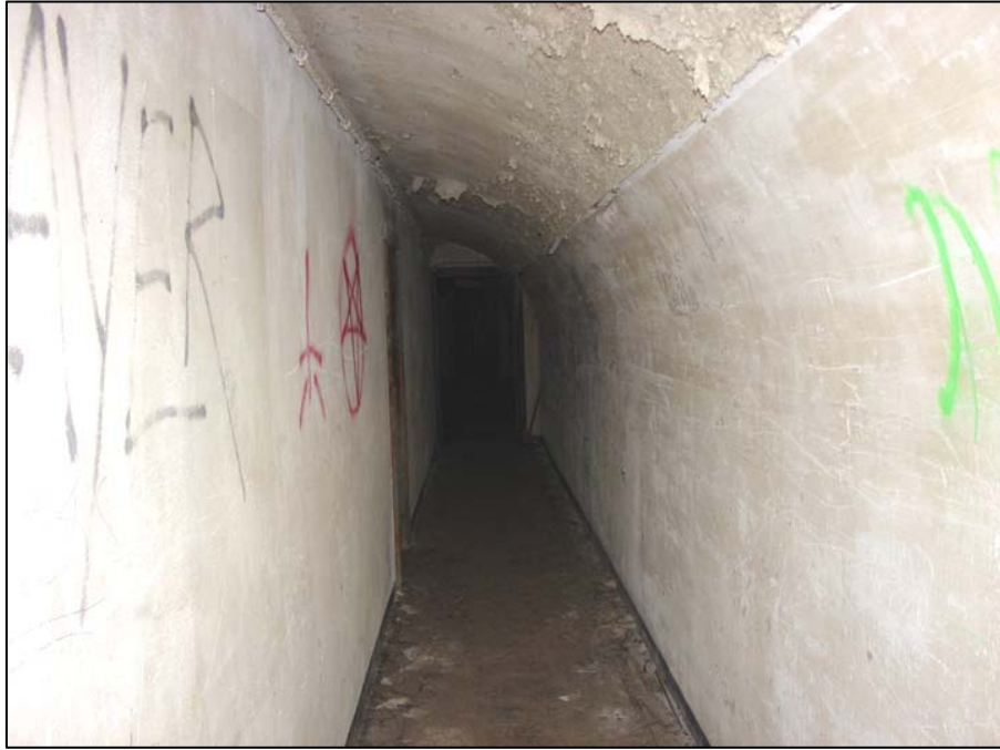
Figure 179. Mortar Battery, within Battery Reynolds, south end of longitudinal gallery (room 126), 2006.
