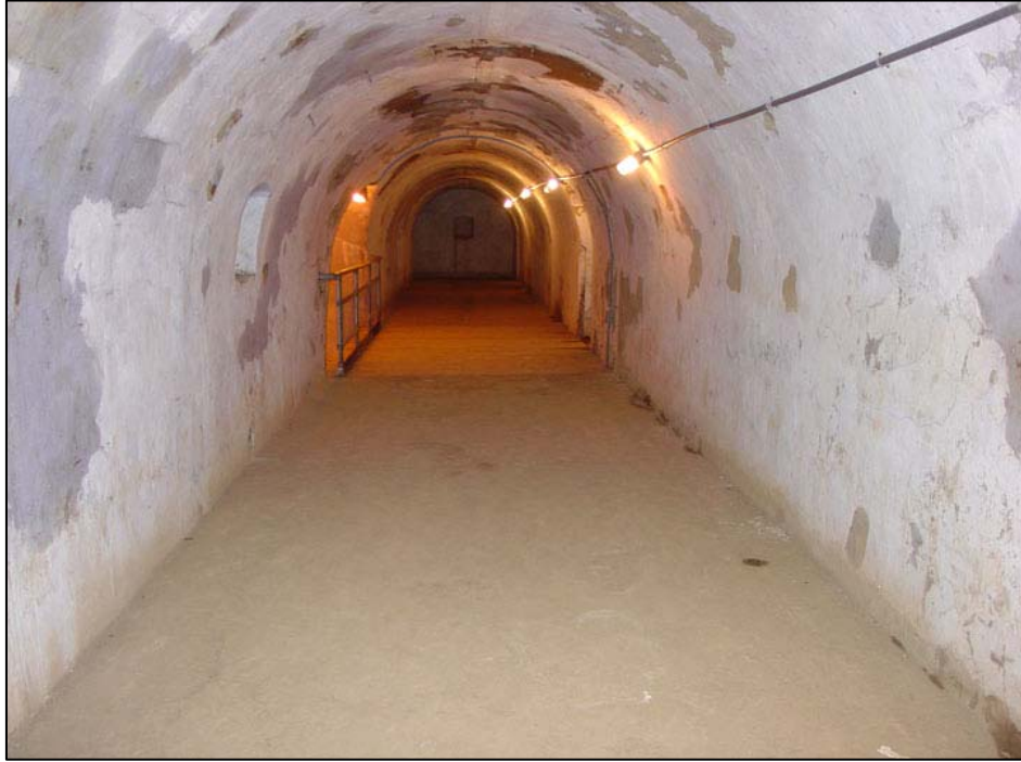
Figure 88. Battery Potter, interior view of second-story north and south transverse galleries (rooms 203 and 205), and wooden bridge connecting them (room 204), 2006.
