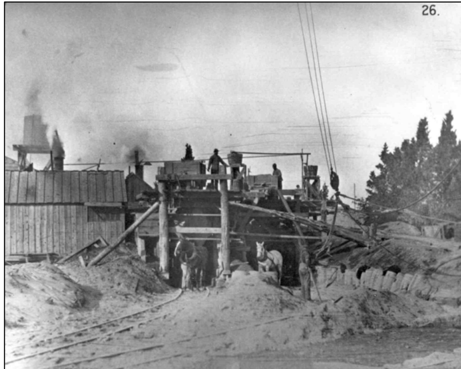
Figure 114. Concrete mixers in operation at Mortar Battery plant, Nov. 14, 1892.
