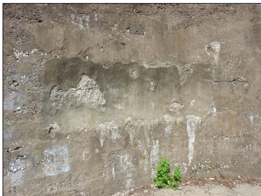
Figure 172. Mortar Battery, section of wall in mortar pit with rounded indentation to allow for swing of gun barrel, 2006.
