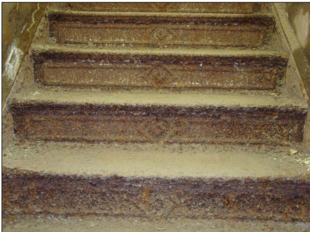
Figure 97. Battery Potter, view of existing condition of iron steps of south stairway (room 108) connecting first and second stories, 2006.
