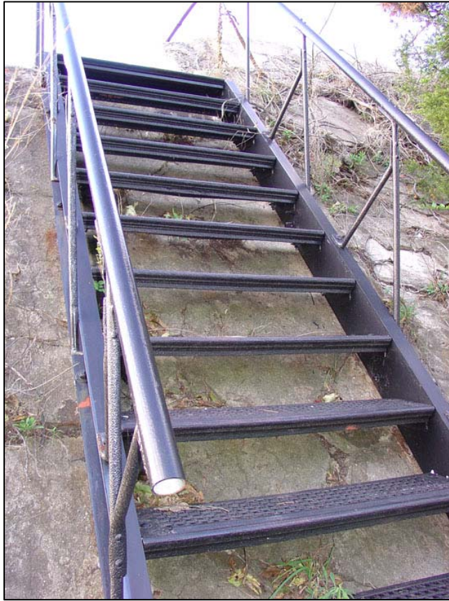
Figure 78. Battery Potter, exterior iron stairway, upper flight, 2005.
