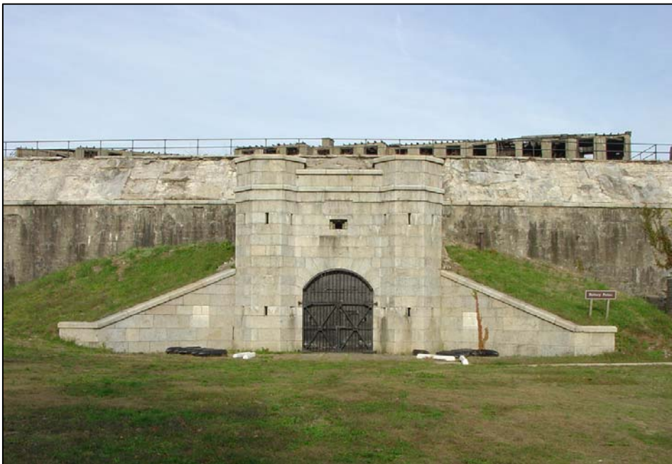
Figure 77. Battery Potter, view of west elevation, 2005.
