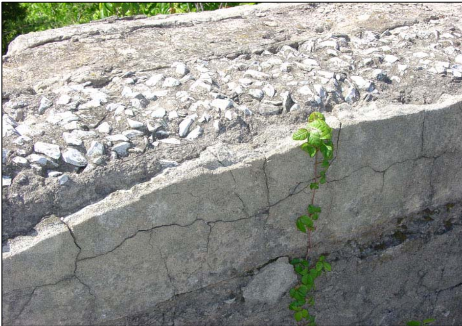
Figure 85. Battery Potter, parapet wall of chemin de ronde , 2005.
