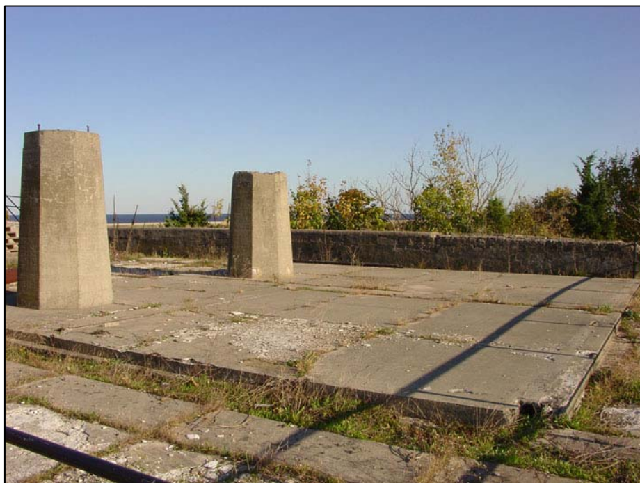
Figure 82. Battery Potter, view to the southwest, showing terreplein and extant elements of missing fire-control stations for Mortar Battery, 2005.
