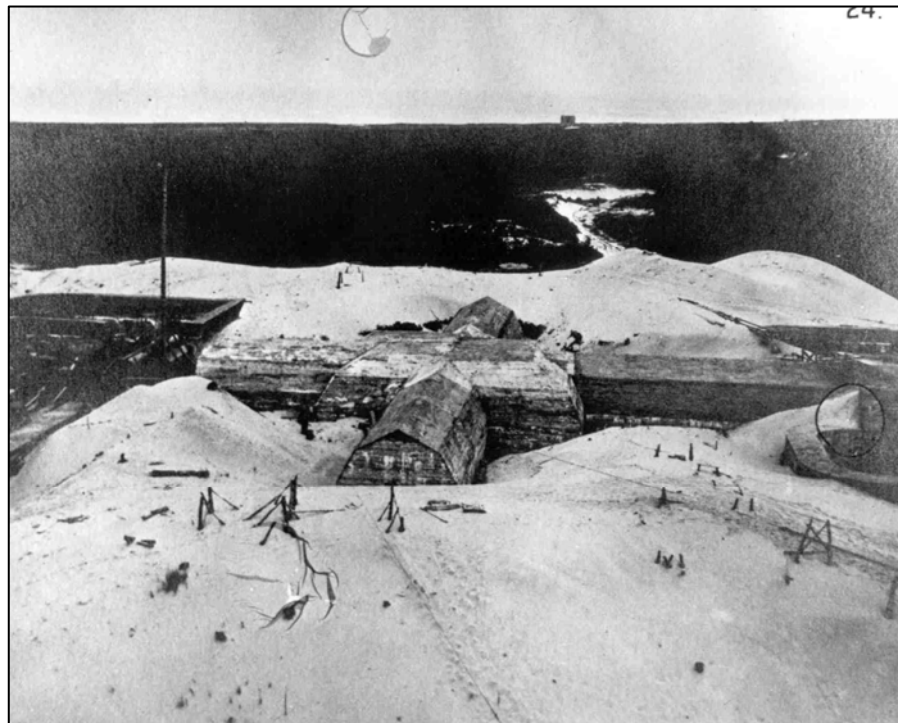
Figure 115. Mortar Battery, as seen from lighthouse, June 7, 1892.
