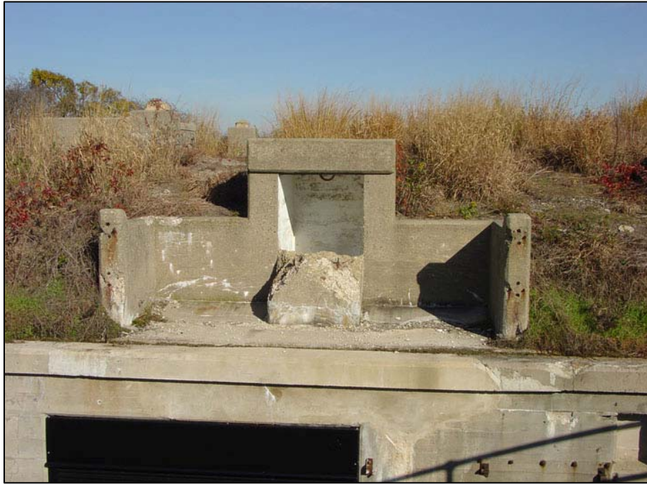
Figure 213. Battery Gunnison, 1943 shell-hoist shed for south emplacement, 2006.
