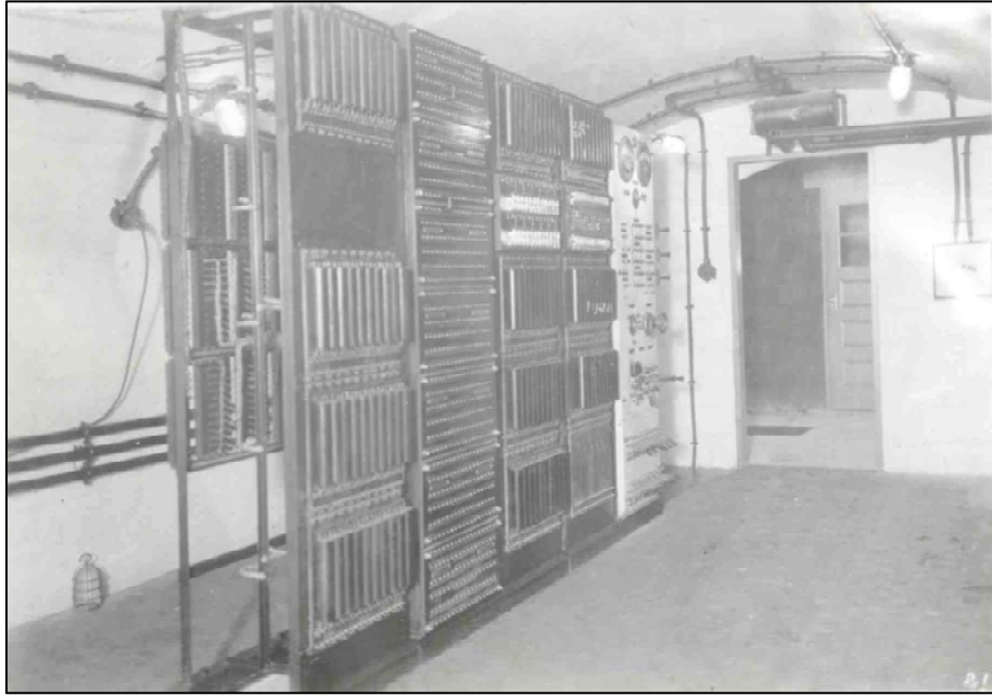
Figure 151. Mortar Battery, interior of switchboard room, ca. 1922.
