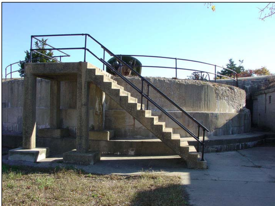
Figure 206. Battery Gunnison, view of north emplacement retaining wall and west stairway, looking east, 2006.
