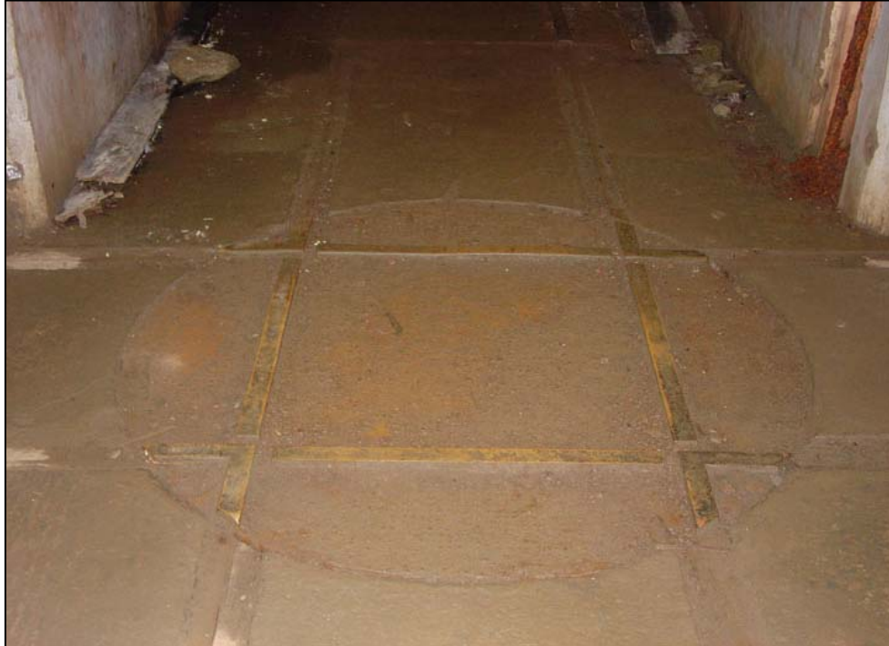
Figure 100. Battery Potter, view of south magazine gallery (room 116), showing gun-metal turntable for ammunition-delivery system, 2006.
