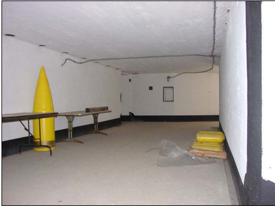
Figure 217. Battery Gunnison, shell room (room 105), looking southeast, 2006.
