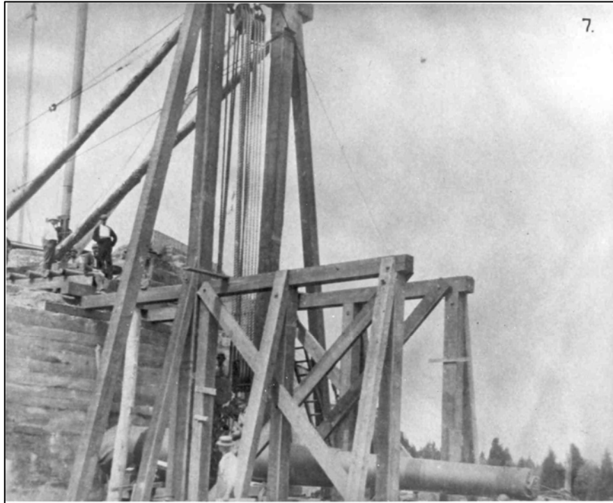
Figure 37. Battery Potter, raising 12-inch B.L. rifle. Photograph no. 7 of 39 with F.Y. 1893 Annual Report.
