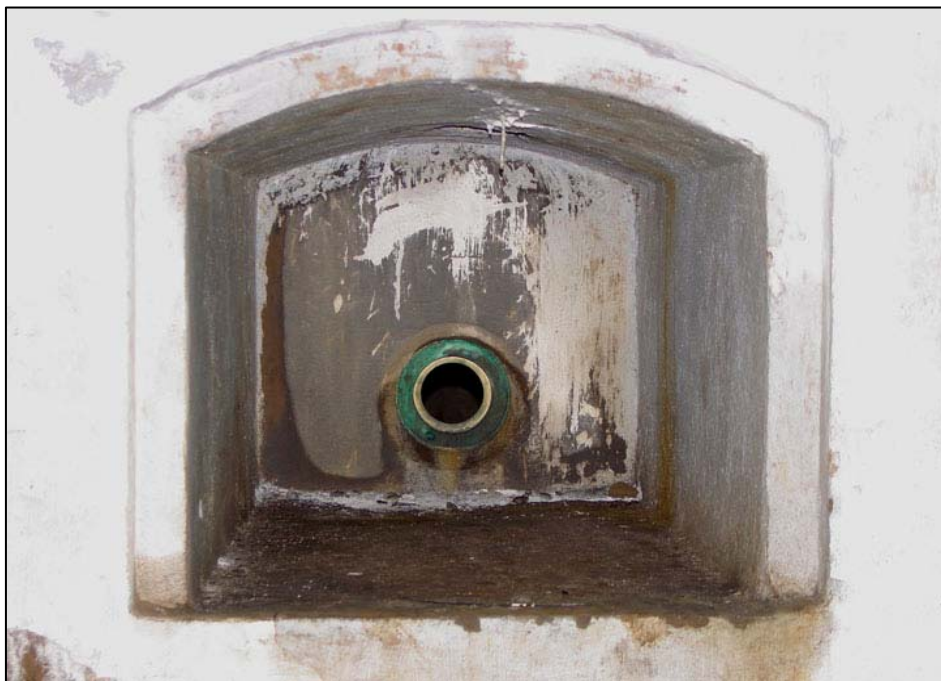
Figure 89. Battery Potter, interior view of niche in wall of transverse gallery for auxiliary lantern lighting system, 2005.
