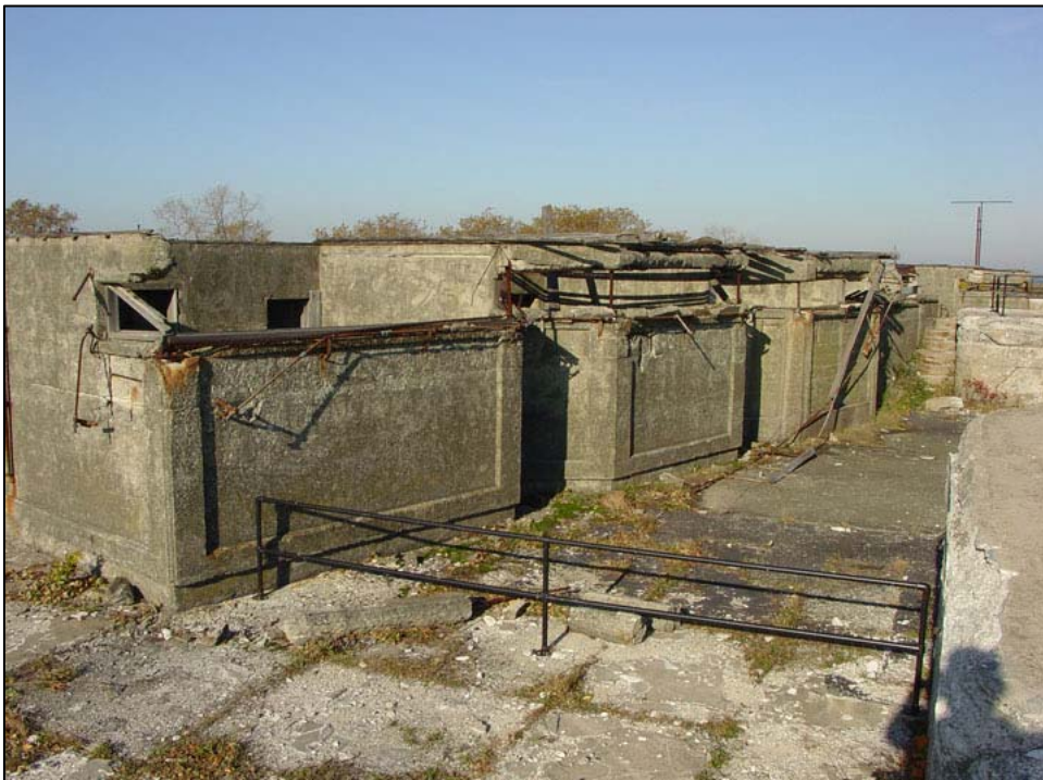
Figure 103. Battery Potter, primary fire-control stations, east elevation of the east rooms (rooms 309, 311, 313) of the three southernmost stations, 2005.
