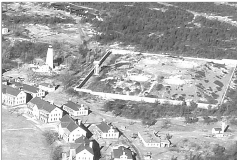
Figure 142. Detail of aerial photograph of Fort Hancock, ca. 1930: view of Mortar Battery, showing tower and station inside west counterscarp wall.
