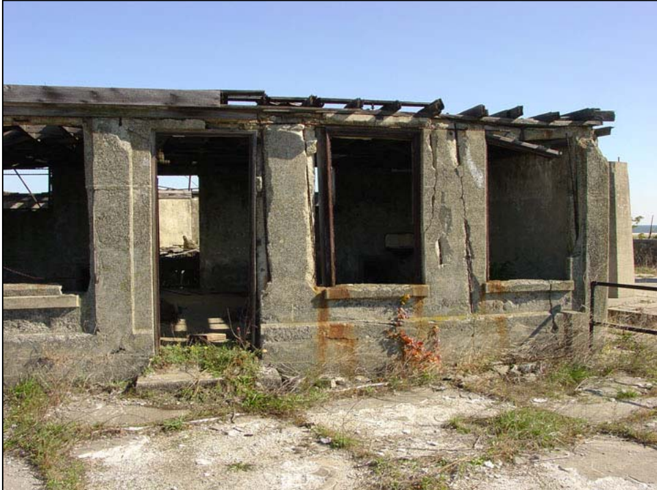
Figure 102. Battery Potter, primary fire-control stations, west elevation of southernmost station (rooms 313 and 314), 2005.
