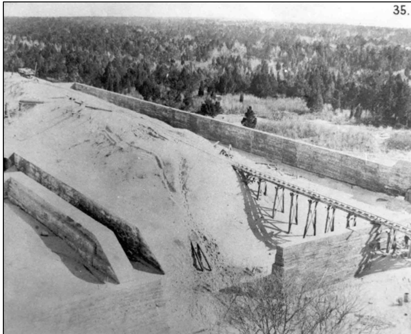
Figure 131. South end of Mortar Battery, as seen from lighthouse, March 13, 1893; view shows counterscarp wall and trestle over wall during construction.
