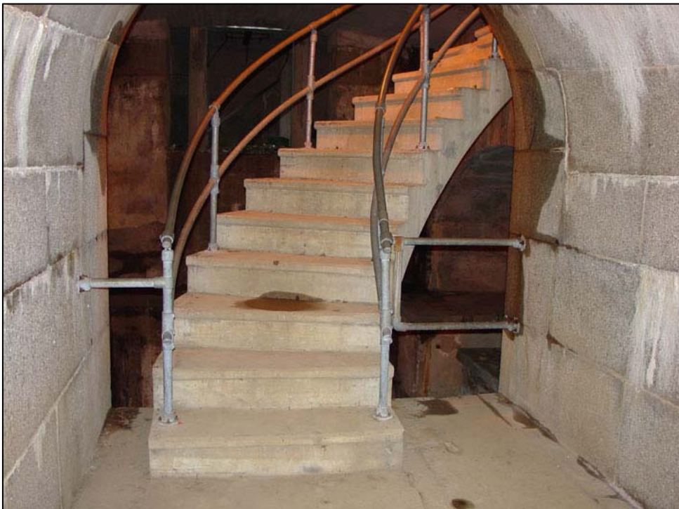
Figure 99. Battery Potter, view of concrete stairway (room 220) connecting north loading gallery (room 209) and terreplein, 2006.
