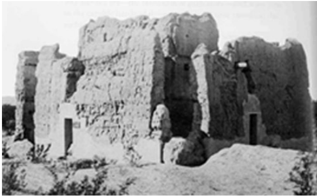
Casa Grande after initial basal stabilization
