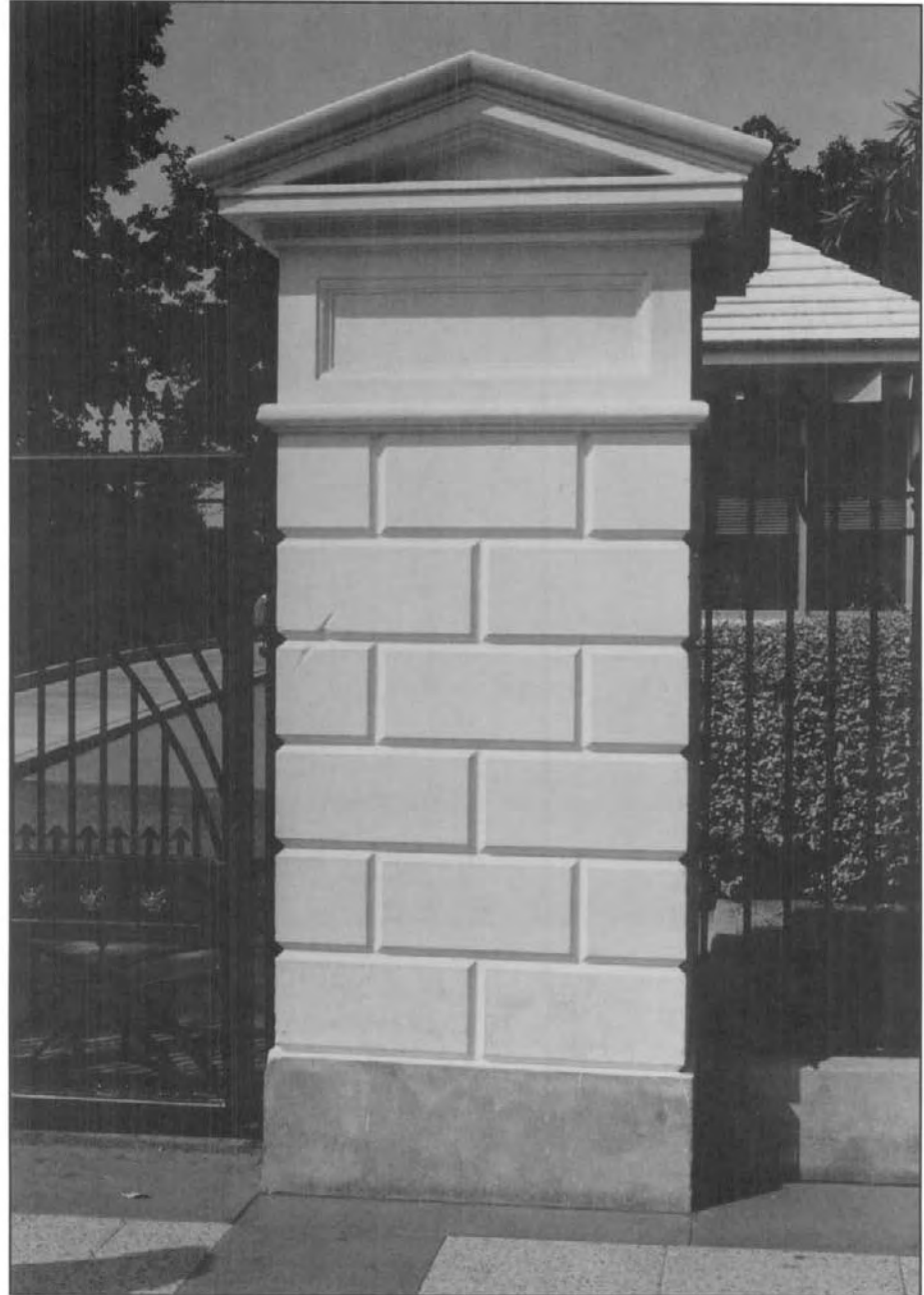
White House, Gatepost Detail
