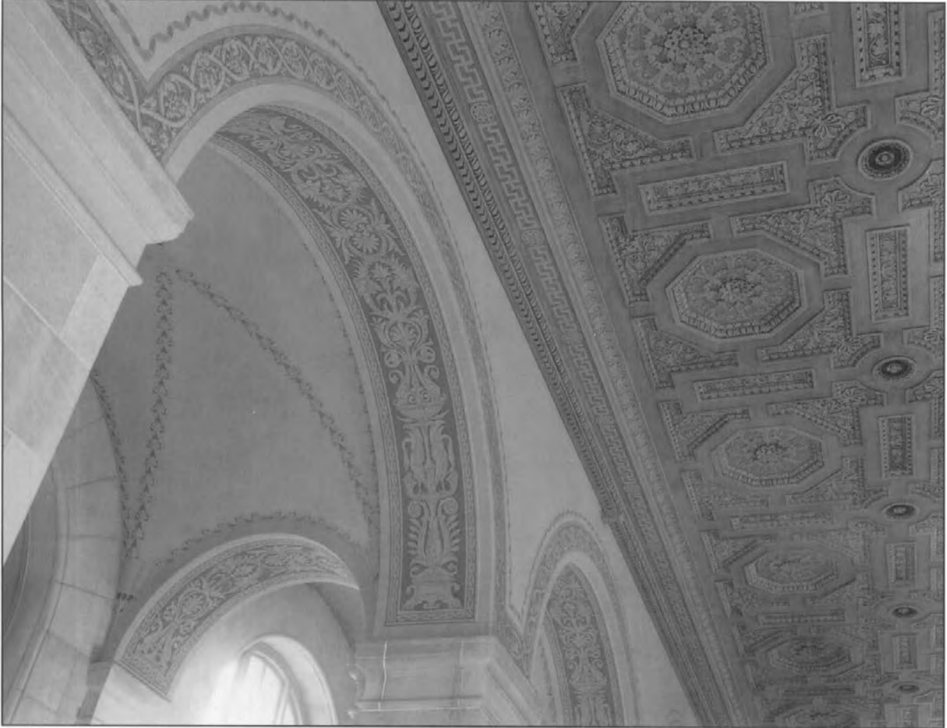
U.S. Department of Commerce Building, Baldrige Hall, Interior Arch and Ceiling Detail
