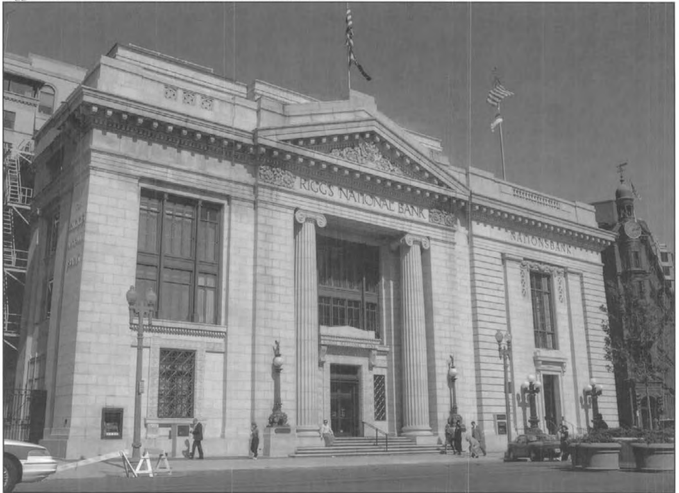
Riggs National Bank and NationsBank, South Elevation
