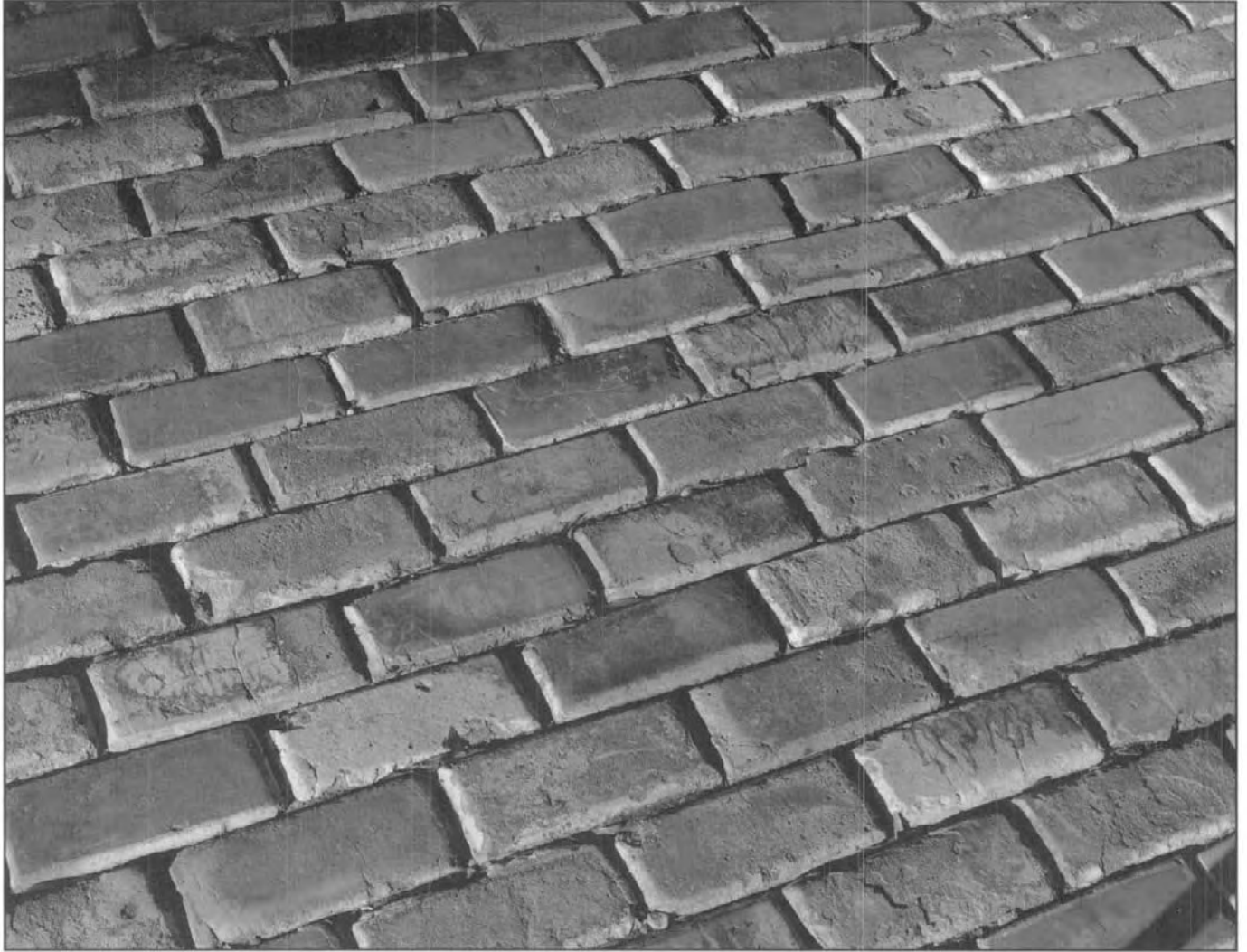
U.S. Treasury Building, Belgian Block Paver Detail
