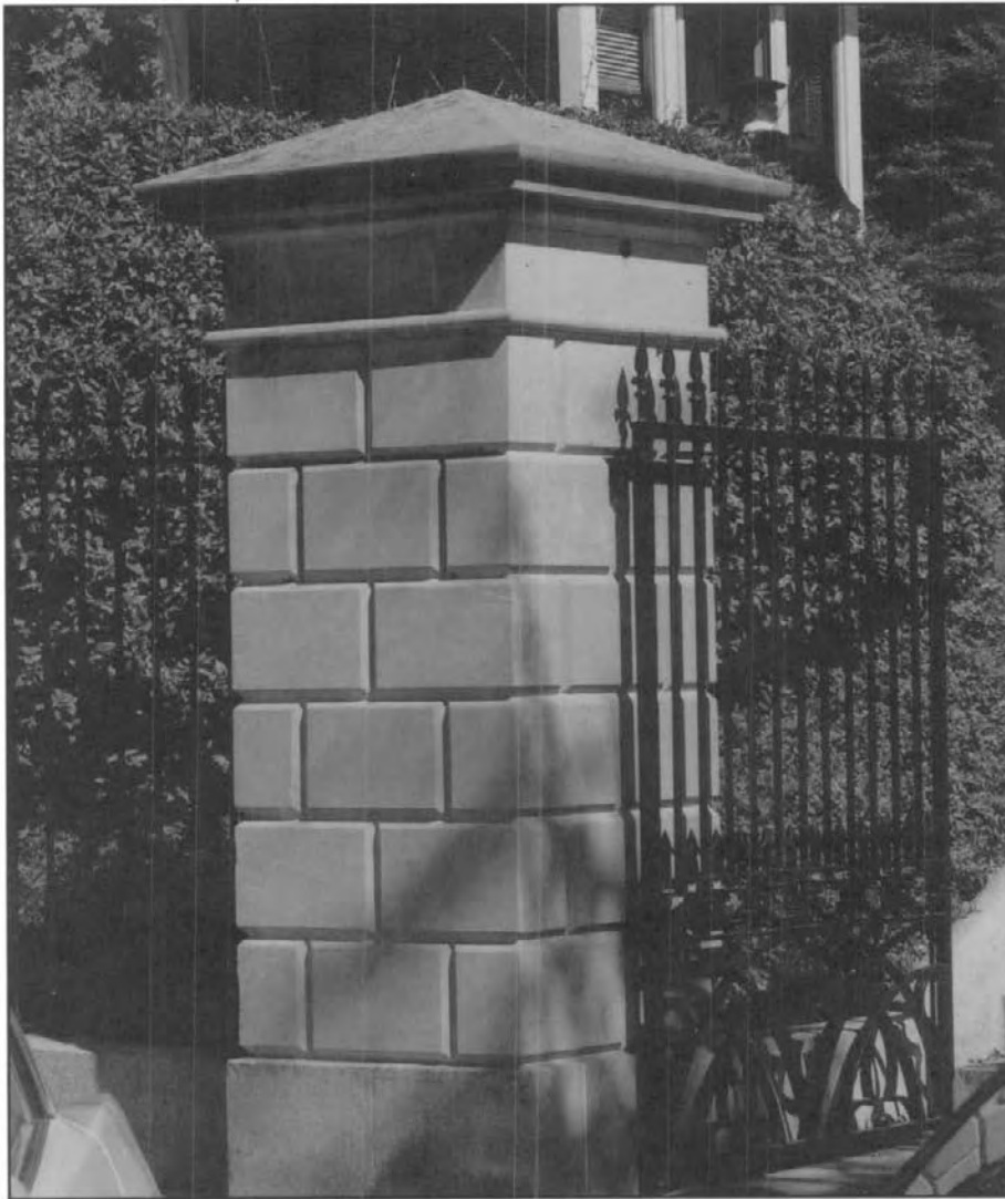
White House, Gatepost Detail
