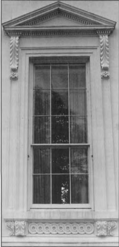
White House, First-Floor Window Detail
