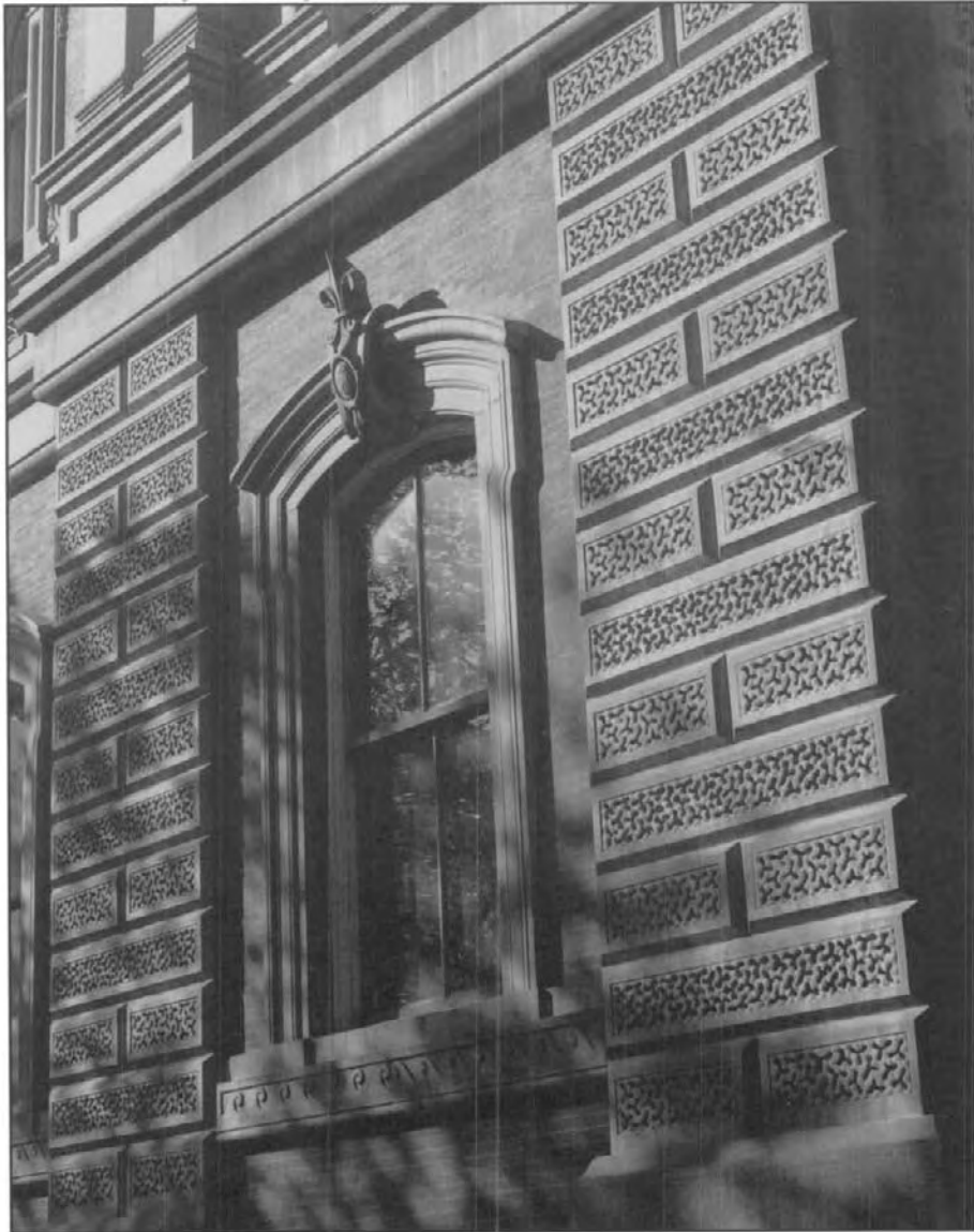
Renwick Gallery, Masonry Detail
