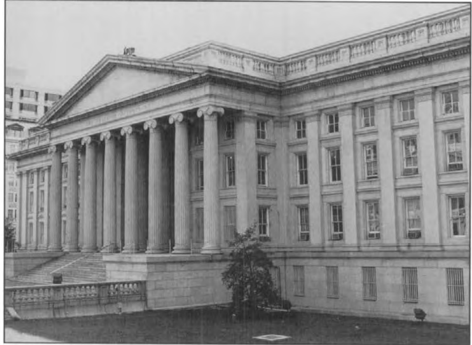
U.S. Treasury Building, North Elevation
