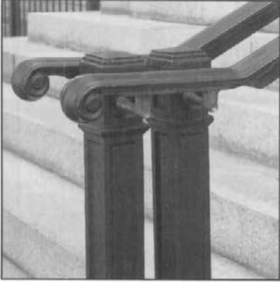
Old Executive Office Building, North Terrace
