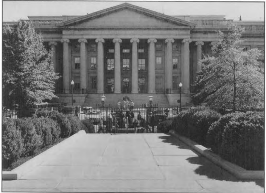
U.S. Treasury Building, West Elevation
