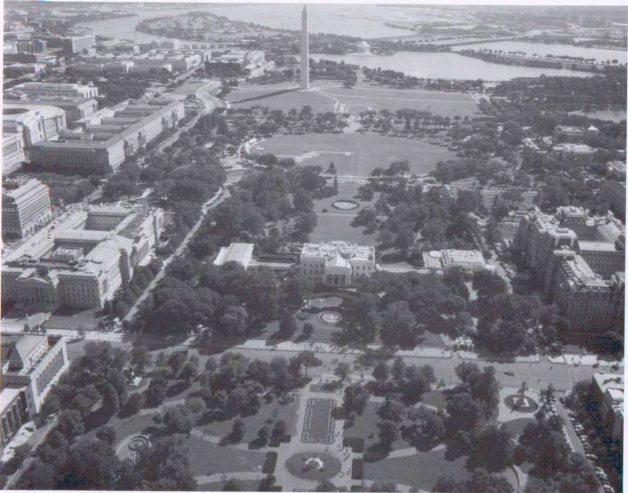
An aerial view of Lafayette Park, the White House, and the Ellipse shows the importance of north/south views, which L'Enfant emphasized in his plan for Washington.
