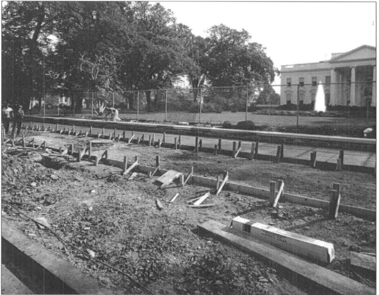
Figure 7-15: Reconstruction of Fence and Sidewalk, Pennsylvania Avenue . Abbie Rowe (photograph), 1965. From White House Fences and Construction . National Park Service, Office of White House Liaison.
