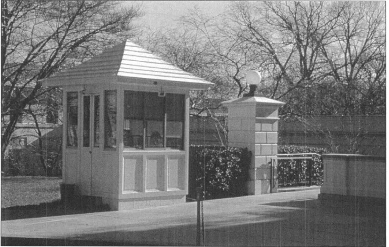
Figure 9-3: Guardhouse Northeast of the White House.
