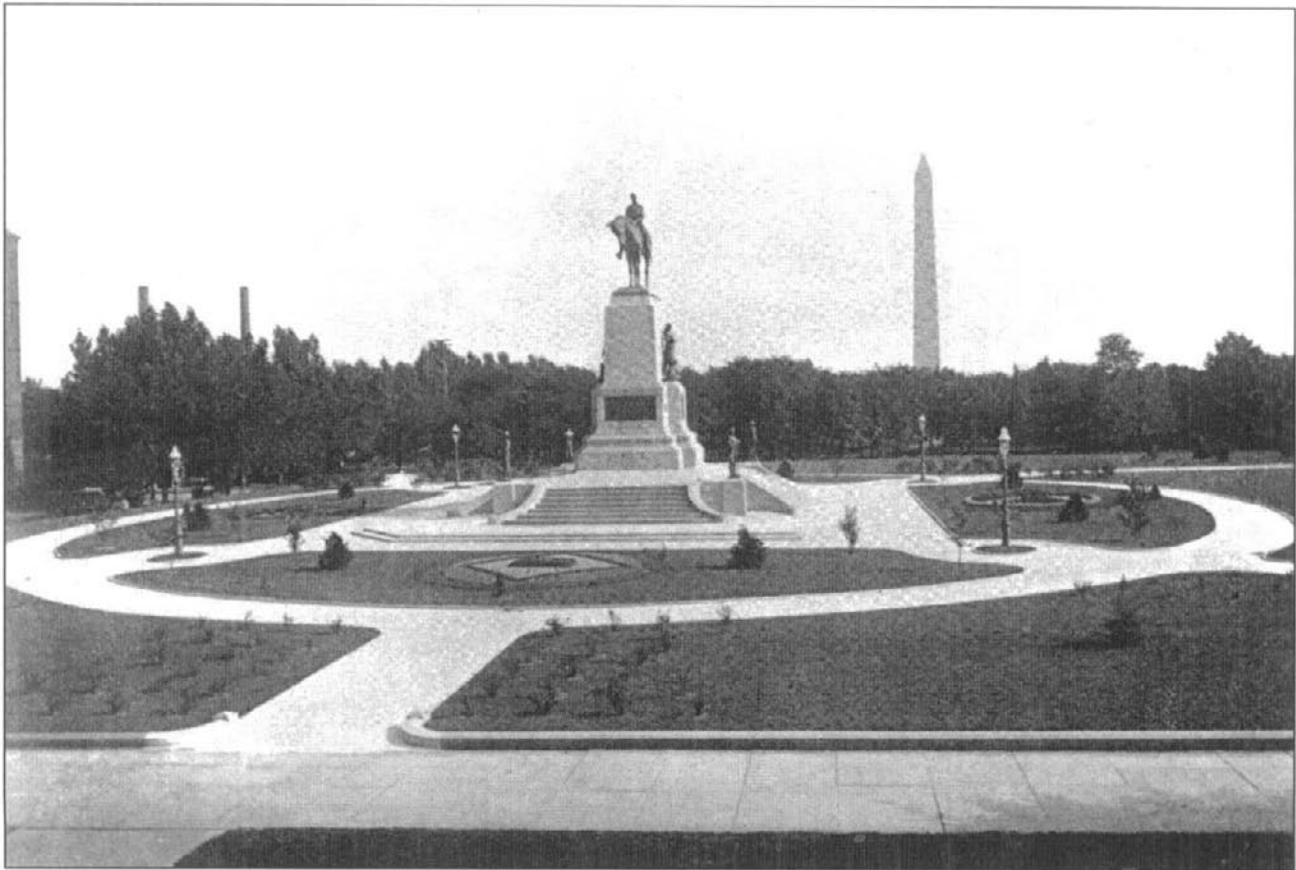
Figure 5-16: Sherman Plaza Showing Landscape Gardening Treatment (view from the Treasury steps, looking south) . Corps of Engineers, Annual Report (photograph), 1905. National Archives, Archives Library Information Center.
