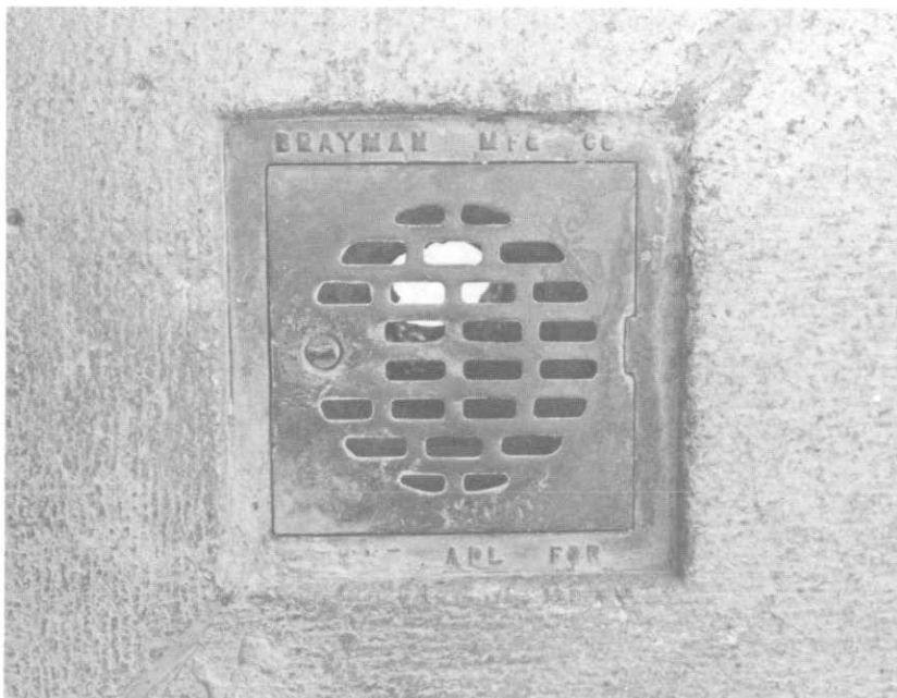
ILLUSTRATION 75. Detail of drain in southwest corner of observation gallery.
