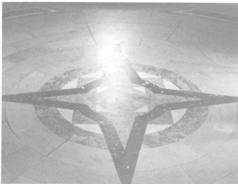
ILLUSTRATION 178. Detail view of decorative marble inlay of rotunda floor.
