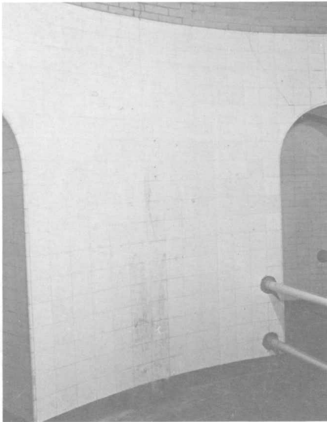
ILLUSTRATION 63. View of typical glazed tile walls, quarry tile floor and bronze handrails at north wall of lower elevator landing.
