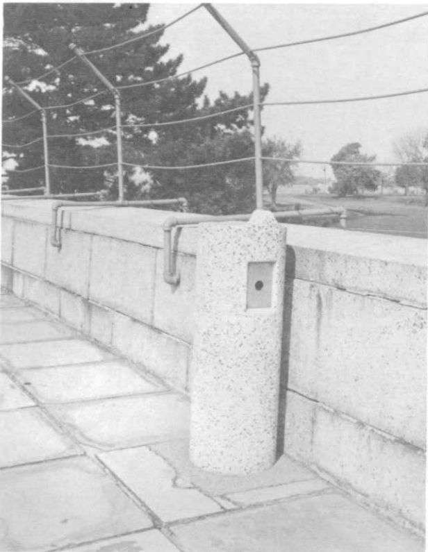
ILLUSTRATION 166. Partial view of east wall of upper plaza showing "safety fence." Concrete cylinder is the base of a drinking fountain no longer in use.
