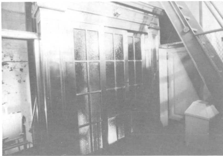
ILLUSTRATION 90. View of south wall of upper elevator landing showing bronze elevator enclosure and panelled partitions. Note panelled door to emergency exit stair in open.
