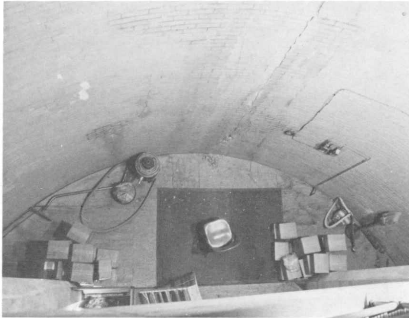
ILLUSTRATION 69. Partial view of "temporary structure" at the second level above lower elevator landing.
