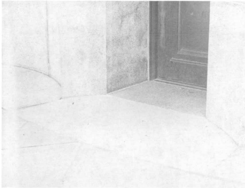
ILLUSTRATION 137. View of sloped concrete ramp at north entrance door.
