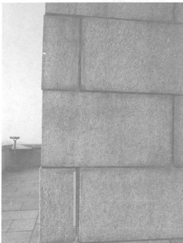
ILLUSTRATION 79. View toward southeast of observation gallery and detail of northeast corner of penthouse.
