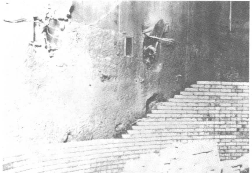
ILLUSTRATION 11. Scars remaining on the inner surface of concrete walling the column well from placing and removing the derrick support system, and partially set brick veneer for the interior finish of the column interior.
