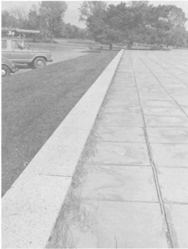
ILLUSTRATION 146. View of north edge of lower plaza, looking toward east.
