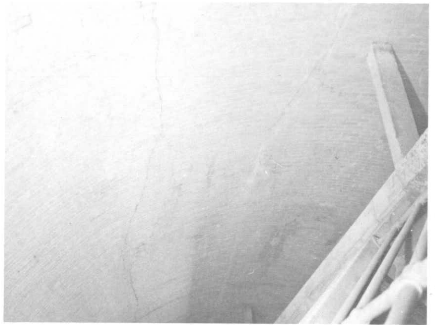
ILLUSTRATION 55. General view of brick crack in north quadrant of column shaft at approximately level 5.
