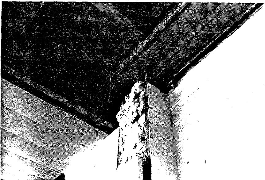
Illustration 55 Manor House Detail, concealed cornice at east wing West side
