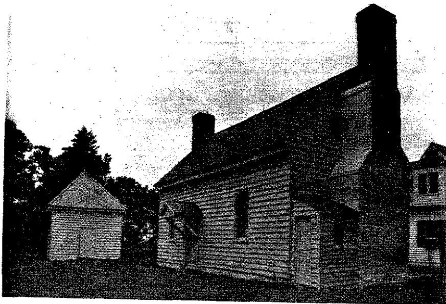
Illustration 74 Outside kitchen from southwest
