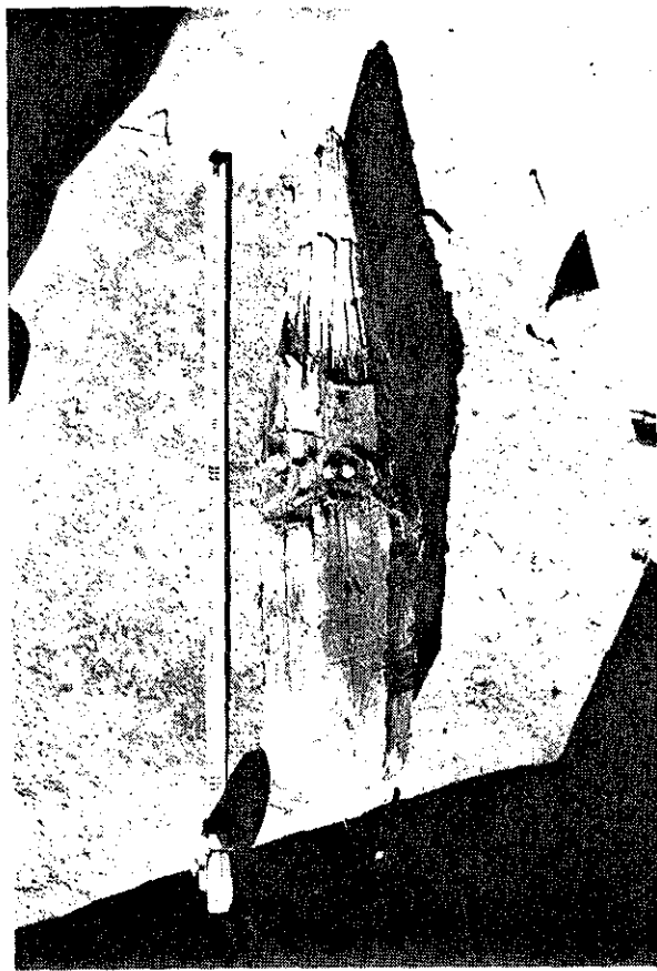
Illustration 110 Smokehouse Roof vent plug
