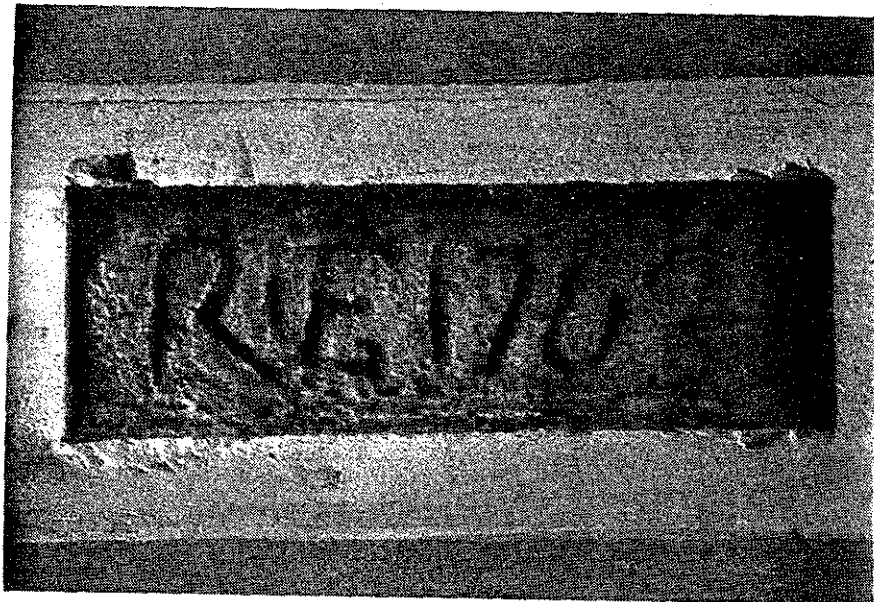
Illustration 62 1981 Manor House, first floor Interior, Room 107 Brick in southwest fireplace "RE 1763"
