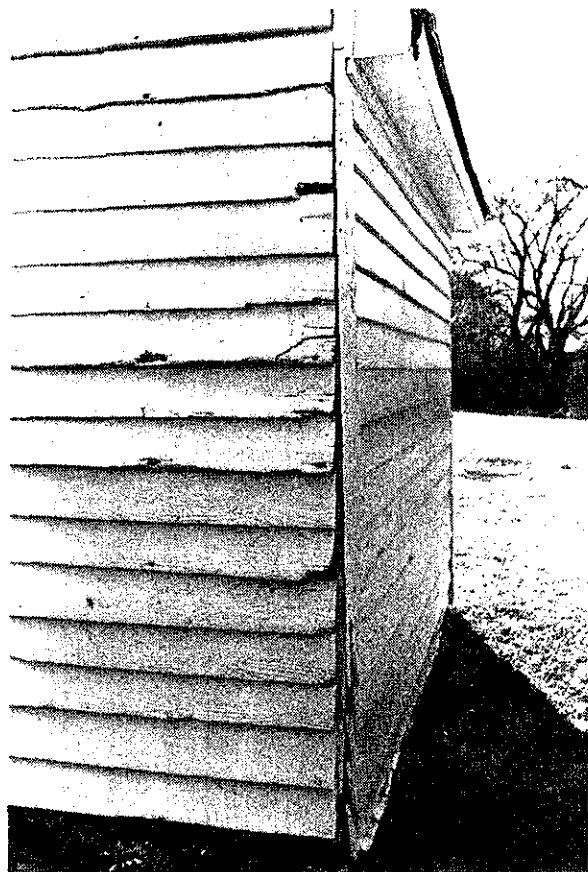
Illustration 103 Old Smokehouse Northwest corner
