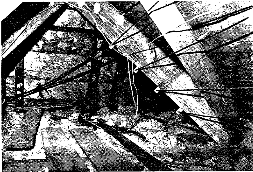
Illustration 68 Manor House Interior, above Room 211 Roof framing from north
