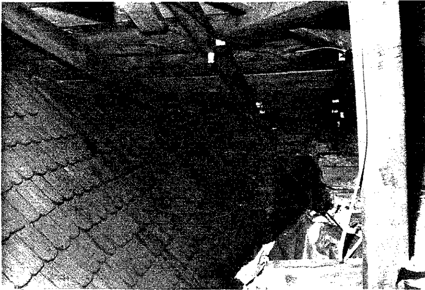
Illustration 71 Manor House Interior, above east wing bathroom from the east
