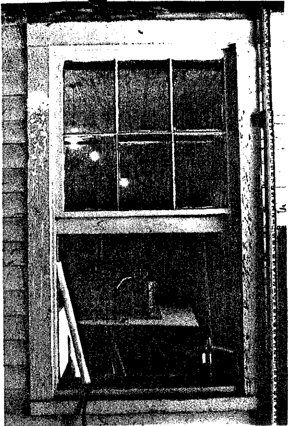
Illustration 91 Carriage House Interior, east addition Detail 1916 window
