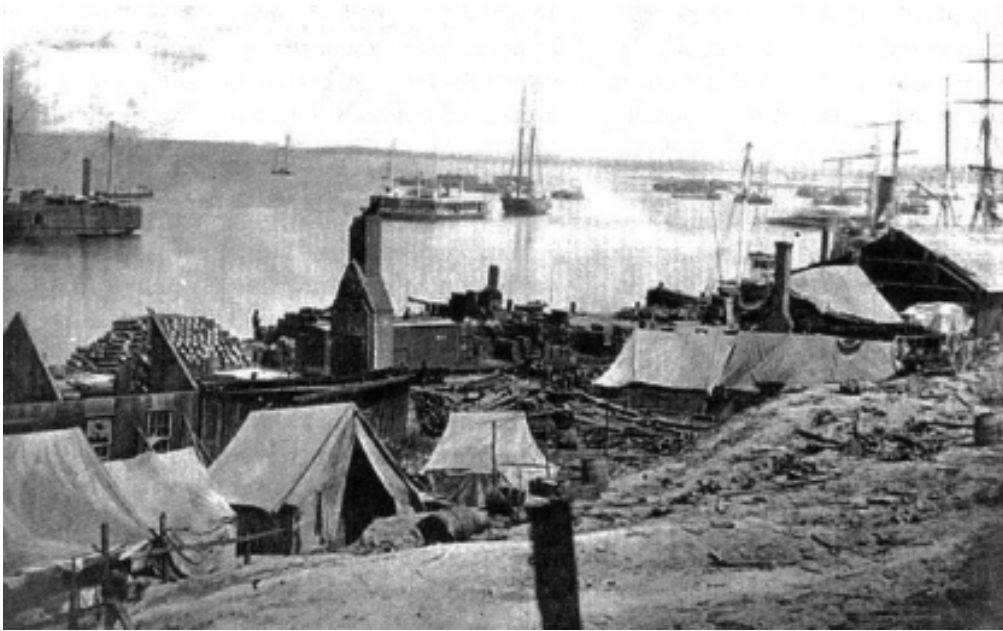
Figure 52. Photograph of the damage caused by the August 9 explosion at City Point (National Park Service).
