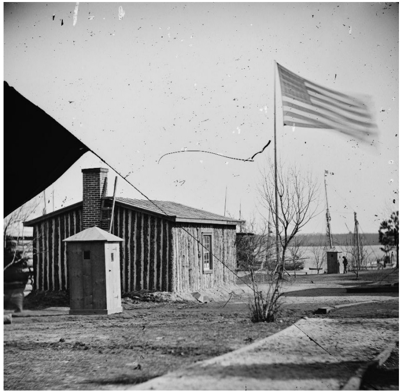
Figure 26- View looking east towards flagpole. Library of Congress, B811-2587.
