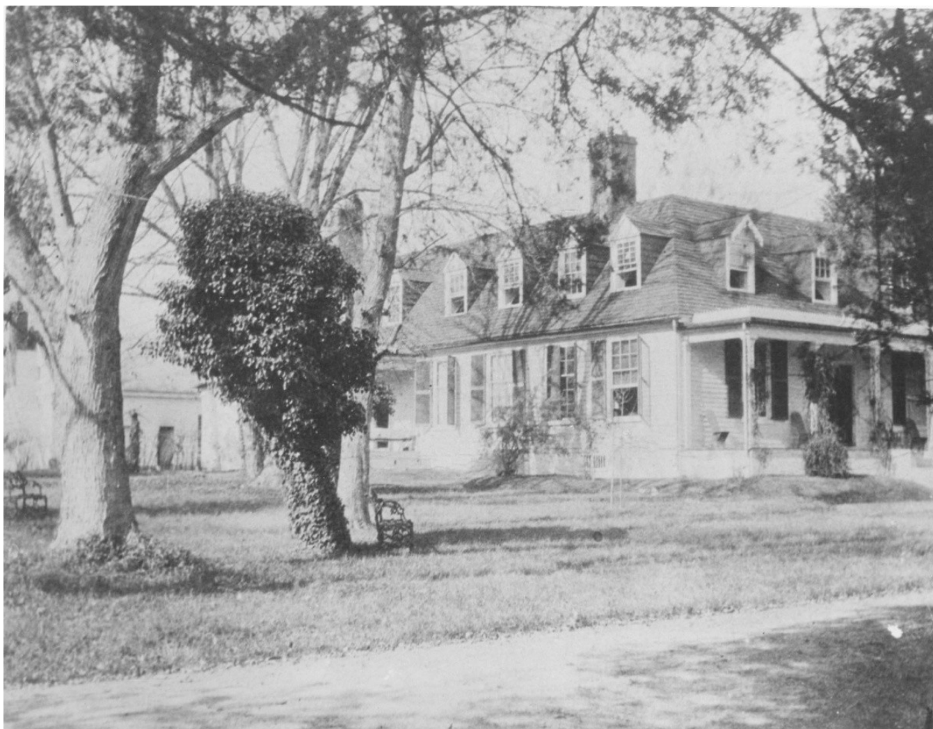
Figure 36- View of south and east facades of Appomattox Plantation. Petersburg National Battlefield.
