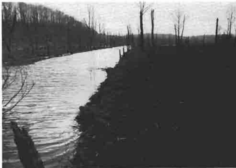
Photograph (22) Canal with water at mile 67.85
