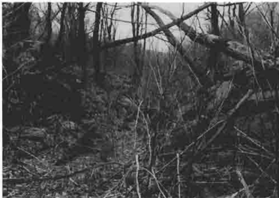
Photograph (39) Remains of guard lock 2 at mile 79.1
