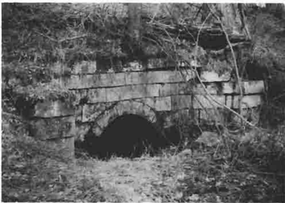
Photograph (28) Remains of an arched canal culvert at mile 76.1
