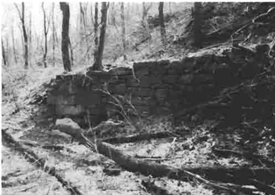
Photograph (34) Remains of guard lock 1 at mile 77.55
