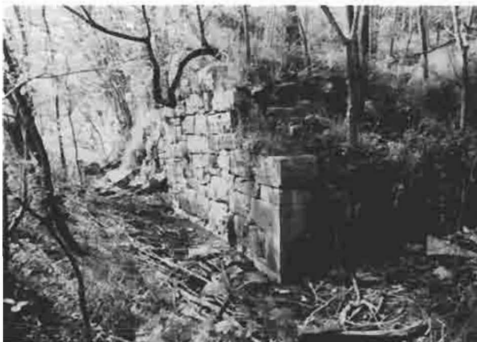
Photograph (68) Partial remains of a stone side wall at lift lock 9 at mile 29.5 below Hollidaysburg
