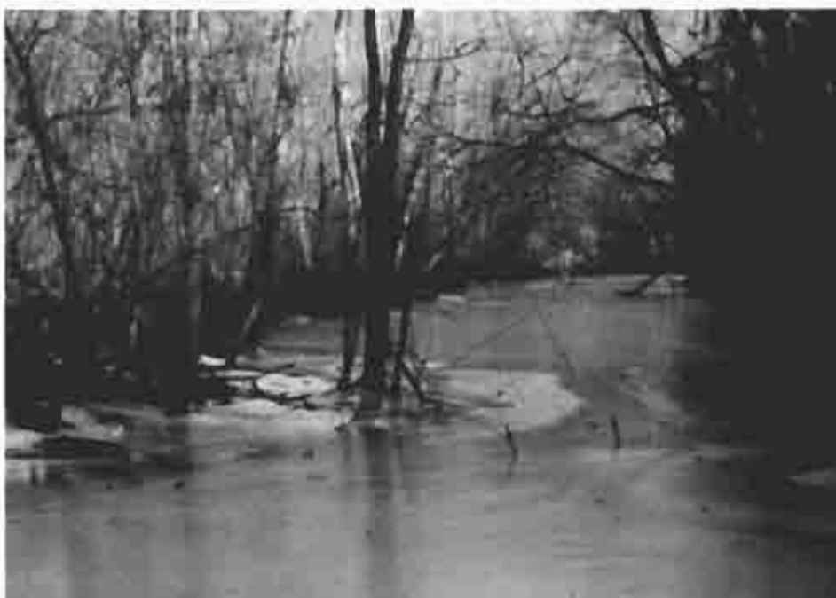
Photograph (70) Canal channel with water at mile 32.45 below Hollidaysburg
