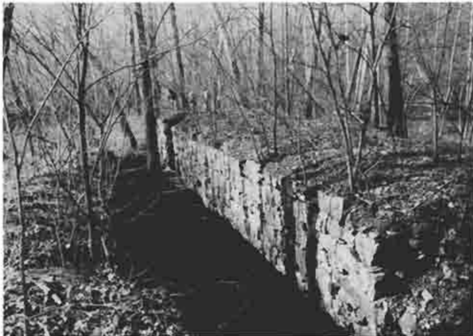
Photograph (57) Remains of guard lock 23 at Porter's Dam at mile 19.3 below Hollidaysburg
