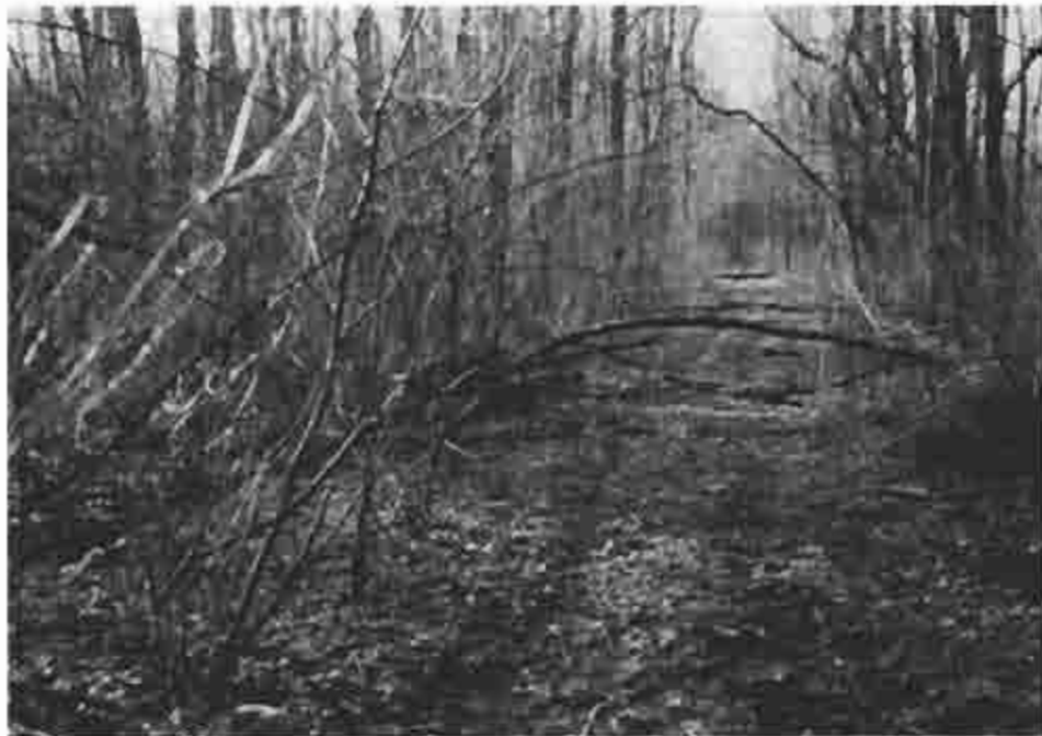
Photograph (29) Remains of the towpath at mile 76.2
