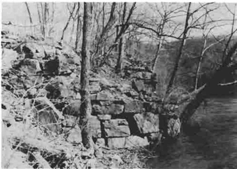
Photograph (56) Remains of the Schmucker's Dam north abutment at mile 17.6 below Hollidaysburg
