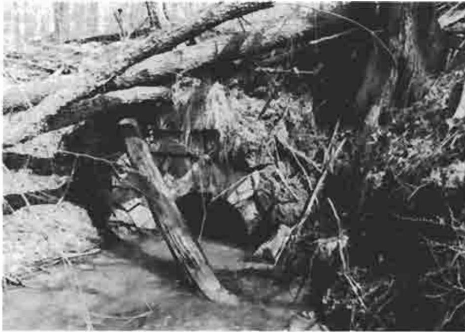
Photograph 15 Remains of an arched canal culvert at mile 57.5
