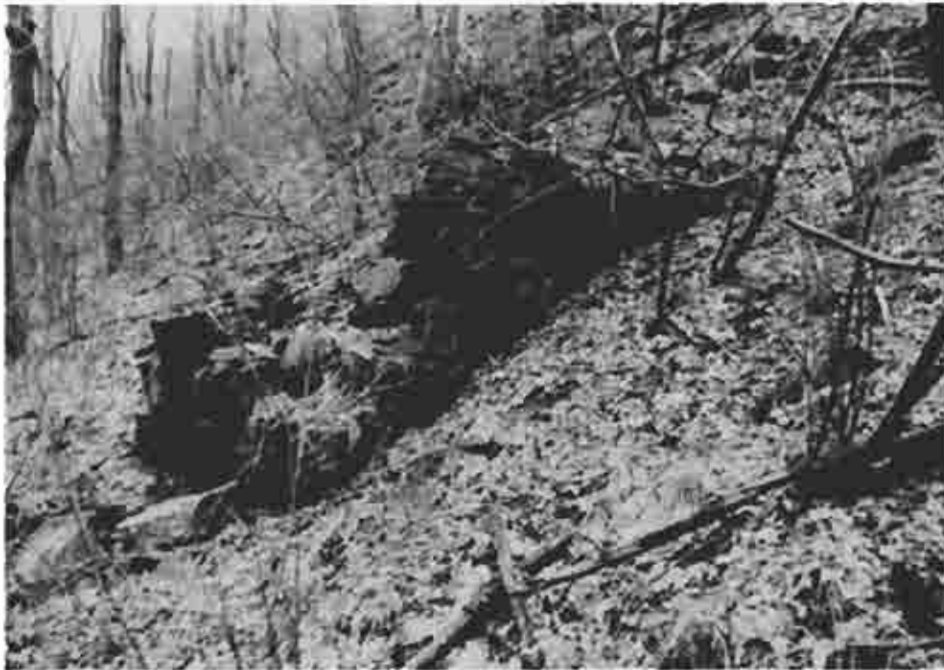
Photograph (41) Remnant of the towpath crossover bridge south abutment at mile 80.6
