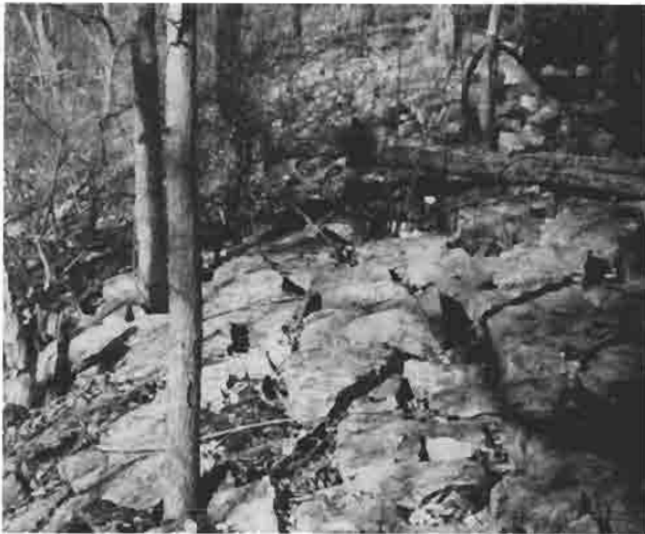
Photograph (48) Remains of the top of the East Reservoir dam used as a feeder for canal water at Hollidaysburg
