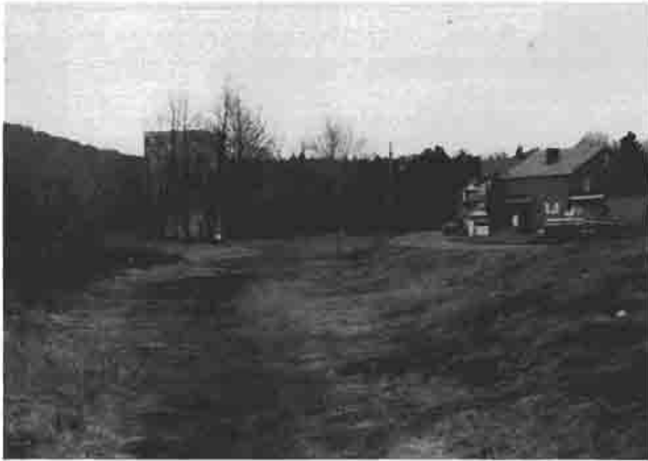
Photograph (13) Remains of the canal viewed from the High Street bridge in Saltsburg at mile 56.0
