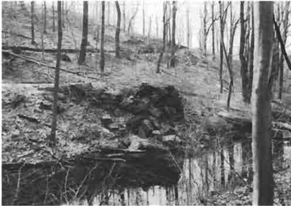
Photograph (33) Remains of a towpath crossover bridge abutment at mile 77.45
