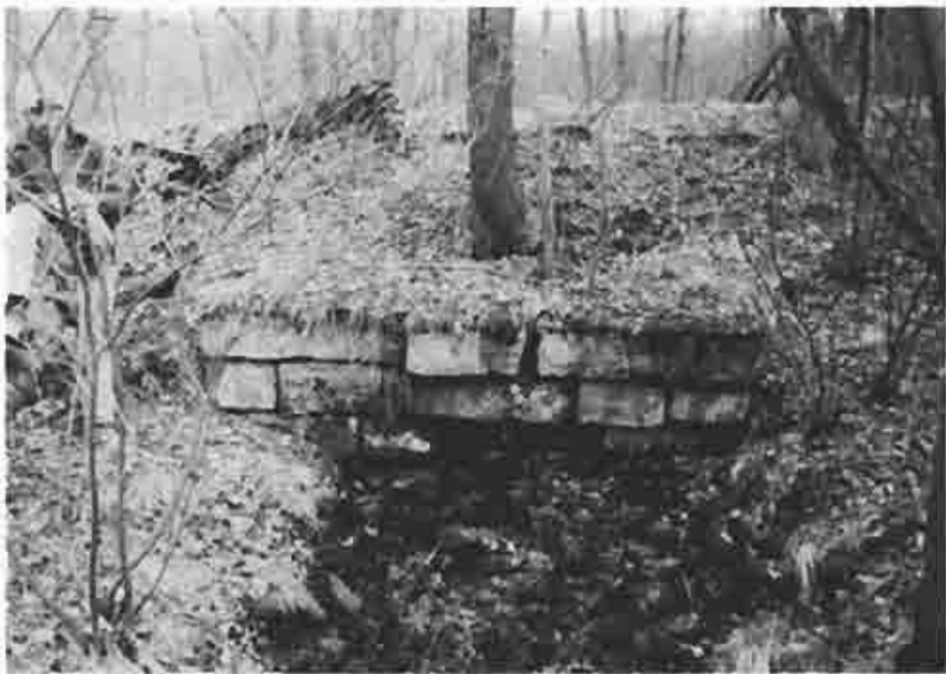
Photograph (18) Remnant of the waste gate at mile 58.4
