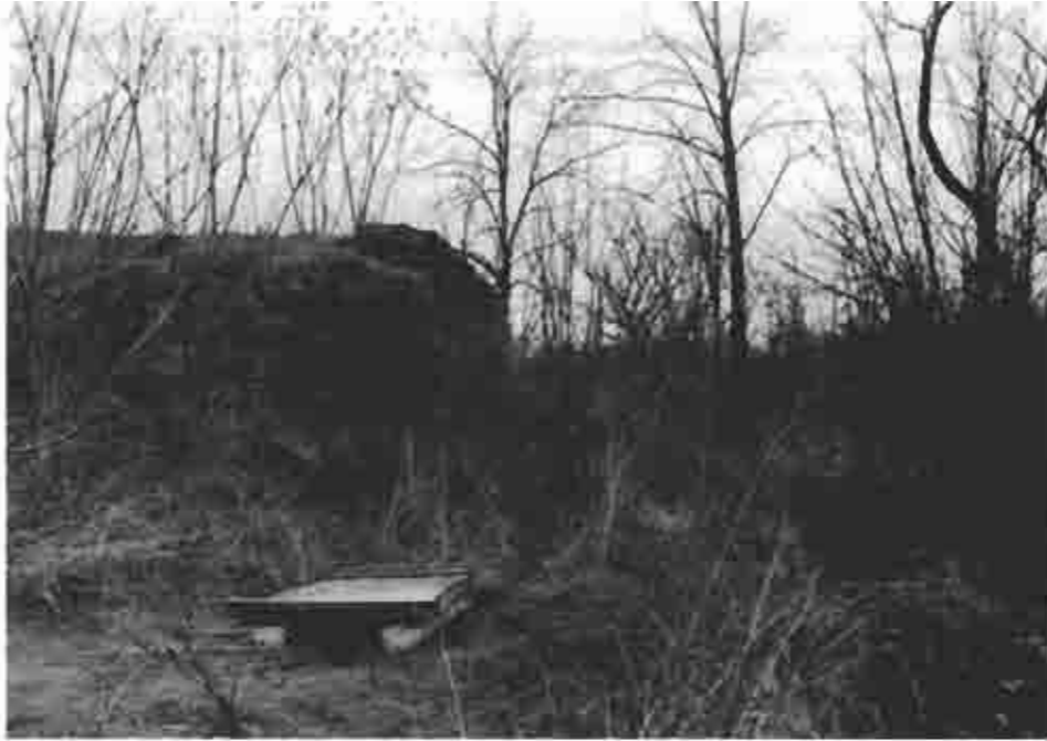
Photograph (51) Northeast abutment of Three Mile Dam at mile 12.3 below Hollidaysburg
