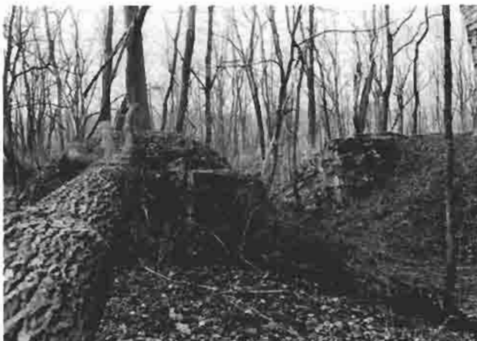
Photograph (61) The remnant of lift lock 20 at mile 20.85 below Hollidaysburg
