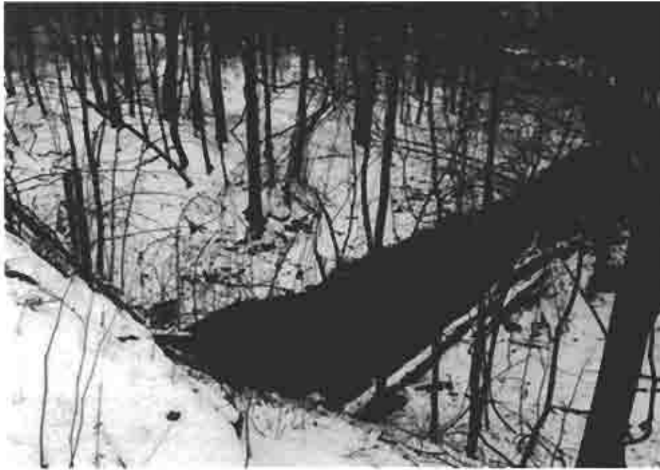
Photograph 19 Site of the Elder's Run aqueduct at mile 59.75
