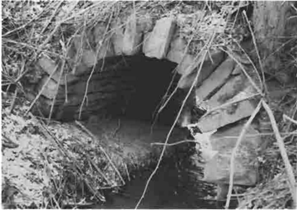
Photograph (25) Remains of the arched towpath culvert at mile 73.85
