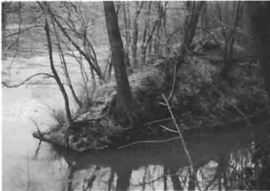
Photograph 9 Remains of a Long Run towpath bridge abutment at mile 50.25
