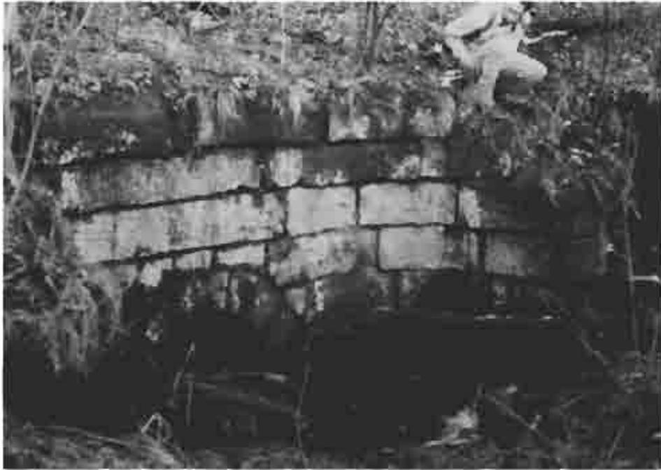
Photograph (31) Well preserved arched canal culvert at mile 76.8
