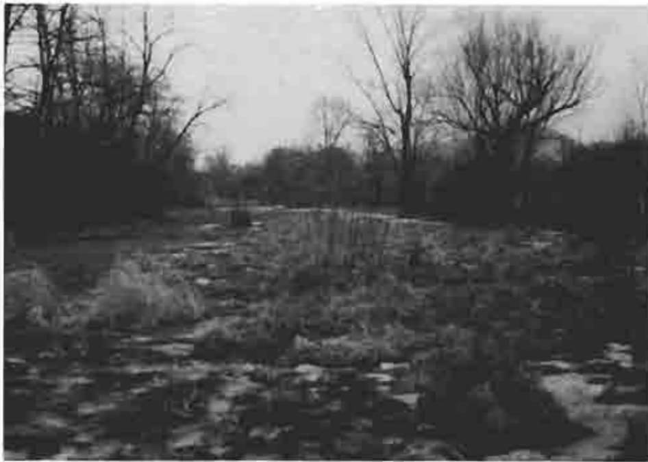
Photograph (50) Site of the canal channel at mile 7.8 below Hollidaysburg
