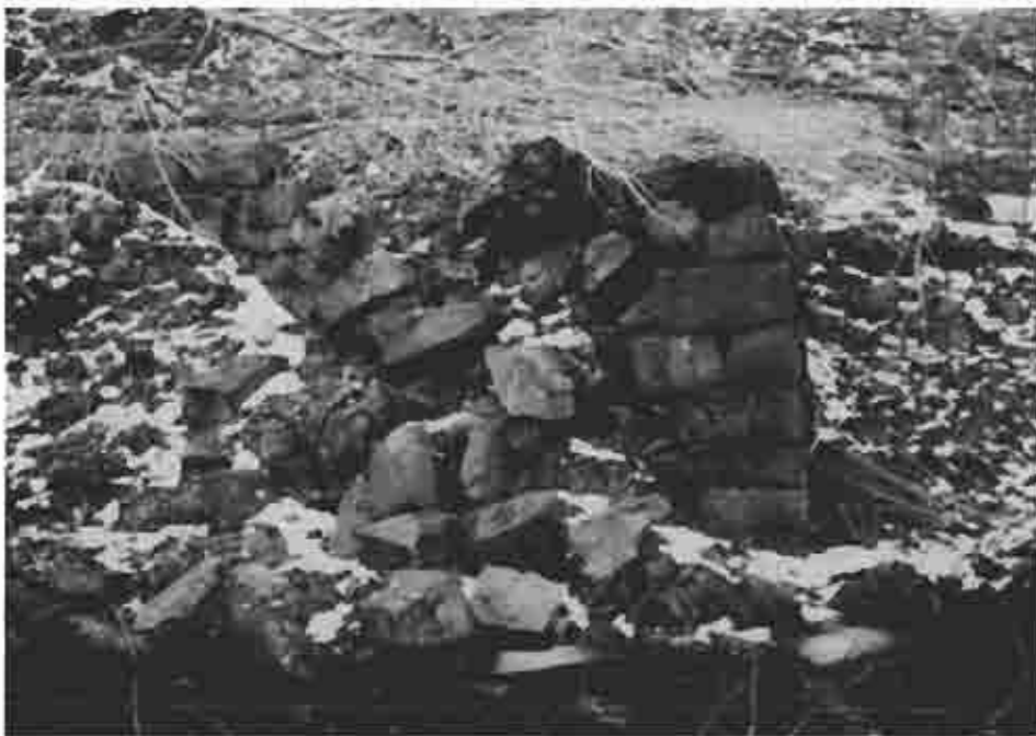
Photograph (32) Remains of a canal bridge abutment at mile 77.0
