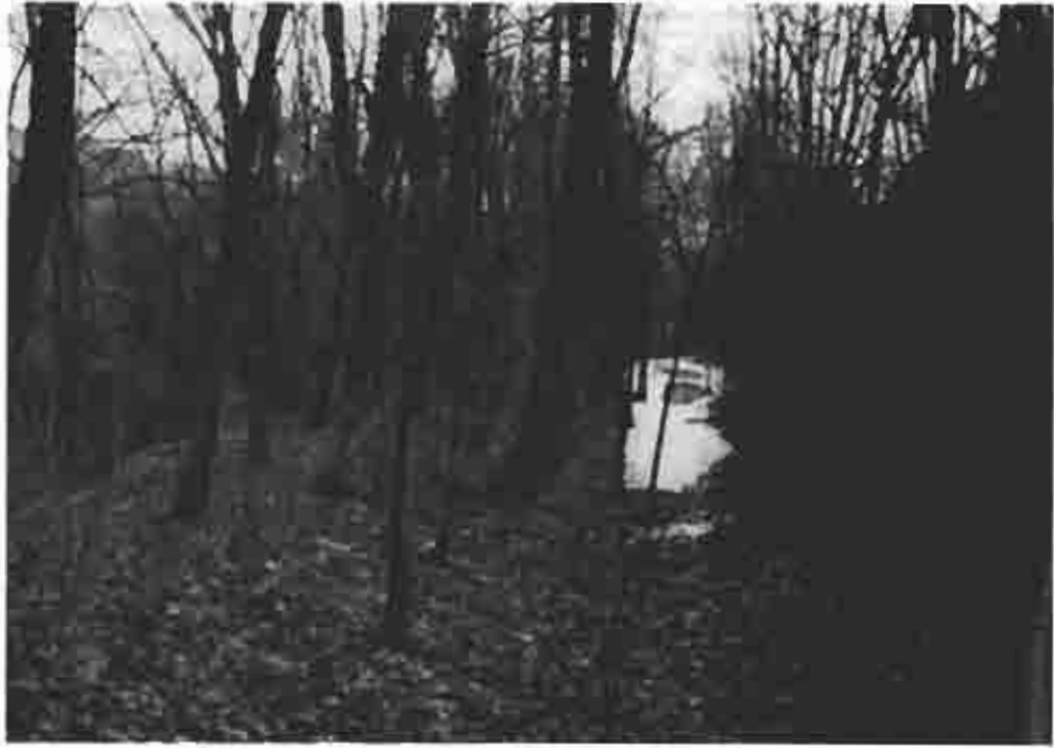
Photograph (49) Remains of the canal channel with some water at mile 6.5 below Hollidaysburg
