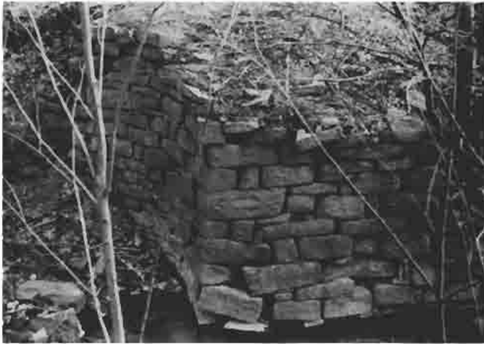
Photograph ⑦ Remnant of the Flat Run towpath bridge east abutment at mile 47.5
