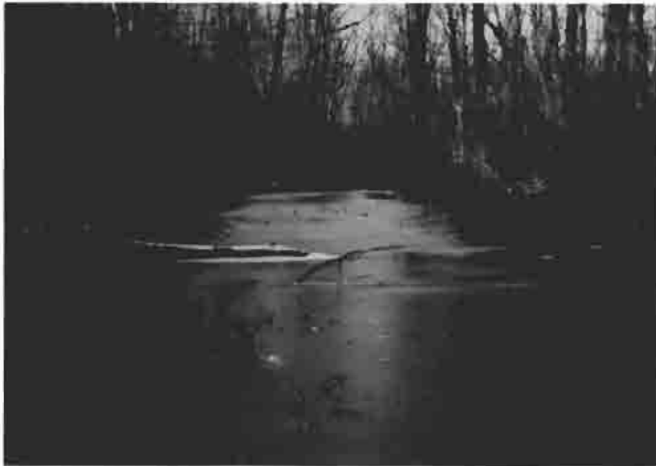
Photograph (27) Canal with water at mile 75.8
