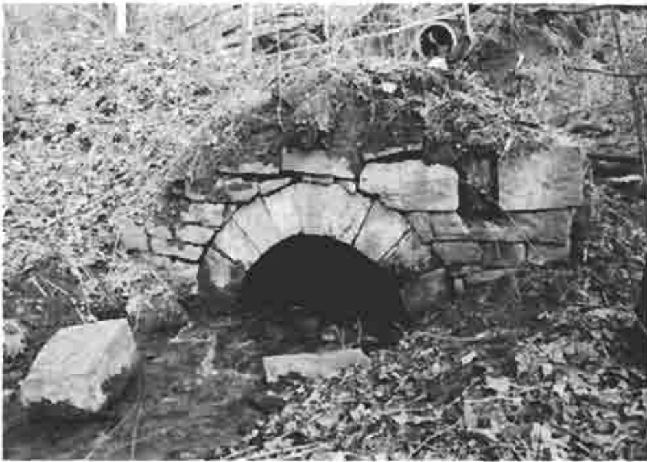
Photograph (14) Remains of an arched canal culvert at mile 57.3
