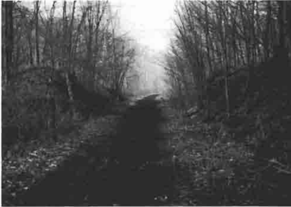
Photograph ⑤ Site of guard lock 2 at mile 45.3. This view looks through the remains at the guard lock
