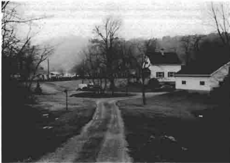
Photograph ③ Site of lift lock 2 at mile 41.65. The circular depression in the center contains the site of this lock
