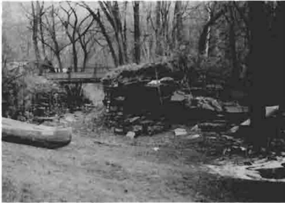
Photograph (73) Remains of the guard lock at the Raytown Feeder Dam at mile 6.3 below Huntingdon
