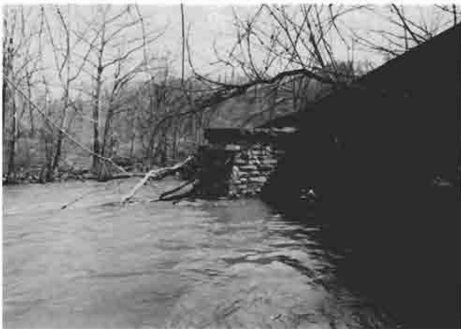
Photograph (54) Remains of the towpath bridge west abutment at mile 16.1 below Hollidaysburg which has been incorporated into a railroad bridge
