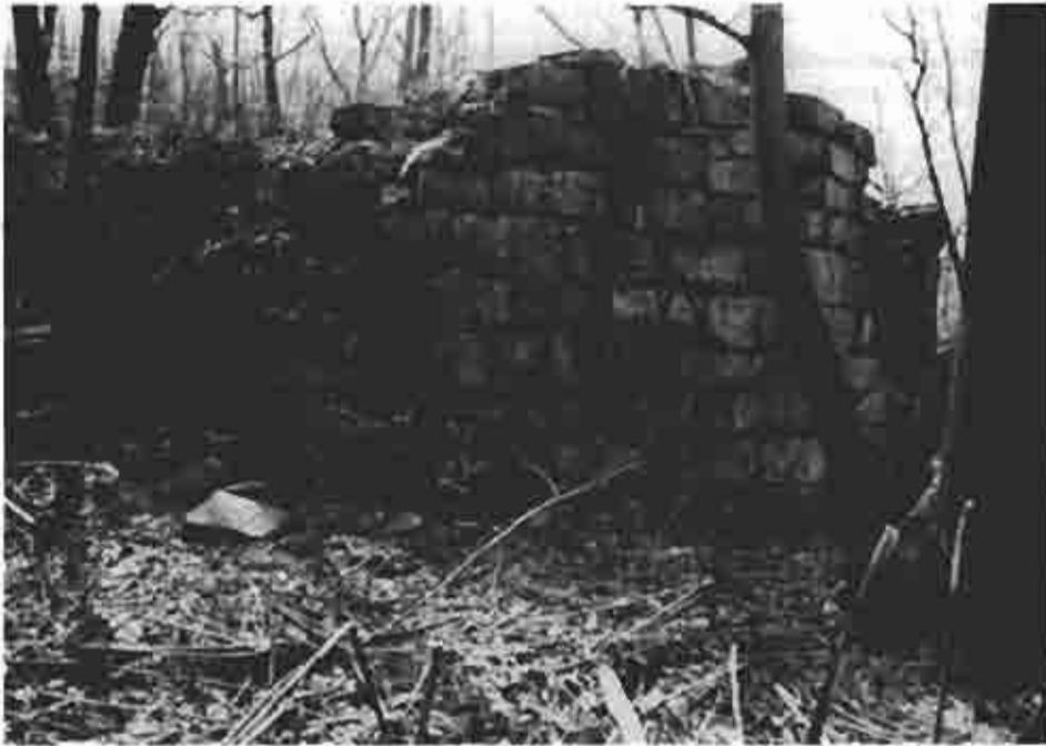
Photograph (35) Remnant of the southwest abutment of dam 1 at mile 77.55
