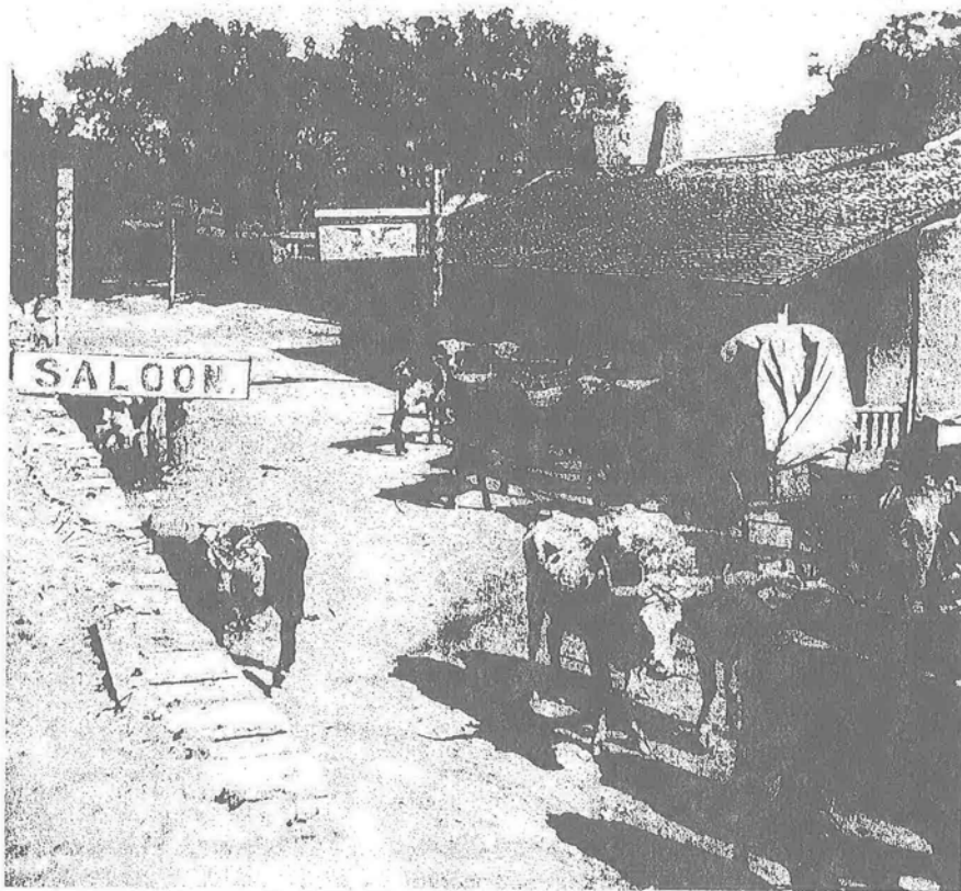
Pigeon's Ranch, looking west, as it appeared in 1880. Three rooms of the building near the top of the photo is the only structure that remains intact today, although it has major structural problems. The animals, men, and wagons stand on the Santa Fe Trail, where Highway 50 is today. "Pigeon's Ranch Glorieta New Mexico June 1880" photograph by Ben Wittick, courtesy of the Museum of New Mexico, Negative MNM 15783, School of American Research Collections, the Palace of the Governors, Fray Angélico Chávez History Library, Santa Fe.
