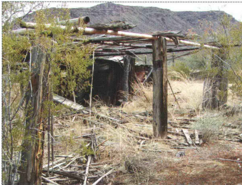
West elevation of the Ramada with Blacksmith Shop behind.
