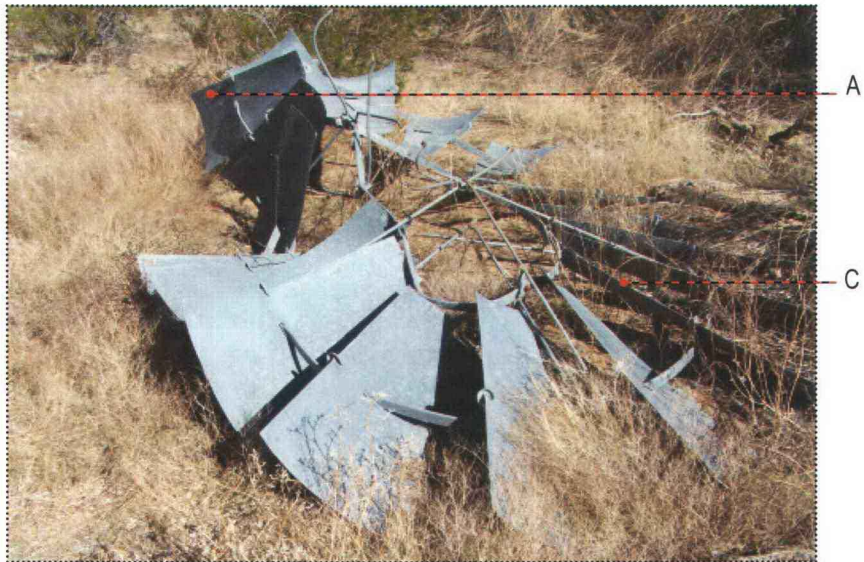
Blades from Windmill 3 lie on the ground near its base. (letters refer to notes in condition assessment table below)
