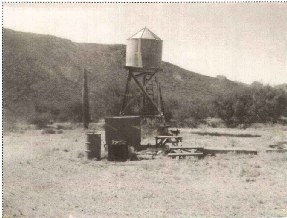
Bates Well and water tower, May 1979, Organ Pipe Cactus NM Photo Archive No. 616
