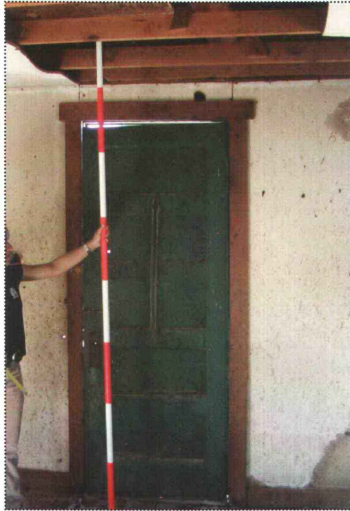
View of the entrance door from the inside.
