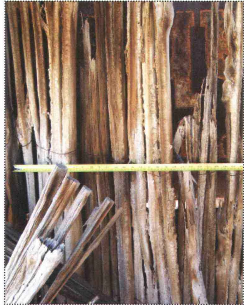
Saguaro ribs tied with barbed wire that clad the Ocotillo Shed.
