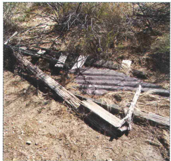
Parts of the structure lying scattered around on the site
