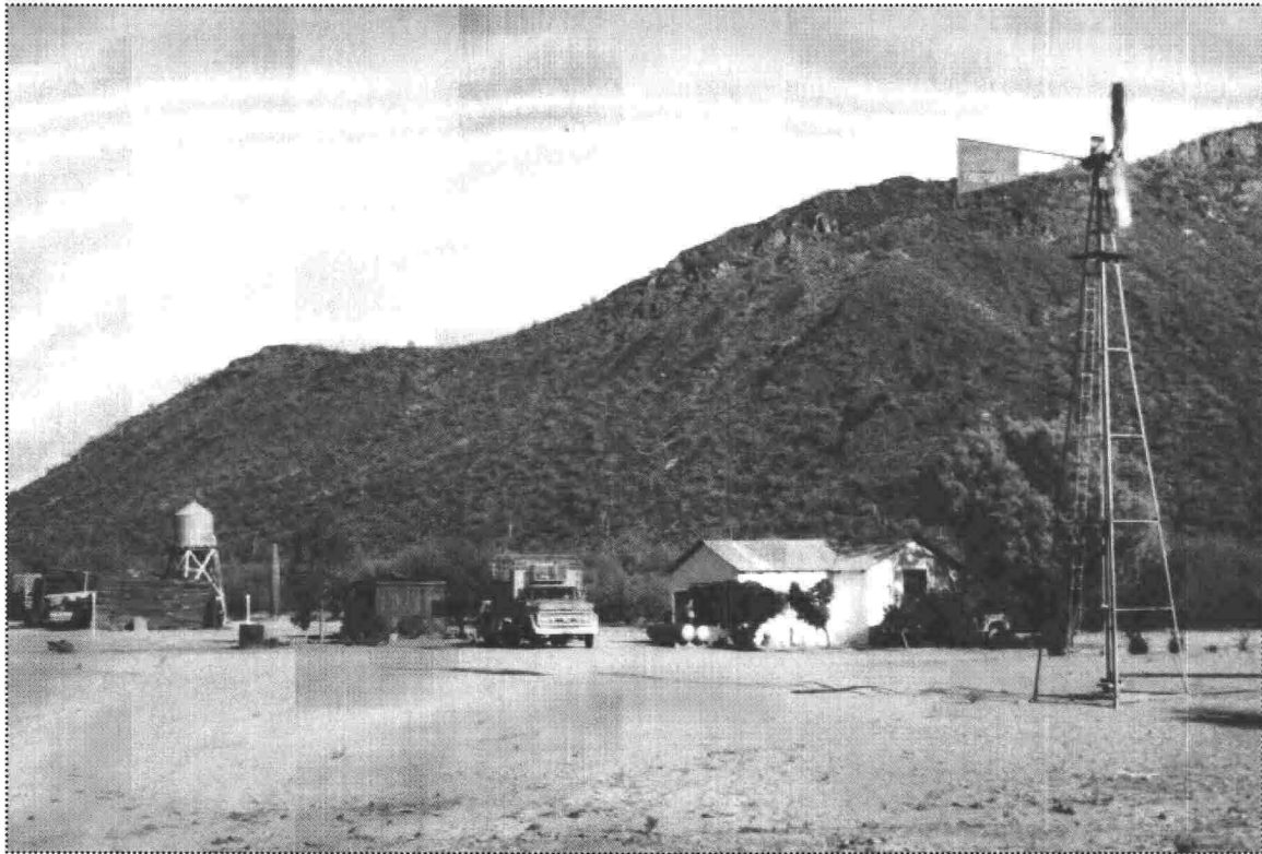
Bates Well water tower (left) Main Ranch House (middle), and Windmill 1 (right), date unknown, Organ Pipe Cactus NM Photo Archives No. 621
