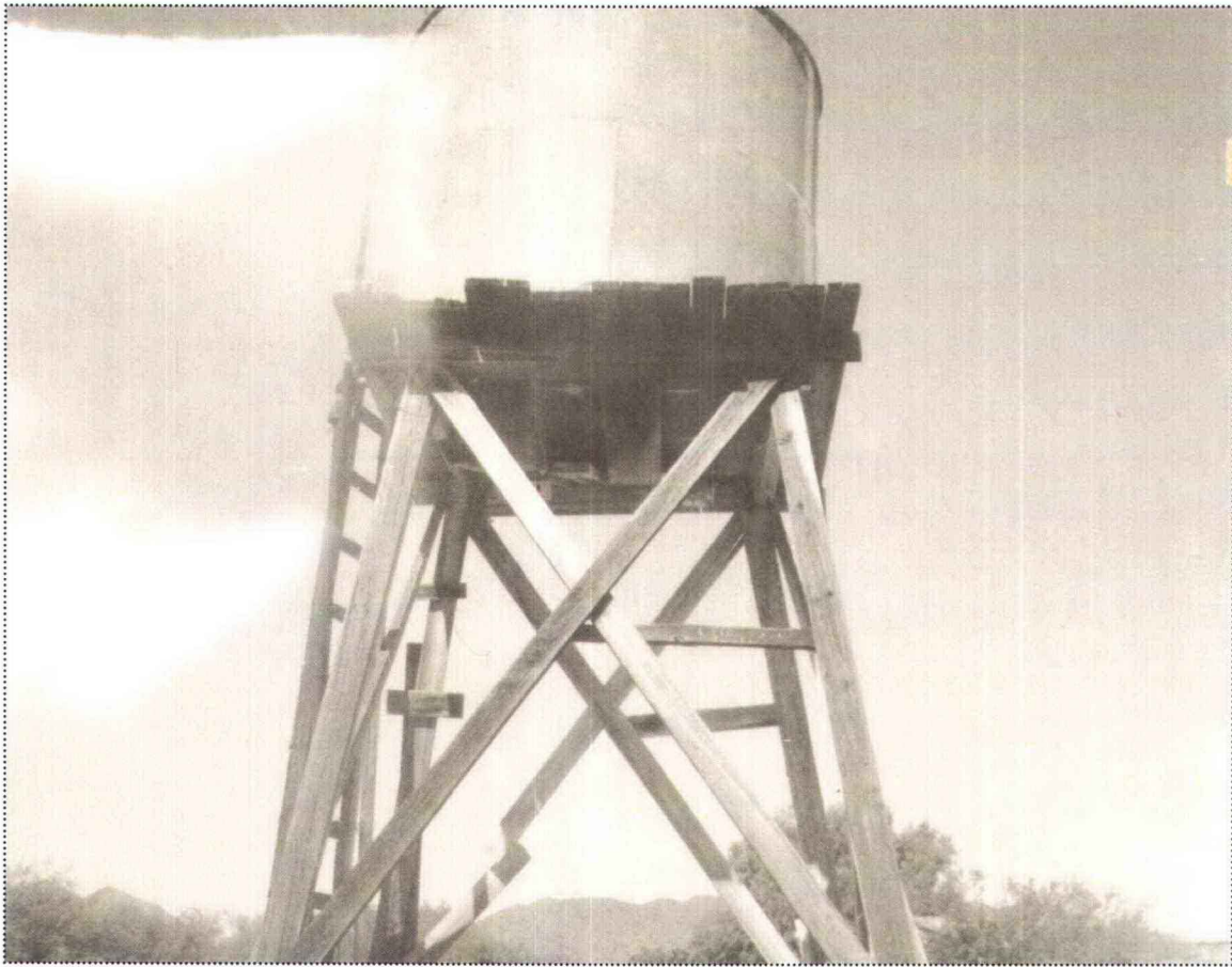
Bates Well water tower, May 1979, Organ Pipe Cactus NM Photo Archive No. 615
