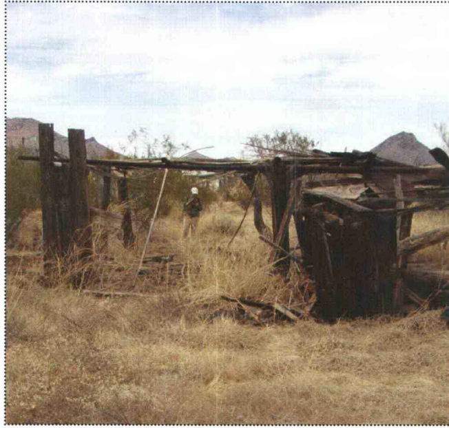
South elevation of the Ramada with Blacksmith Shop to the right.
