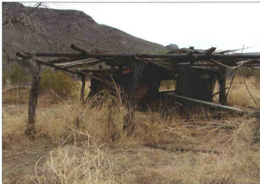
North elevation of the Ramada with Blacksmith Shop behind. The structure of the ramada consists of mesquite logs and railroad ties supporting steel piping with a combination of milled lumber, saguaro ribs and steel piping providing the cladding.
