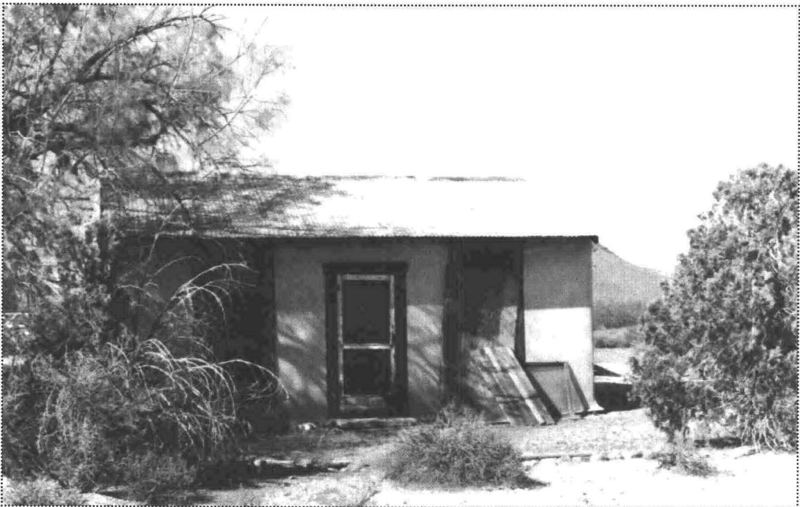
Main Ranch House south facade, April 1989, Organ Pipe Cactus NM Photo Archives No. 3783
