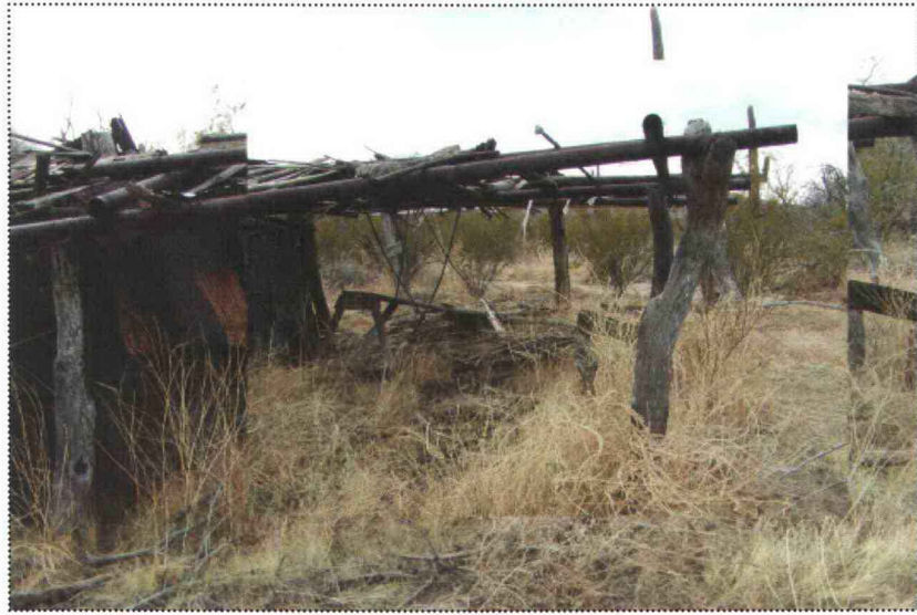
East elevation of the ramada with Blacksmith Shop to the left.
