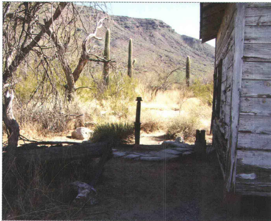
View of the arrastra situated right next to the east wall of the Bunkhouse
