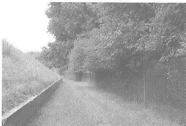
FIGURE 49. Funeral Mound (Mound C) retaining wall, looking west, 2006.
