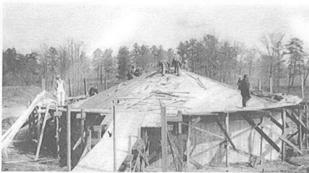
FIGURE 23. Earth Lodge reconstruction of concrete shell, 1937. (OCMU Collection)
