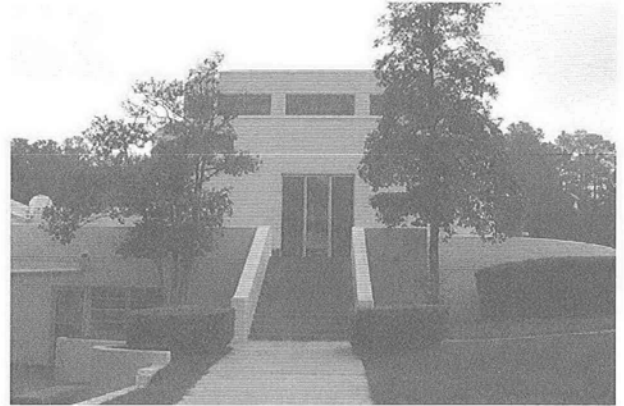
FIGURE 36. Southwest elevation of Visitor Center, 2006.
