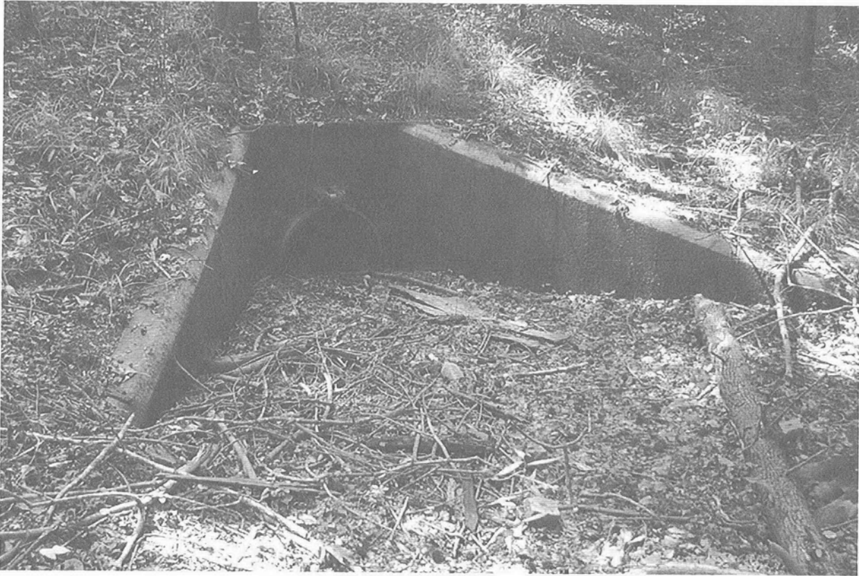
FIGURE 56. Culvert on the Lamar levee, 2006.
