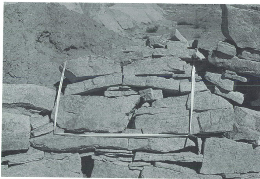
Figure 17. The east wall of Structure 2 before stabilization.
