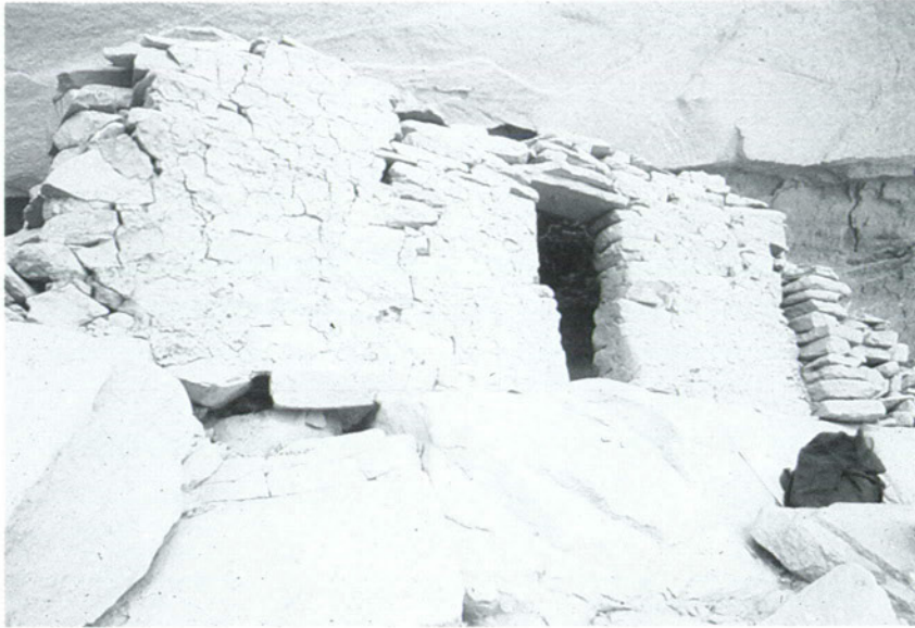
Figure 33. The nature of the other In-and-Out House (42Ka595), is shown here, with T-shaped doorway and crack in wall at the left. The crack was stabilized with soil-epoxy mortar, but subsidence of the boulders upon which the structure reposes has caused further cracking since the photo was taken.
