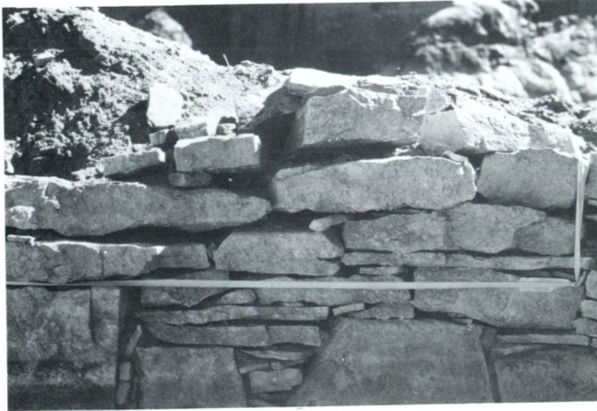
Figure 15. The south wall of Structure 1 before stabilization.
