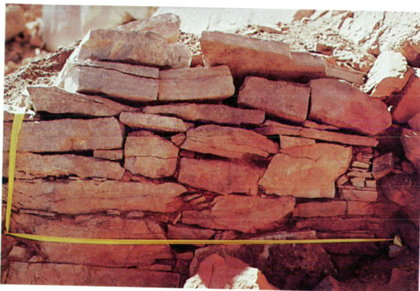
Figure 20. The west wall of Structure 1 before stabilization.
