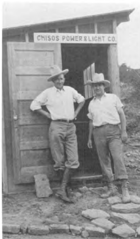
S. Herbert Evison and Conrad L. Wirth stand before the power plant installed by the army for the CCC camp in the area known as the “basin” near the top of Chesos Mountain, at that time a Texas State park. Later it became a part of Big Bend NP.
