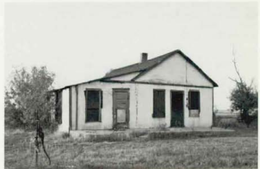
FIGURE II-1: The Charles Williams house. A typically modest residential structure in Nicodemus, the gable-end portion dates to the pre-1920s, and the lean-to addition was added in the 1930s. Like a number of wood frame structures in Nicodemus, the building has been stuccoed with a plaster mixture of cement, water, sand, and hog hair. Interestingly, the northeast room of the house was operated as a post office by William's wife, Elizabeth, in the 1930s. (Photograph: La Barbara Fly)
