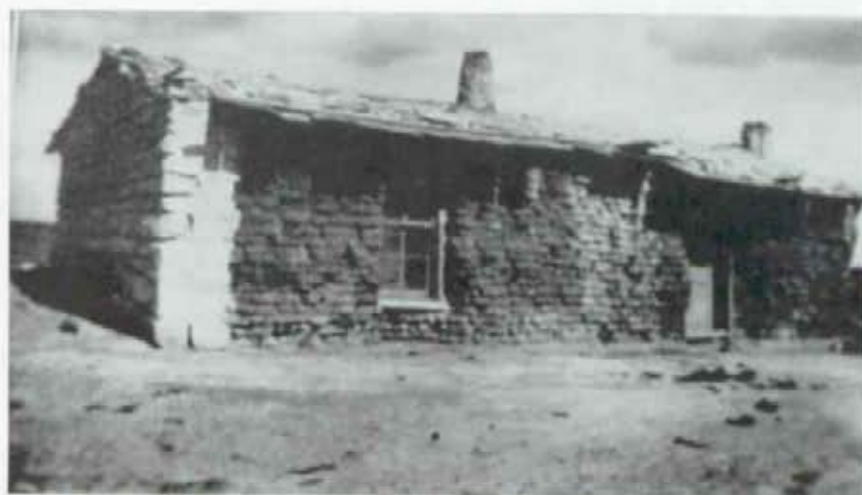
FIGURE I-7: This rare historic photograph of an above-ground Nicodemus sod house, or "soddy," was identified as the Tuss-Lacey house by present-day local residents. Note that one elevation is of limestone construction, a popular but more expensive and time-consuming building method than was usually employed. The structure is no longer extant. (Photograph: Ernestine VanDuvall)
