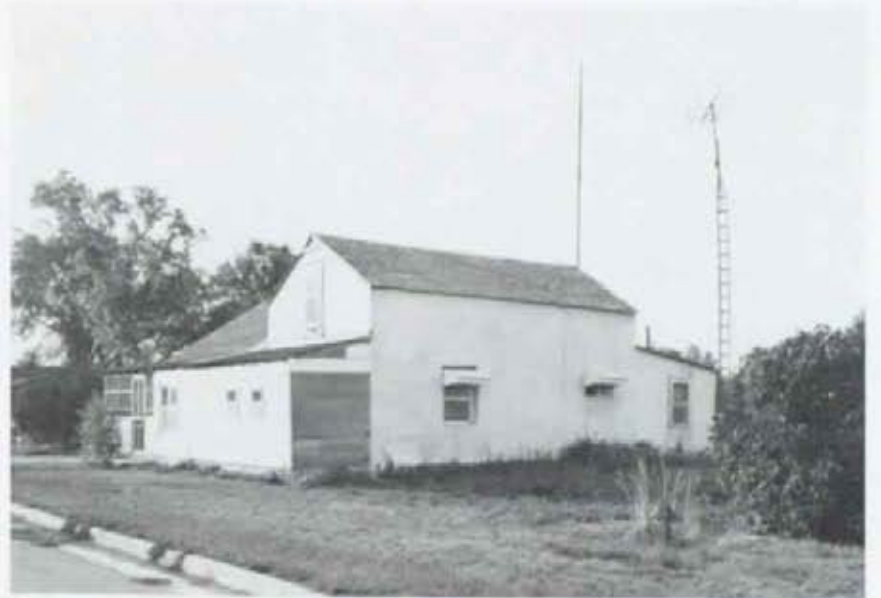
FIGURE II-9: The Saint Francis Hotel (now referred to as the Fletcher-Switzer residence). Zach Fletcher's 1881 hotel is the two-story stuccoed portion to the right, and originally featured a cut limestone appearance with a one-story stone kitchen addition on the east. This historic structure has received numerous alterations and additions over the years, but remains as one of the oldest extant historic buildings in Nicodemus today. (Photograph: Clayton Fraser)
