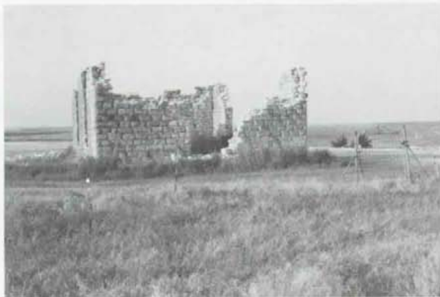
FIGURE II-4: Of the three nineteenth-century satellite communities surrounding Nicodemus, only one, Mount Olive, exhibits physical remains today. This ruin is all that remains of the Mount Olive Church. One of the three standing limestone ruins associated with the community, this structure was burned during the 1930s when a routine "burning off" of the grass in the nearby cemetery got out of control. Two similar ruins, a school house and a residence, stand nearby. (Photograph: Clayton Fraser)
