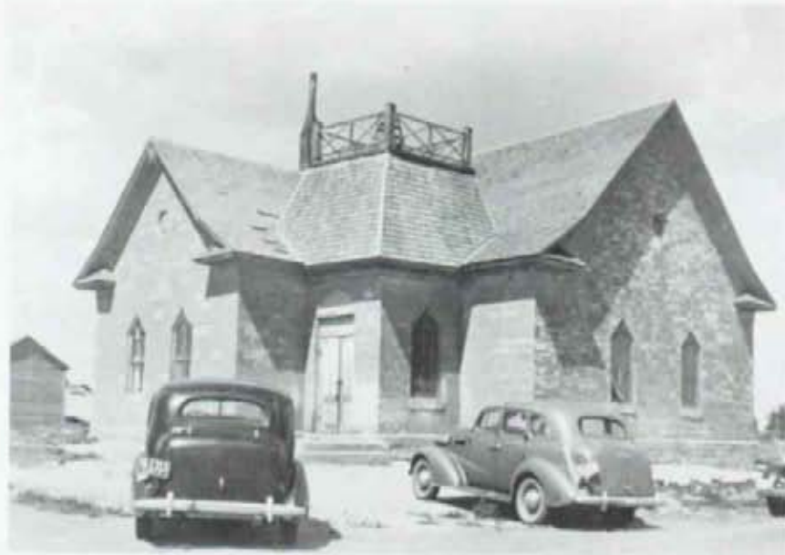
FIGURE II-8: A 1943 photograph of the First Baptist Church shows the structure after a 1930s windstorm blew off the original bell tower. Local tradition has it that the present structure, which was completed in 1907, was built around an earlier and smaller church. After the exterior of the present building was completed, the older structure was removed piece by piece through the front door. (Photograph: William T. Belleau, 1943. Source: Fort Hays State College, Fort Hays, Kansas)
