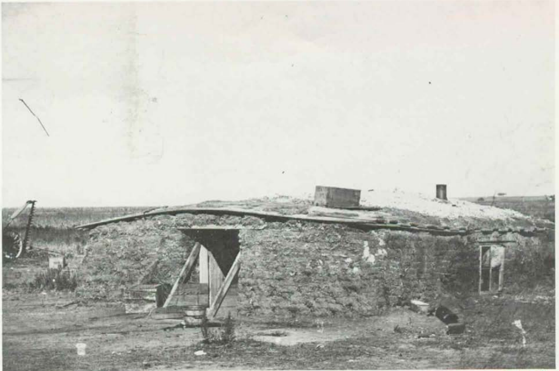
FIGURE II-3: This historic photograph of a nineteenth-century sod house in western Kansas shows what typical, first-generation buildings in Nicodemus must have looked like. These combination half sod and half dugout structures were easily and quickly constructed from local materials. Reputedly warm in winter and cool in summer, nonetheless, life in these structures must have been hard at best. (Photograph: Kansas State Historical Society, Topeka, Kansas)
