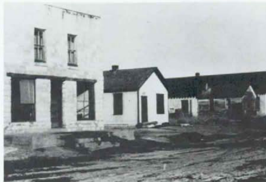
FIGURE III-9: Washington Street in Nicodemus, looking east in the 1940s. Though the Depression and dust storms of the 1930s are over, this view of the town causes one to question the town's recovery. From left to right, these structures are: the Masonic Hall, Jenny Riley's Restaurant, the Priscilla Art Club, and Township Hall. (Photograph: Black American West Museum, Denver, Colorado)
