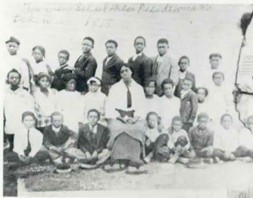
FIGURE III-2: The 1915 class at Fairview School, Nicodemus, Kansas. Each year the single-room school would typically feature one class of youngsters, from grade school to high school age. After 1945, all children in the Nicodemus area went to the District No. 1 School, and the Fairview School building was moved to the District No. 1 School site, for additional classroom space. (Photograph: Bernice Bates)
