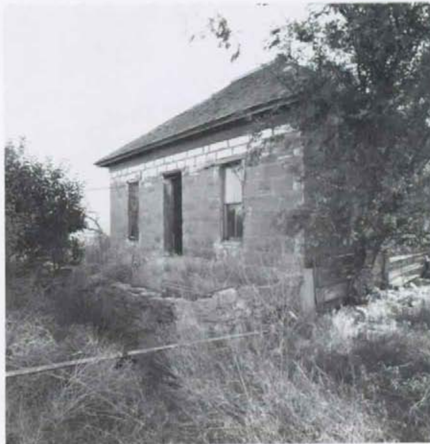
FIGURE II-7: Rectangular in plan with a clipped gable roof, the John Edwards house features cut limestone quarried from bluffs near Nicodemus. Simple cut limestone, hand-quarried from the ground, represented the most sophisticated and efficient method of construction in Nicodemus. Note the wood lintels over the windows and door. (Photograph: Clayton Fraser)
