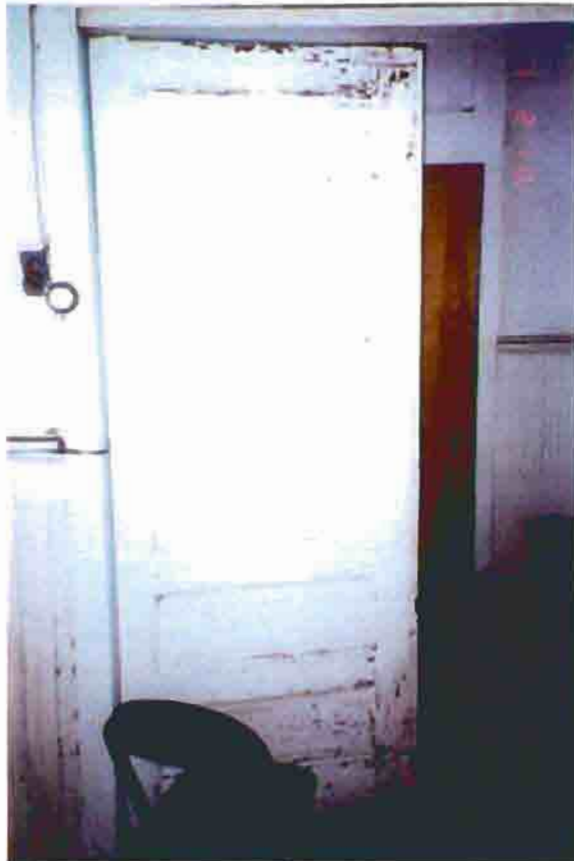
Photo B-23. The First Baptist Church, door from the vestibule to the sanctuary, February 2001. This door is typical of the six-panel doors throughout the church. Photo by Bahr Vermeer Haecker Architects, Lincoln, Nebraska.
