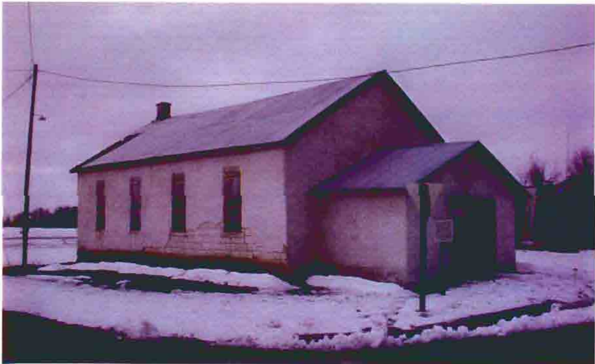
Photo A-12. The A.M.E. Church, view from the southeast, February 2001. Photo by Wiss, Janney, Elstner Associates, Northbrook, Illinois.
