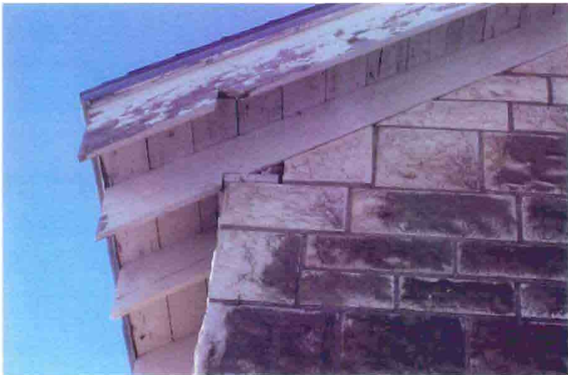
Photo T-14. The Township Hall, wood fascia and false rafters, February 2001. Photo by Wiss, Janney, Elstner Associates, Northbrook, Illinois.
