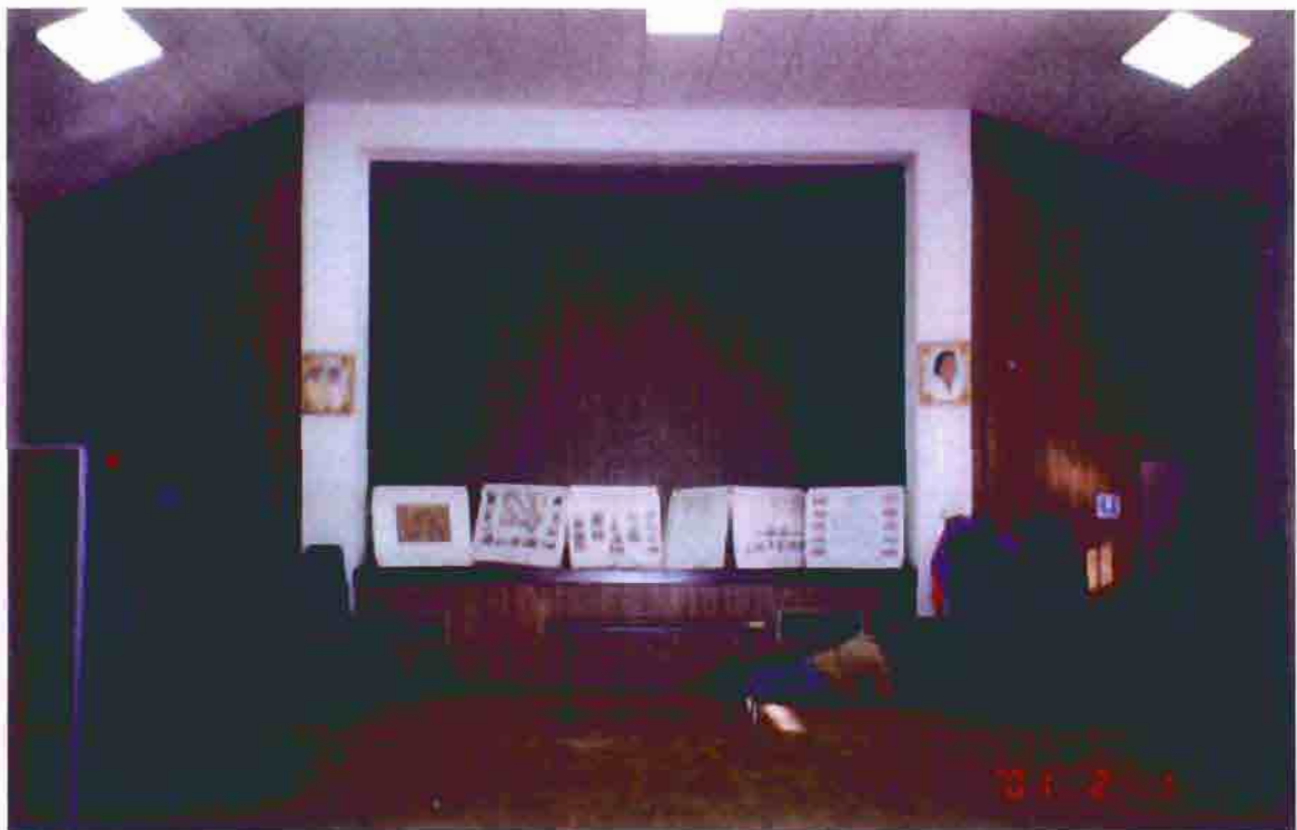
Photo T-26. Township Hall, interior view of main hall towards the stage, February 2001. Photo by Bahr Vermeer Haecker Architects, Lincoln, Nebraska.
