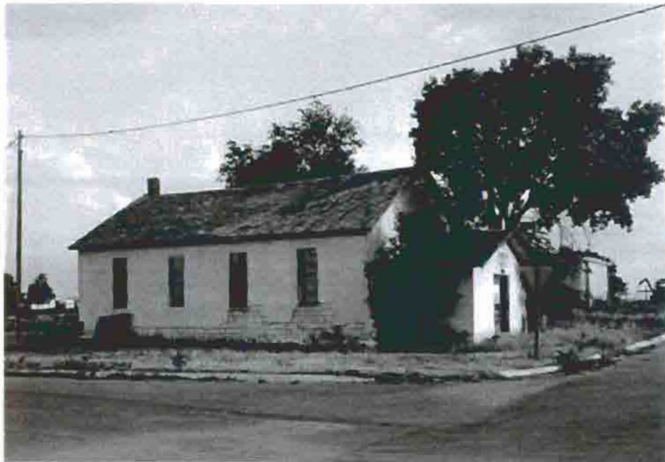
Photo A-9. The A.M.E. Church, view from the southeast, 1983. HABS photo by Clayton T. Fraser.
