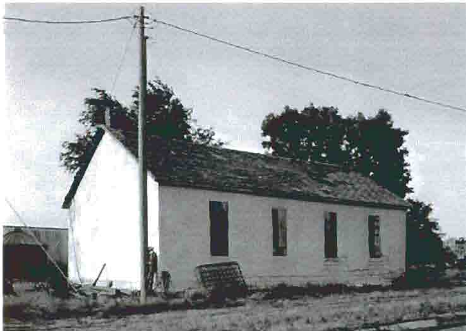
Photo A-7. The A.M.E. Church, view from the southwest, 1983. HABS photo by Clayton T. Fraser.
