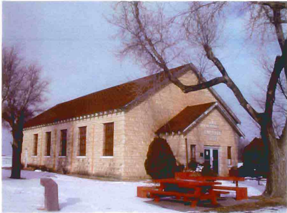
Photo T-8. The Township Hall, view from the southwest, February 2001. Photo by Wiss, Janney, Elstner Associates, Northbrook, Illinois.
