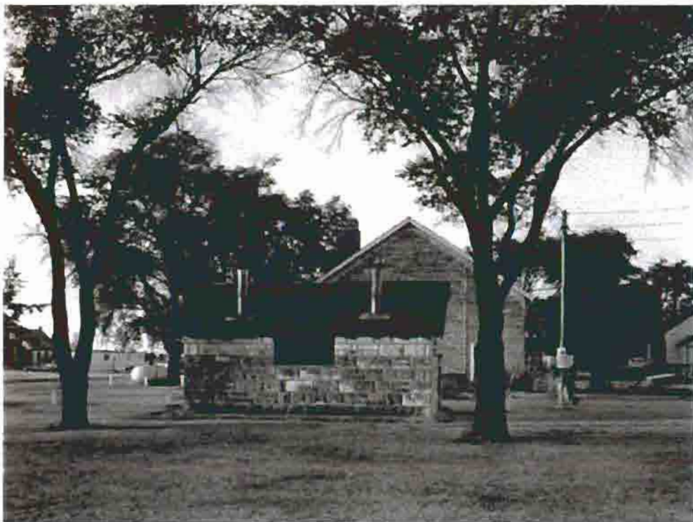
Photo T-6. The Township Hall, view from the north showing the original privy, 1983. HABS photo by Clayton T. Fraser.
