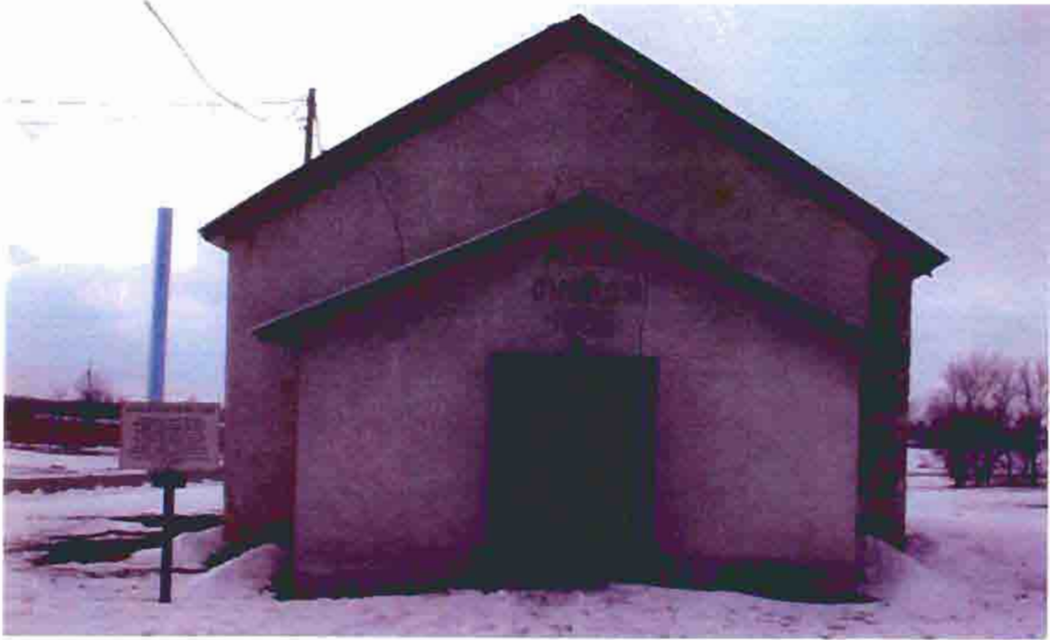
Photo A-11. The A.M.E. Church, east elevation, February 2001. Photo by Wiss, Janney, Elstner Associates, Northbrook, Illinois.
