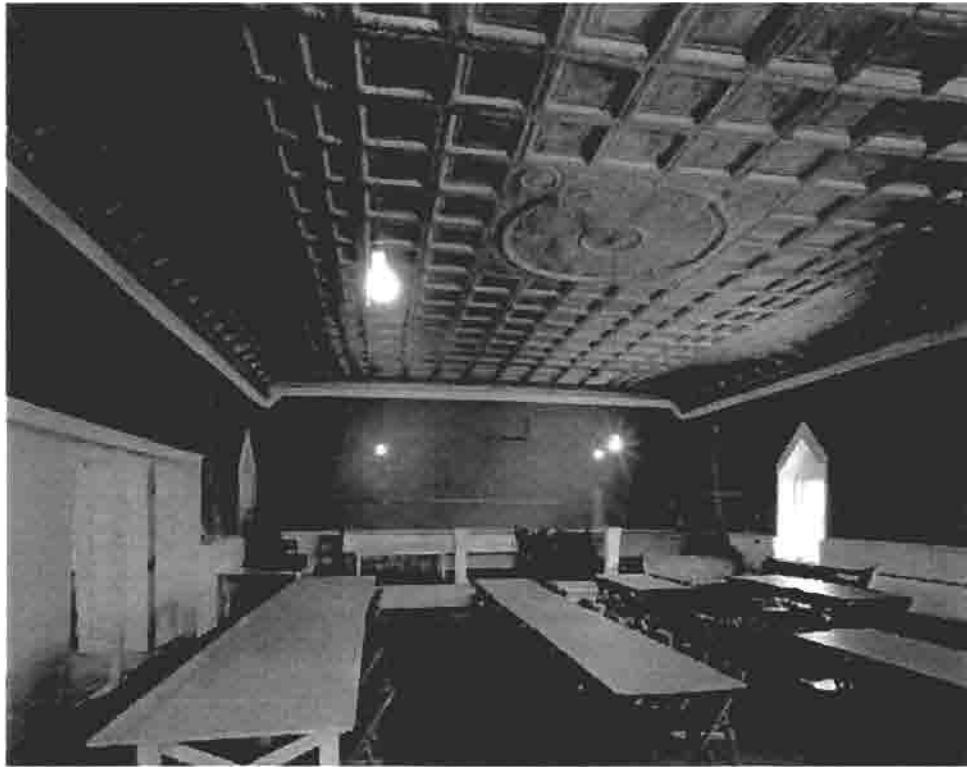
Photo B-11. The Old First Baptist Church, interior view, 1983. HABS photo by Clayton T. Fraser.
