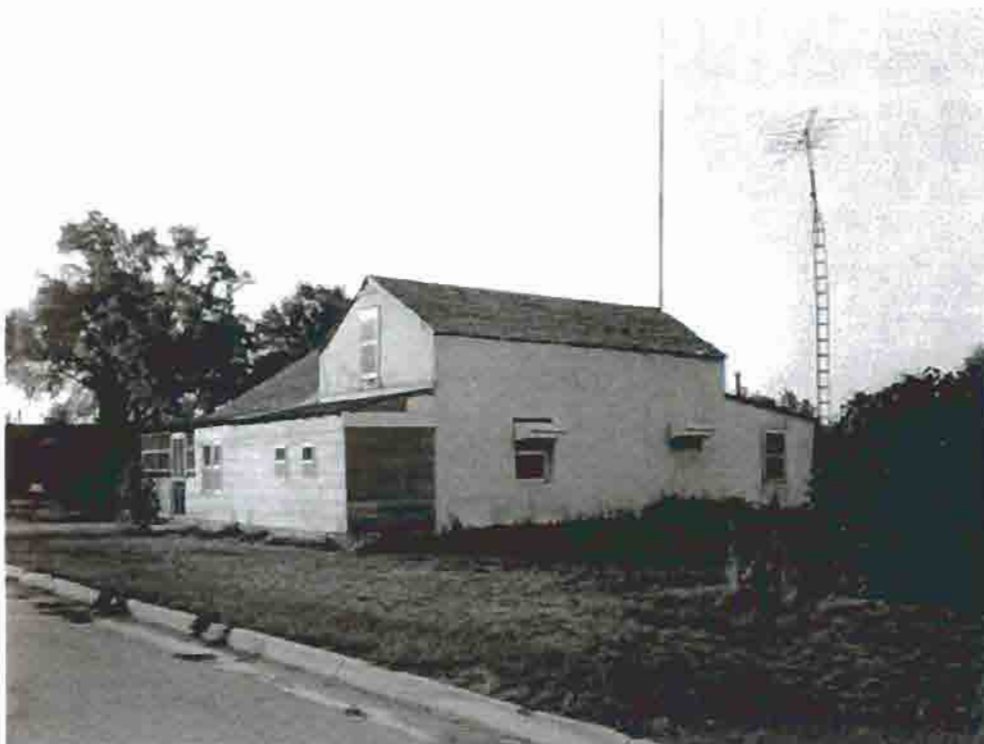
Photo F-7. The Fletcher-Switzer House, view from the northwest, 1983. HABS photo by Clayton T. Fraser.
