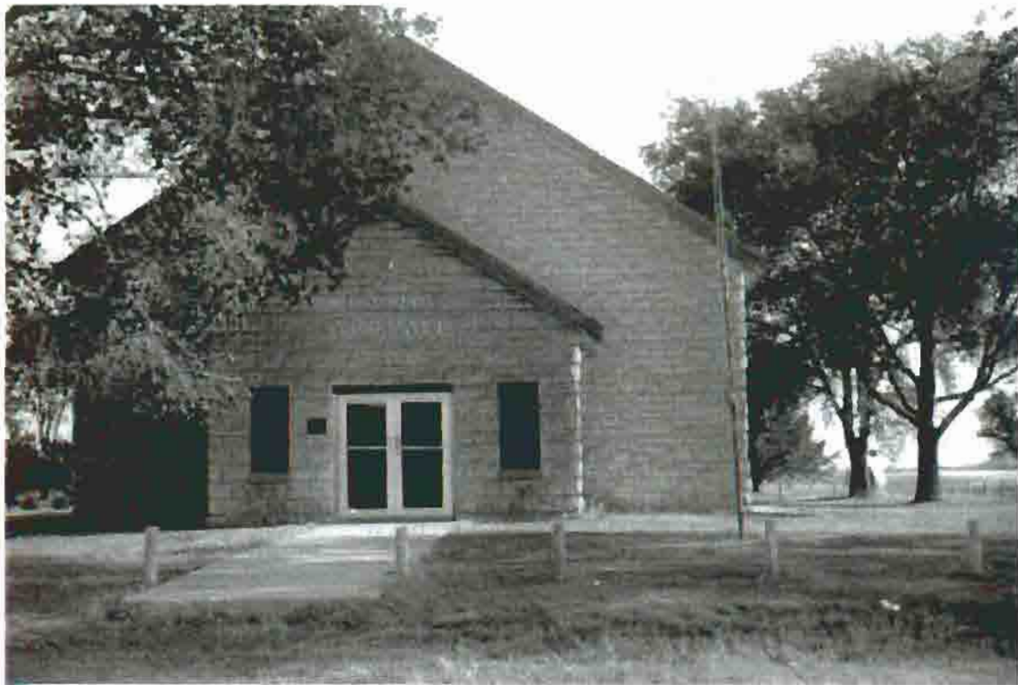
Photo T-4. The Township Hall, view from the south, 1977.
