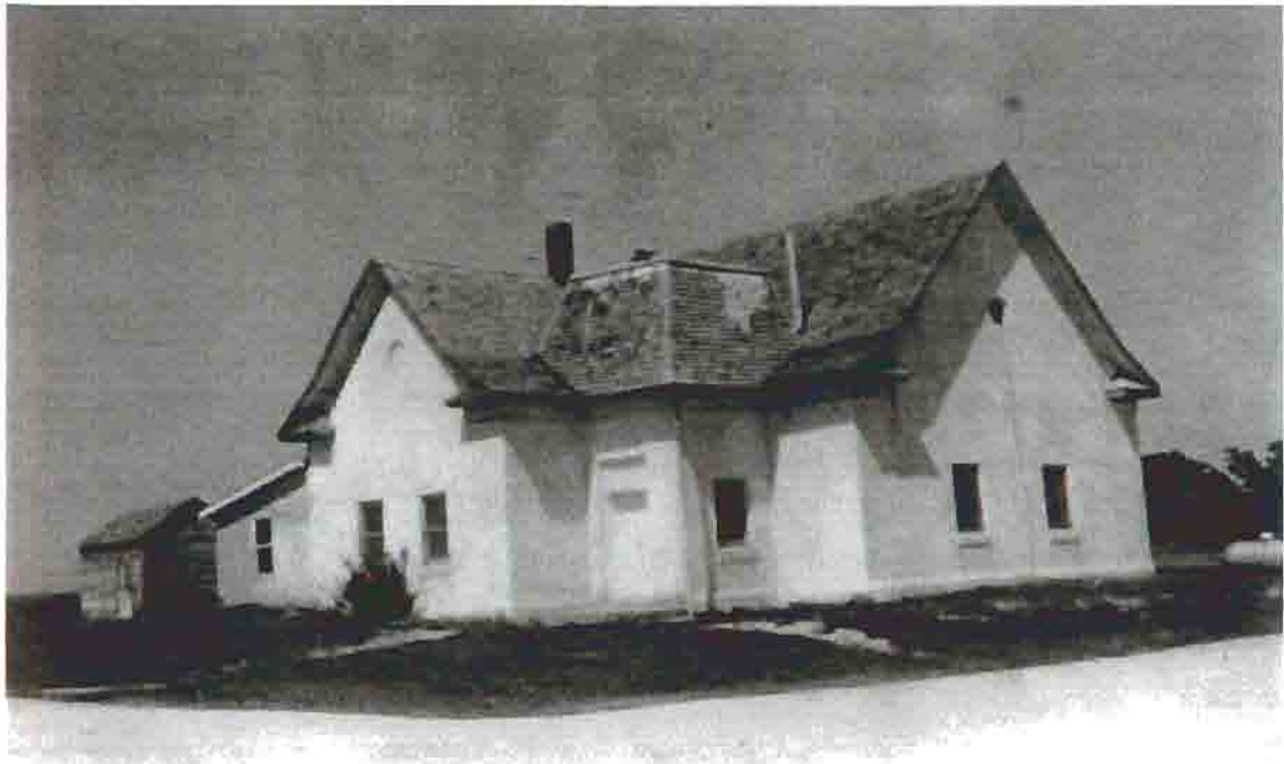
Photo B-7. The Old First Baptist Church, view from the southwest, circa late 1960s. Compared to Photo B-6, this shows the construction of the northwest Study addition. Historical Society collection.
