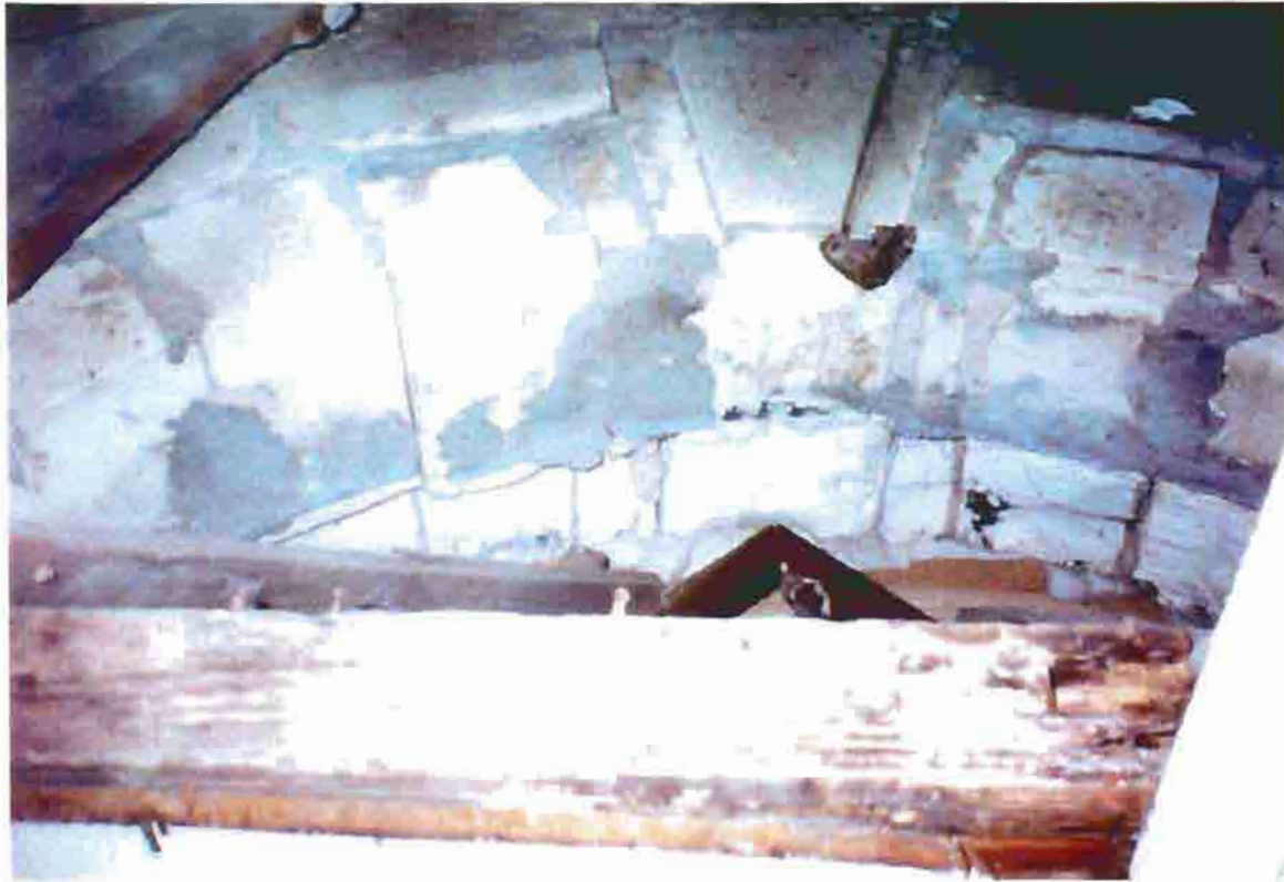
Photo A-27. The door between the sanctuary and east anteroom of the A.M.E. church, February 2001. The stone arch and keystone were originally visible on the exterior, when this doorway was the main entrance to the church. When the east anteroom addition was constructed, this doorway was lowered to accommodate the lower ceiling of the east anteroom (extreme foreground). Photo by Bahr Vermeer Haecker Architects, Lincoln, Nebraska.
