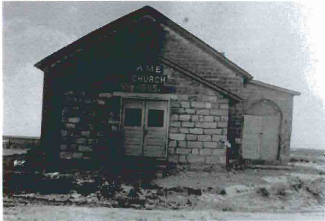
Photo A-1. The A.M.E. Church, view from the east showing the various additions to the original building, 1943. HABS photo by William T. Belleau.
