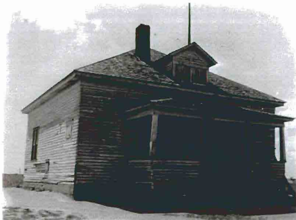
Photo S-1. The District No. 1 School, view from the southeast showing the original porch and dormer windows, 1943. Photo by William T. Belleau.
