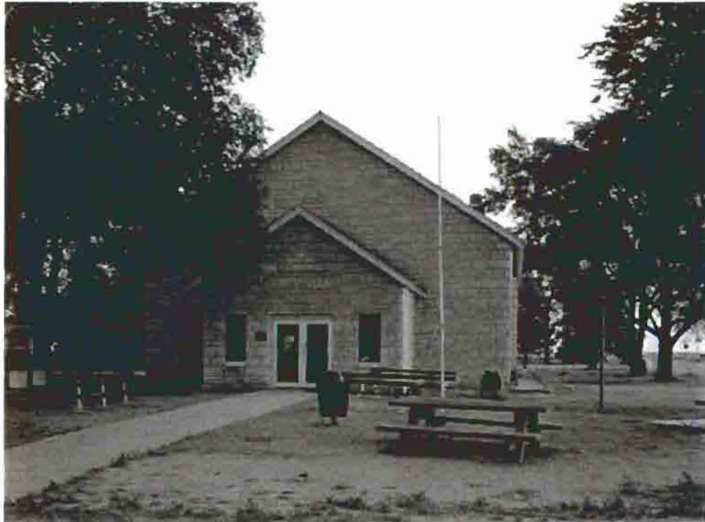
Photo T-5. The Township Hall, view from the south, 1983. HABS photo by Clayton T. Fraser.
