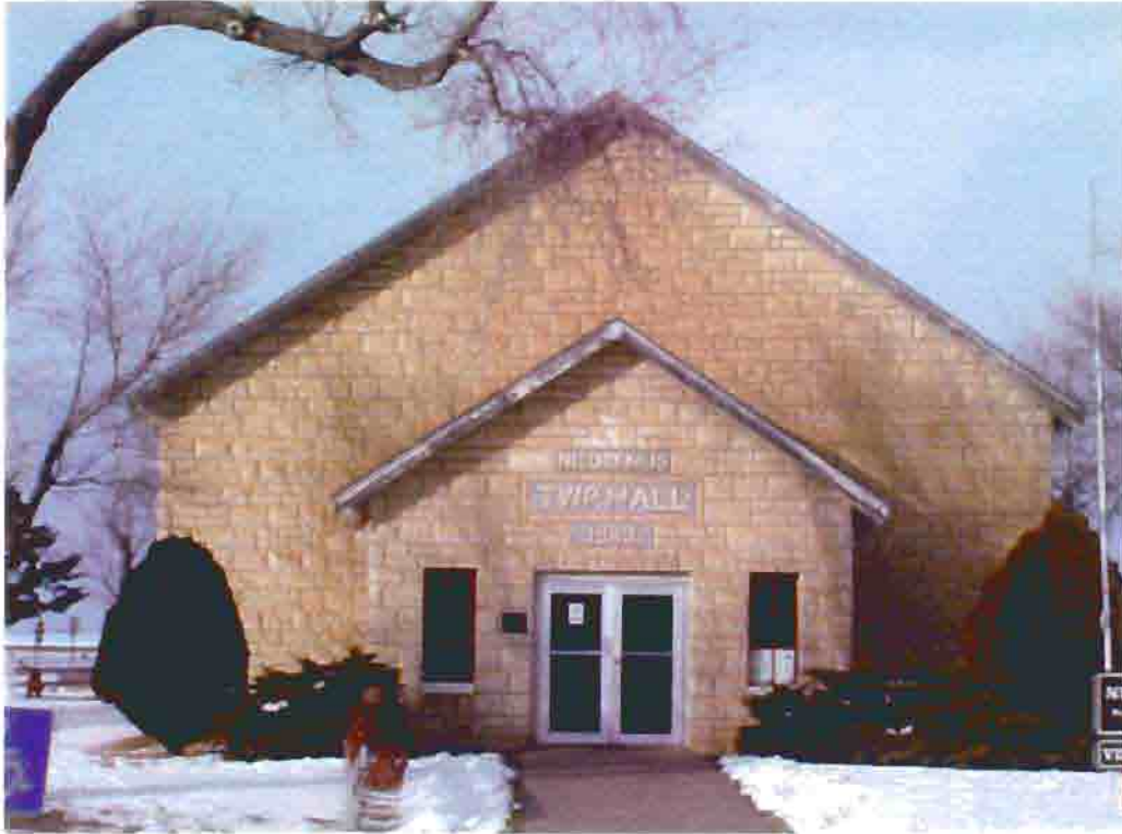
Photo T-9. The Township Hall, south elevation, February 2001. Photo by Wiss, Janney, Elstner Associates, Northbrook, Illinois.
