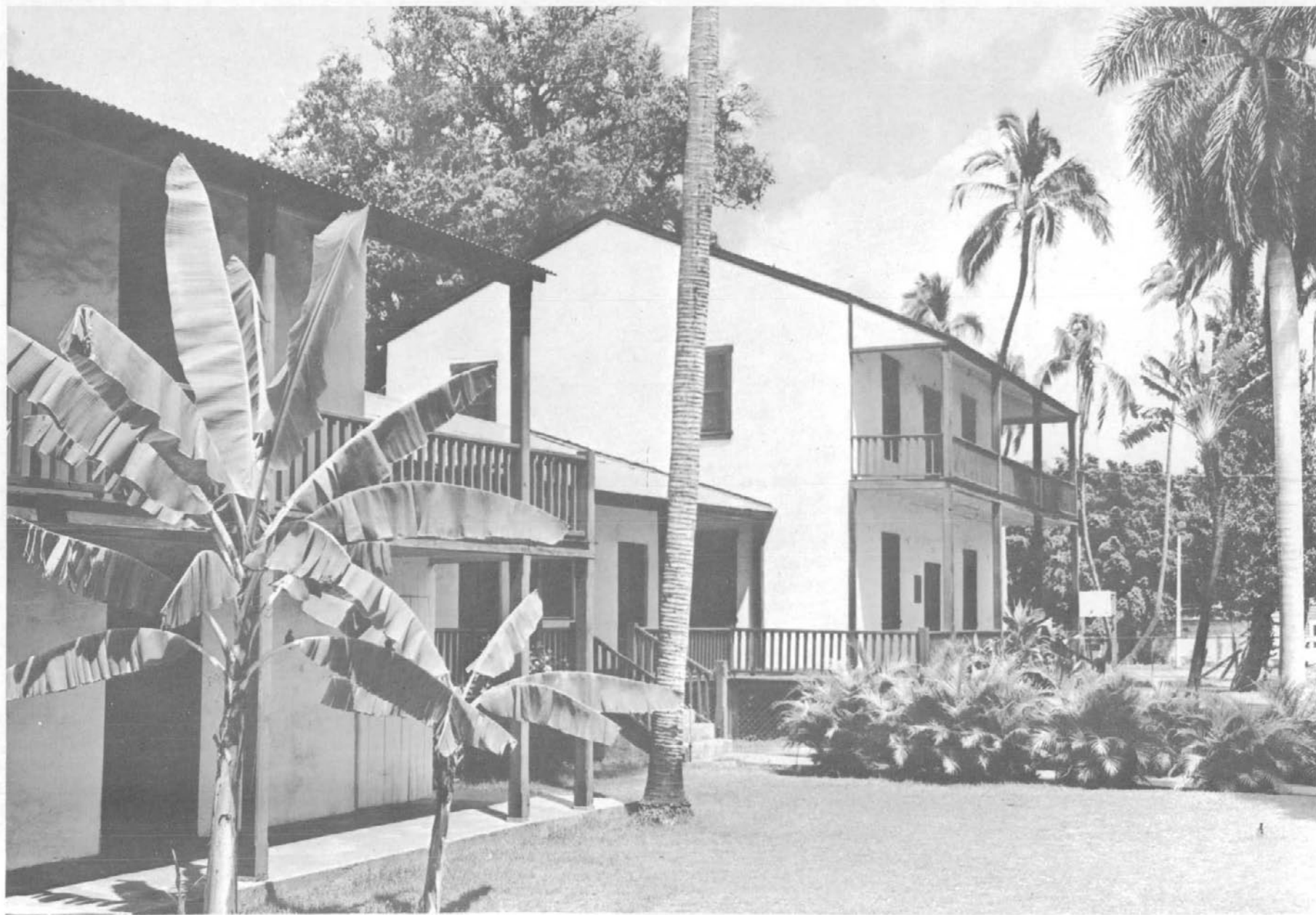
Baldwin House, Lahaina; the main house (right) was completed in 1835; wing (left) was added by Dr. Dwight Baldwin as a dispensary about 1847-9.
