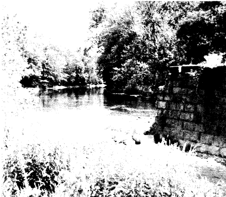
Remnant railroad abutment
