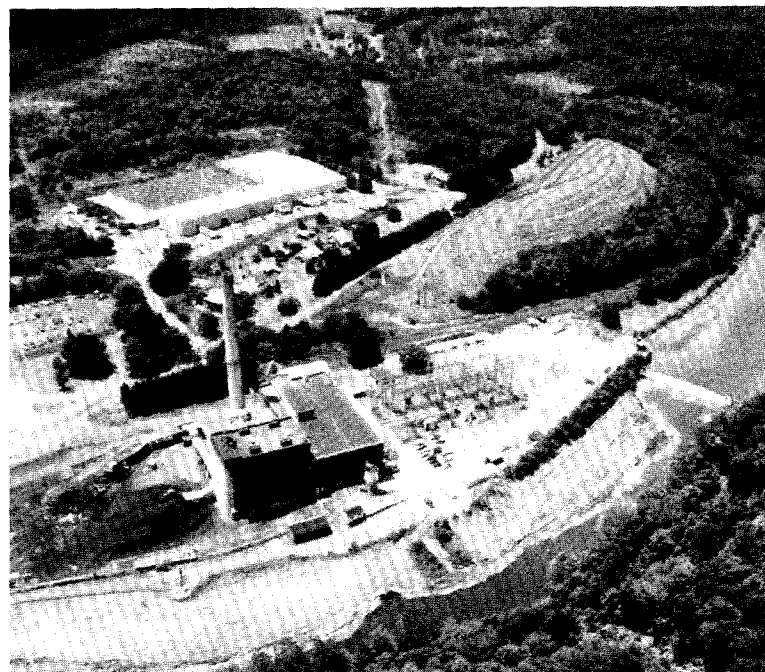
Williamsburg power plant
