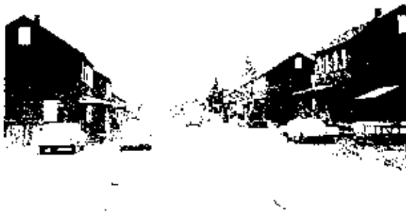
Figure 7-1 Anthracite miners' dwellings, built ca. 1850 in Eckley, Luzerne County, Pennsylvania. Houses like these were copied by coal companies in southwestern Pennsylvania, Maryland, Virginia, West Virginia and elsewhere. Courtesy of the National Register of Historic Places.
