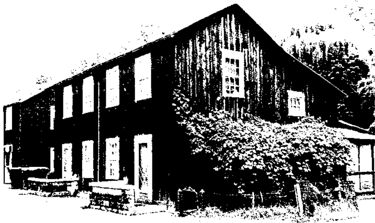
Figure 7-2 Semi-detached, vertical-plank miners' dwelling in Lonaconing, Maryland, built ca. 1840. Courtesy of the National Register of Historic Places, 1983.
