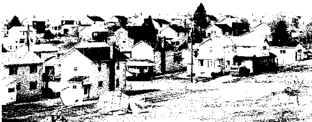
Figure 5-2 Four-room company houses built by the Ebensburg Coal Company in 1912. Taken by Jet Lowe, HAER photographer, 1988.
