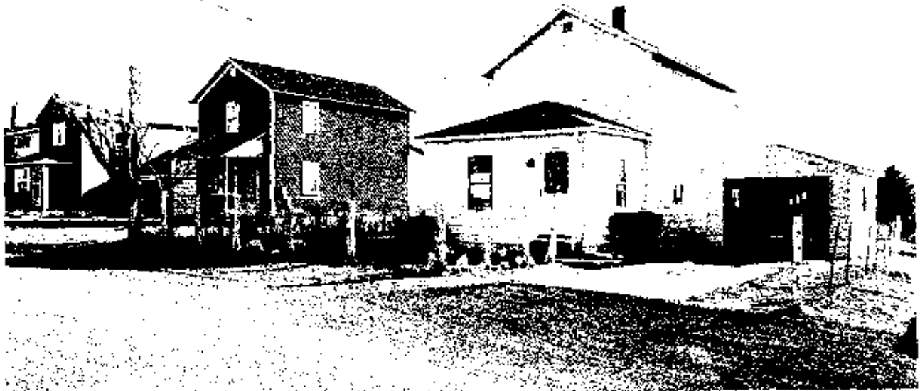
Figure 5-7 Four-room miner's houses built in 1911-12.
