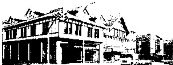
Figure 4-6 View of main Eureka Department Store, dating from 1899 and standing on the east corner of 15th Street and Somerset Avenue.
