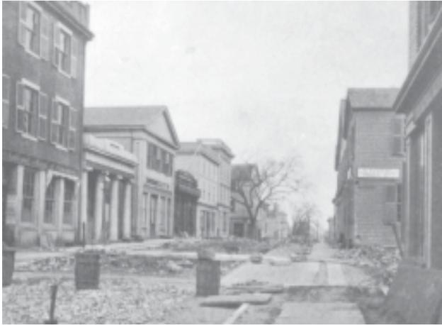
Figure 50: North Water Street, looking north from Union Street, mid-1860s. Excavations during the installation of the municipal water system temporarily interrupted traffic along New Bedford's "Wall Street." Many typical elements of the waterfront streetscape, including granite runners, hitching posts, and gas lamps, are visible. The elm for which Elm Street is named, seen at center, was one of the few street tree plantings in the Four Corners area.
