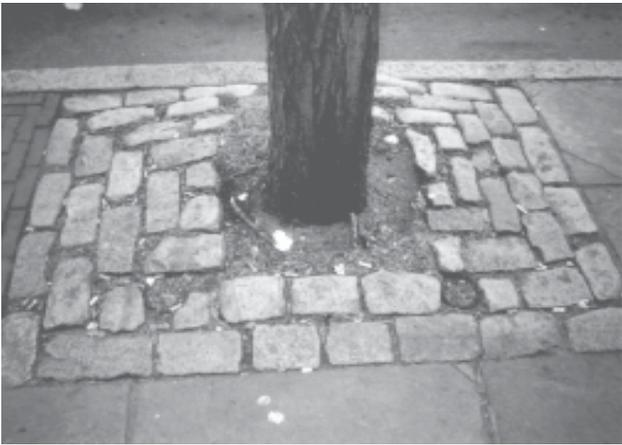
Figure 142: Belgian block used as paving over tree pits, 1997.
