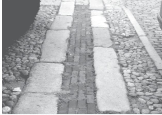
Figure 144: Granite runners on Centre Street sidewalk, 1997.
