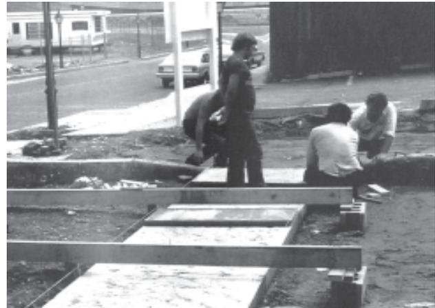
Figure 129: Sidewalk reconstruction on Centre Street, ca. 1976. Working with WHALE, architect Tom Hauck designed a patchwork of brick and cobblestone sidewalks to reflect the character of individual buildings within the district.
