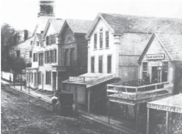
Figure 31: William Street, looking west from Purchase Street, ca. 1852. The cobblestone paving and bluestone sidewalks were probably installed in the mid-1840s. The entire block was cleared by 1856, when construction of the Free Public Library (now City Hall) began. Some buildings, including the one at center that now stands at the southwest corner of Eighth and William Streets, were relocated.
