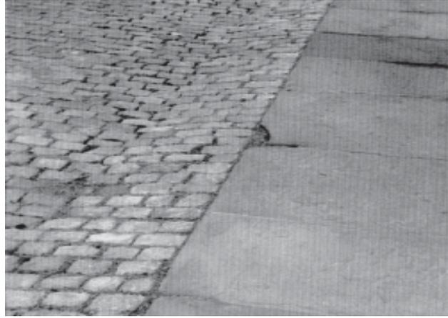
Figure 145: Flagstone panels used in sidewalk paving, 1997.
