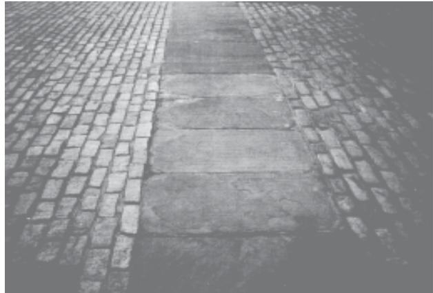
Figure 146: Flagstone panels used in crosswalk, 1997.
