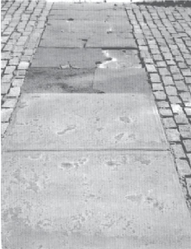
Figure 147: Concrete formed to resemble flagstone paving, 1997.
