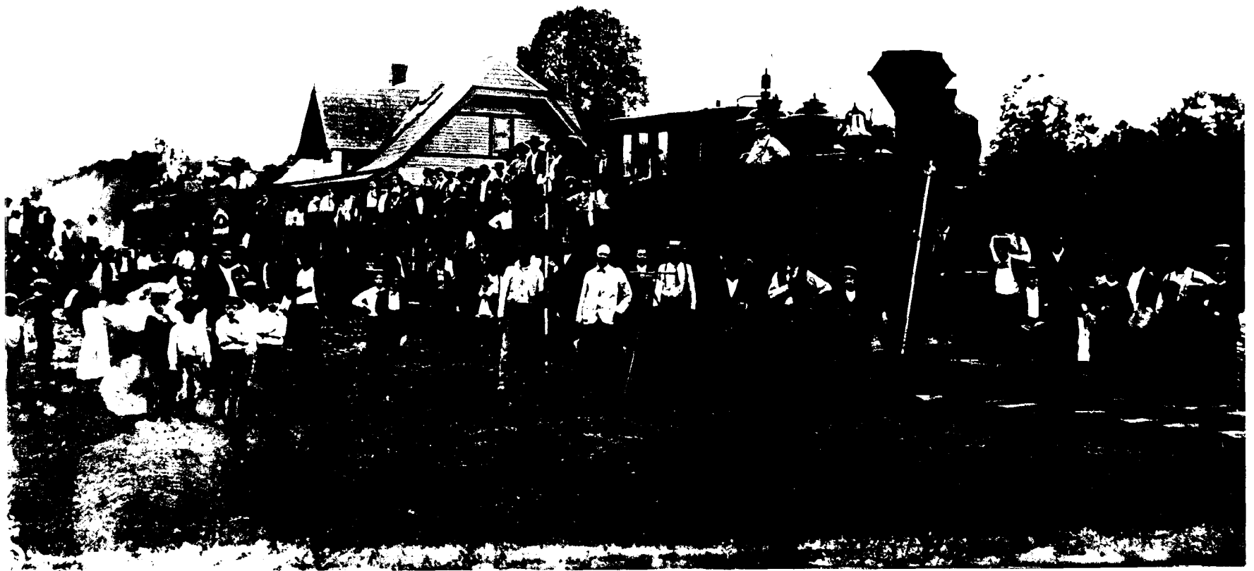
46. Railroad depot at Briel Avenue.
