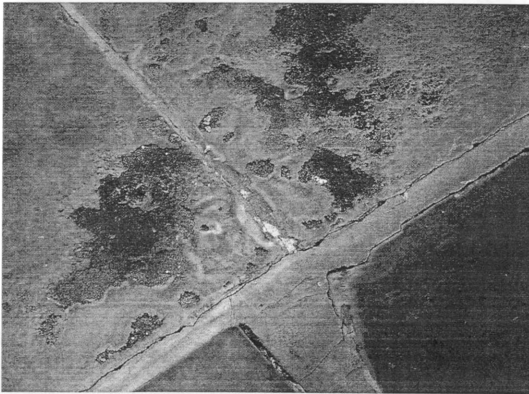
Between the bases of the columns, the marble floor is darkly stained. Areas of encrustation are pronounced in these locations. [JGWA, 2005]
