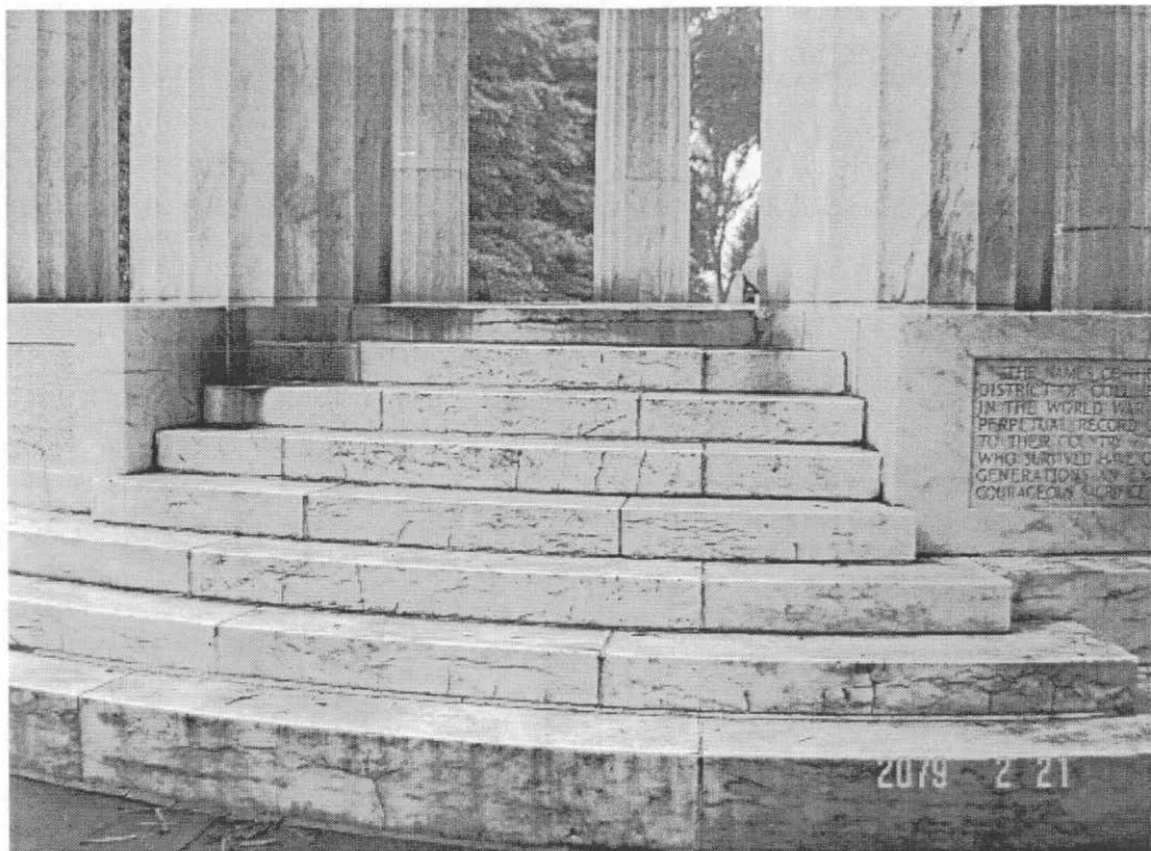
In the marble base and stairs, the cracks are predominantly horizontal. [MSSC, 2005]
