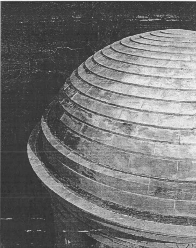
Views of the dome from the south, looking northeast (upper photo) and northwest (lower photo). Note the shallow gutter construction in the protruding cornice. [JGWA, 2005]
