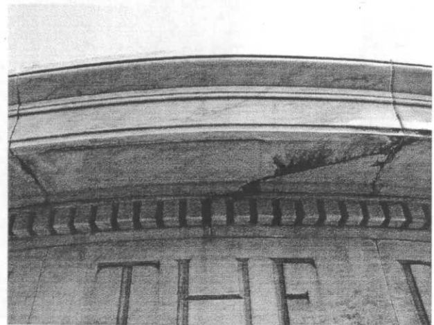
Photo 9. Crack extending from right joint to center of the cornice soffit.
