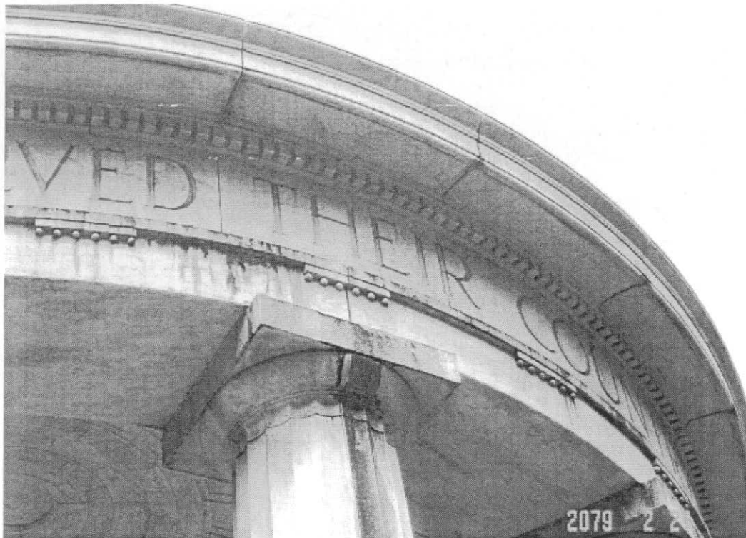
Mortar is missing and deteriorated in many locations on the entablature. [MSSC, 2005]
