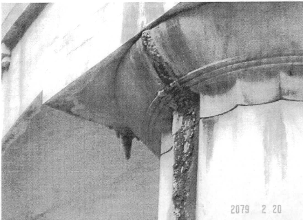
Stalactite on base of entablature. [MSSC, 2005]
