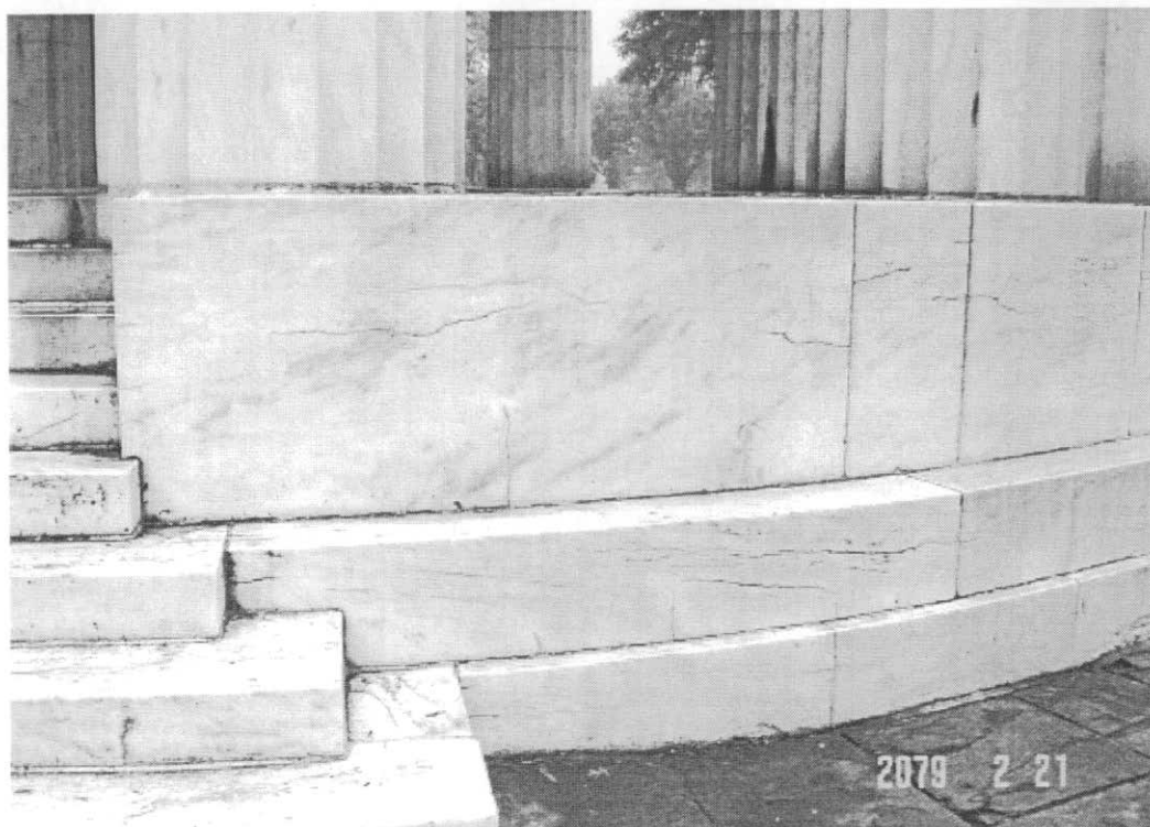
Dark-colored biological growth is present on marble in shaded areas. The blocks exhibit surface cracking. [MSSC, 2005]
