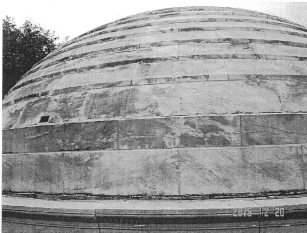
The marble of the dome exhibits dark mottling. [MSSC, 2005]
