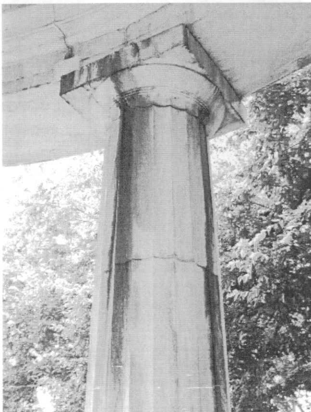
Vertical staining on interior of column. [MSSC, 2005]
