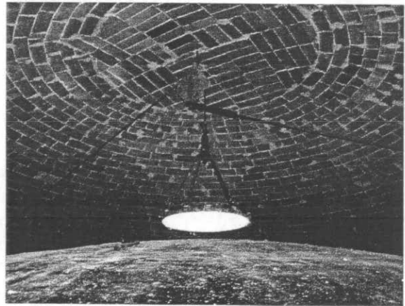
Photo 4. Interior surface of outer dome and counterweighted ceiling oculus.
