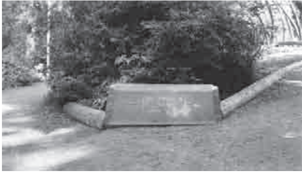
Figure 4.65: The intersection of the main trail (left) and south approach to the Administration-Operator Building illustrating log edging and sign installed in May 1941. Walter Finn, May 1941 monthly report. National Archives II, College Park, Maryland, RG 79, PI 166, E7, Central Classified Files, 1933-1949, Muir Woods, box 2293.
