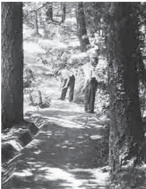
Figure 4.42: CCC/CWA crews at work on the Dipsea Trail through the northwestern corner of Muir Woods, June 1934. Note drainage swale along left side of trail. J. Barton Herschler, Muir Woods June 1934 monthly report. National Archives II, College Park, Maryland, RG 79, PI 166, E7, Central Classified Files, 1933-1949, Muir Woods, box 2293.
