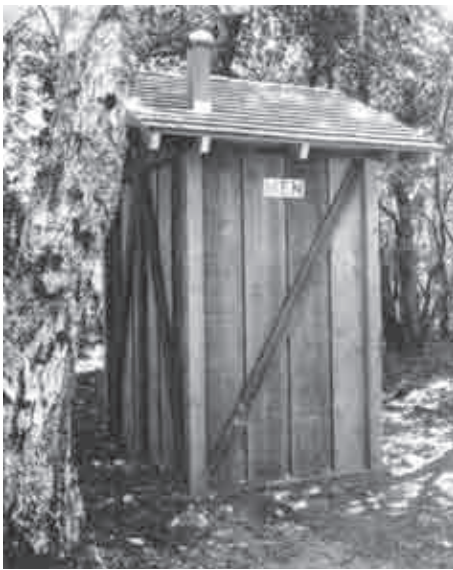
Figure 4.43: One of two matching dry pit toilets built at the Deer Park area off the Dipsea Trail, June 1934. J. Barton Herschler, June 1934 monthly report. National Archives II, College Park, Maryland, RG 79, PI 166, E7, Central Classified Files, 1933-1949, Muir Woods, box 2293.
