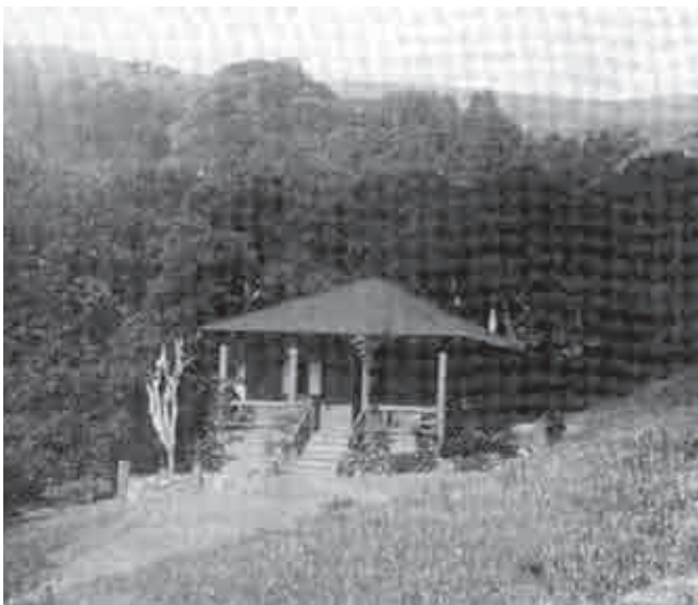
Figure 2.16: Stolte cottage in Homestead Valley, built in 1905, illustrating local use of rustic design with log and branch columns and porch railings, photographed c.1910. Courtesy Lucretia Little History Room, Mill Valley Public Library, Mill Valley, California.
