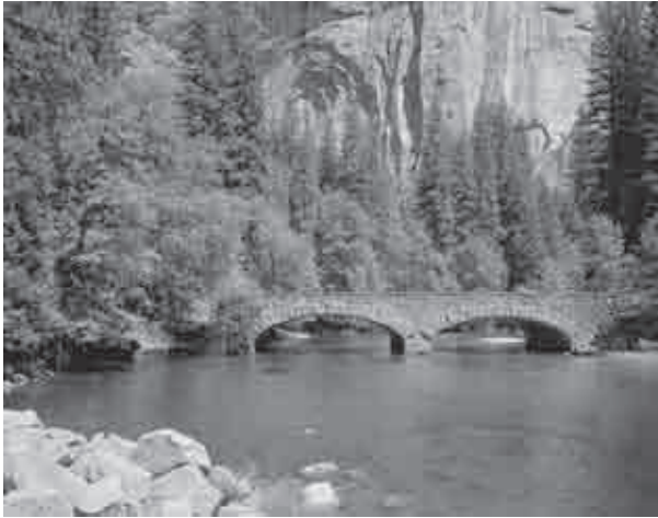
Figure 4.24: The Ahwahnee Bridge over the Merced River (1928), illustrating use of modern construction (concrete) beneath a rustic skin of stone veneer characteristic of mature phase of rustic design in the NPS, photographed 1991. Historic American Engineering Record, CAL 22-YOSEM, 21 (CA-100).
