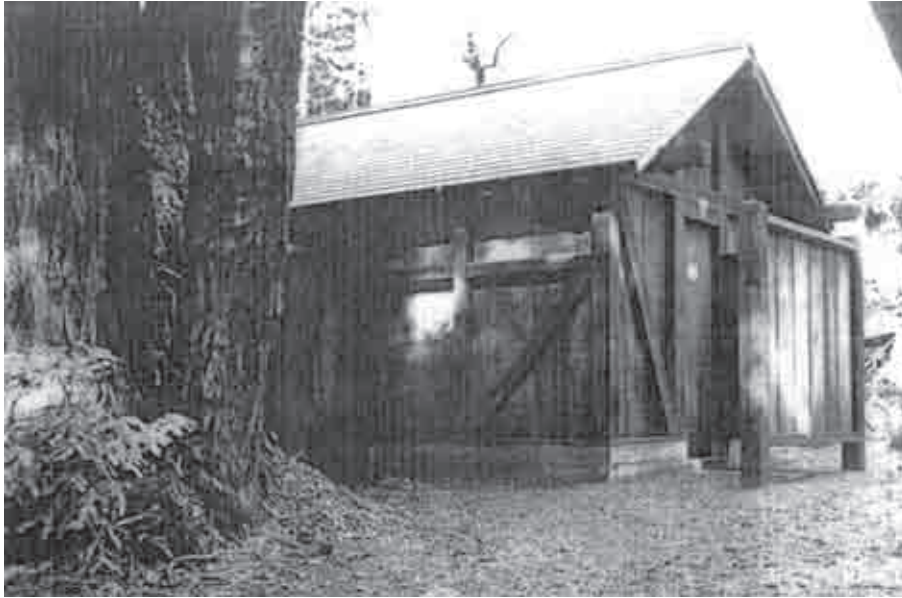
Figure 3.43: The first modern comfort station at Muir Woods, built in 1928 along old Muir Woods Road (service drive) near the lower picnic area, using similar but more prominent exposed timber-frame detailing as used on the Custodian's Cottage, photographed December 16, 1928. This building was later known as the main comfort station. Courtesy Golden Gate National Recreation Area, Park Archives, GOGA 32470 B36, Muir Woods Collection.
