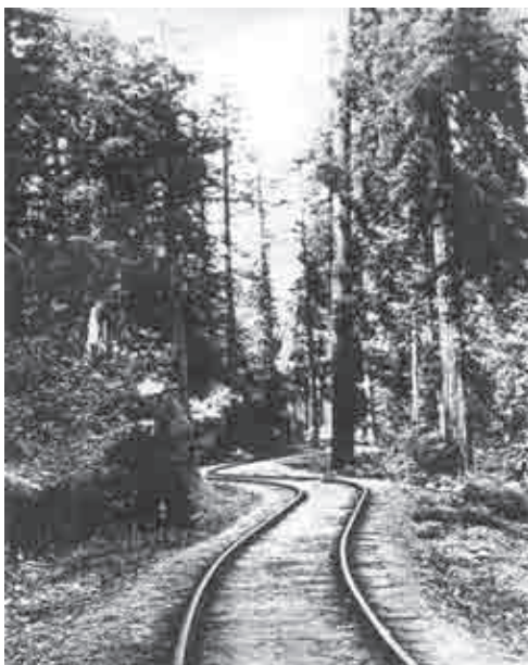
Figure 2.18: The Redwood Canyon branch line of the Mill Valley and Mt. Tamalpais Scenic Railway, illustrating narrow, twisting alignment through the forest, c.1910. Courtesy Ted Wurm Collection, published in Ted Wurm, The Crookedest Railroad in the World (Interurban Press, 1983).
