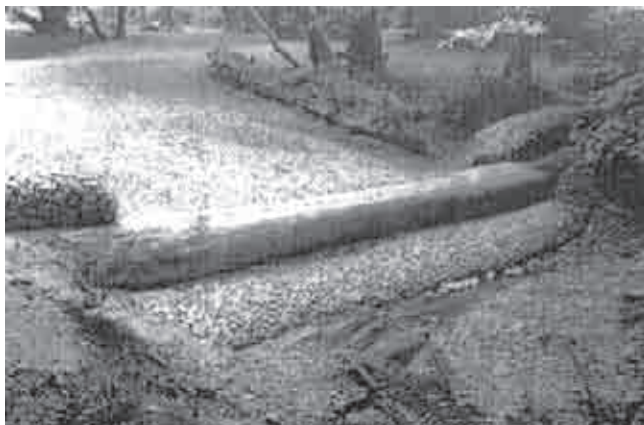
Figure 4.32 (left): Log check dam in Redwood Creek near the Emerson tree during construction, September 20, 1932. The log had a diameter of 36 inches. Courtesy Golden Gate National Recreation Area, Park Archives, box 35/5, Muir Woods Collection.
