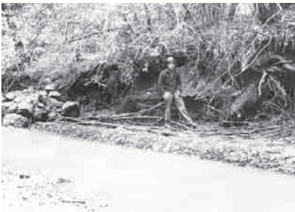
Figure 4.38 (below): Erosion around old basket-type revetment, photographed 1937. The identity of the person is not known. J. Barton Herschler, April 1937 monthly report. National Archives II, College Park, Maryland, RG 79, PI 166, E7, Central Classified Files, 1933-1949, Muir Woods, box 2293.
