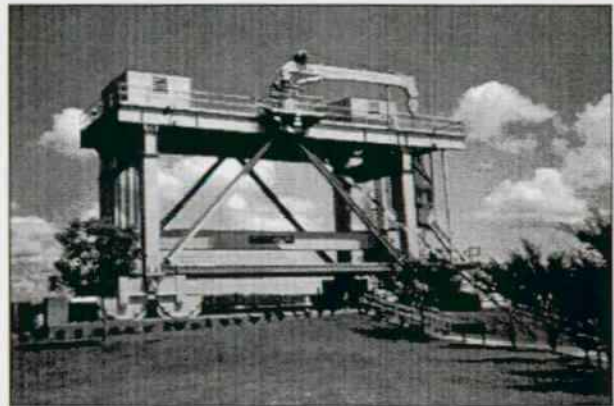
▲ U.S. Army Corps of Engineers Diversion Control Structure
