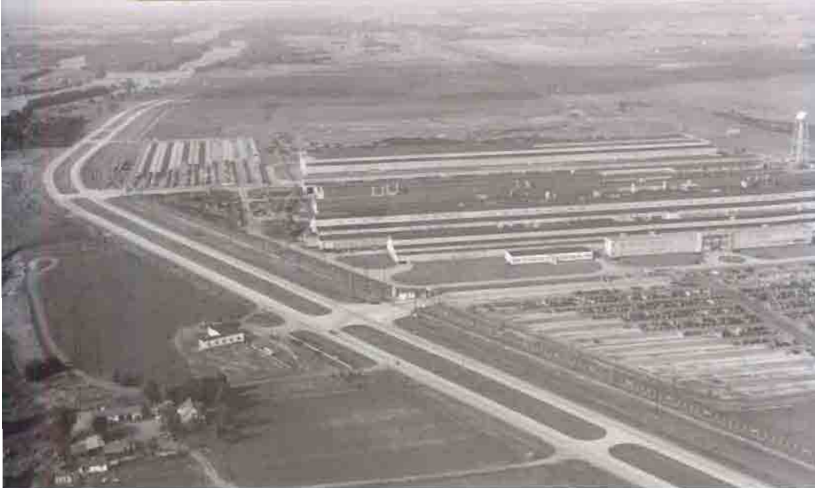
FIGURE 6. East River Road, Fridley, 1945. The Northern Pump Company is the large building complex. Minneapolis Star Journal Tribune Photograph, Minnesota Historical Society.
