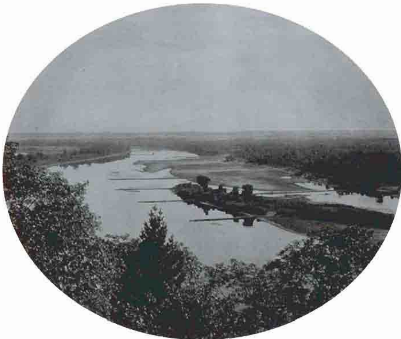
FIGURE 10 Channel construction at Pine Bend, Minnesota, 1891. Photo by Henry P. Boss, St. Paul District, Corps of Engineers.
