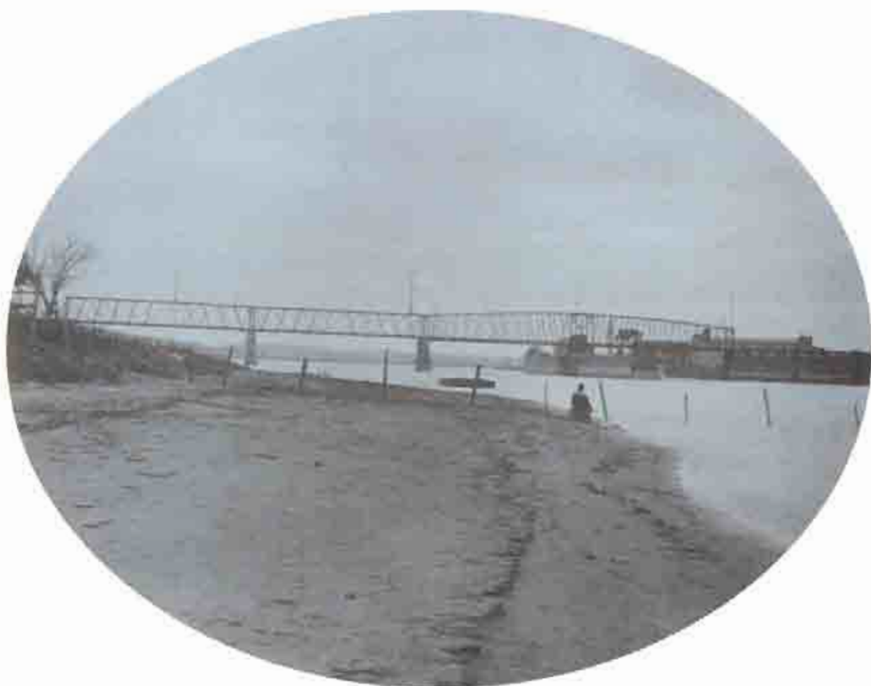
FIGURE 5. Chicago, Milwaukee & St. Paul Railroad Bridge, Hastings, Minn., 1905. By Henry P. Basso. Rock Island District, Corps of Engineers.
