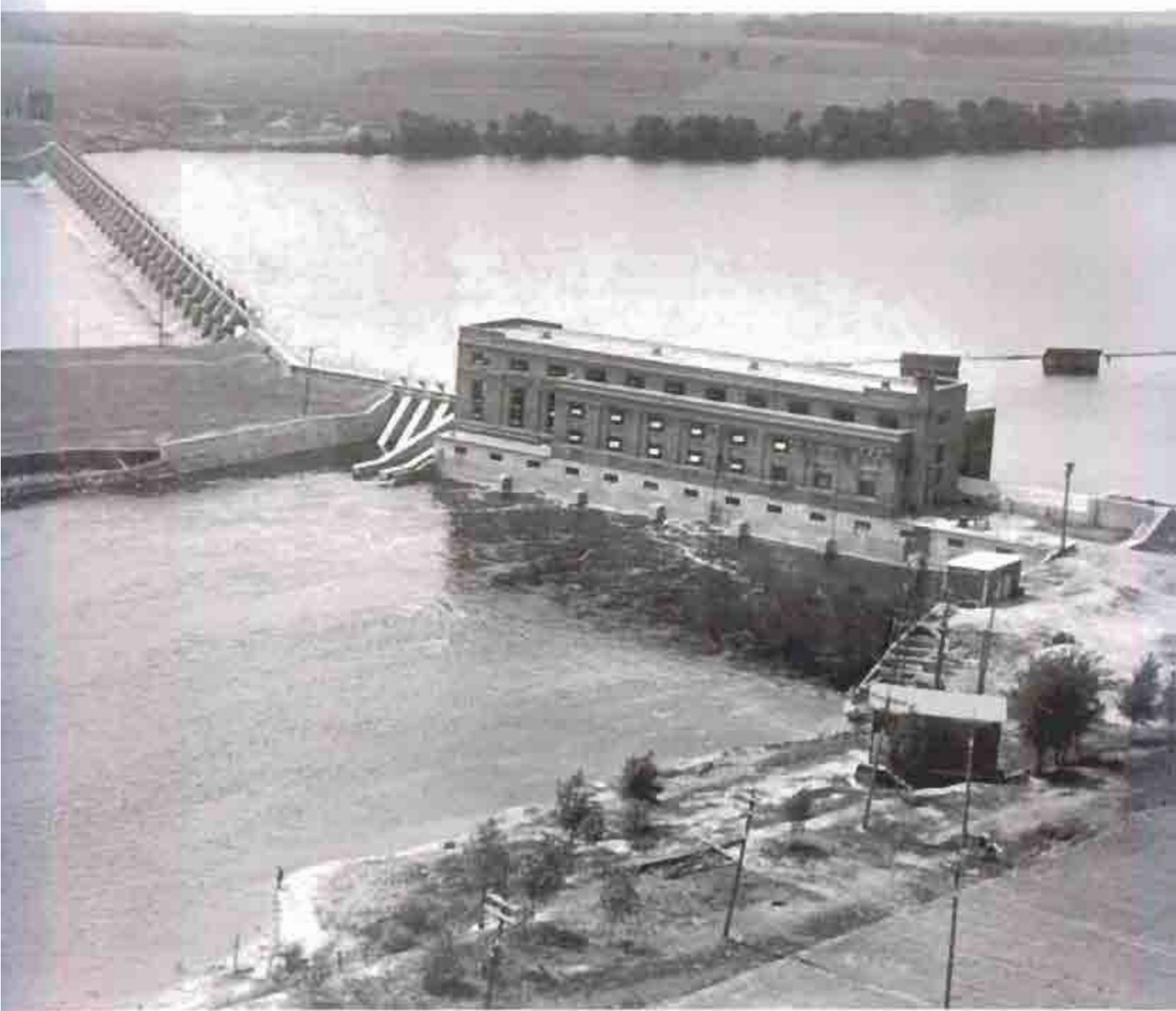
FIGURE 2.1 Crook Rapids Dam and Power Plant, 1928. Photo by Paul Hamilton. Minnesota Historical Society.
