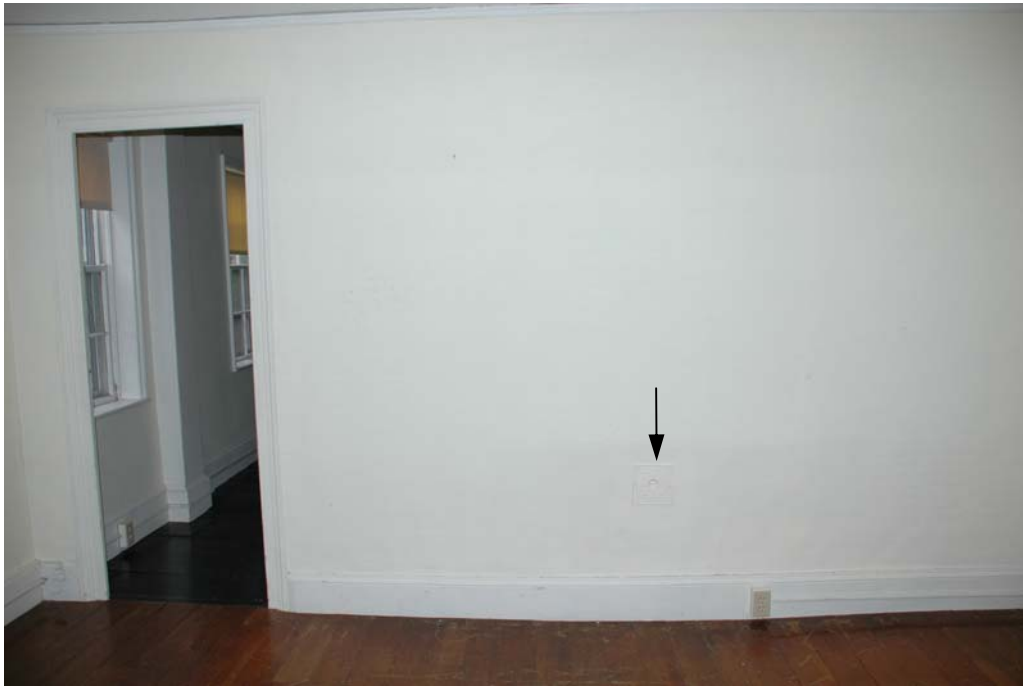
Figure 207-4. West elevation of Room 207 with Door 1/208 that leads to Room 208. The floor sags in the middle, at the possible location of a stove heater. The former stove vent plate is found on the wall above this area, now painted over (see arrow).
