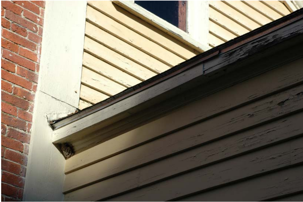
Figure SE-21. Deteriorated roof cornice at northeast wing.
