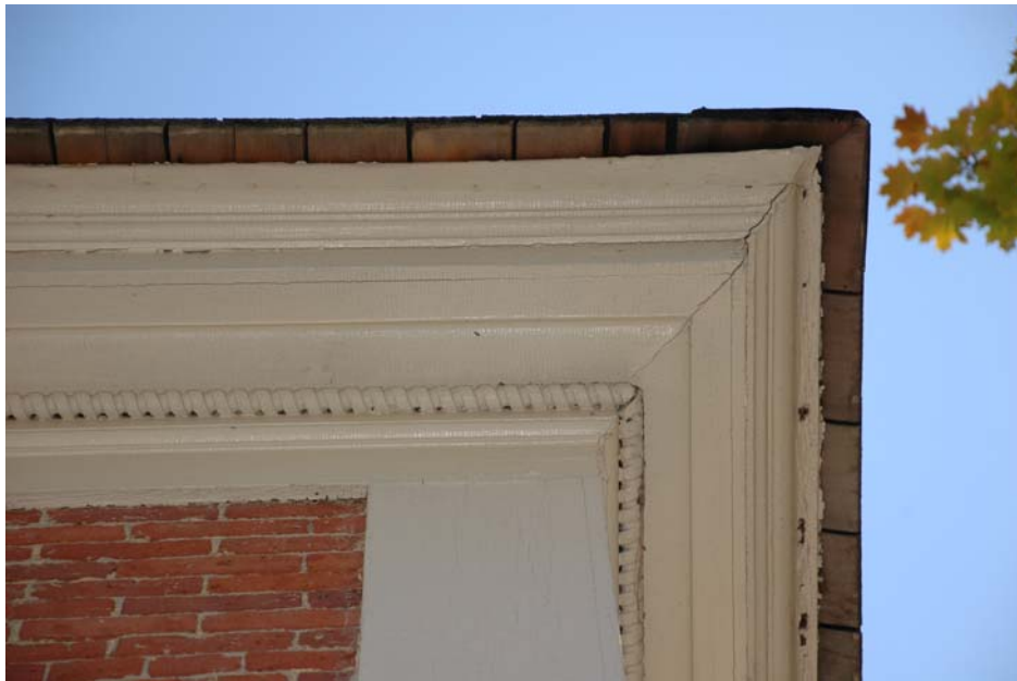
Figure 1.3A-9. John Nelson House eave cornice at the main block.
