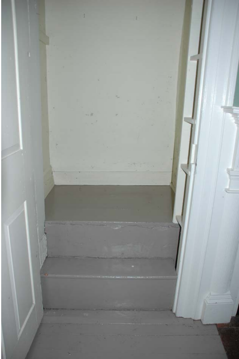
Figure 104-5. Room 104, detail of closet interior showing the remaining masonry base of the original removed bake oven in Room 106. The bottom riser and tread are wood and the top riser is the painted face of the masonry with wood boards applied to the top. The remnants of cut-off shallow shelves are visible behind the right door jamb.
