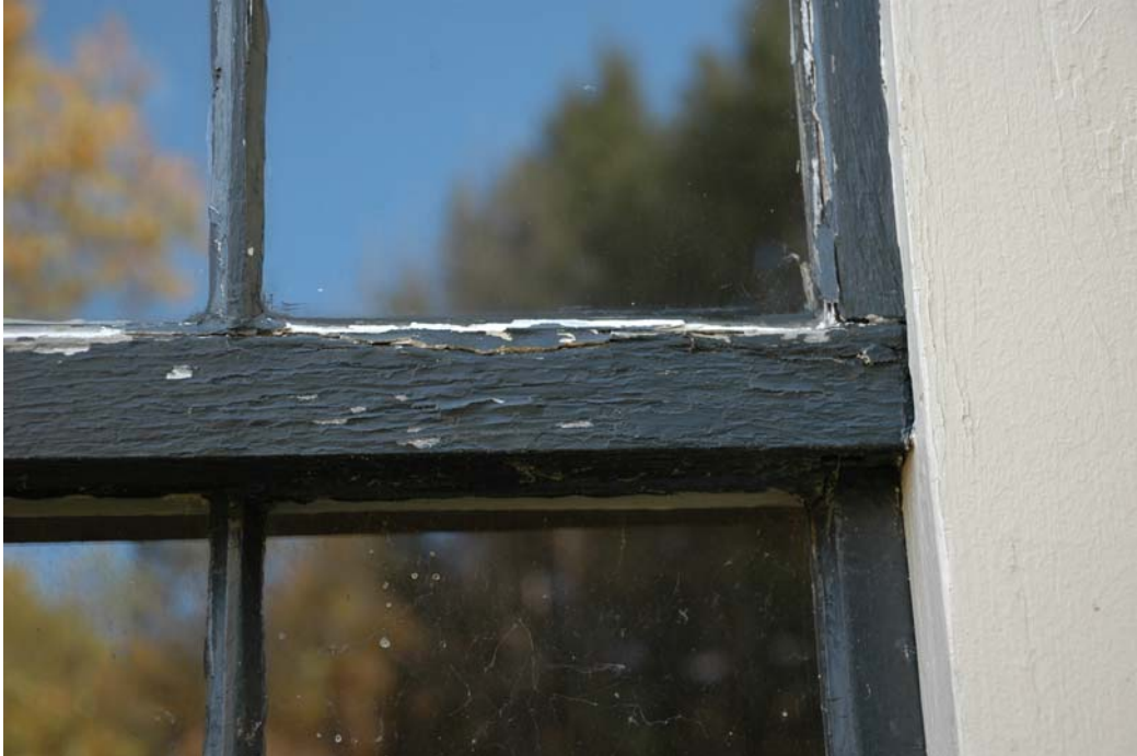
Figure NE-14. Detail of deteriorated wood sash at Window #112.
