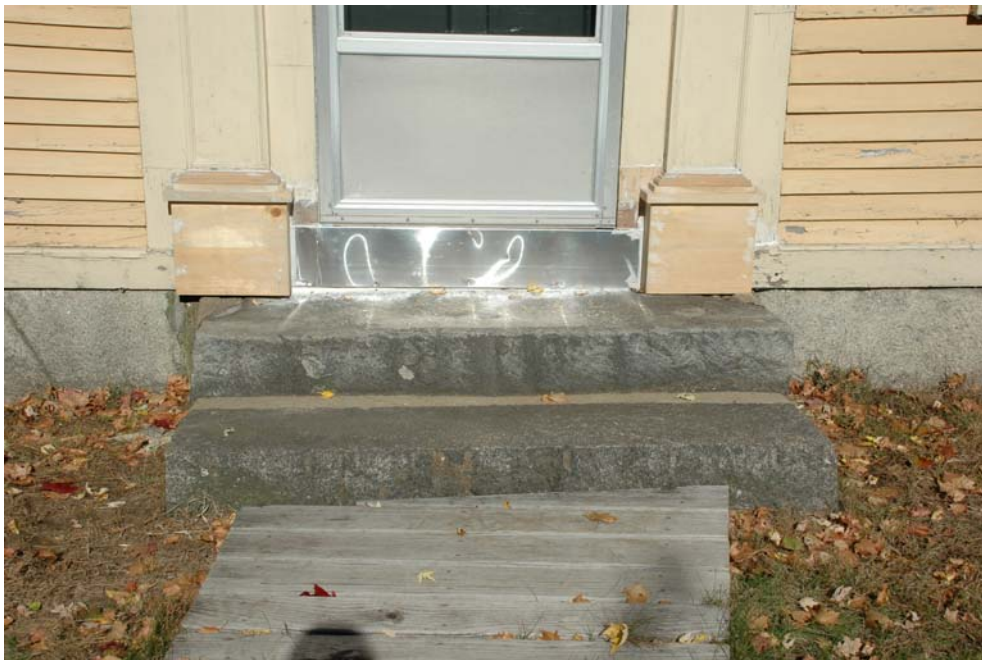
Figure 1.3A-18. Granite slab foundation walls and steps at Door 1/101.
