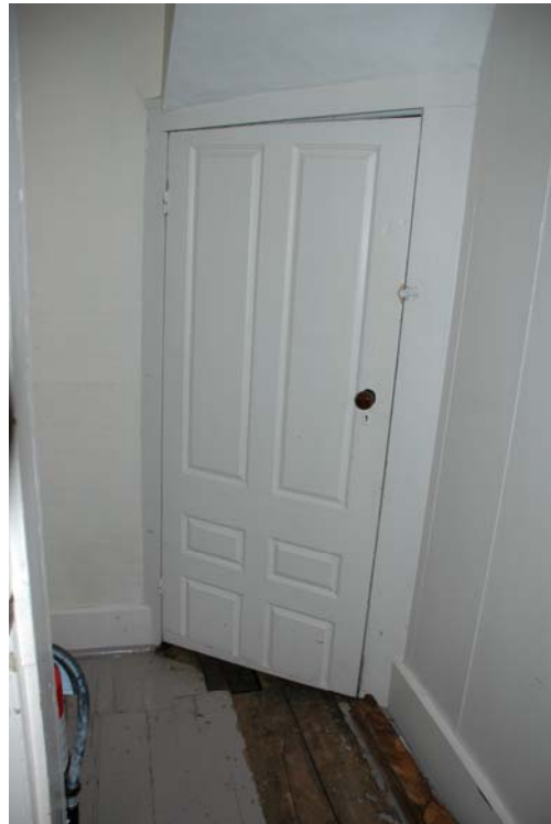
Figure 205-5. North and east elevations of Room 205 with Door 1/205 that leads to the attic, Room 209. The door leaf has been modified to accommodate the sloping floor.
