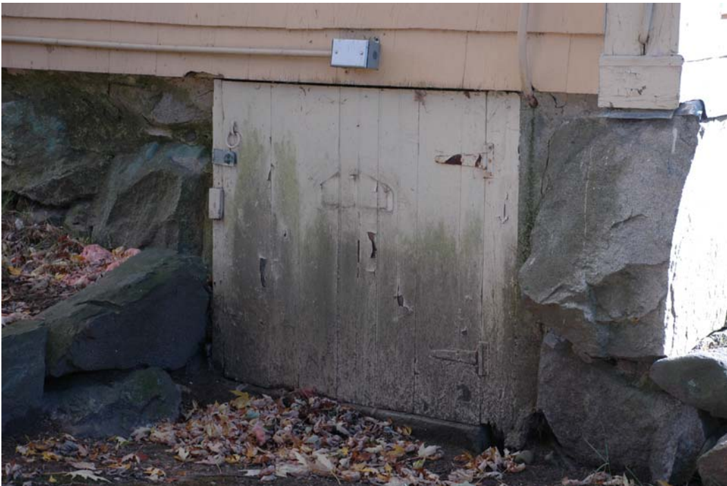
Figure NE-12. Door 1/003: exterior entrance to basement Room 003.
