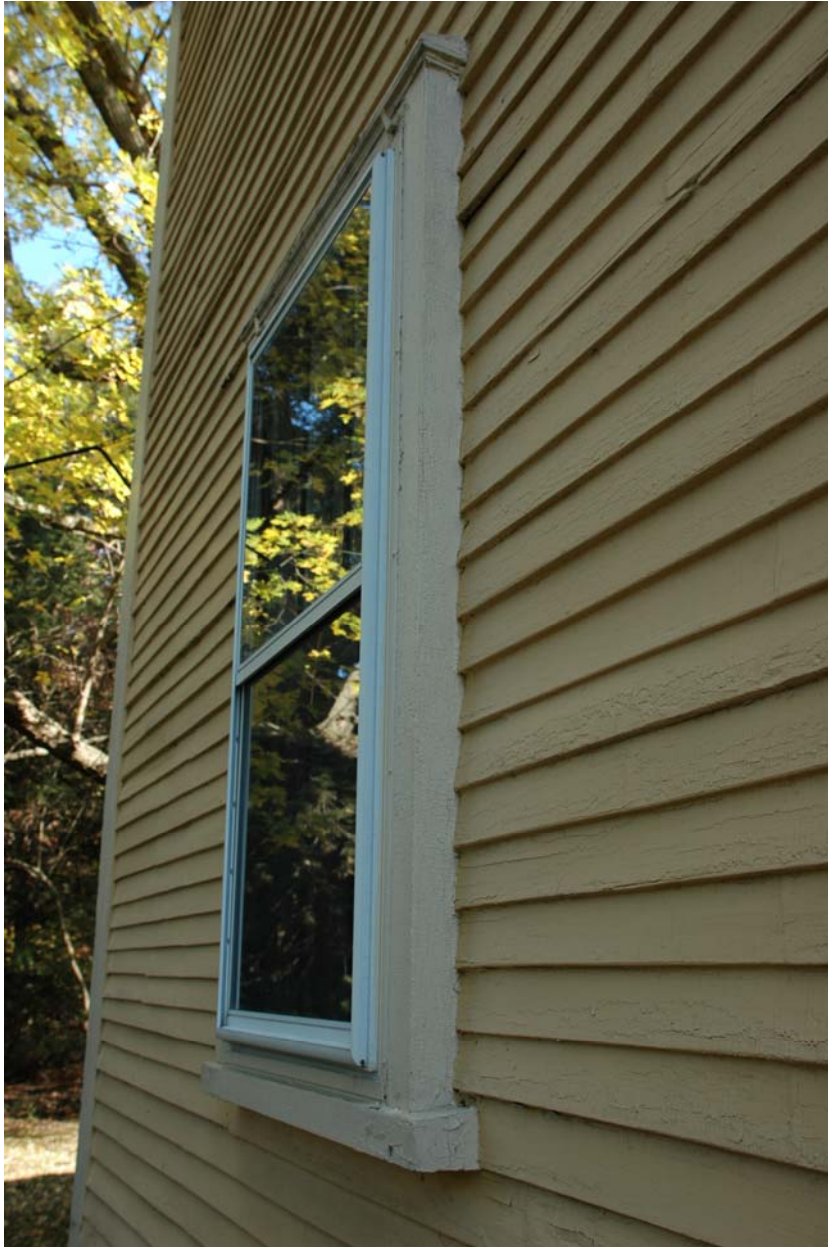
Figure SE-16. Window Type w-A: 6-over-6 double hung window with flat board trim and cornice. An aluminum triple-track storm window is attached to the wood frame. This window type is found at the south, west and north elevations of the northwest wing. On the south elevation Type w-A is found at #101, 102, 201, 202, & 203.
