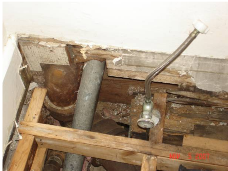
Figure S-7. Sister beam and cut beam at northeast corner.
