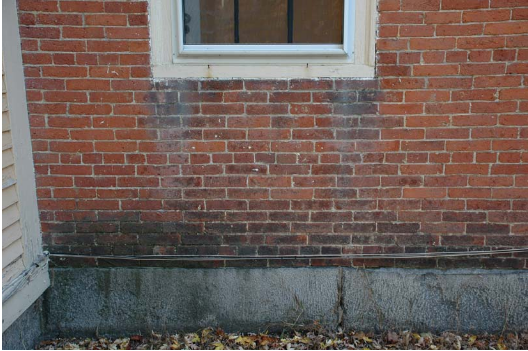
Figure WE-6. Granite slab foundation and brick wall at west elevation of main block. Brick wall and stone foundation wall exhibit significant water staining.
