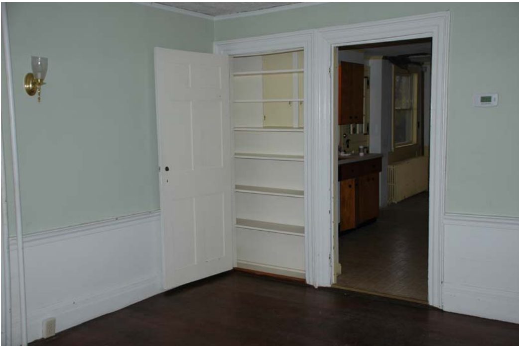
Figure 106-4. North and east elevations of Room 106. Door 3/106 is on the left and Door 4/106 is on the right. Door 4/106 leads to Room 107 and is missing a door leaf (the pintel hinges and latch receiver are still intact).
