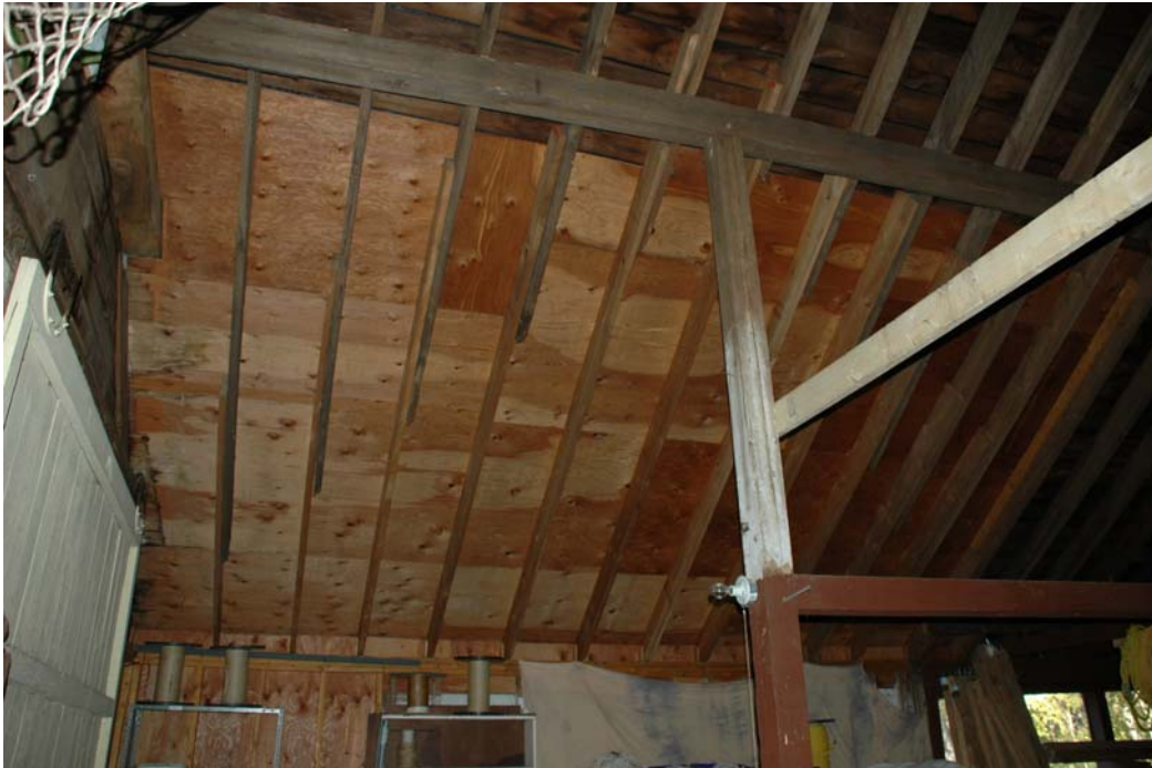
Figure B102-3. Room B-102, looking west at the ceiling. The plywood roof sheathing and sistered rafters were installed in 1979.
