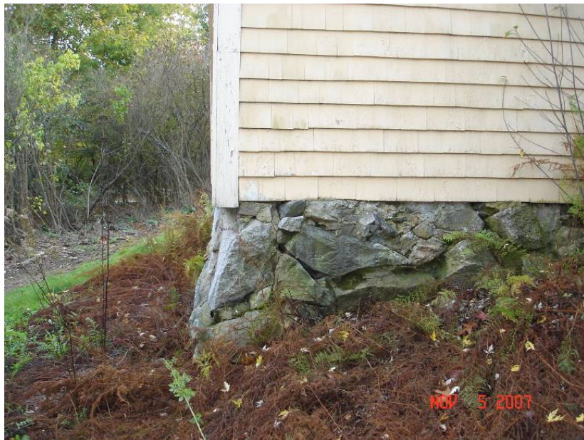
Figure S-14. Foundation at northeast corner.
