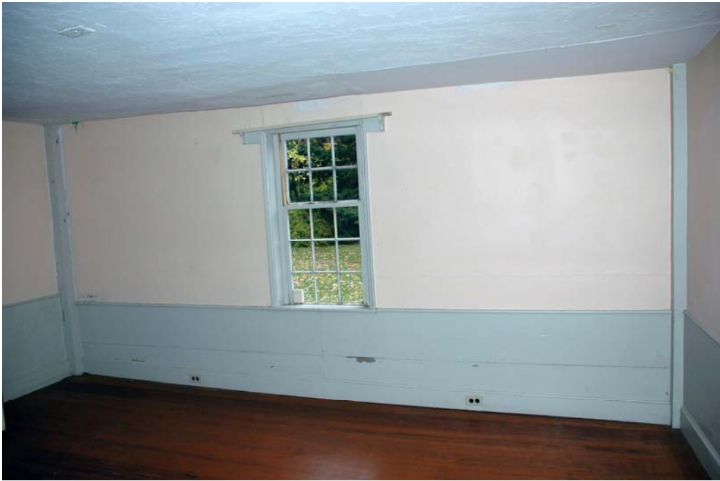
Figure 108-4. North elevation of Room 108 with Window 112.
