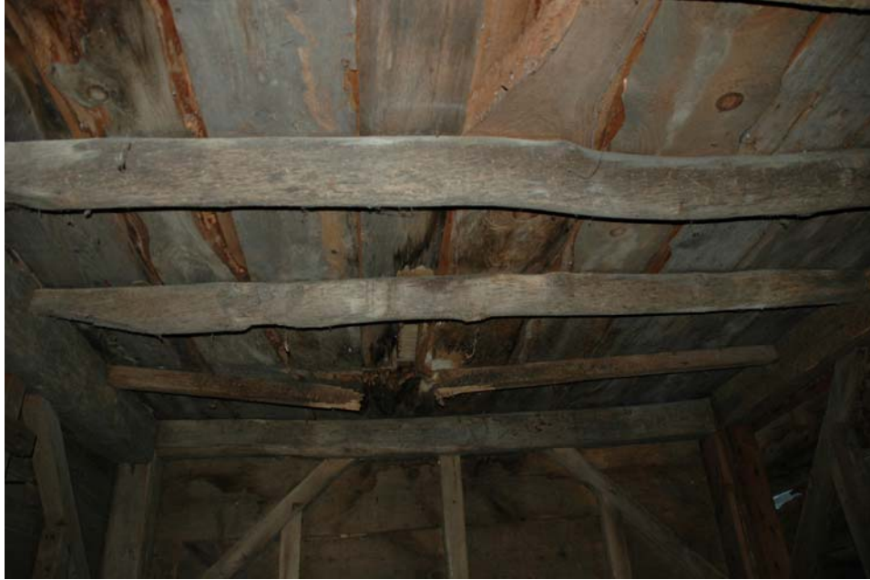
Figure 110-2. Ceiling view of Room 110, including damaged joist in background.
