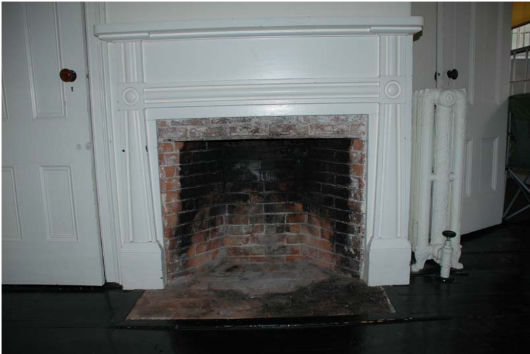
Figure 208-5. Room 208, detail of fireplace.
