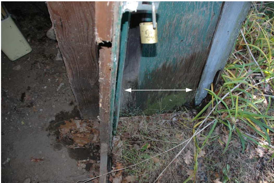
Figure B101-6. Room B-101, jamb at Door B-1/101 where the south wall has projected out due to structural deterioration. The arrows show the extent of movement.
