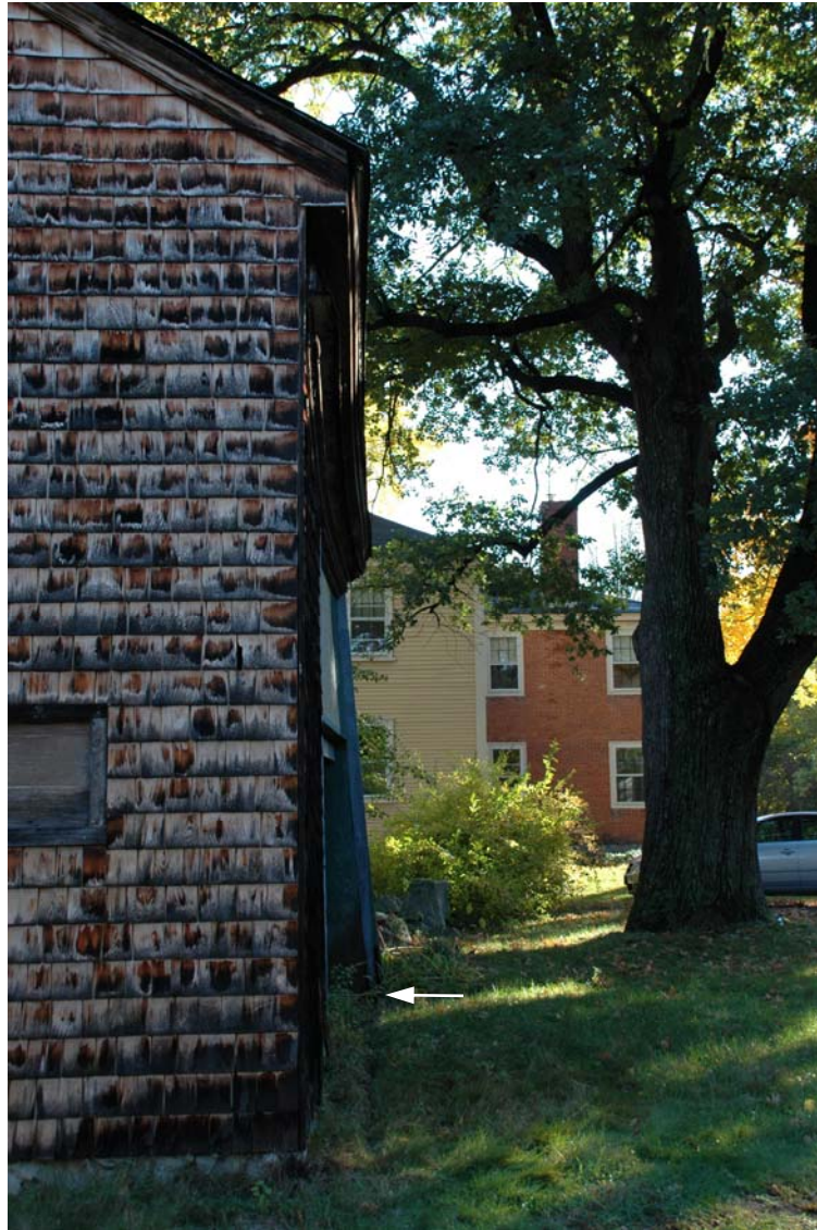
Figure SE-3. View looking east, showing the extent of movement of the south elevation due to structural deterioration.
