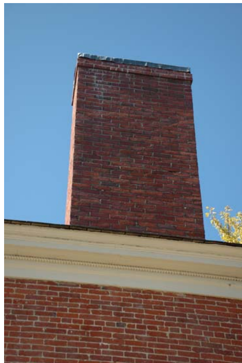
Figure EE-8. East main block chimney.
