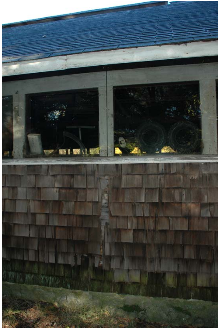
Figure EE-6. Windows #B-106 at the east elevation of the north block. The deteriorated condition of the shingles is typical along the east elevation.
