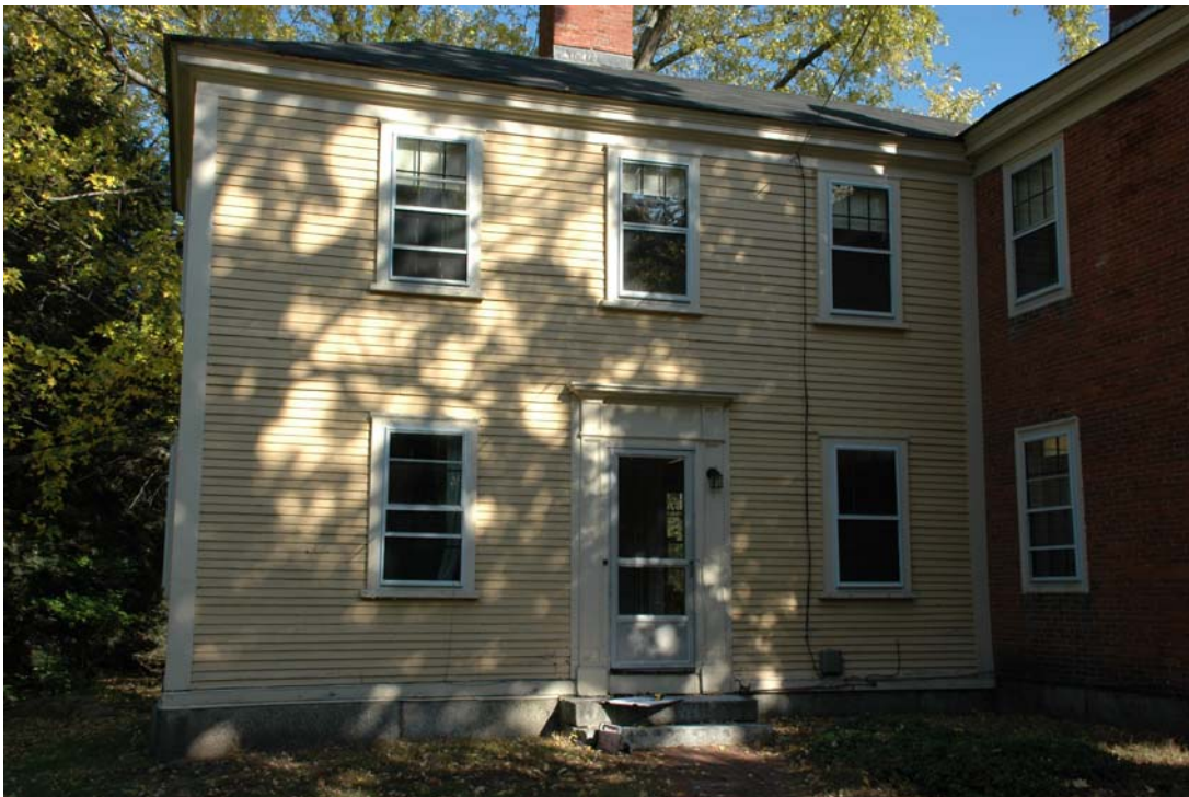
Figure SE-3. South Elevation of northwest wing.
