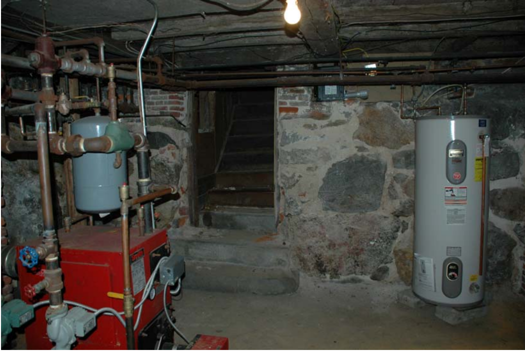
Figure 001-1. North wall of Room 001 with opening in foundation wall for former staircase, now cut off at the first floor level.
