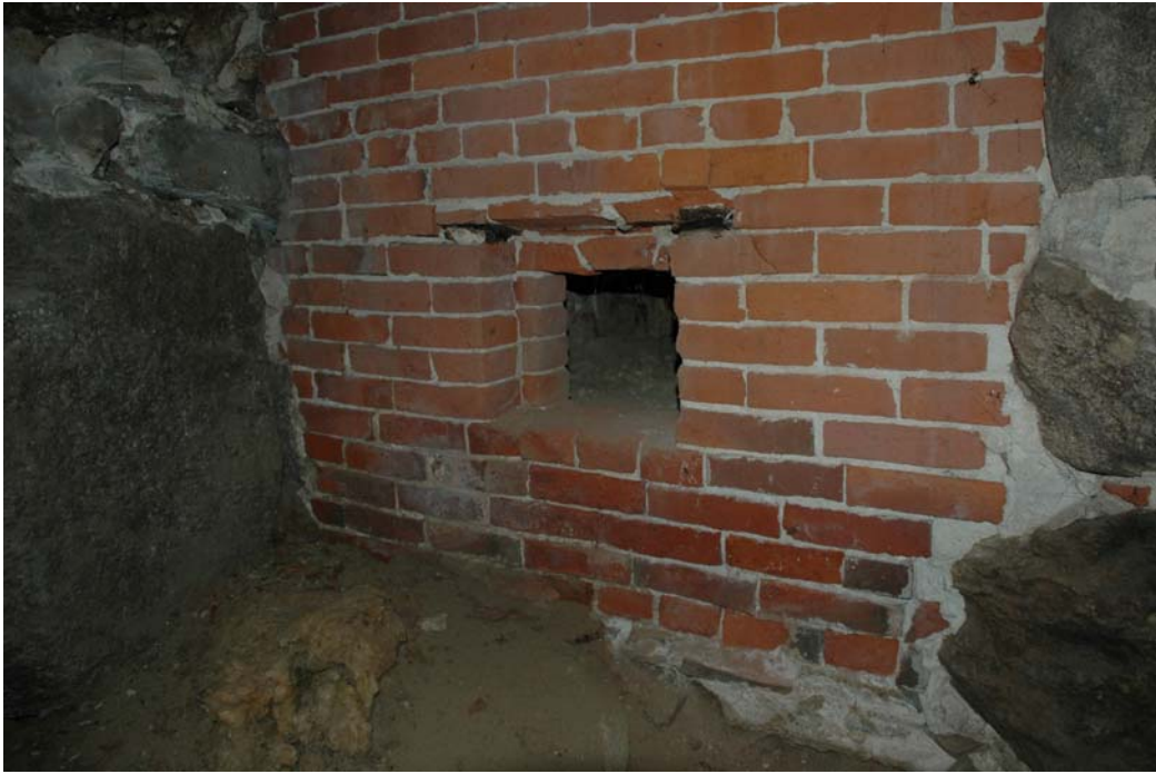
Figure 003-3. Room 003, northern section of the east wall showing the brick foundation wall of the earlier first floor bake oven, now removed.
