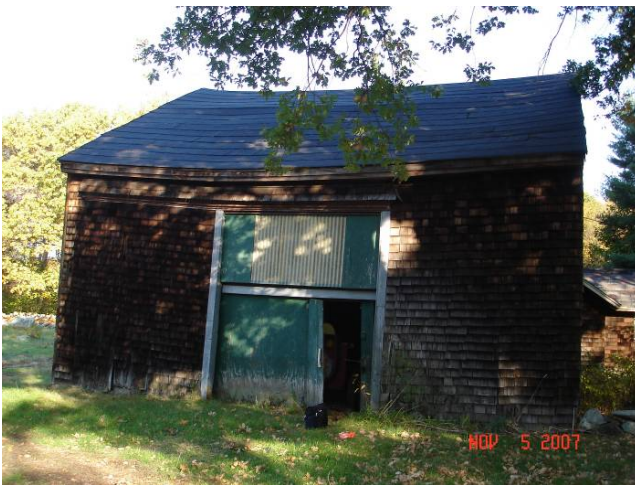
Figures BS-6 & 7. Roof line and soffit line sag – the structure is out of plumb.
