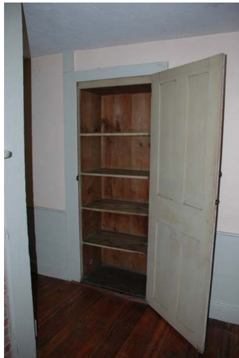
Figure 108-7. Room 108, Door 3/108 closet. The closet interior walls and shelves appear to have been added, indicating that this door may have previously been used as a passage door.
