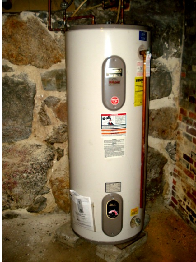
Figure P-2. Domestic Hot Water Heater
