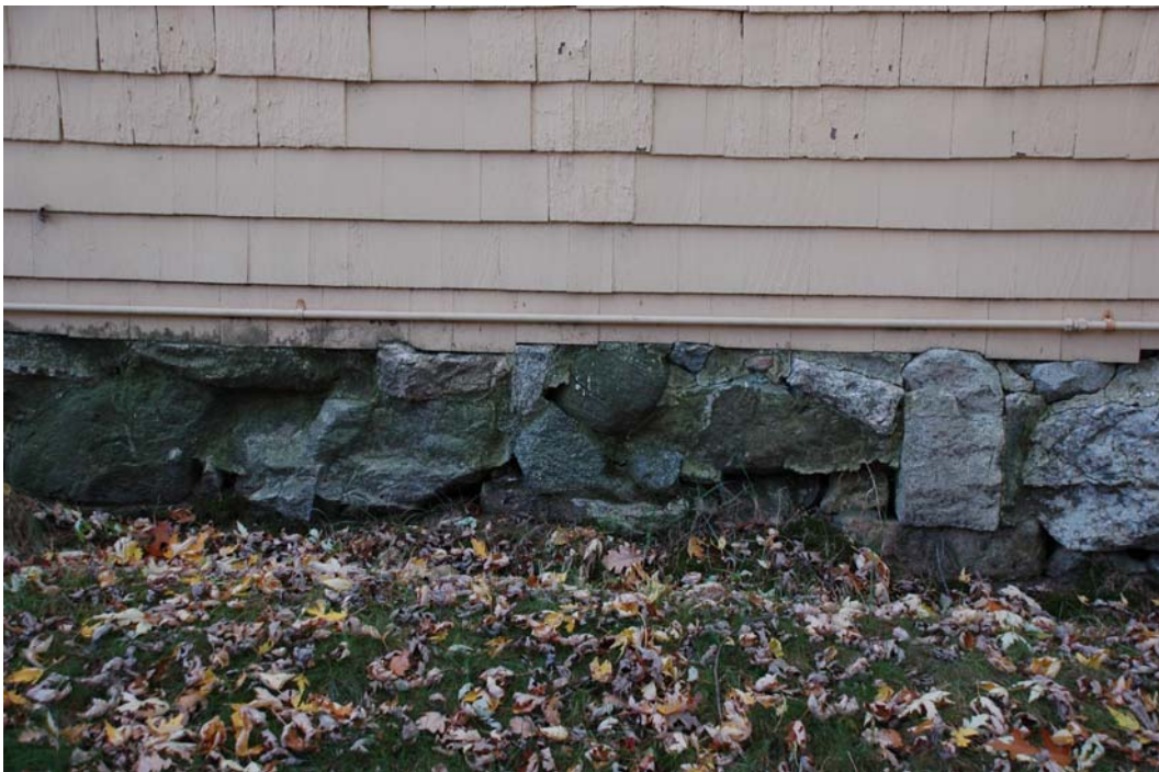
Figure NE-5. Random rubble stone foundation wall and painted shingle siding at north elevation.
