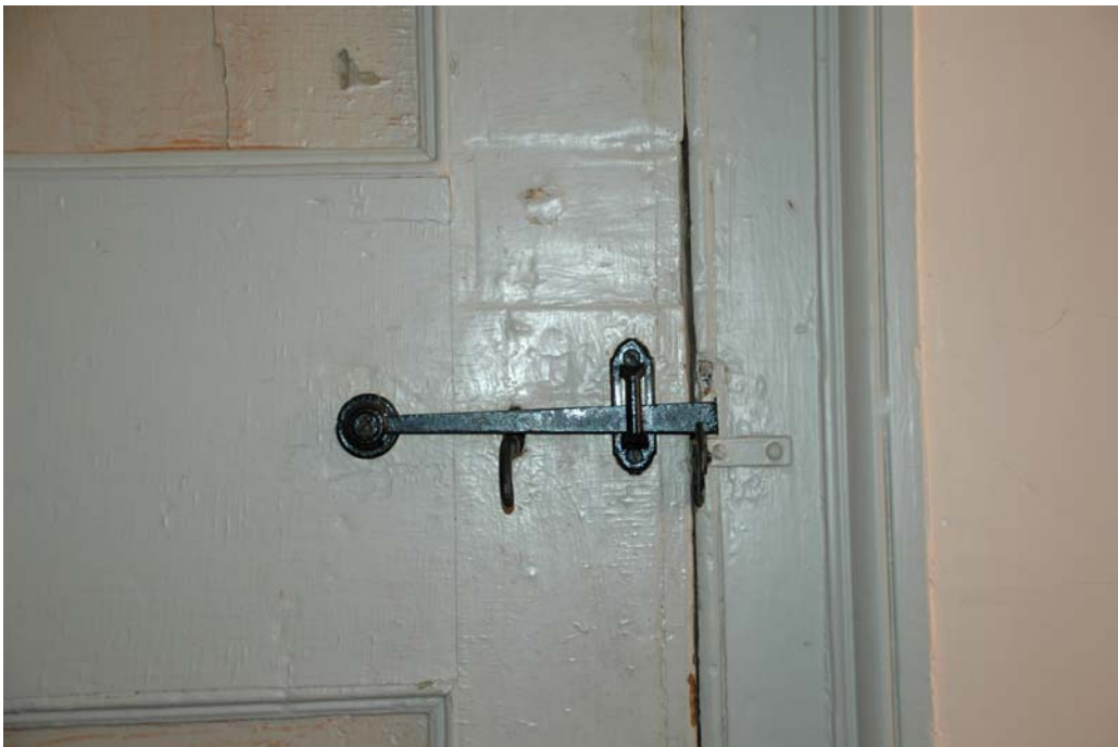
Figure 1.3A-39. Reproduction thumb latch, Room 108. There is a scar on the door from a former rim box lock.
