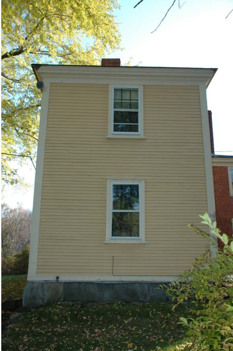
Figure WE-2. West Elevation of northwest wing with windows #117 & 217, both Type w-A.
