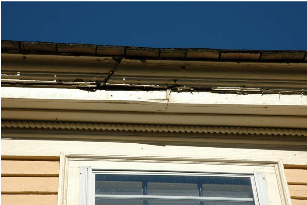
Figure SE-20. Deteriorated roof cornice at the center of main block, above window # 208.
