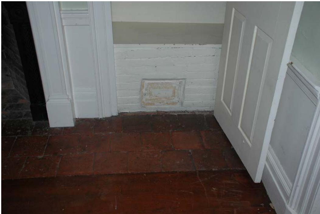
Figure 106-6. Room 106, detail of continuous hearth at closet and brick base of original bake oven in the bottom section of the closet. The small section of chair rail and baseboard between the fireplace and the closet is different than the rest of the room.
