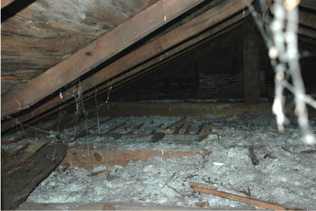
Figure S-2. King post framing in background.
