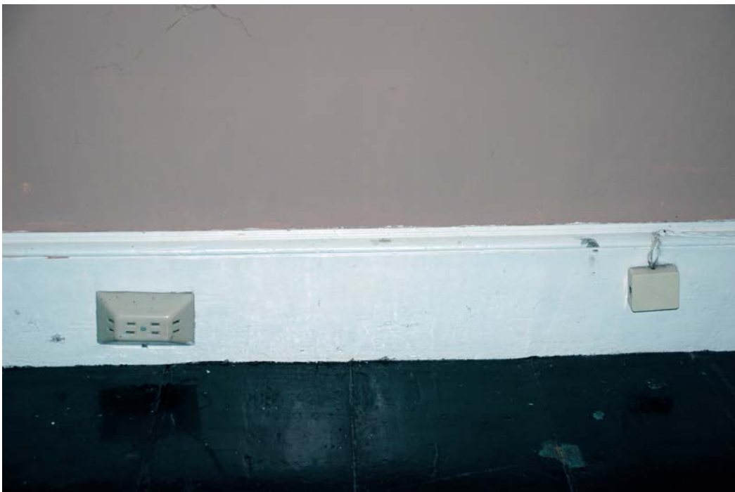
Figure 202-7. Room 202, detail of baseboard with surface mounted outlets and wires.
