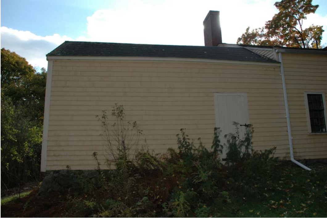
Figure NE-2. North Elevation of northeast wing.
