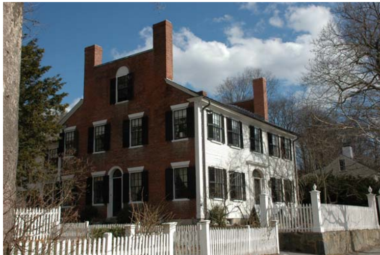
Figure 1.3A-16. House in Concord, MA with brick end walls.
