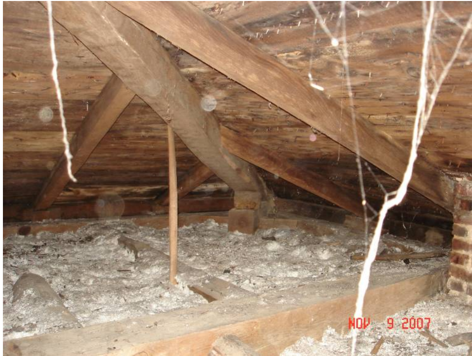
Figure S-11. Hip rafter connection to hammer beam support.
