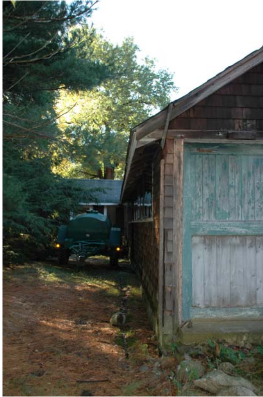
Figure NE-2. East side of north elevation, north block, with Door B-2/102 in the foreground. The north elevation of the east wing is in the background.
