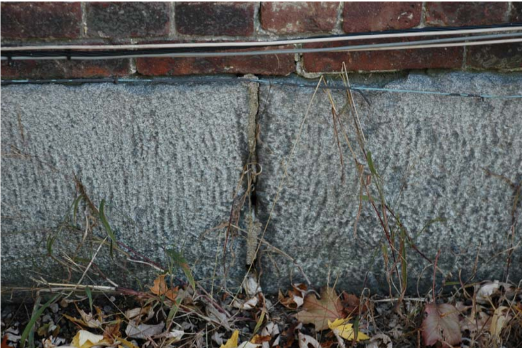
Figure WE-7. Detail of foundation wall at west elevation of main block, showing condition of shrunken and missing mortar.
