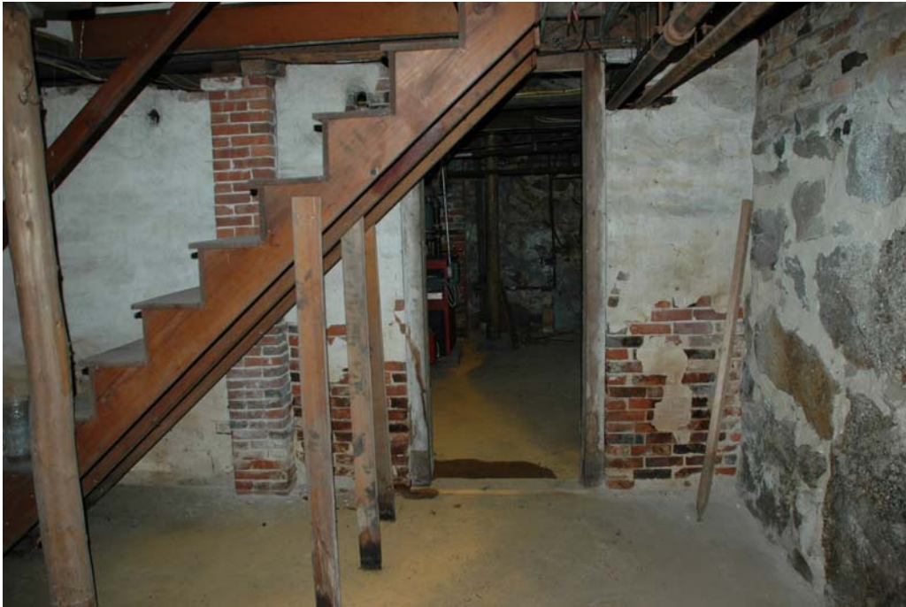
Figure 002-3. West wall of Room 002, looking toward basement stair and to Room 001.
