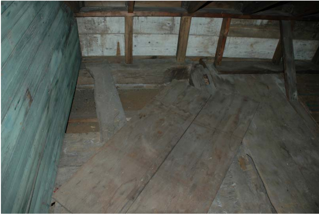
Figure 210-3. Room 210, looking north above the 18 th century block. There is a board and batten door over an opening in the floor, shown moved in this image. It is possible that this opening was for a former staircase, as the opening aligns with the scars on the walls and ceilings below in Room 108.
