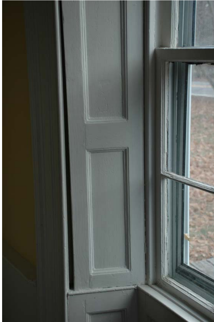
Figure 1.3A-30. Paneled interior window shutters in Room 102.
