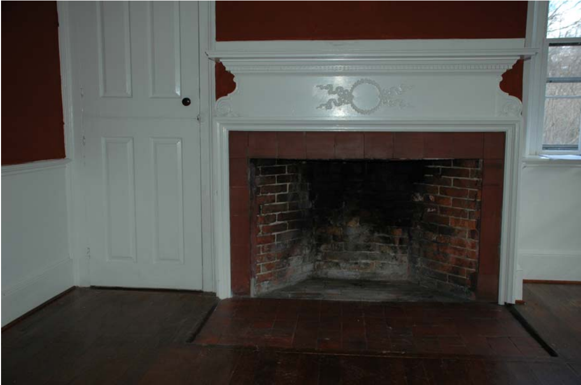
Figure 1.3A-22. Fireplace in Room 103.
