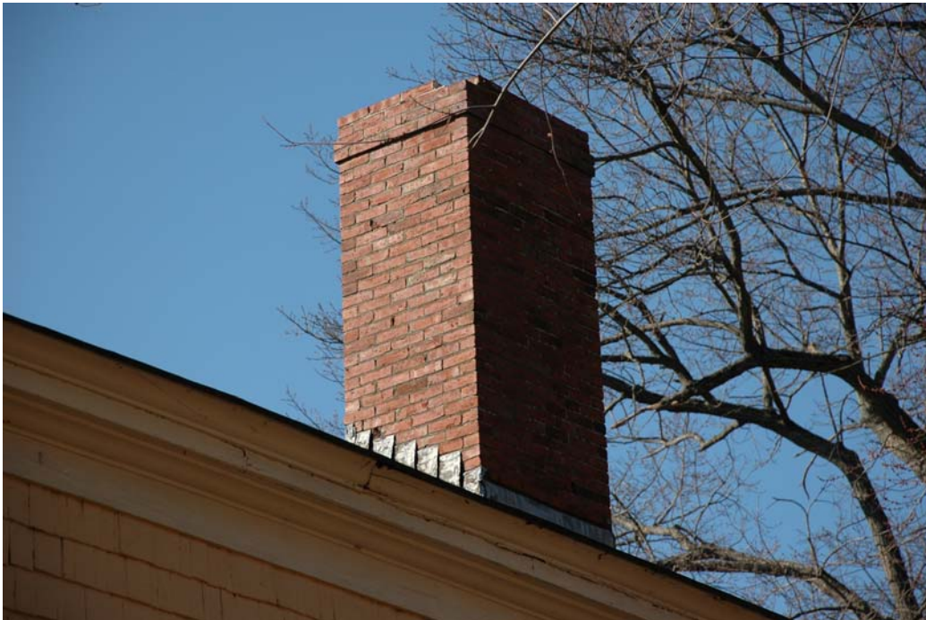
Figure NE-9. Brick chimney on the north elevation at the northwest wing.
