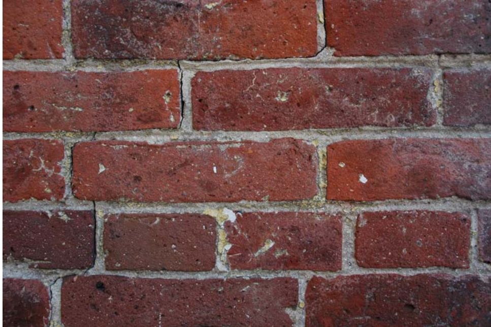
Figure 1.3A-17. Detail of one of the John Nelson House brick end walls, with remains of the painted surface in the mortar and brick crevices.
