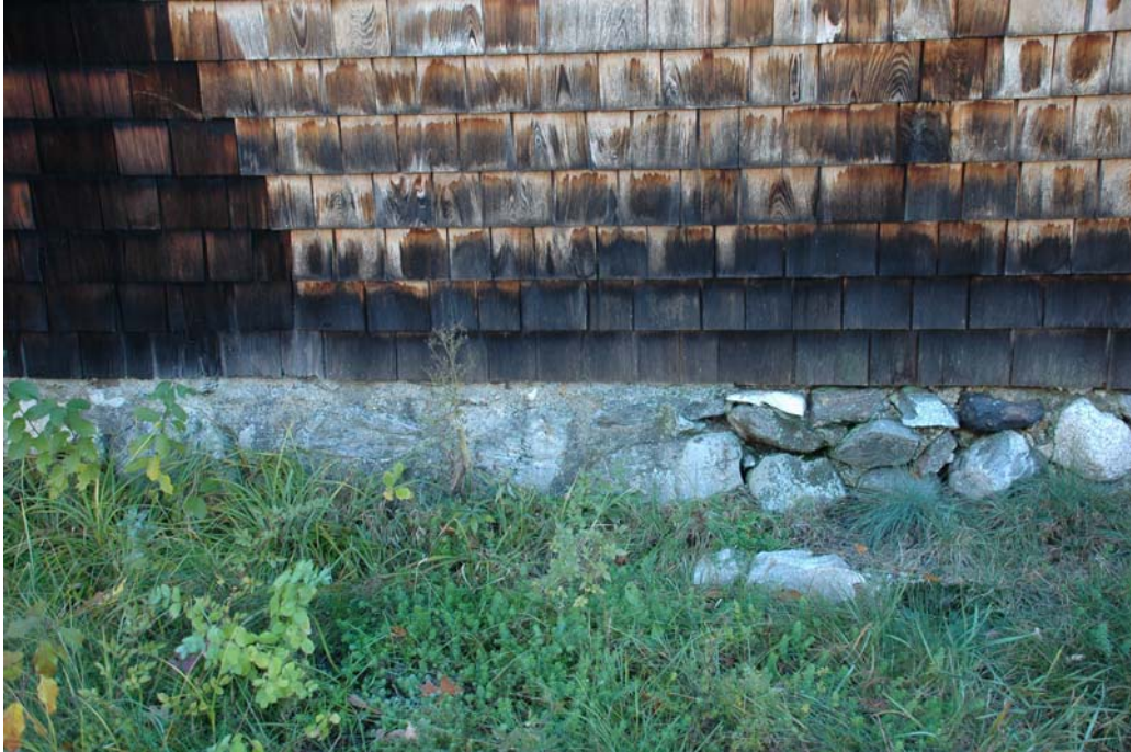
Figure WE-4. Foundation wall at west elevation, where the now-demolished west wing extended from the west wing on the right half of the foundation wall.
