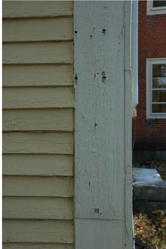
Figure 1.3A-8. Horizontal clapboard siding and corner board.
