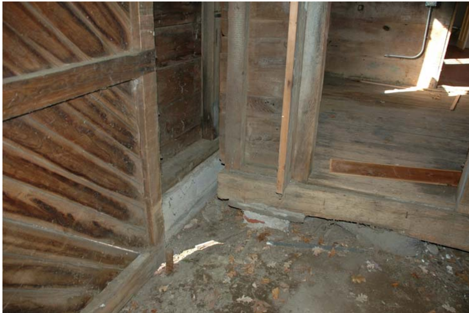
Figure 110-3. South west corner of Room 110. Carriage house Door 1/110 is on the left, and Door 2/110 leading to Room 109 is on the right. The floor is earth.
