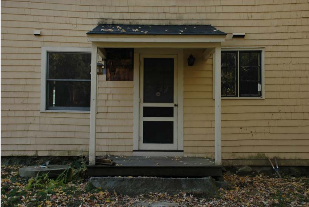
Figure NE-11. Door 1/107, Windows 113, 114, and rear porch.
