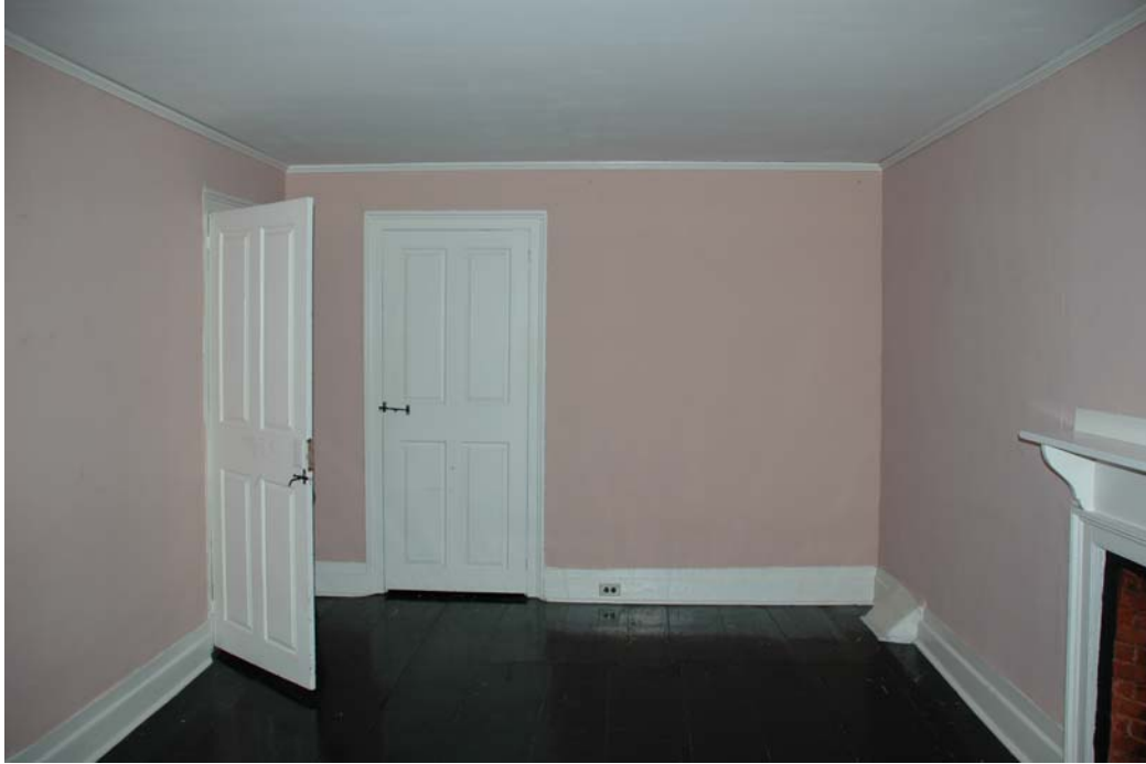
Figure 204-3. North and west elevations of Room 204. Door 1/204 on the left leads to Room 201. Door 2/204 leads to the closet, Room 204A.
