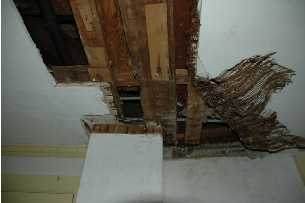
Figure 107-4. Room 107, ceiling view with plaster removed to expose failed structural members.
