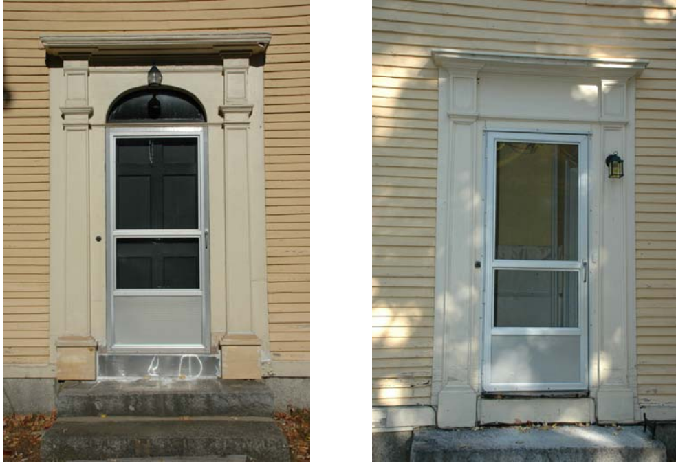
Figure 1.3A-13. Door 1/101 on the left and Door 1/105 on the right.
