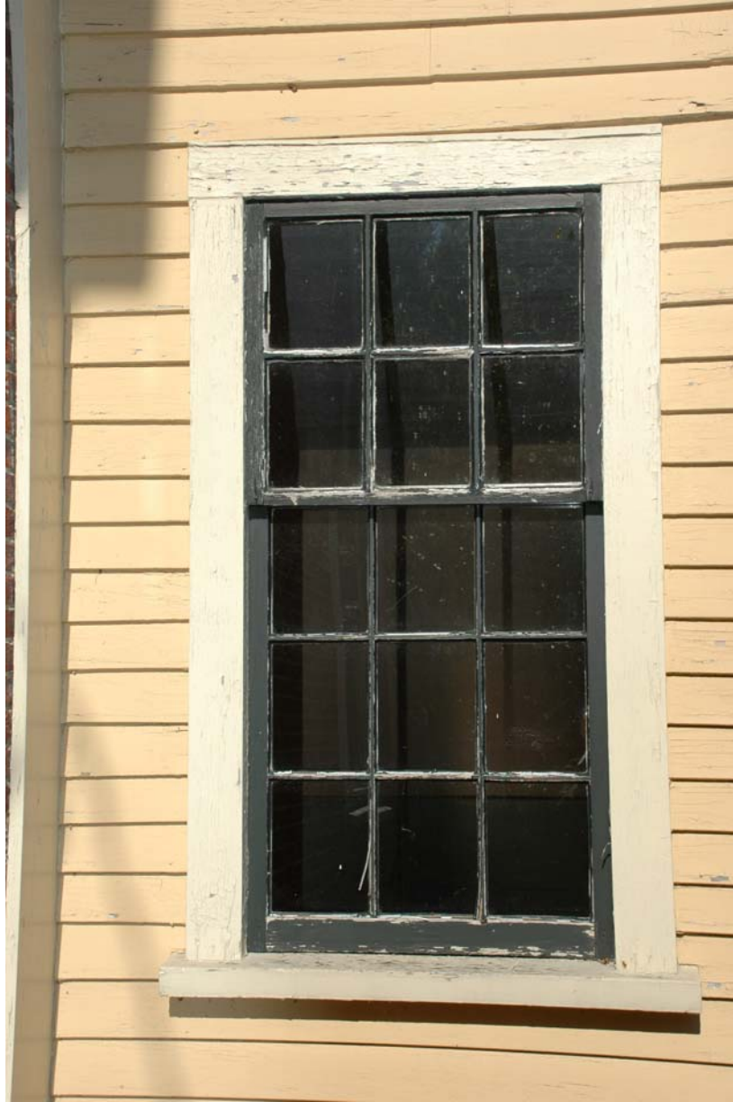
Figure SE-18. Window Type w-C: 6-over-9 single hung with flat board trim. On the south elevation Type w-C is found at Window #110.
