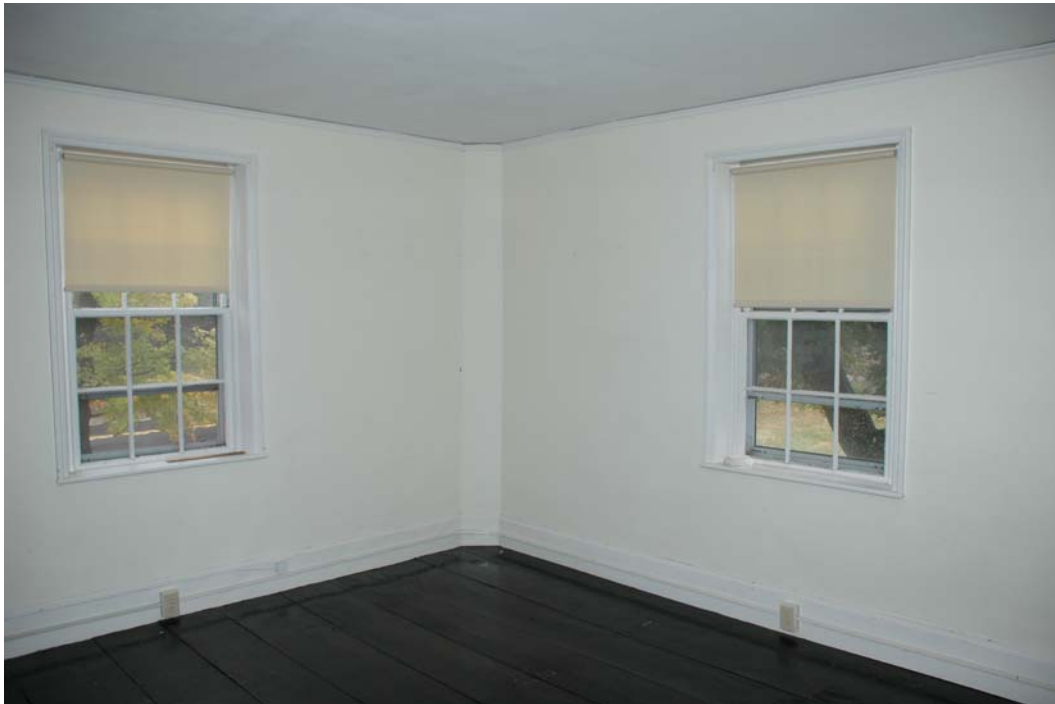
Figure 208-3. Room 208, looking southwest with an angled corner finish, most likely enclosing a corner post.
