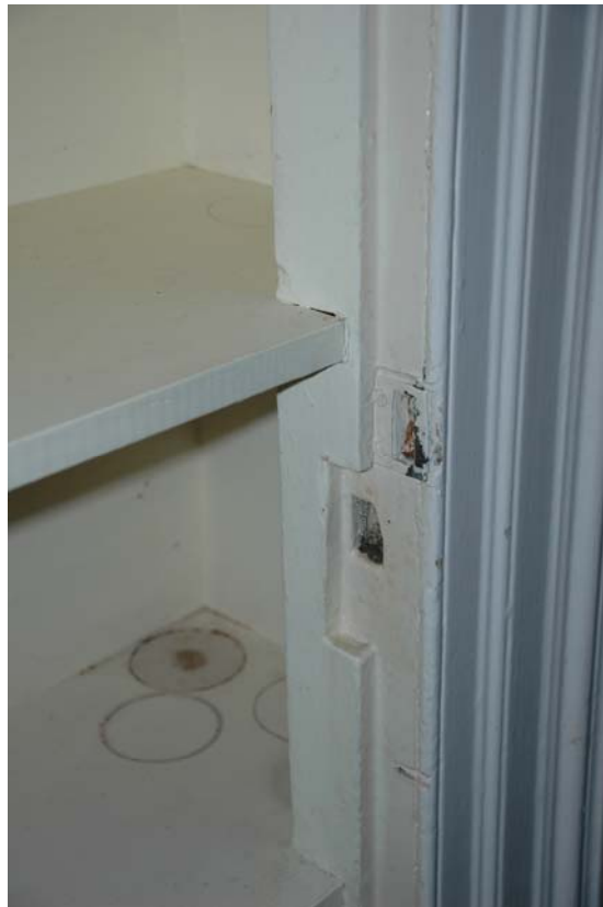
Figure 106-8. Room 106, detail of right jamb at Door 3/106 showing indentation in door stop for the original box rim lock.
