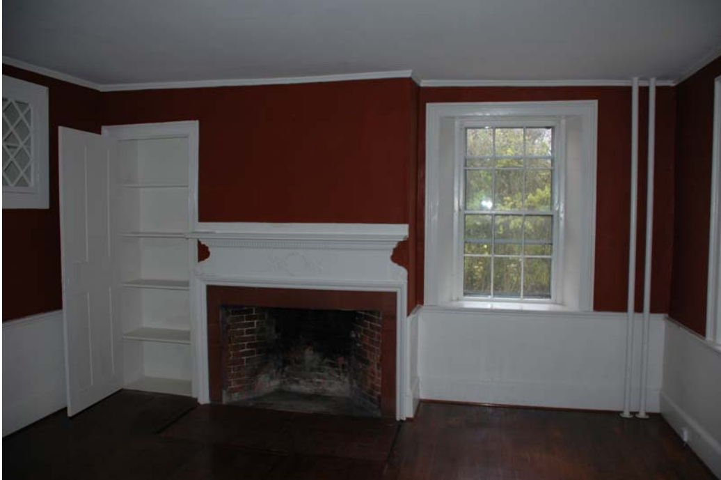
Figure 103-2. North elevation of Room 102 with fireplace and Door 3/103 leading to a wall cabinet.
