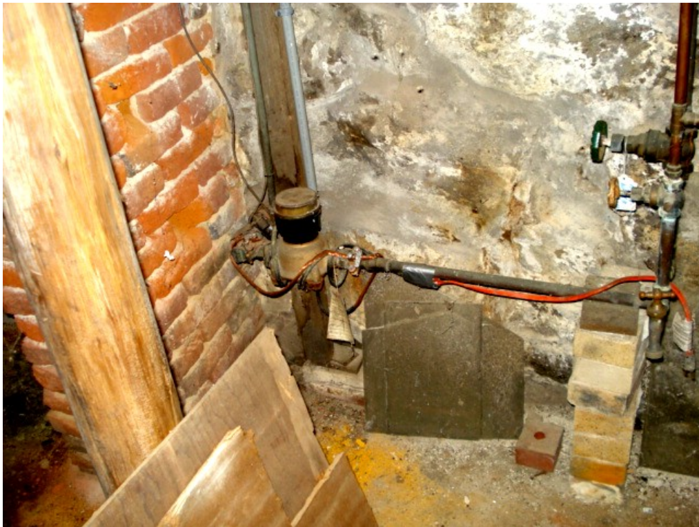
Figure P-1. Domestic water service
