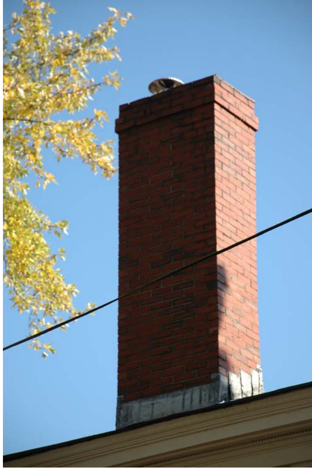
Figure WE-10. Brick chimney at the west elevation of the main block.
