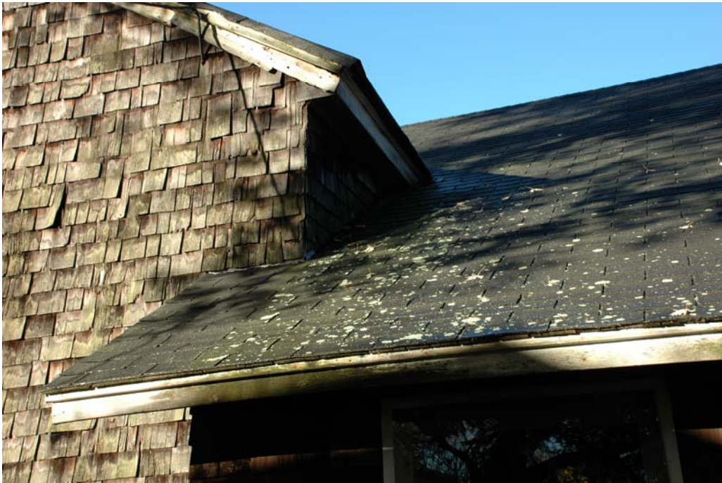
Figure EE-5. Roof condition at east elevation where the north block roof, right, intersects with the main block roof, left.
