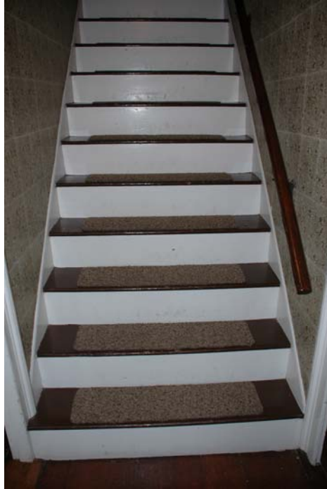
Figure 101-1. Room 101, looking north at stair.
