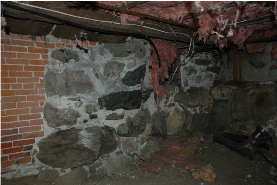
Figure 003-2. Room 003, east wall. This may have been the exterior foundation wall prior to the construction of the northwest wing second phase. The wall appears to have been significantly reworked at some point, with the brick infill at the fireplace and bake oven foundations.
