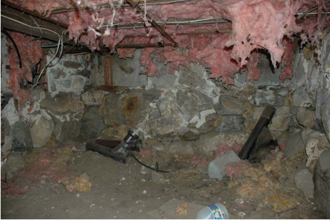
Figure 003-1. Room 003, south wall.
