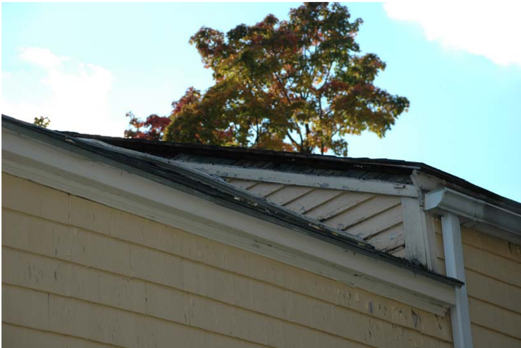
Figure EE-6. East rear addition gable end wall above northeast wing. The raking board is deteriorated and has detached from wall.
