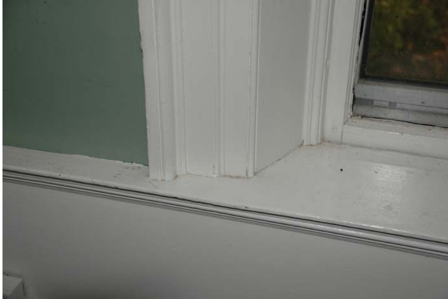
Figure 1.3A-34. Window casing, Room 104. The door casing in this room is similar, as well as in Room 204.
