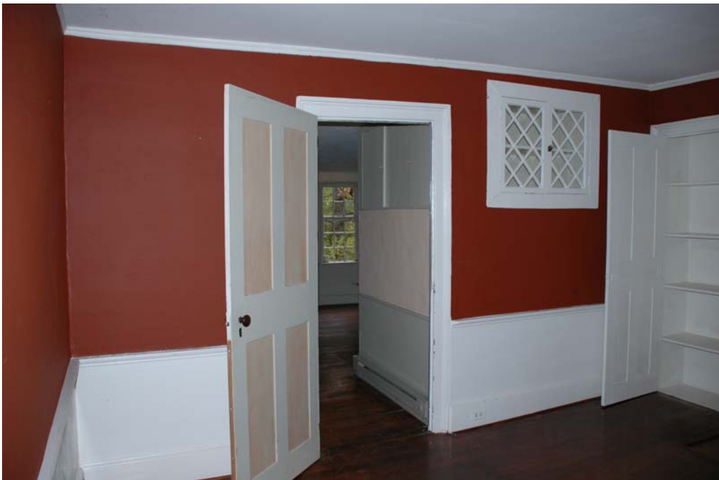
Figure 103-3. North elevation of Room 103 with Door 2/103 leading to Room 108. The wall cabinet with diagonal-patterned glass doors is above the masonry mass of the bake oven and fireplace in Room 108.
