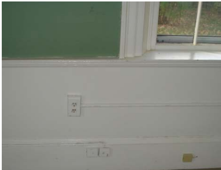
Figure E-6. Typical telephone and CATV wiring.
