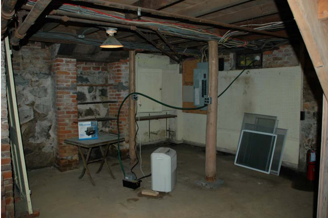
Figure 002-1. East and south walls at Room 002, with the brick fireplace support on the east wall and Window #002 on the south wall.
