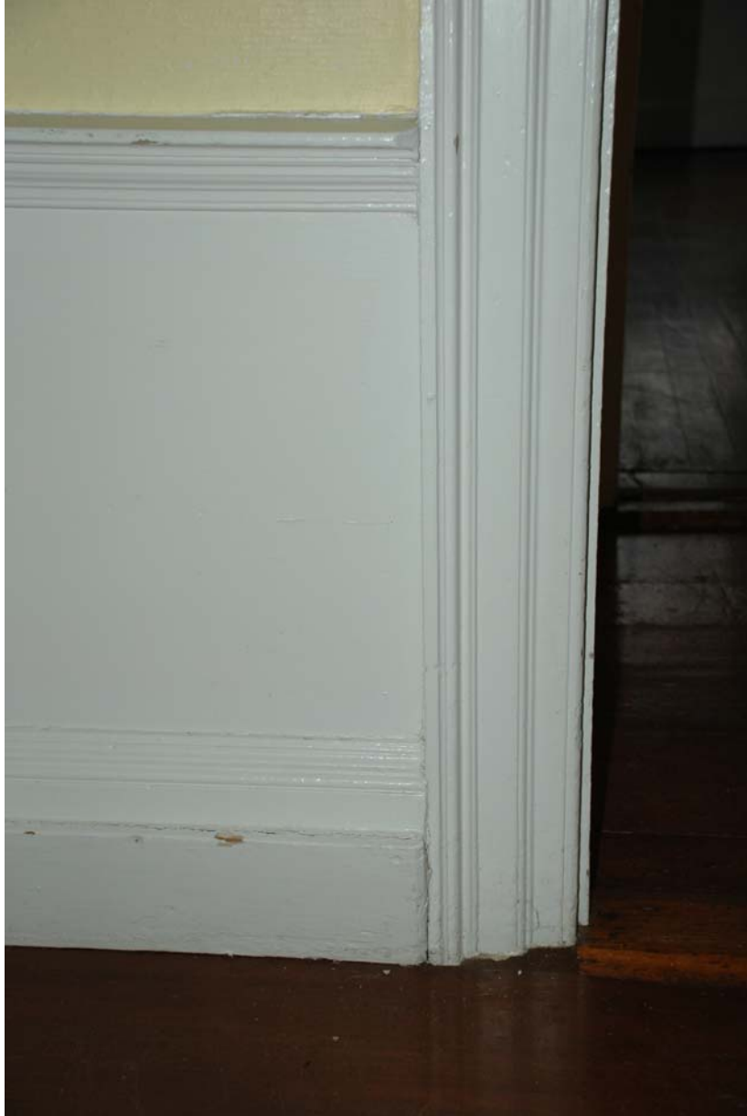
Figure 102-4. Room 102, detail of wood wainscot, chair rail, 2-piece baseboard, and door casing as found at Door 3/102.
