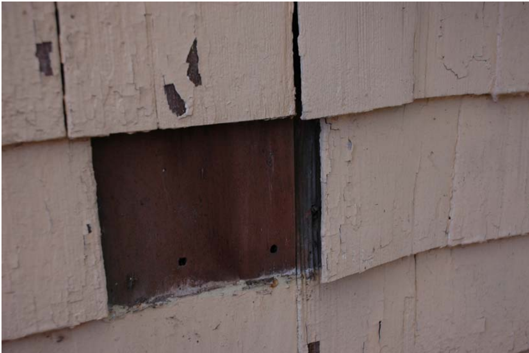
Figure NE-7. Deteriorated and missing areas of shingle siding at the north elevation.
