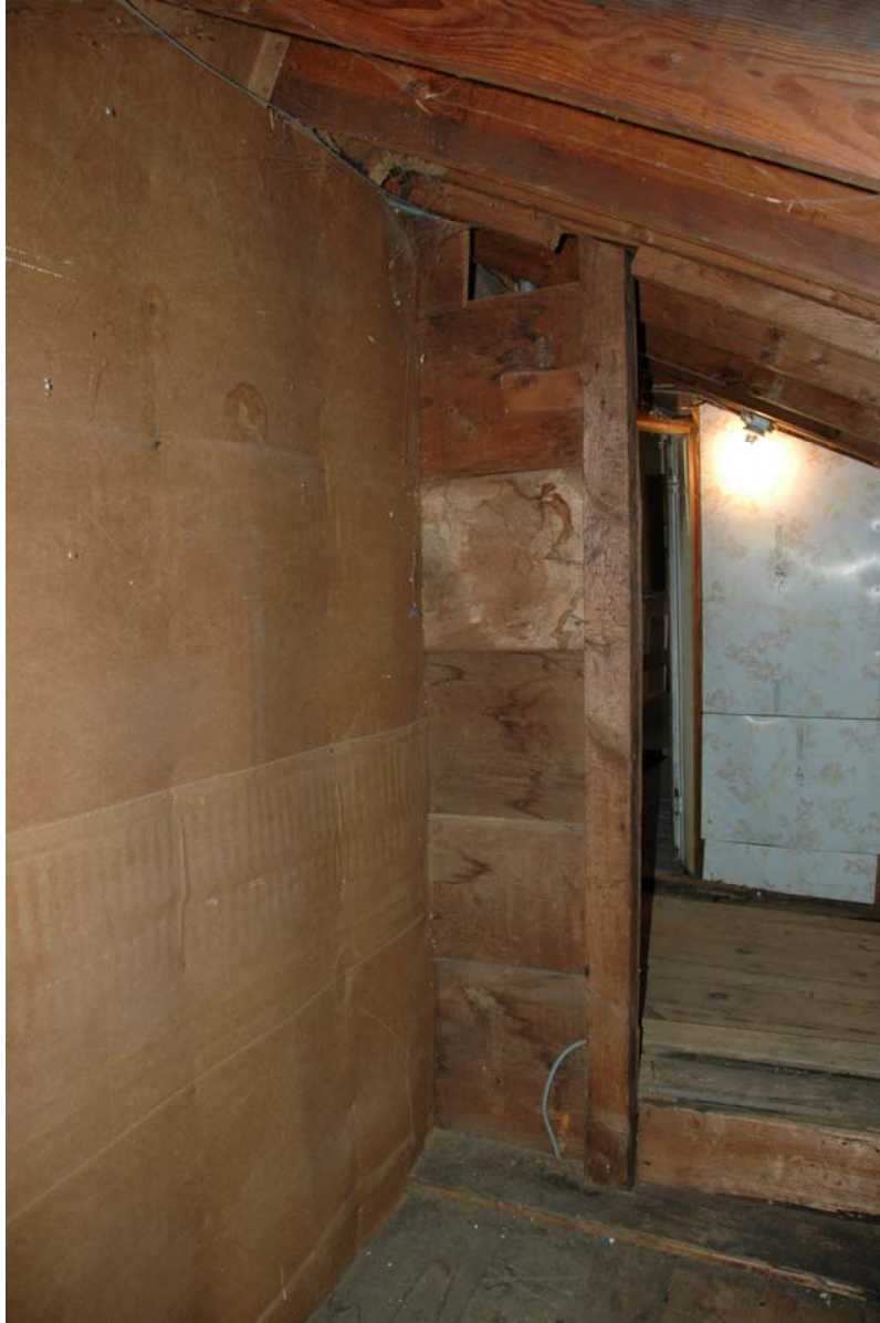
Figure 209-5. Room 209, looking west at the possible 18 th century frame wall, in center. The floor steps up at this point where the 18 th century block meets the northwest wing.
