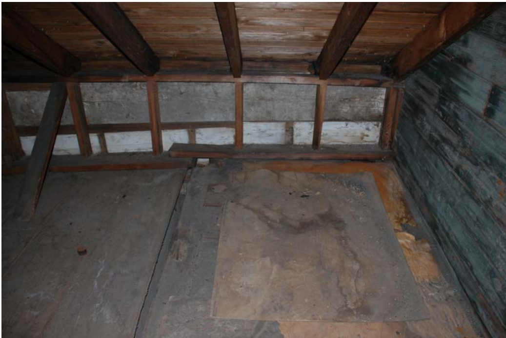
Figure 210-2. Room 210, looking south at southwest corner. The original east wall plate of the 18 th century block, running north-to-south is seen at the middle-left. The attic floor to the left of this is in the northeast wing. The horizontal board partition on the right that divides the attic space above the 18 th century block was added later.
