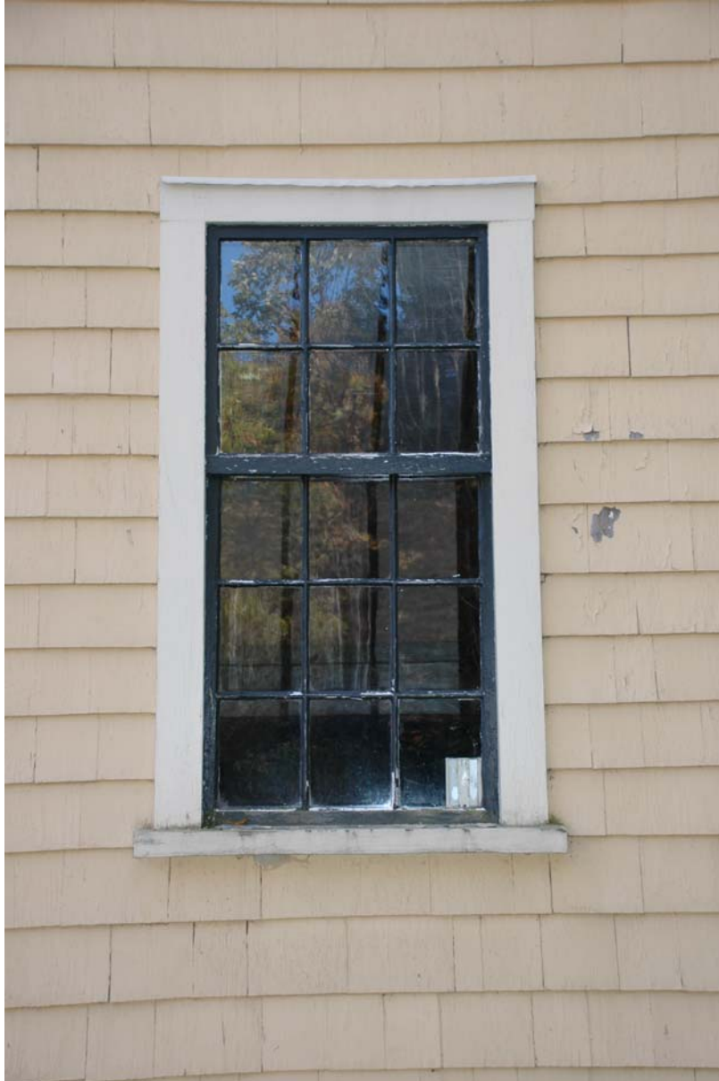
Figure NE-13. Window #112, Type w-C. Wood sash and sill are deteriorated.
