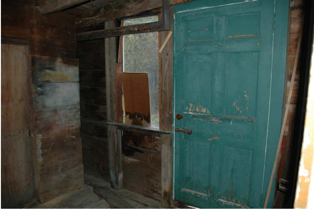
Figure 109-2. Room 109, south elevation with Door 1/109 and Window 111 (sash missing).
