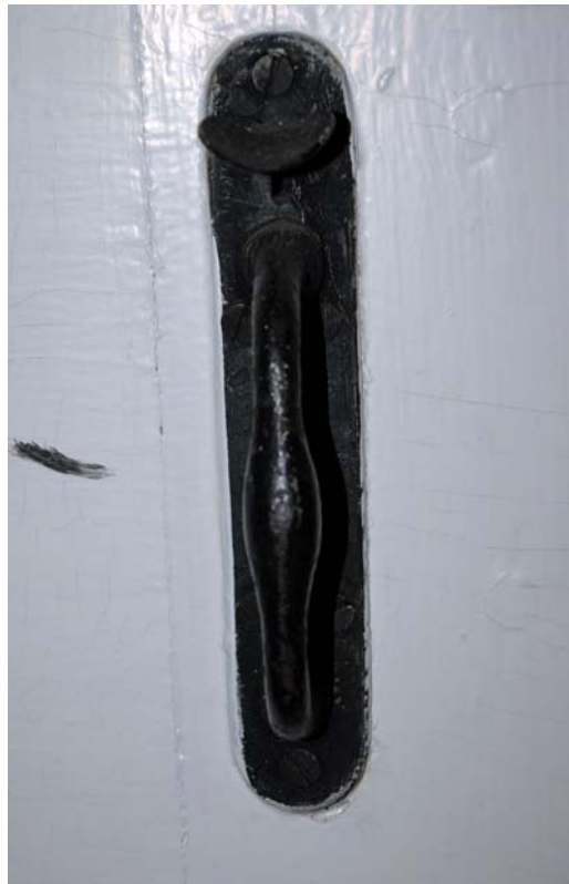
Figures 202-4 & 5. Thumb latch door hardware found at Doors 2/202, 1/203 and 2/204.
