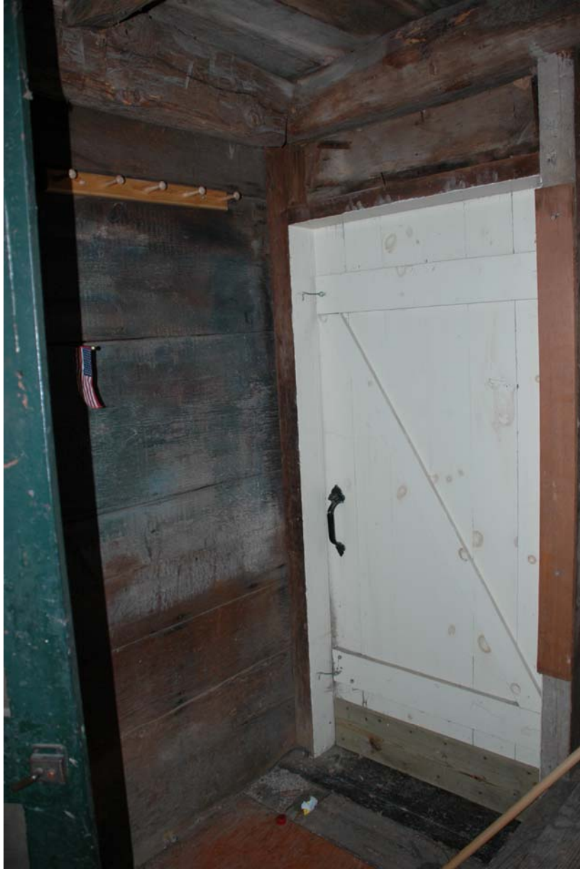
Figure 109-4. West and north elevations of Room 109, with Door 2/109 leading to the exterior.
