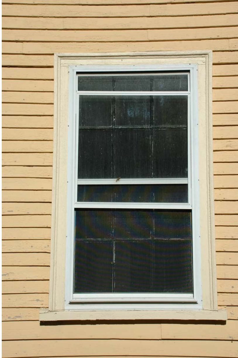
Figure SE-17. Window Type w-B: 6-over-6 double hung window with profile backband trim, found only at the main block. An aluminum triple-track storm window is attached to the wood frame. On the south elevation Type w-B is found at #105, 106, 107, 108, 206, 207, 208, 209, & 210.
