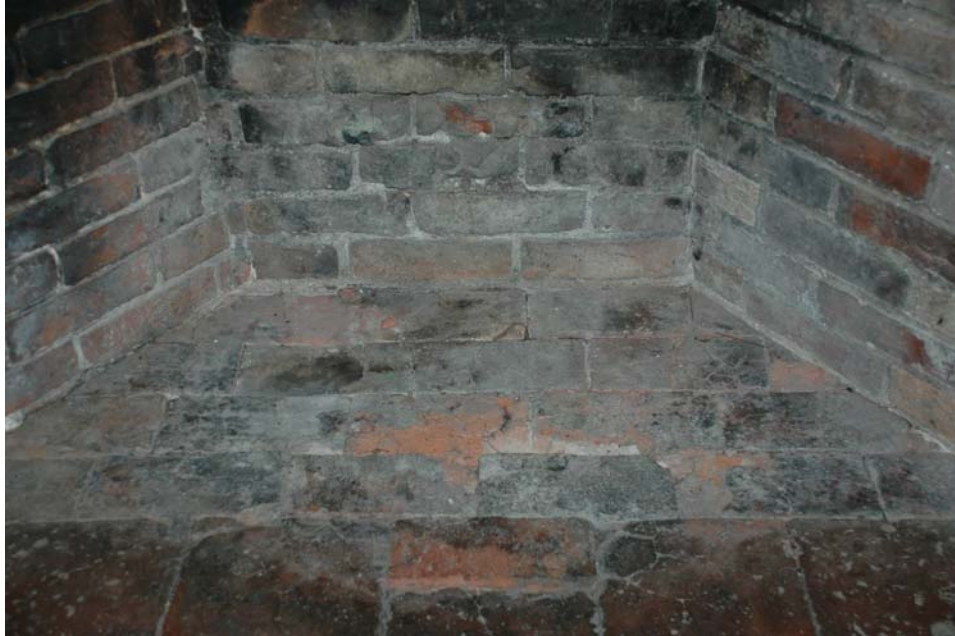
Figure 106-7. Room 106, detail of firebox condition with damaged and stained surface, typical of fireplaces throughout the house.
