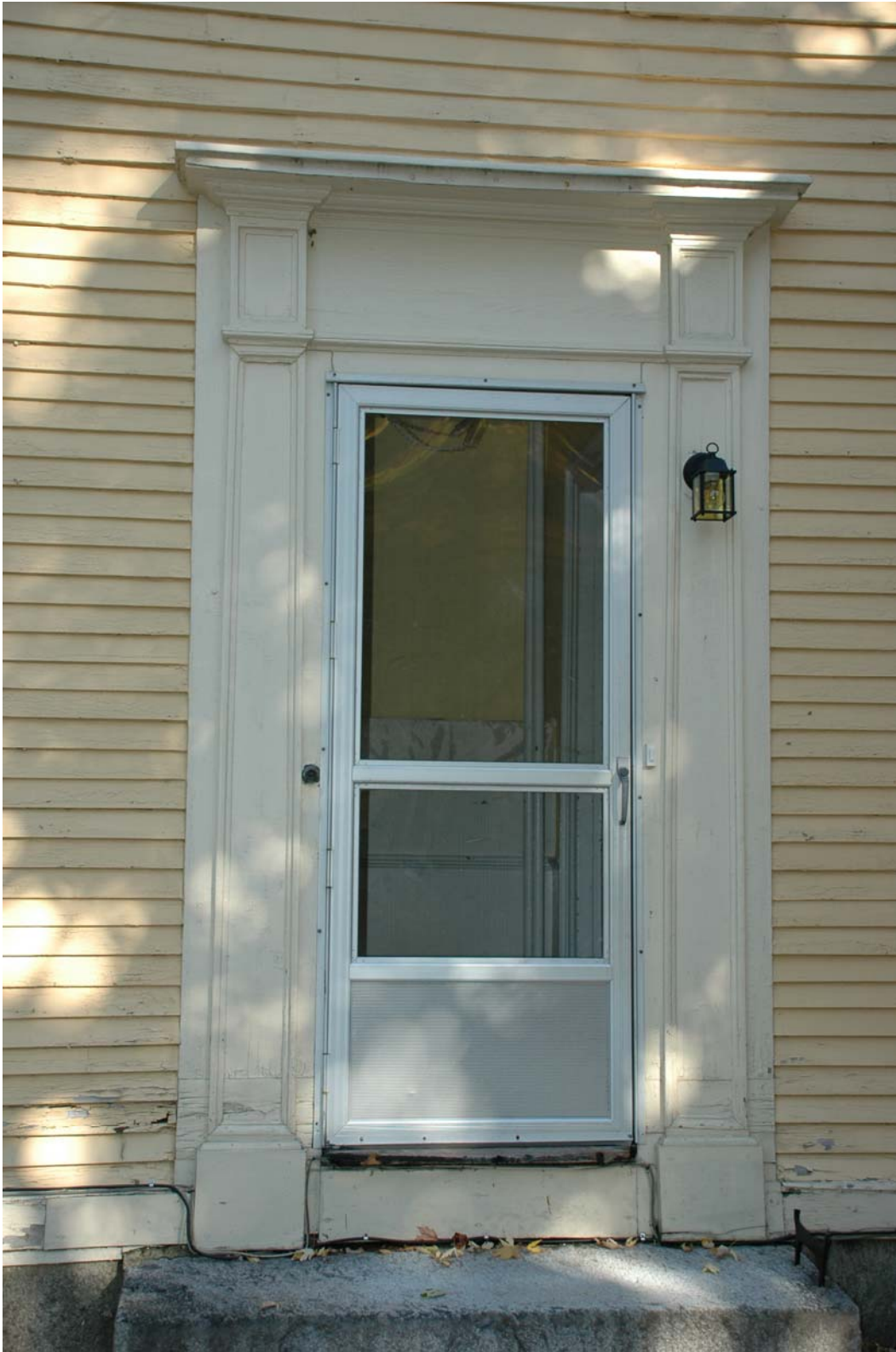
Figure SE-9. Door 1/105 – entrance to the northwest wing.
