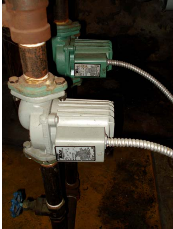
Figure H-4. Hydronic circulator pumps.
