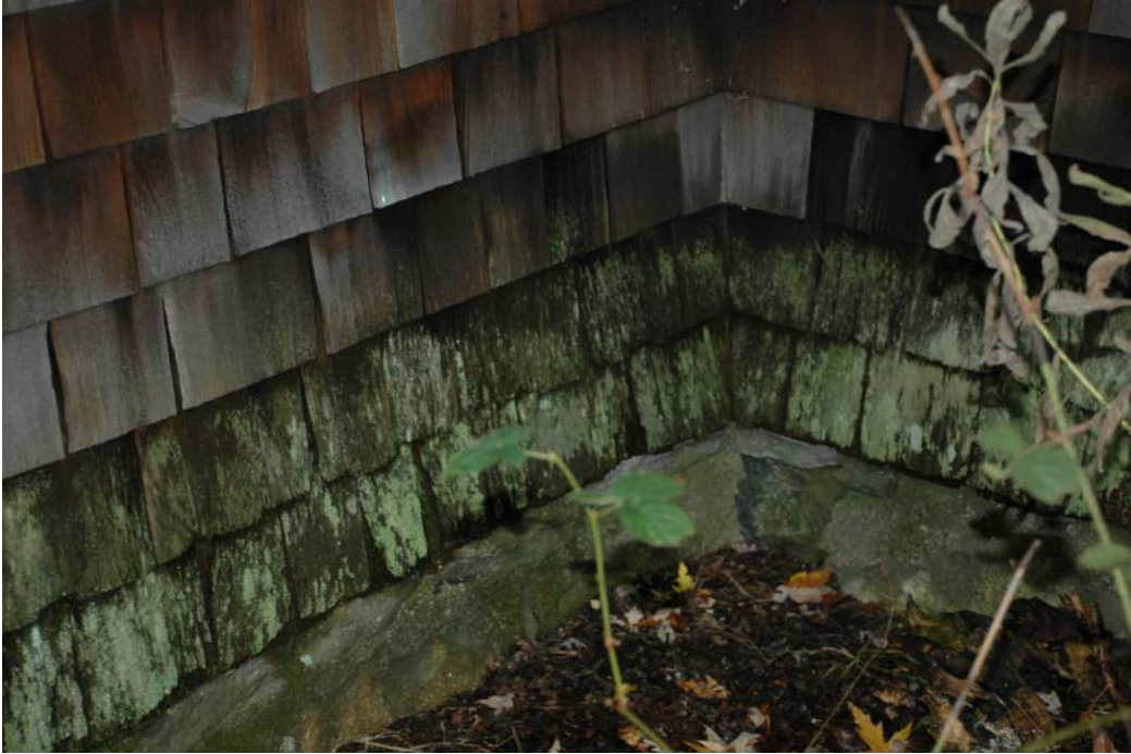
Figure EE-4. Wall condition at east elevation, with mossy and vegetative growth on the wood shingles and masonry foundation.
