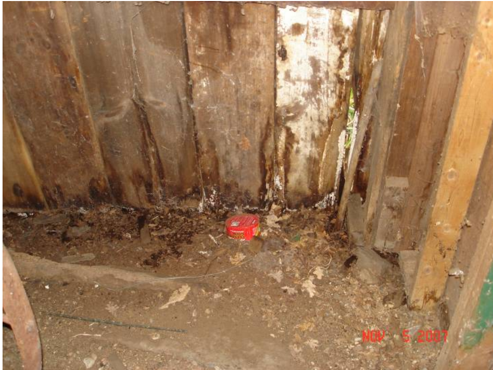
Figure BS-3. Missing sill beams at southeast corner.
