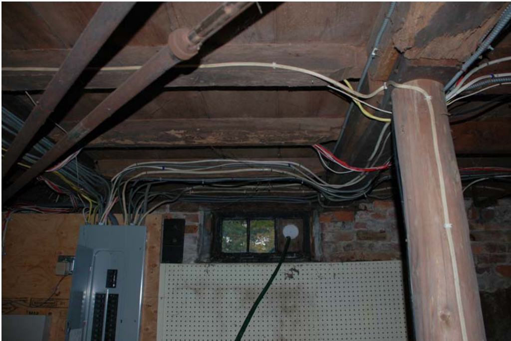
Figure 002-4. South wall of Room 002, with Window #002. The beam on the right is severely deteriorated.
