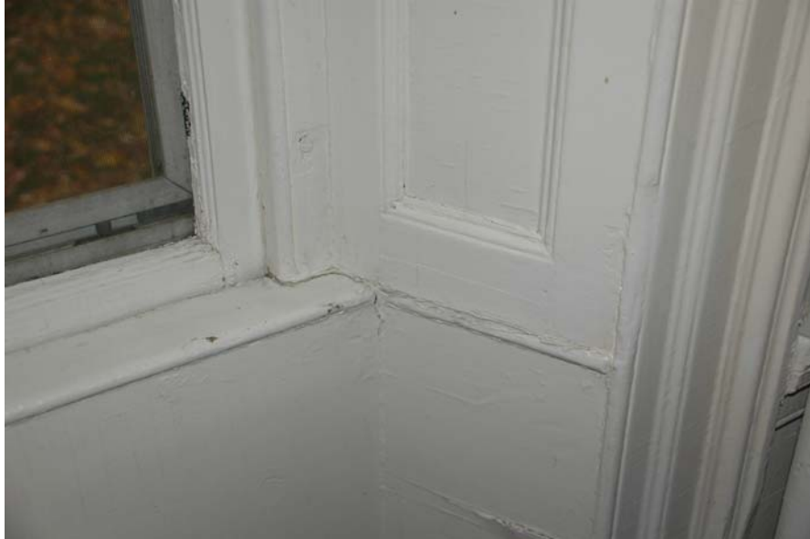
Figure 1.3A-32. Window casing detail with paneled splayed jambs, Room 106.
