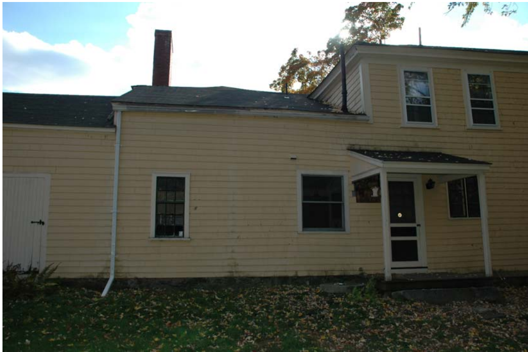
Figure NE-3. North Elevation of original 18 th -century block. This section is the only location that has a gutter and downspout.
