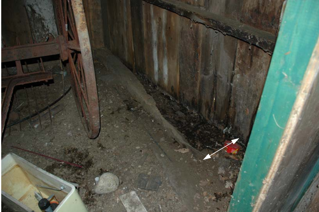
Figure B101-5. Room B-101, interior view of south wall that has projected out due to structural deterioration. The rotted sill plate at the left arrow is the original wall line.
