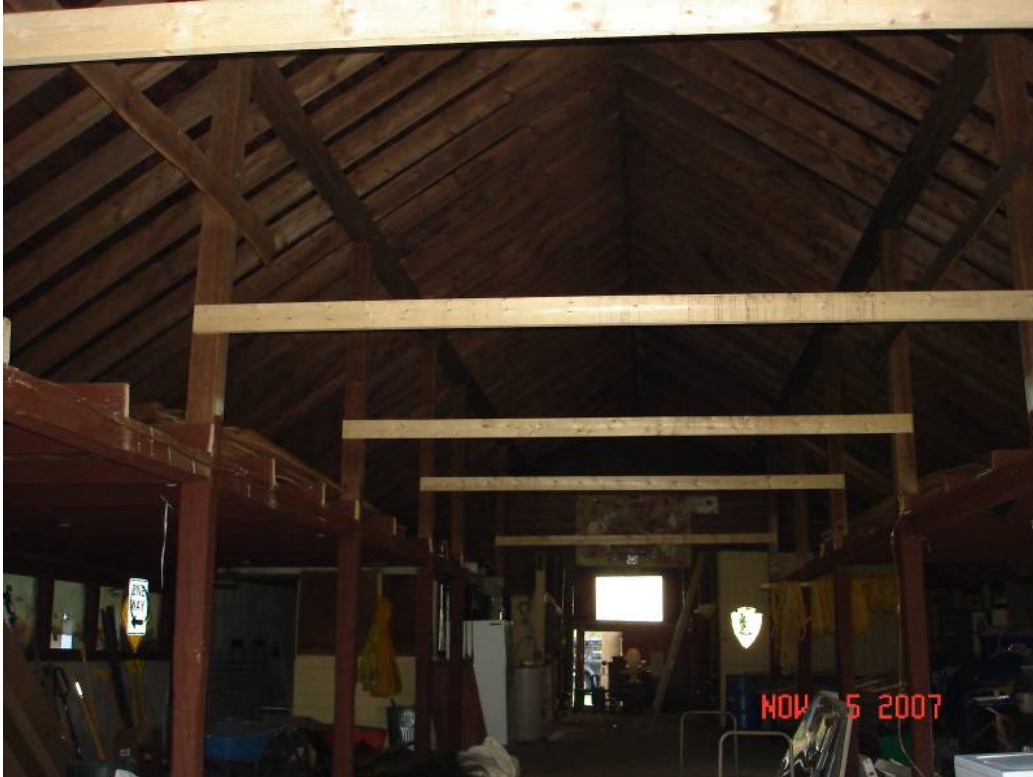
Figure BS-15. North block framing.
