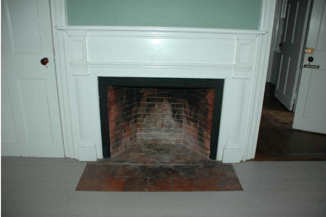
Figure 104-4. Room 104, detail of fireplace.
