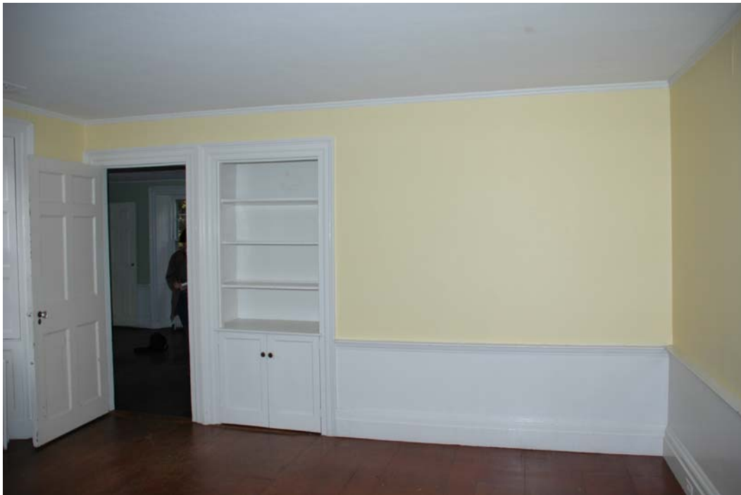
Figure 102-3. North elevation of Room 102. Door 1/102 is on the left and Door 2/102 is on the right. The doors share an integral casing and threshold. Door 2/102 may have originally opened to a stair that led to the second floor.
