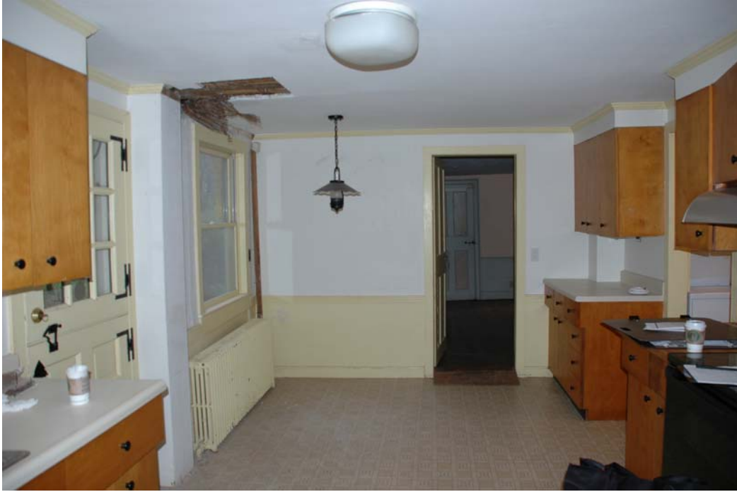
Figure 107-2. Room 107, looking east with Door 1/108 that leads to Room 108. A concealed post is on the north wall, left, to the right of exterior Door 1/107.
