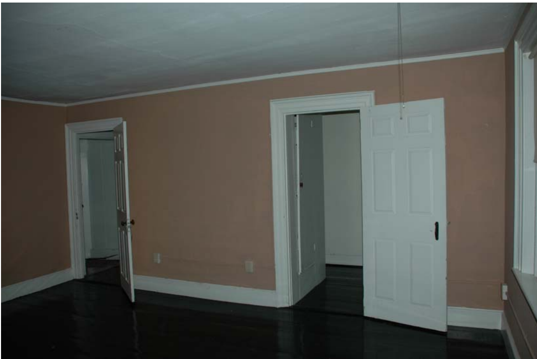
Figure 202-3. East elevation of Room 202 with Door 1/202 on the left that leads to Room 201 and Door 2/202 on the right that leads to Room 203. Both doors are identical in size and panel configuration, although the hardware is different.
