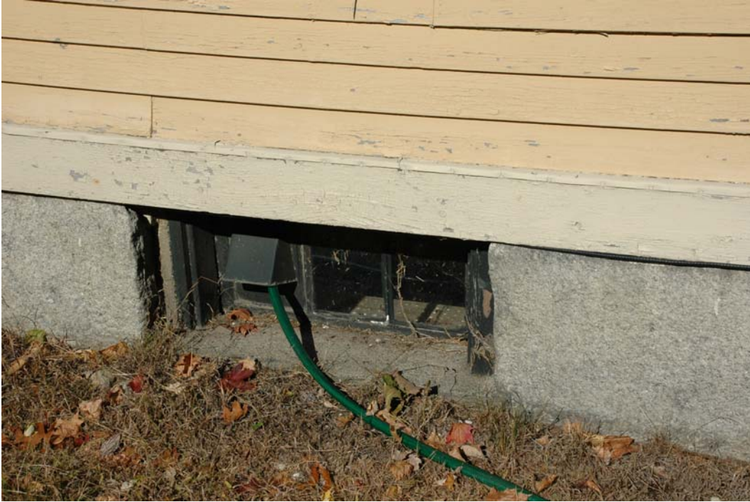
Figure SE-19. Window Type w-H: 3-light fixed basement window. On the south elevation this window is found at locations #001 and 002.
