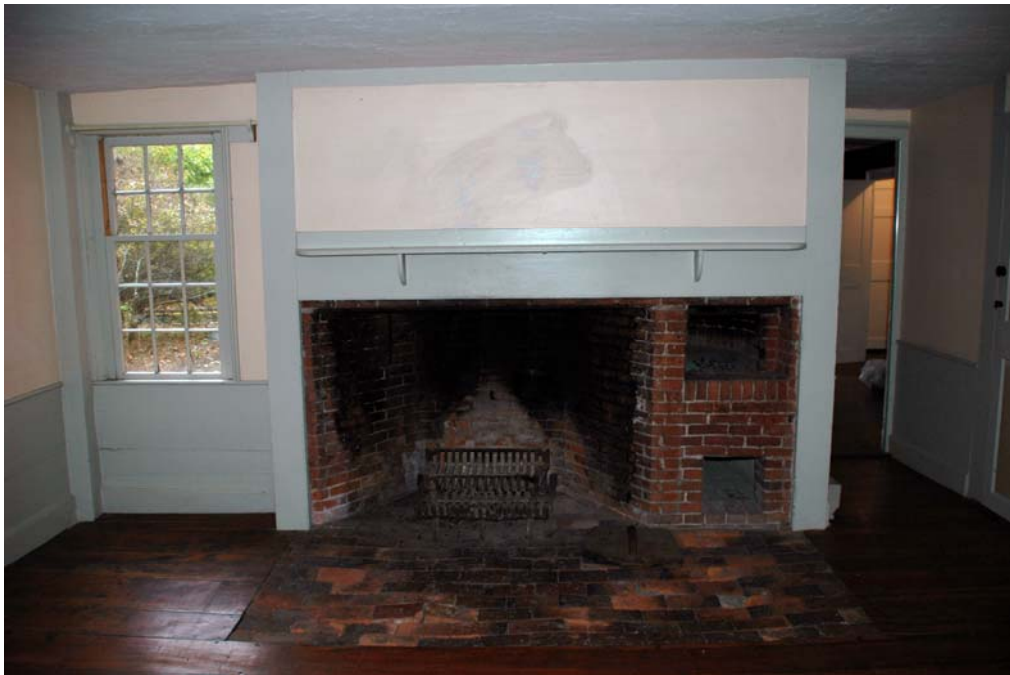
Figure 1.3A-19. Fireplace in Room 108.
