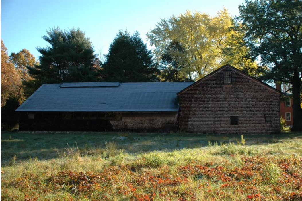
Figure WE-1. West elevation of the barn. The main block is on the right and the north block is on the left.
