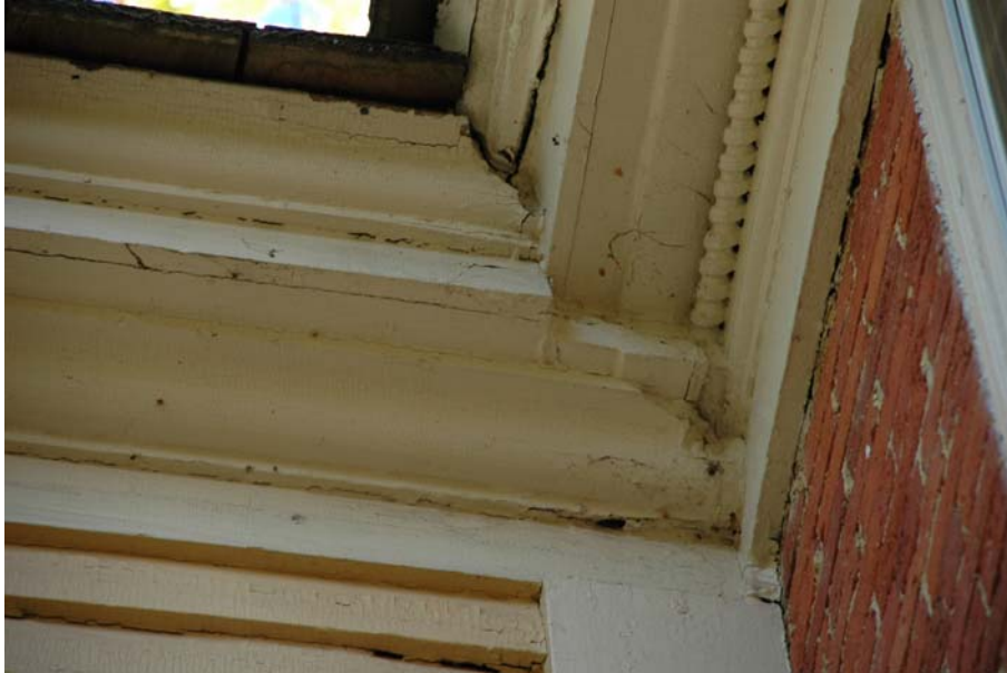
Figure 1.3A-12. Awkward intersection between roof eave cornices, northwest wing on the left and main block on the right.
