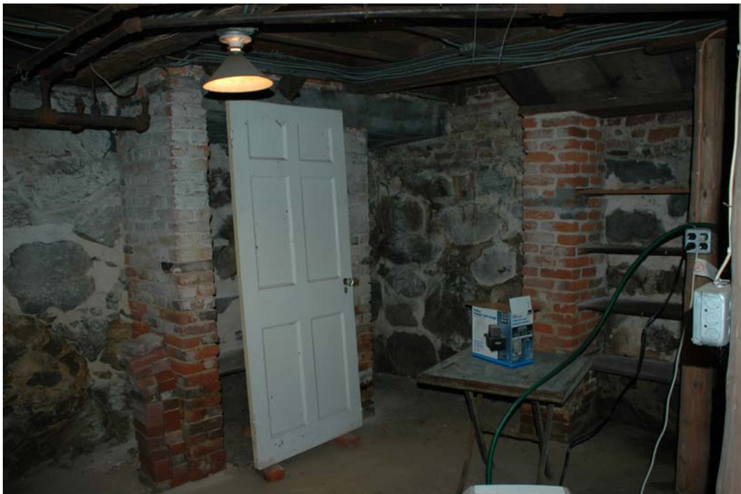
Figure 002-2. North and east walls of Room 002, with the brick supports under the Room 108 fireplace that were underpinned and reworked when the main block was constructed.
