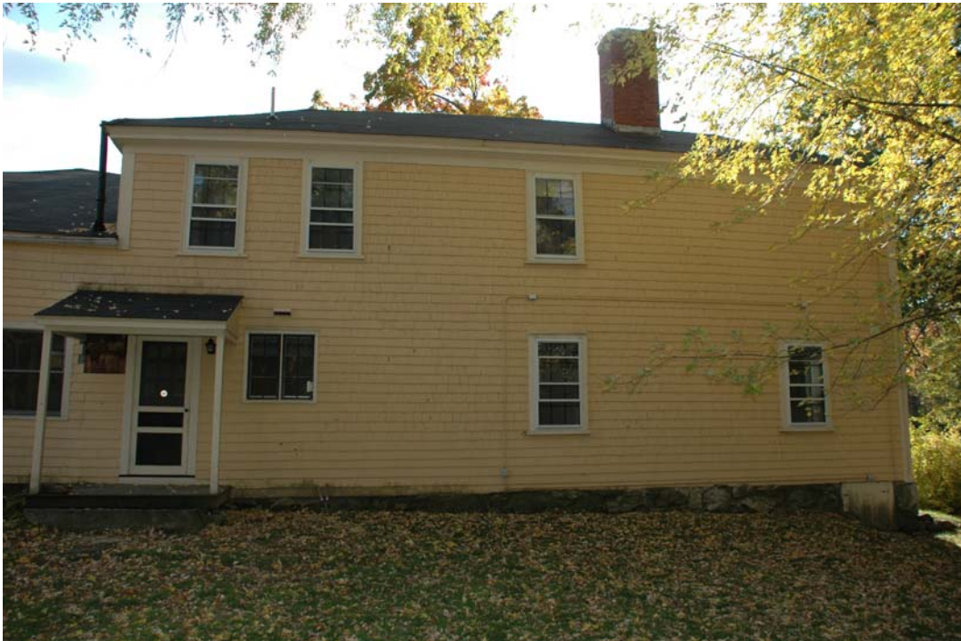
Figure NE-4. North Elevation of northwest wing.
