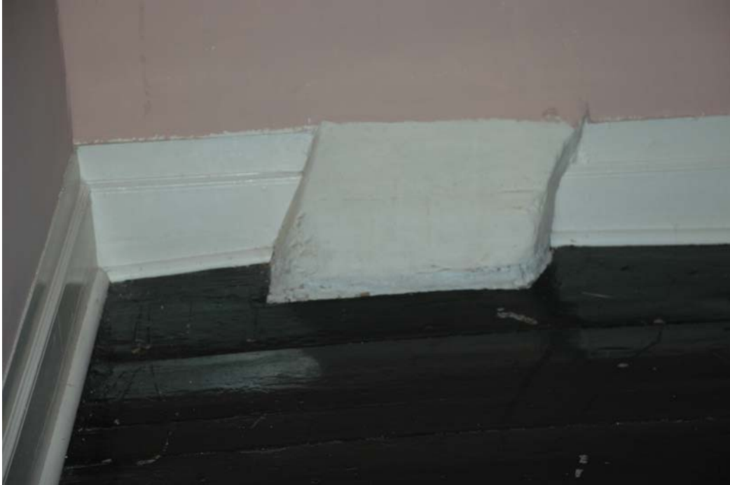
Figure 204-5. Room 204, exposed portion of masonry flue at northeast corner of room.
