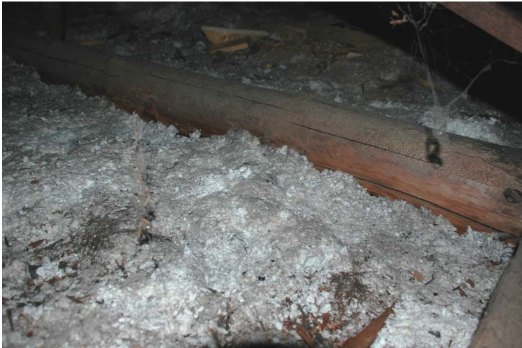
Figure 301-2. Room 301, the attic space in the west section of the main block showing the log ceiling joist, typical above Room 202, and cellulose insulation.
