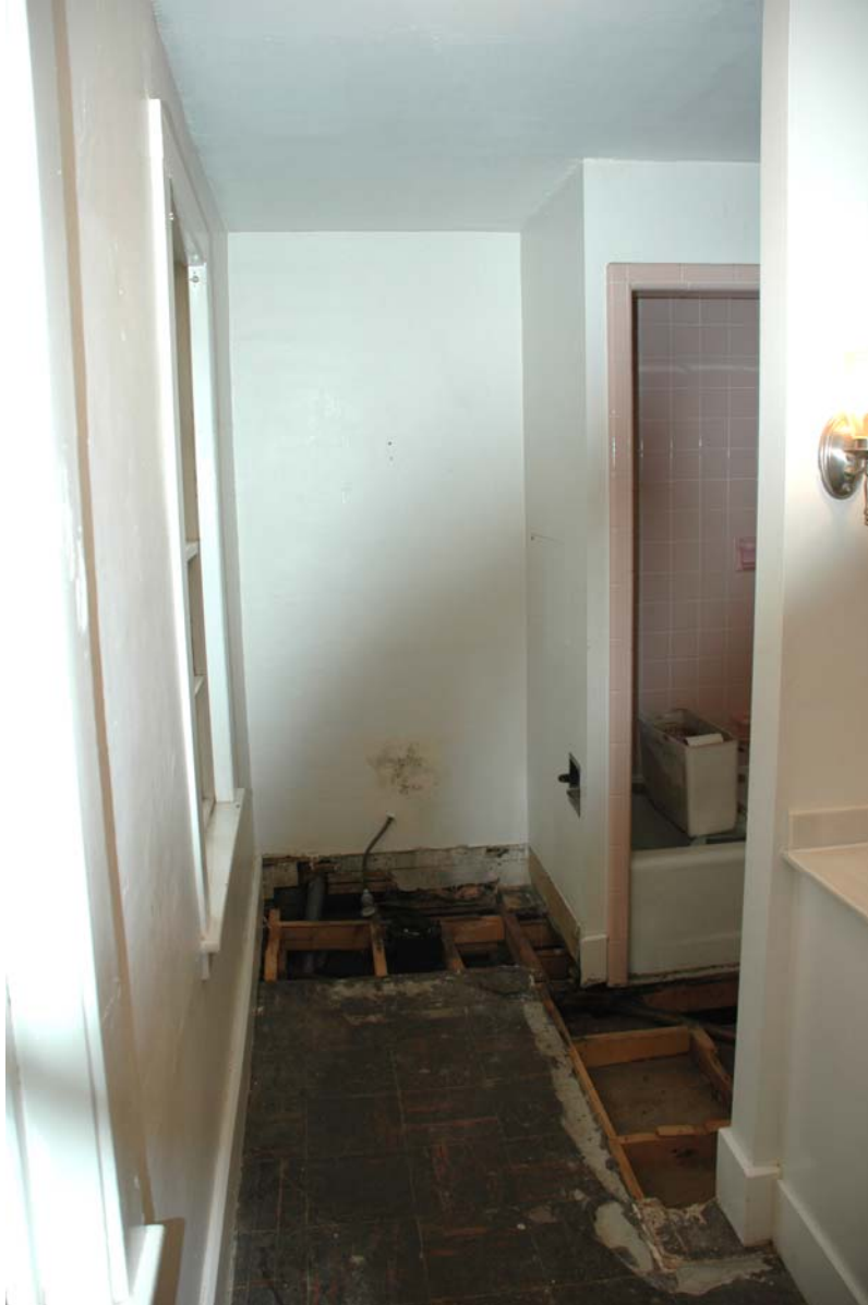
Figure 206-2. Room 206, looking east. A portion of the floor and subfloor was previously removed. Sleepers were installed to correct the sagging floor prior to the installation of the partition wall on the right, the bathtub and surround, and the tile floor.
