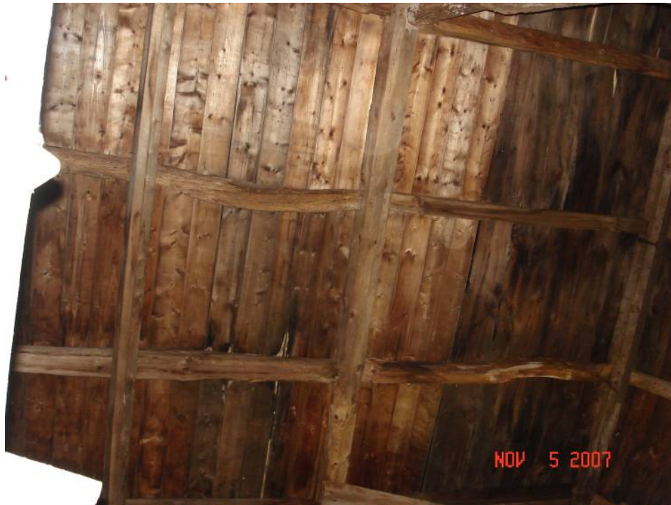
Figure BS-4. Buckled secondary rafters.
