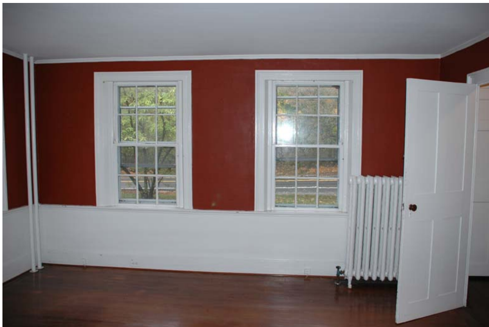
Figure 103-1. South elevation of Room 103 with Windows 108 and 107.
