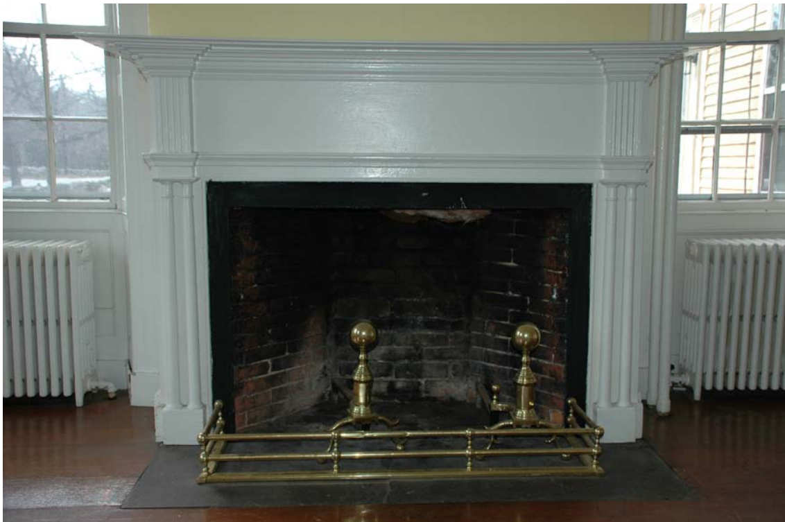
Figure 1.3A-20. Fireplace in Room 102.
