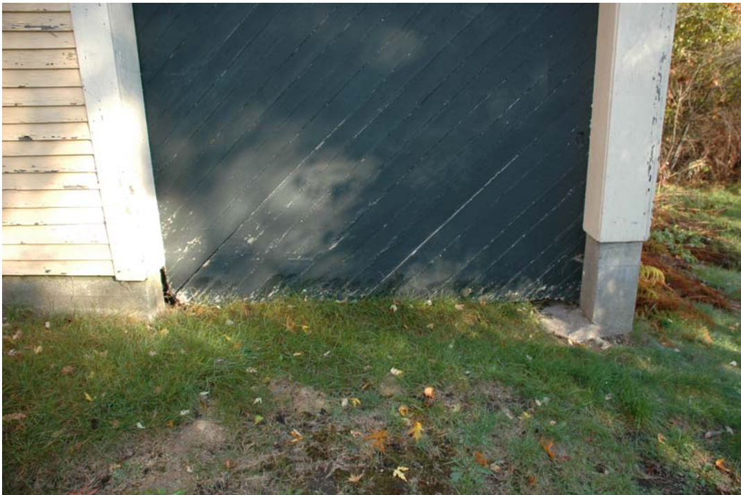
Figure SE-15. Door 1/110: detail showing deterioration at the lower edge of the diagonal-board carriage house door. The foundation at south elevation of carriage house is formed concrete.
