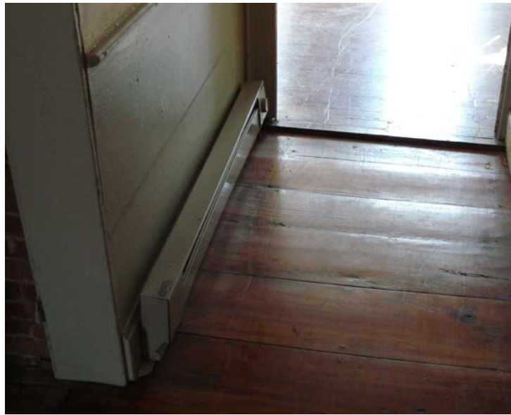
Figure H-3. Electric Baseboard.
