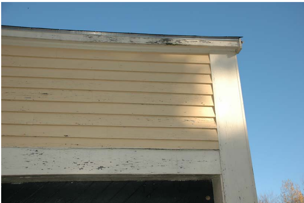
Figure SE-22. Deteriorated roof cornice at east side of northeast wing.
