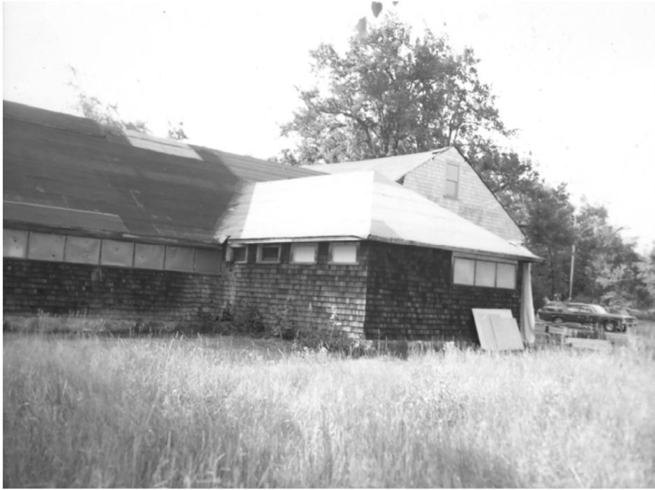
Figure 1.1B-2. West elevation of the Barn prior to the 1979 removal of the c.1900 west wing. Minute Man National Historical Park Archives, 1979.
