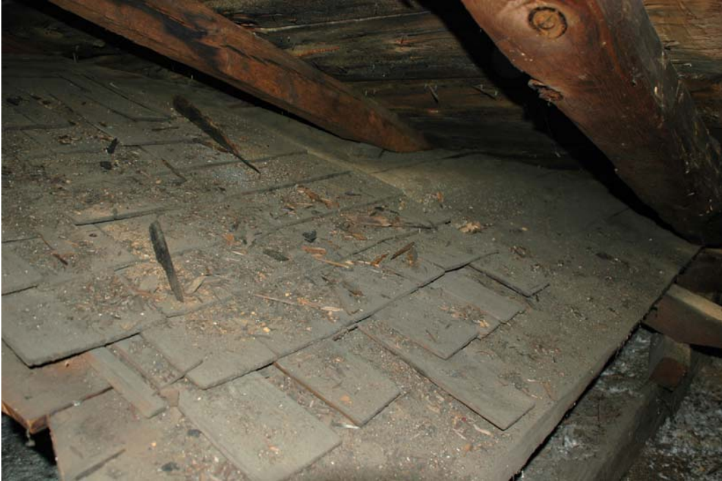
Figure 301-1. Room 301, looking west above the north side of the main block. The partial north main block hip roof, with sheathing boards and shingles intact, is visible with the northwest wing roof overframing above.
