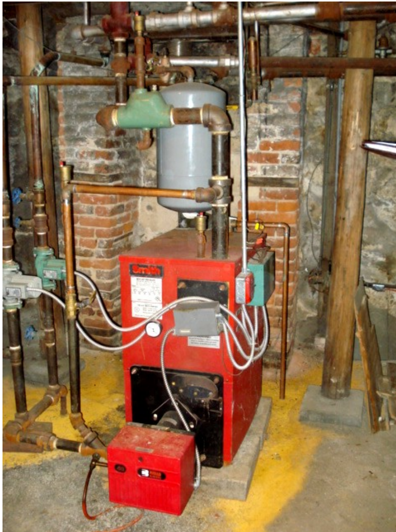
Figure H-1. Hot water boiler.
