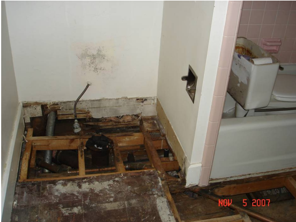
Figure S-9. Shimmed floor at northeast corner.
