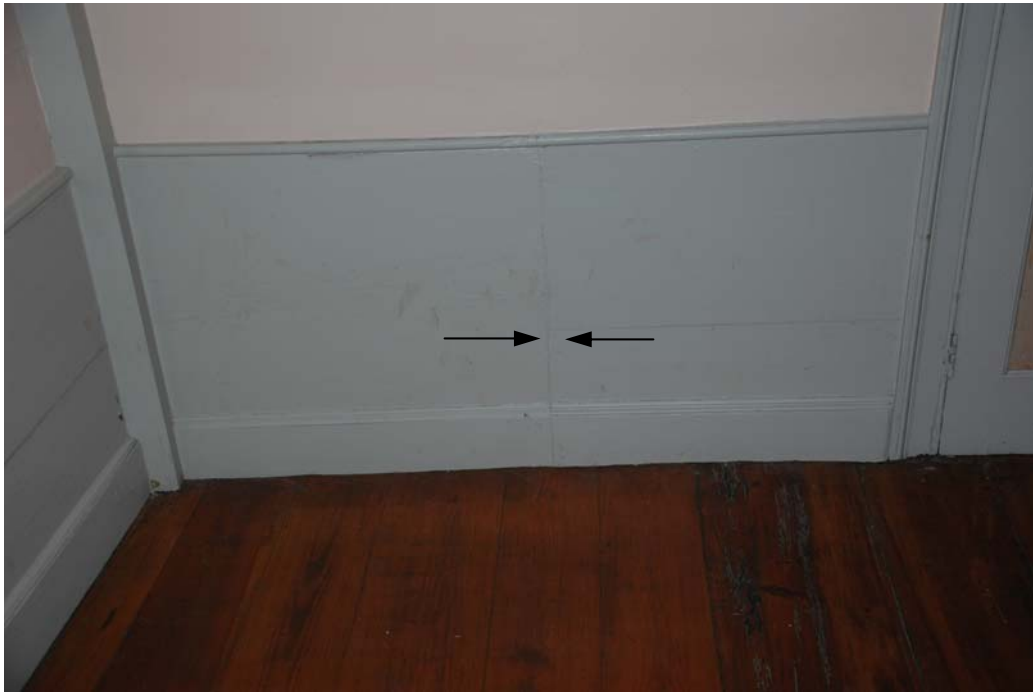
Figure 108-2. North section of the East elevation of Room 108, showing the joint in the chair rail, wainscot and baseboard indicating that the north section was infilled (see arrows in the photo).
