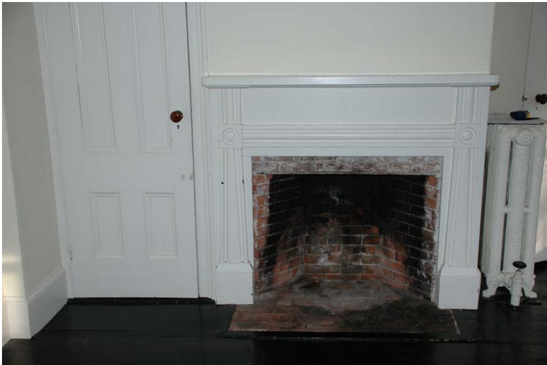
Figure 1.3A-27. Fireplace in Room 208.
