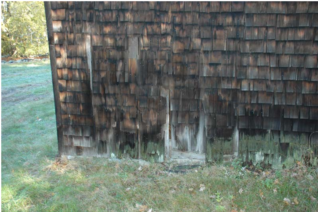
Figure SE-2. Deteriorated shingles, wall sheathing and sill plate at west corner of the south elevation, main block.
