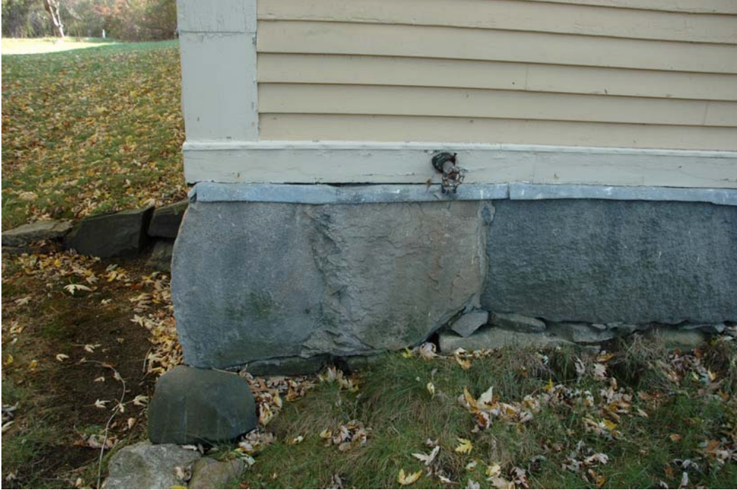
Figure WE-4. Foundation wall at west elevation of northwest wing.
