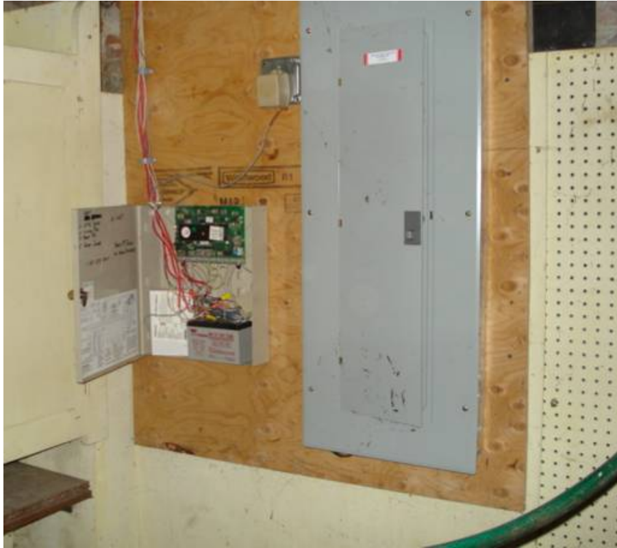
Figure E-3. Main panelboard.
