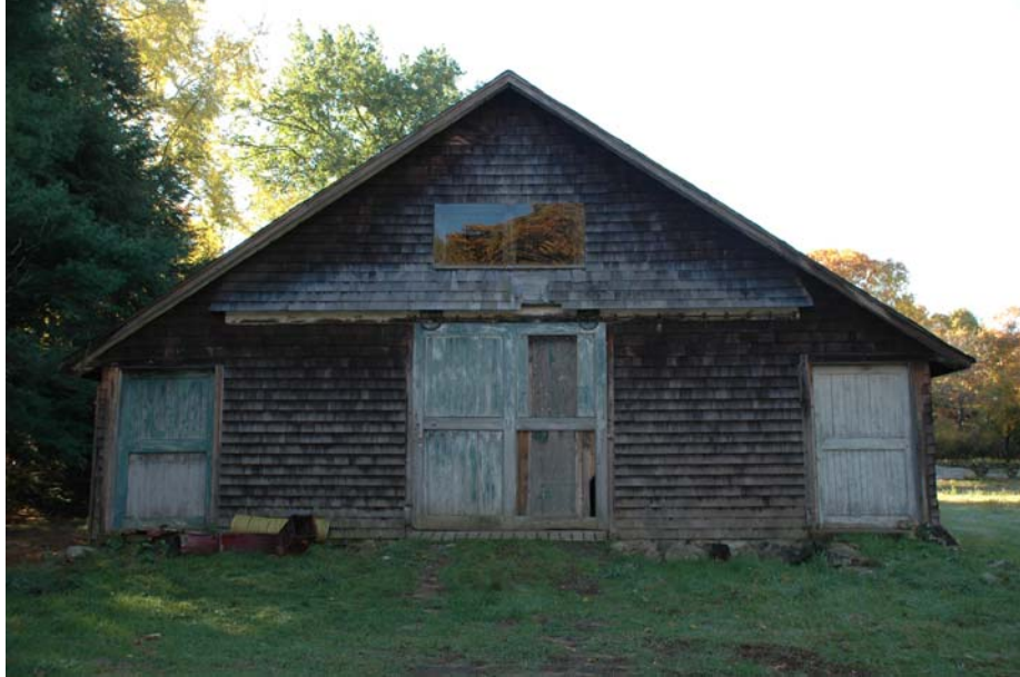
Figure NE-1. North elevation of the barn, north block.
