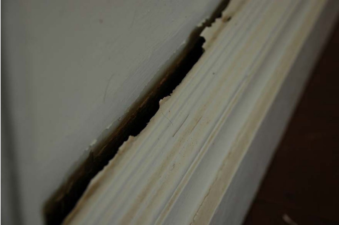
Figure 1.3A-29. Paint markings on the wainscot behind the baseboard in Room 102, below the height of the current paint markings, suggest that the baseboard was originally installed slightly lower. The baseboard may have been removed for the current floor installation and then reinstalled.
