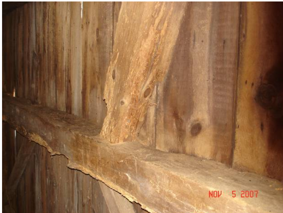
Figure BS-10 & 11. Deteriorated/missing structural members.
