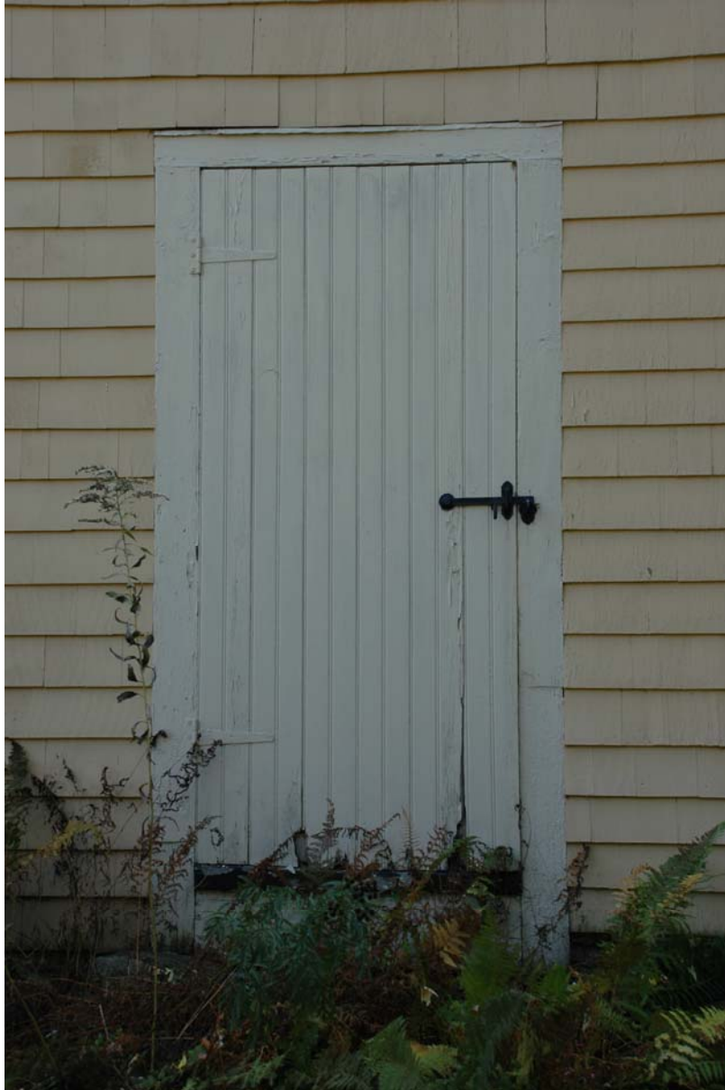
Figure NE-10. Door 2/109: board-and-batten door with deterioration along the bottom and the sill.
