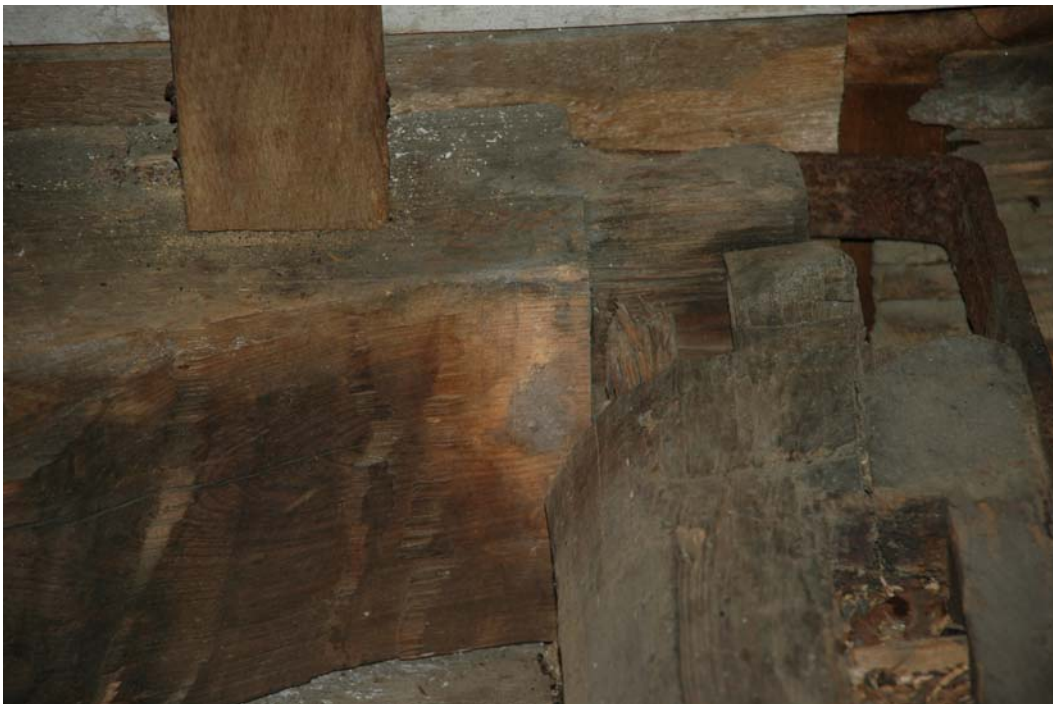
Figure 210-4. Room 210, showing the original tenon plates at the northeast corner of the 18 th century block (the corner post is missing).
