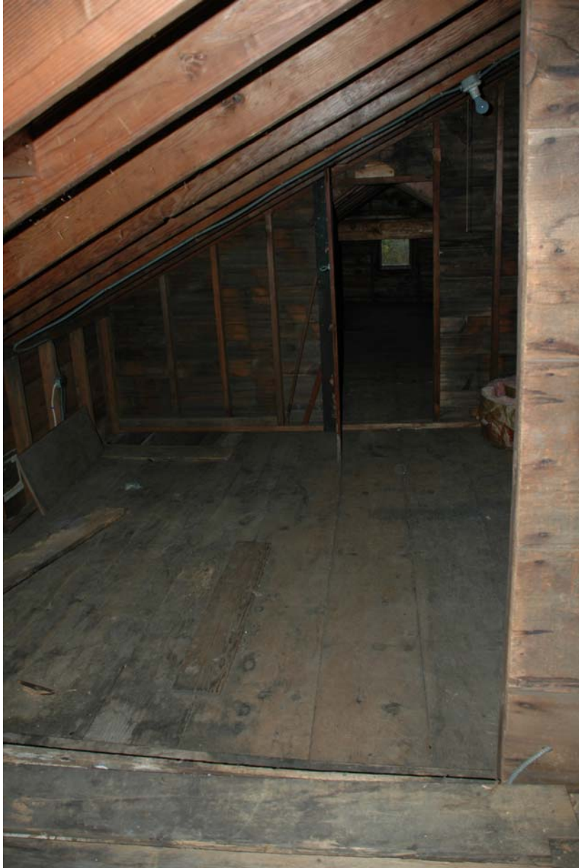
Figure 209-4. Room 209, looking east. The attic space is above the original 18 th century block. The partition wall in the right foreground with horizontal sheathing boards and wrought nails is possibly 18 th century, however further investigation is needed to determine this. The frame partition wall in the background was added later and divides the original 18 th century attic space.
