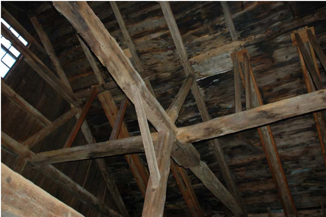
Figure B101-2. Room B-101, showing repairs to the rafters and roof sheathing.
