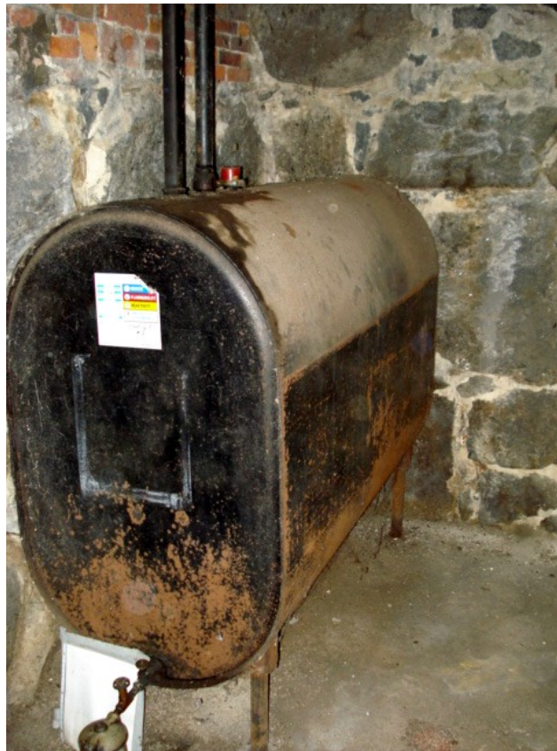
Figure H-2. Heating Oil Tank.
