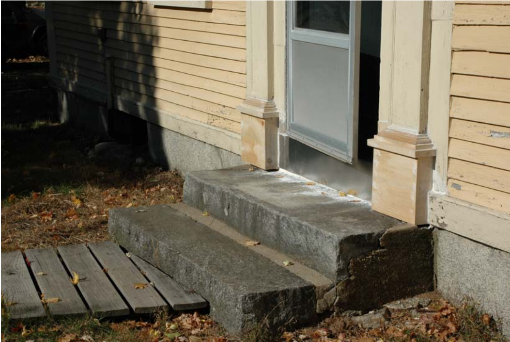
Figure SE-11. Detail of Door 1/101 showing new aluminum flashing at the sill and replaced pilaster bases. The granite slab steps were previously repaired with incompatible cement-based mortar.
