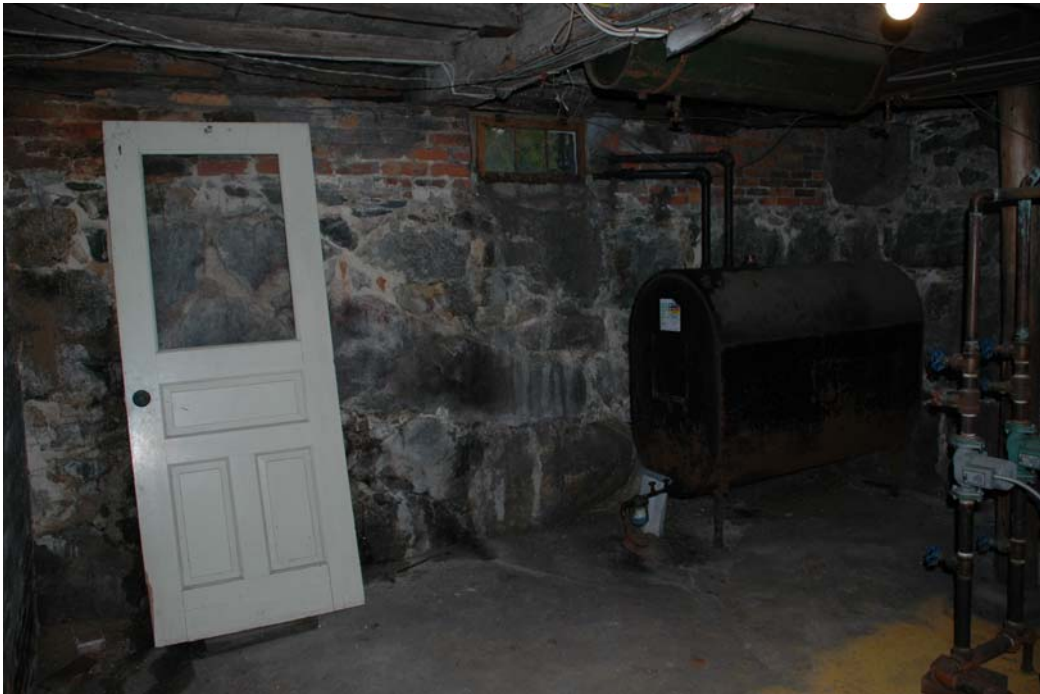
Figure 001-2. South wall of Room 001 with Window #001.
