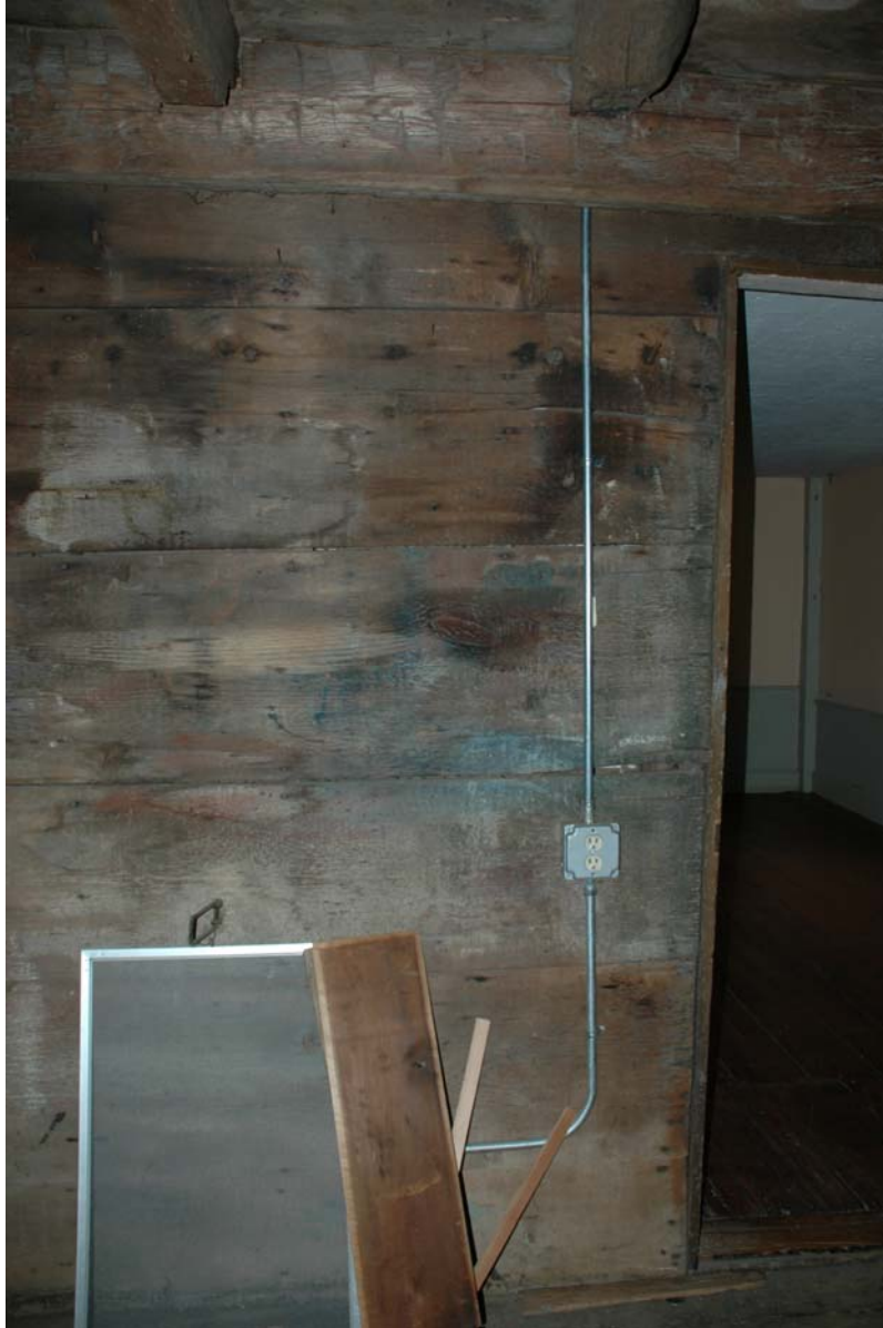
Figure 109-1. West elevation of Room 109. The horizontal wall boards are possibly the original exterior sheathing boards of the 18 th -century block.
