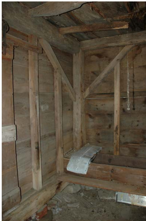
Figure 110-1. West and north elevations of Room 110. The room was constructed of what appears to be salvaged antique materials.
