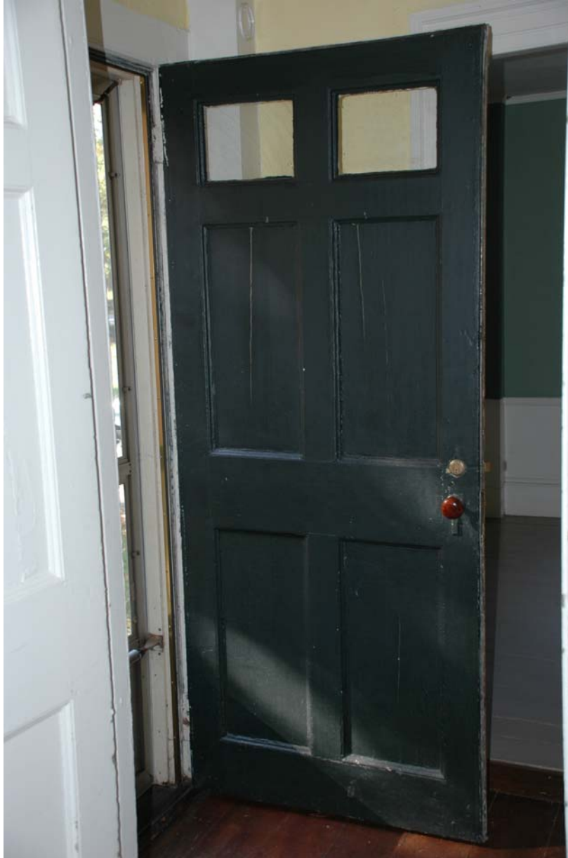
Figure 105-1. Room 105, looking west. Door 1/105 is open to the exterior face.
