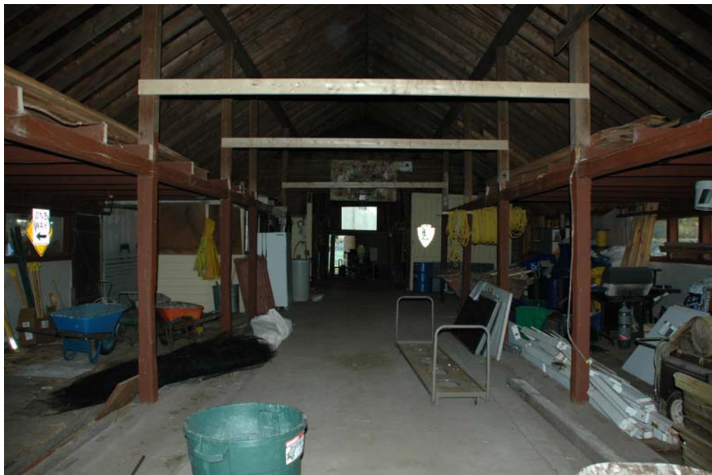
Figure B102-2. Room B-102, looking south toward Door B-2/101 and Room B-101.
