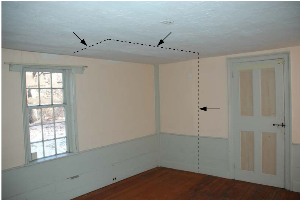
Figure 108-3. Room 108, northeast corner showing scars on north wall, ceiling and floor where the conjectured partition walls and staircase were located.
