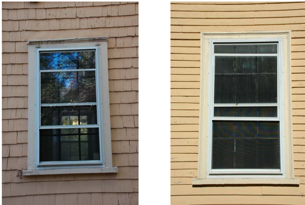
Figure 1.3A-5. Windows Type A on the left and B on the right.
