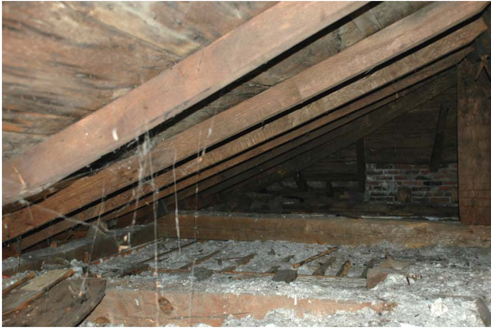
Figure 301-3. Room 301, looking east in the attic above the main block. The chimney mass and king post are in the right background. The roof rafters and board sheathing (now overframed by the northwest wing) are in the right foreground.
