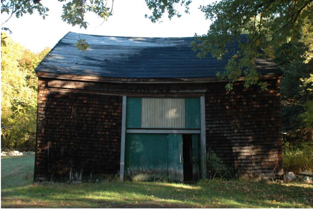
Figure SE-1. South elevation of Barn at the main block.
