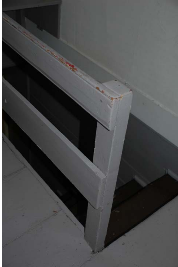
Figure 205-6. Room 205, staircase and railing.
