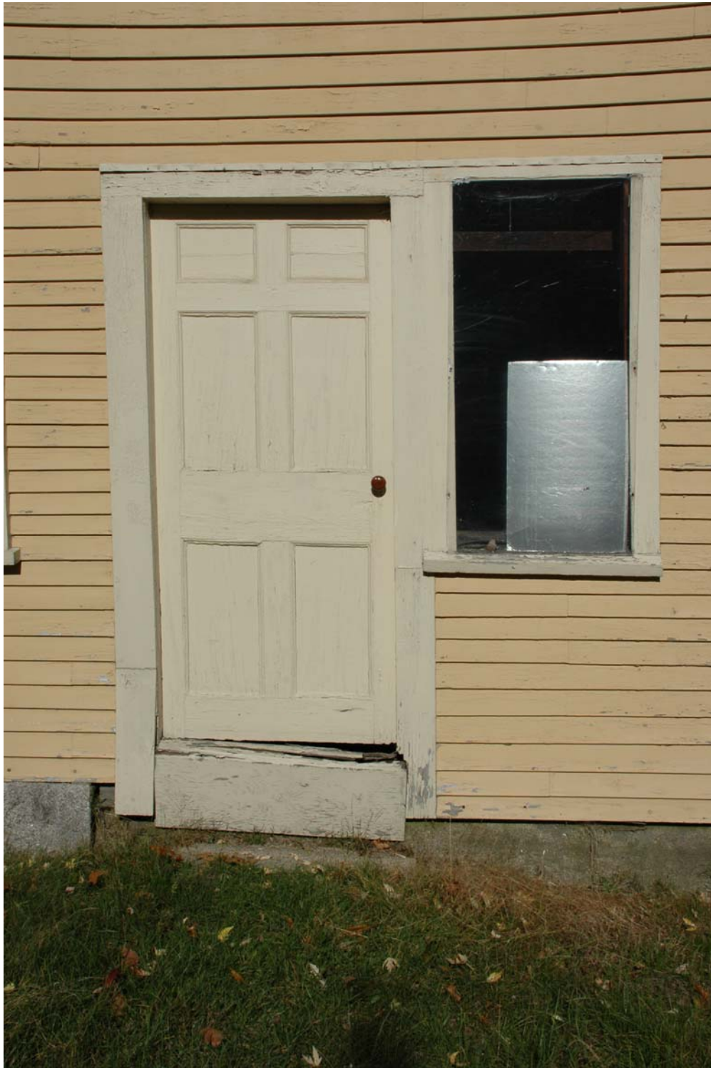
Figure SE-13. Door 1/109 and Window #111, Type w-D. The door sill is extremely deteriorated. The window sash is missing and has been replaced with a single piece of Plexiglas. The foundation wall is granite block on the left of the door, at the 18 th century block, and formed concrete to the east of this point.
