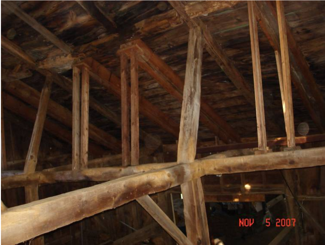
Figure BS-5. Shoring struts supporting the north roof.
