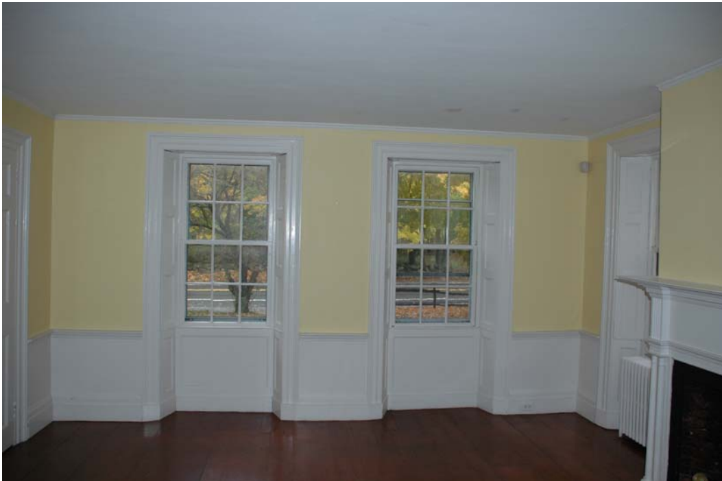
Figure 102-1. South elevation of Room 102, showing the splayed and paneled window jambs with recessed sills.
