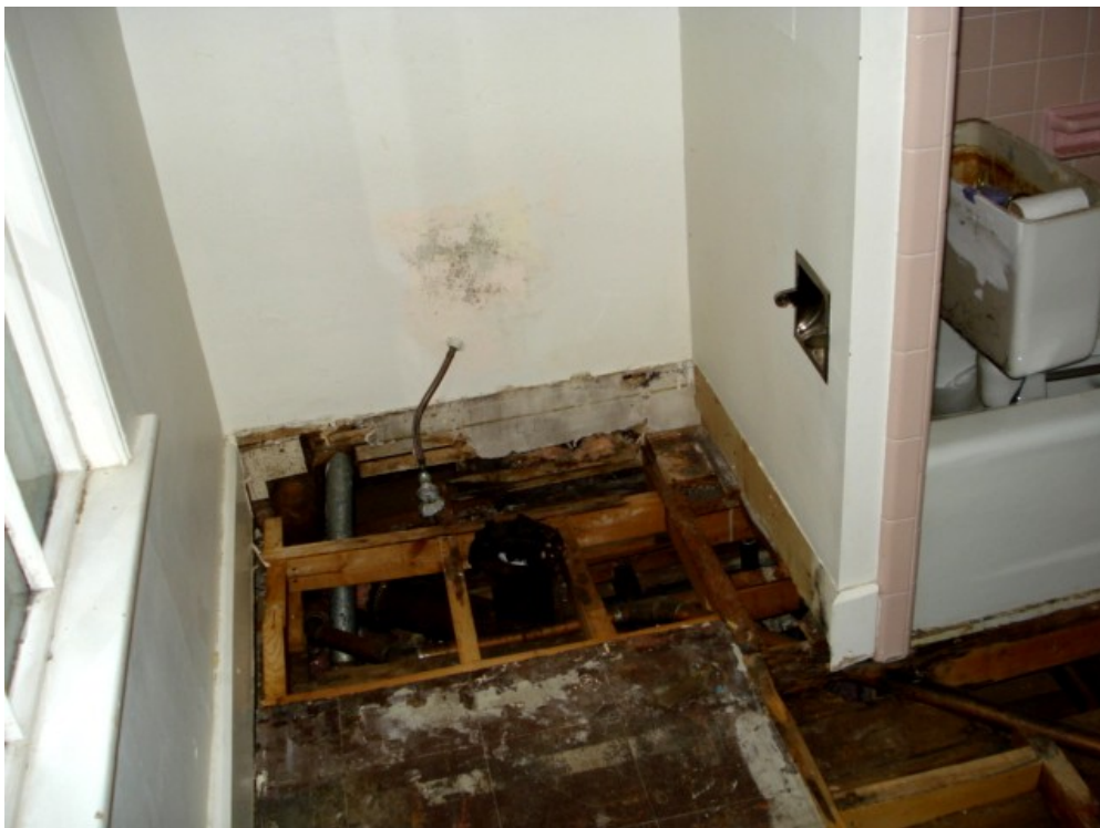
Figure P-3 & 4. Upper Level Plumbing Fixtures.
