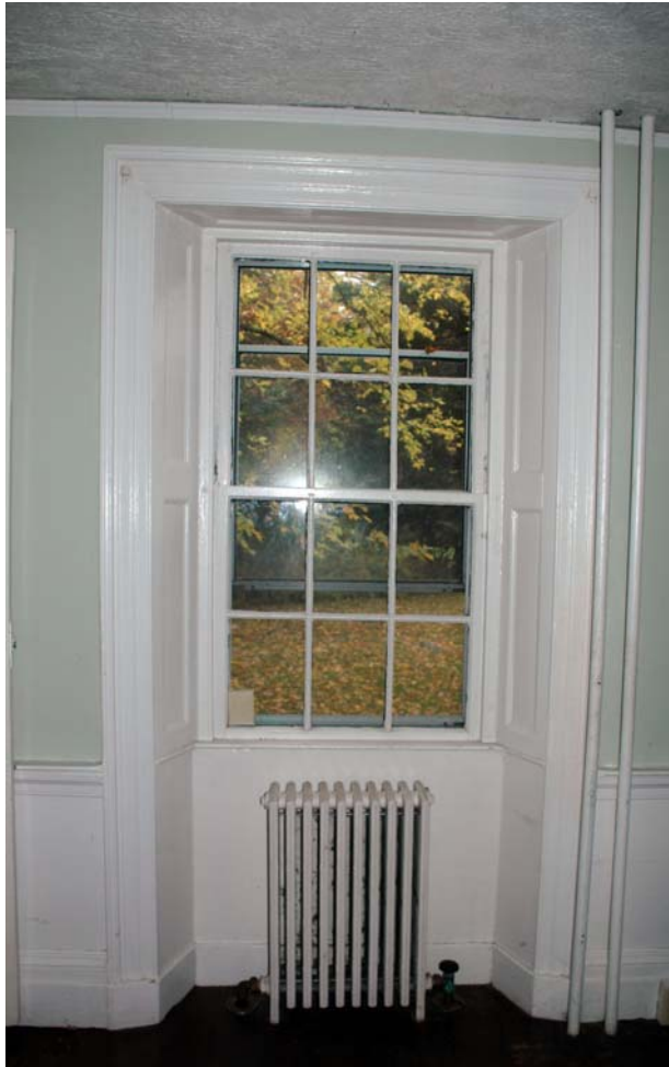
Figure 106-9. Room 106, window elevation with paneled jambs above the sill and horizontal board wainscot below.
