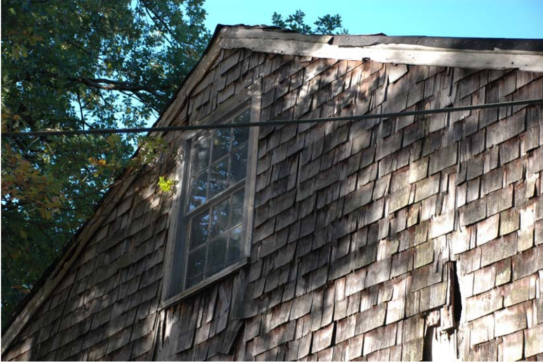
Figure EE-2. Detail of east gable end at main block with window #B-201.
