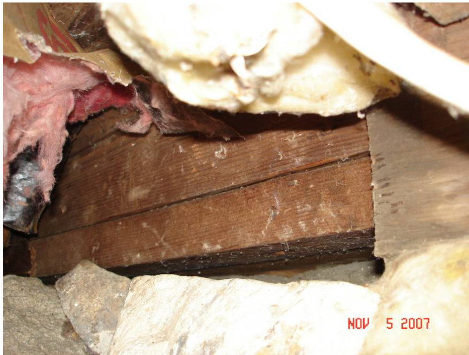
Figure S-6. Replaced section of south sill beam below door.
