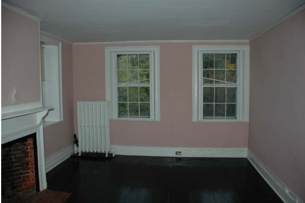
Figure 204-1. South elevation of Room 204, with Windows 209 & 210.
