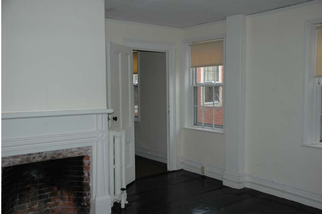
Figure 208-2. Southeast corner of Room 208. Door 1/208 leads to Room 207. The boxed-out area to the right of Window 202 most likely conceals a frame post. This post aligns with the post located directly below in Room 105. The posts in the northeast and southeast corners may have been part of an earlier exterior frame wall.
