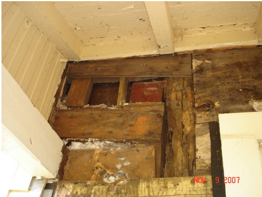
Figure S-8. Deteriorated post with exposed end of sister beam located to the left.
