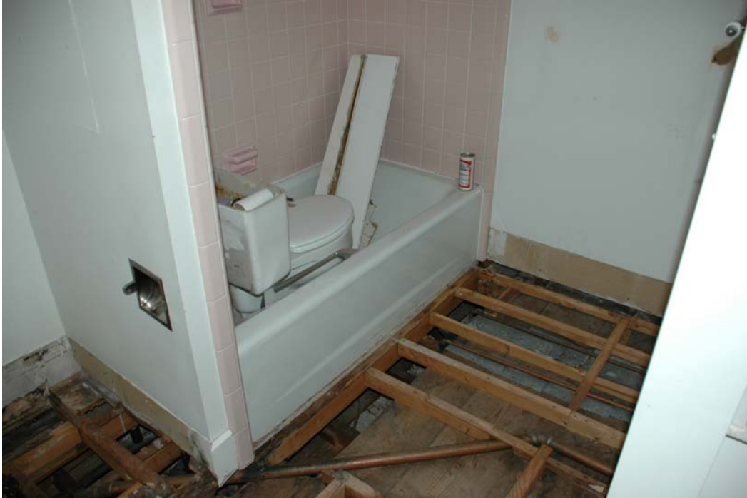
Figure 206-3. Room 206, looking southeast showing removed finish floor and leveling sleepers on top of the original floorboards, which run continuous under the south wall that separates Room 206 from Room 205.
