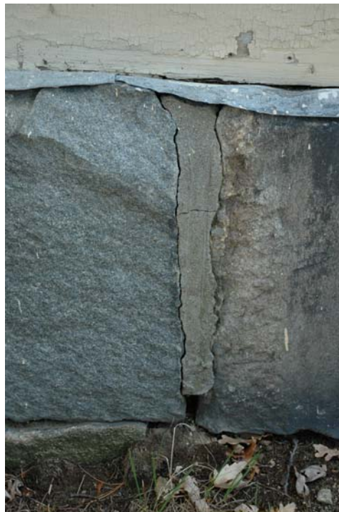
Figure WE-5. Detail of west elevation foundation wall showing condition of shrunken and cracked mortar.
