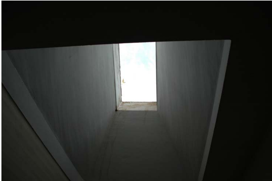
Figure 205-4. Skylight in Room 205.
