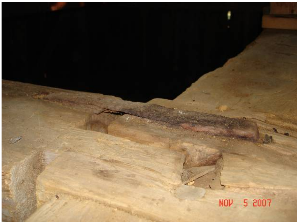
Figure BS-12 & 13. Tenon pull-out at upper tie-beam.
