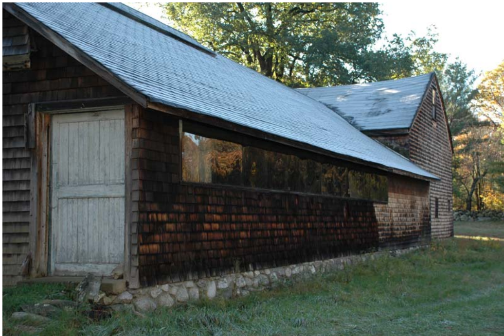
Figure WE-2. West elevation of the north block, looking towards the southeast.
