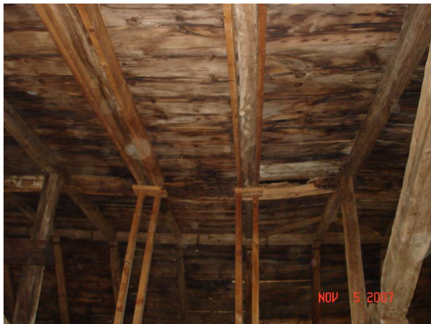
Figure BS-9. Sagging and deteriorated framing under north block roof projection.
