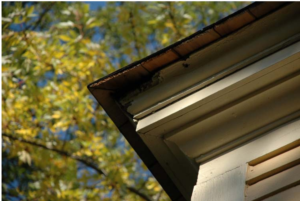
Figure 1.3A-11. John Nelson House eave cornice at the northwest wing.
