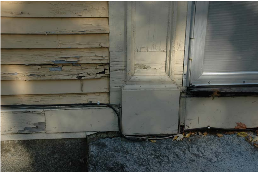
Figure SE-8. Condition of sill, pilaster, wood siding and apron board at Door 1/105.
