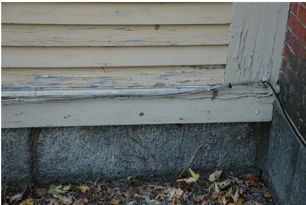
Figure SE-6. South Elevation foundation wall at northwest wing where it meets the main block, showing condition of granite foundation wall, mortar, apron board, siding and corner board.
