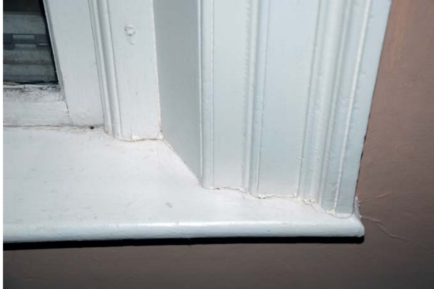
Figure 1.3A-36. Splayed window jamb at Room 201.
