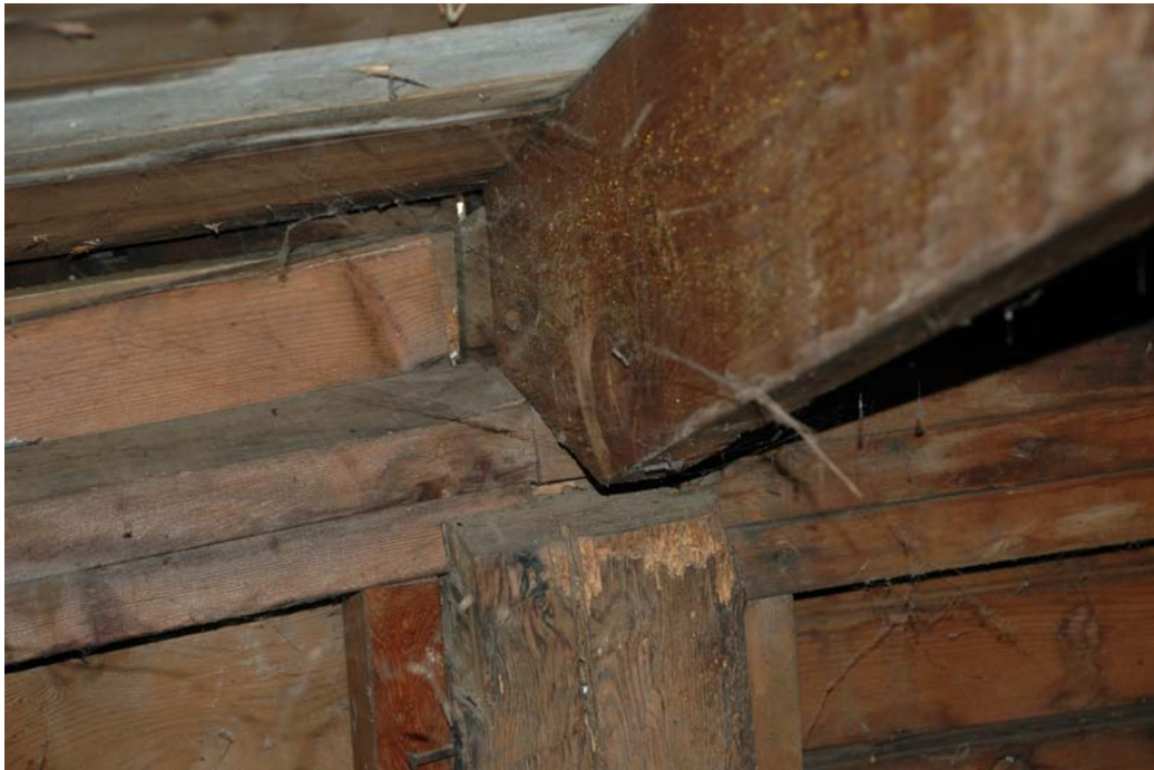
Figure 209-3. Room 209, detail of cut-off 18 th century structure corner post on north wall, as well as later roof plate, rafter, and knee wall framing.
