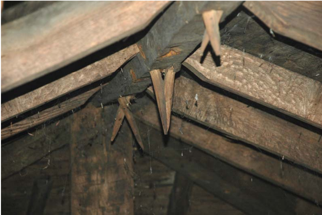
Figure 301-4. Room 301, view of the 5-sided ridge beam in the main block with pegged rafters and king post in the background.
