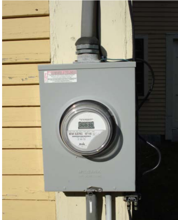
Figure E-2. Utility meter.
