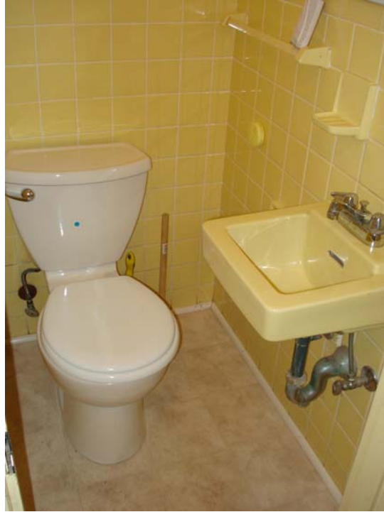
Figure P-5. Lower Level (half bath) Plumbing Fixtures.
