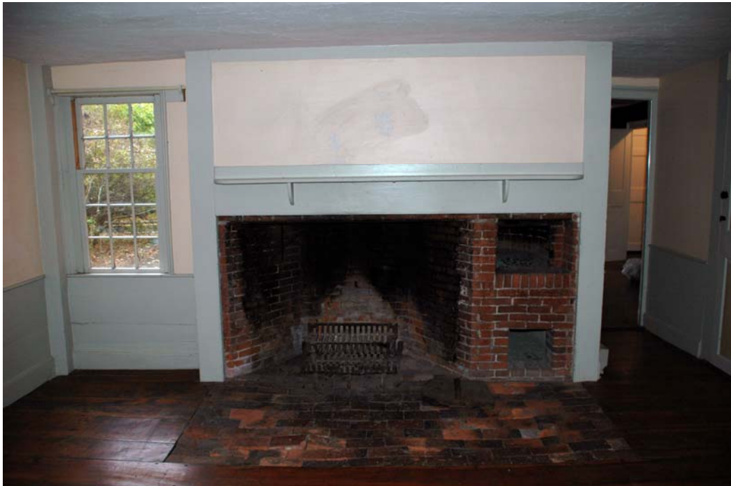
Figure 108-6. Room 108, south elevation with Window 110 and Door 2/103.
