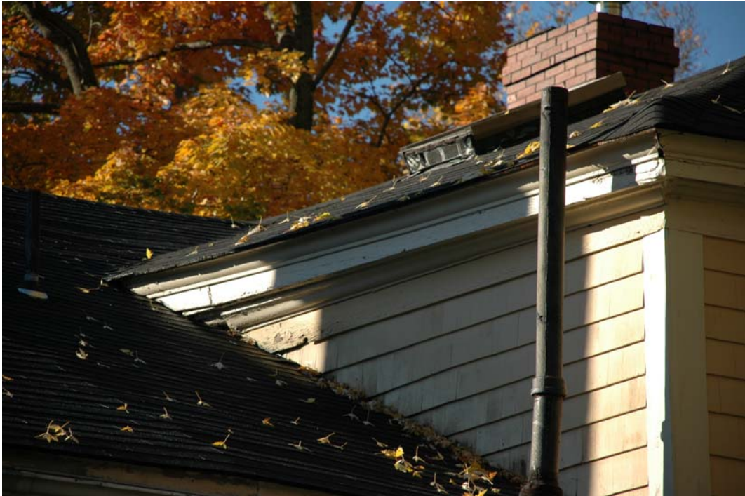
Figure EE-7. The exposed portion of the northwest wing at the east elevation. The skylight (window # 218) can be seen above the roof eave, below the chimney.
