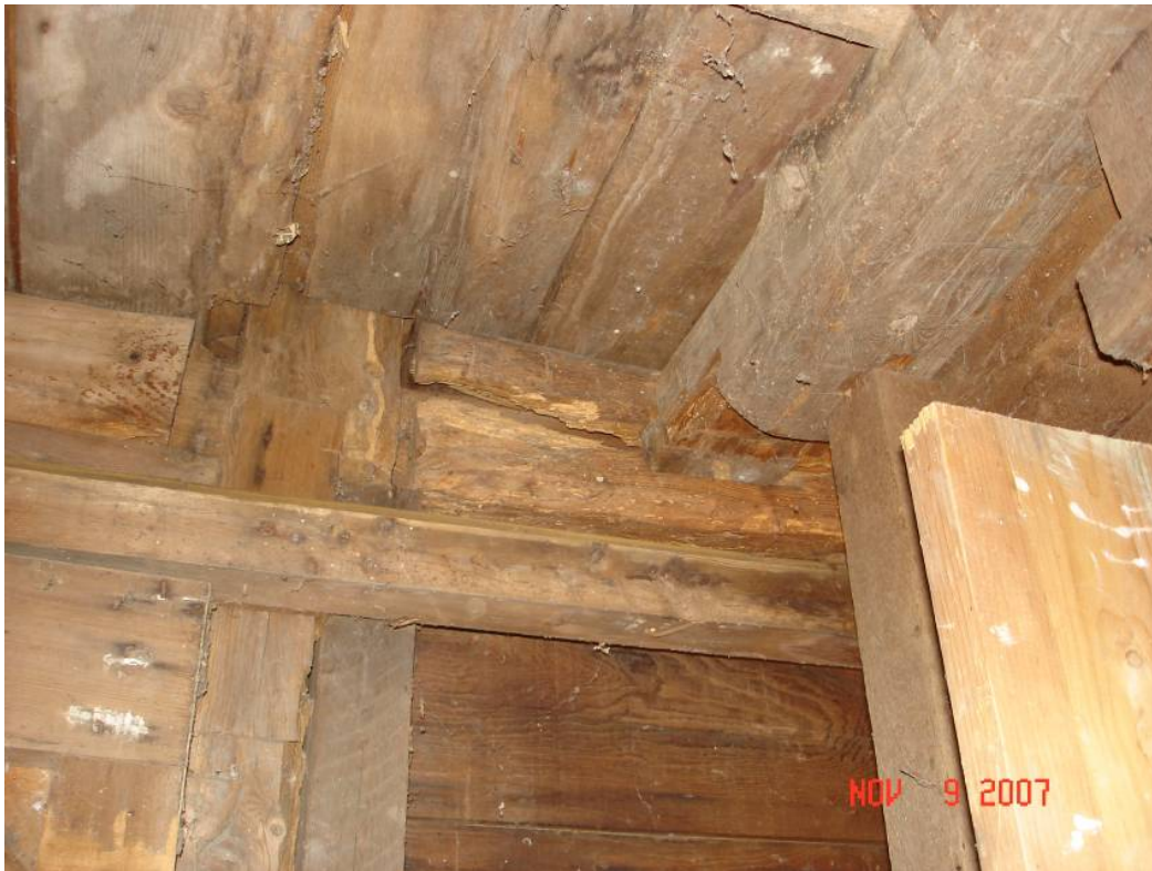
Figure S-15. Tenon pullout on tie-beam at south wall.
