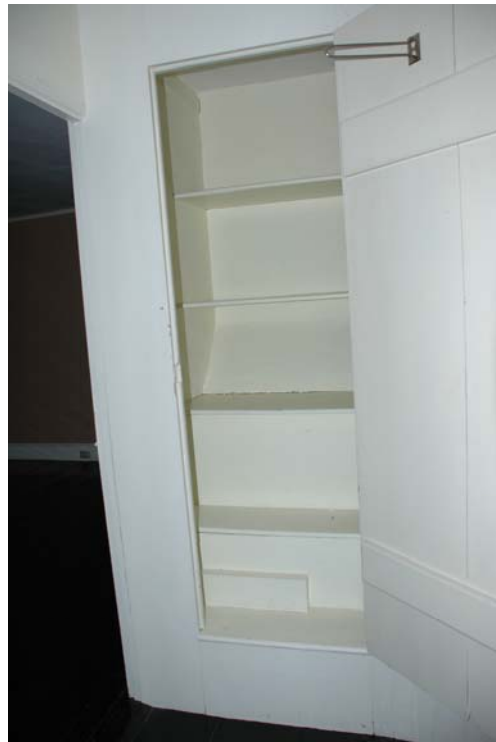
Figure 203-2. North elevation of Room 203 with Door 2/203 that leads to a closet.
