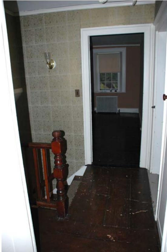
Figure 201-1. West elevation of Room 201, with Door 1/202 leading to Room 202.
