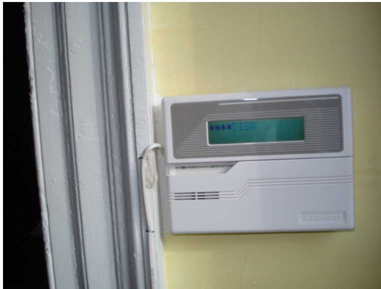
Figure E-5. Security key pad.
