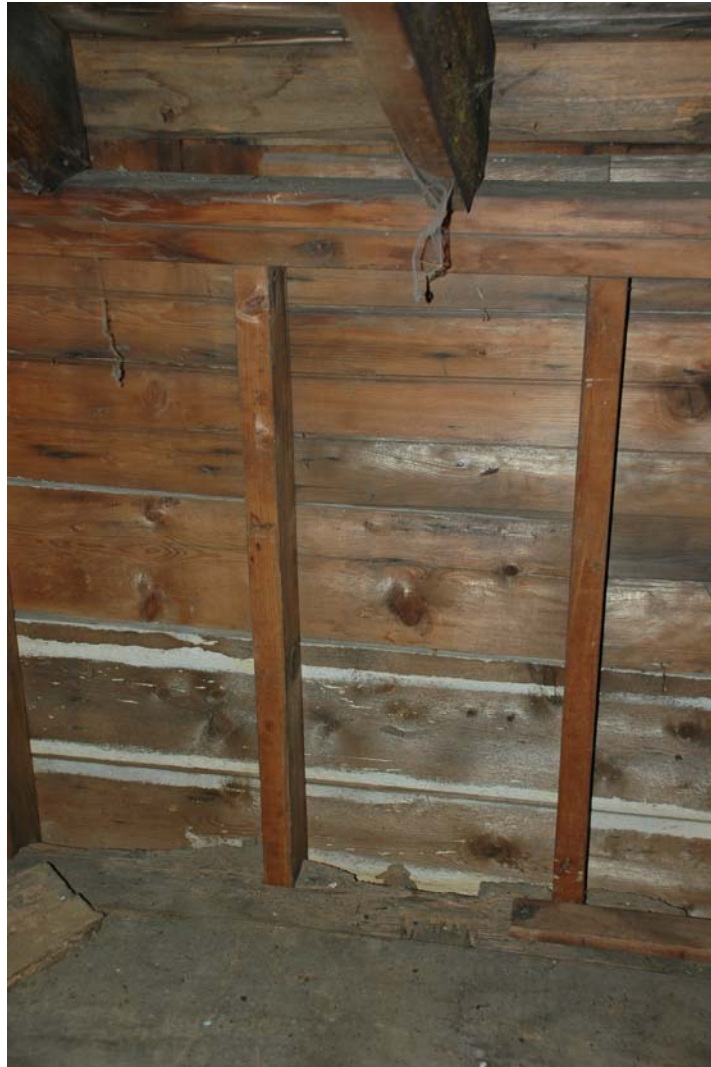
Figure 209-1. Room 209, knee wall along north wall. The wall stud members appear to have been added, as the original sill plate below has empty pockets that would have contained the original wall studs.
