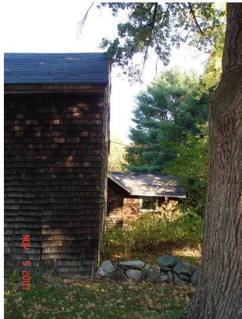
Figures BS-6 & 7. Roof line and soffit line sag – the structure is out of plumb.
