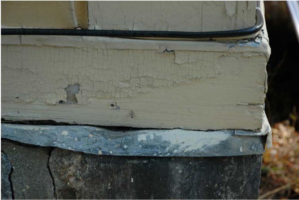
Figure WE-8. Corner board and apron at the west elevation of the northwest wing, exhibiting cracked and peeling paint.
