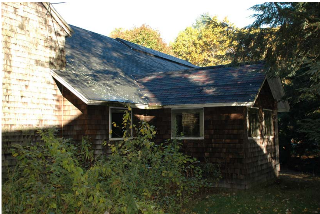
Figure EE-3. East elevation of c. 1830's north block addition on the left and the c. 1900 east wing addition on the right.
