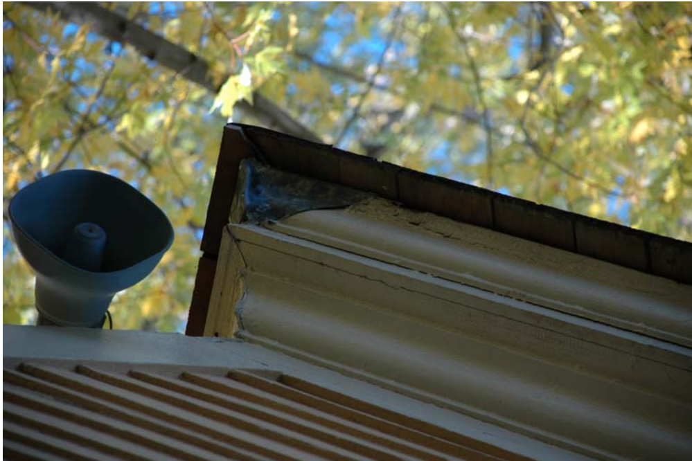
Figure WE-9. Roof cornice at west elevation, with deteriorated crown molding covered with metal. An alarm speaker is attached to the adjacent wall.
