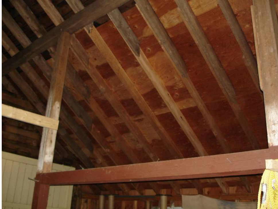
Figure BS-16. Roof framing at southeast corner.
