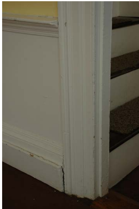
Figure 1.3A-28. Door casing, Room 102. The window casing in this room is similar.
