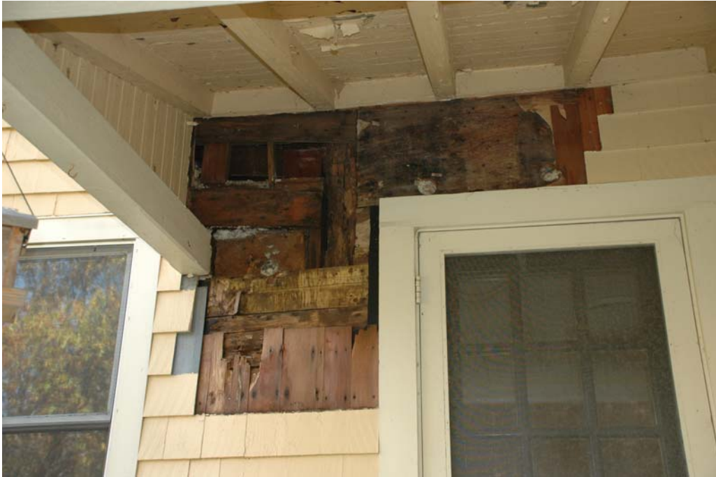
Figure NE-8. Wall under rear porch where shingles and sheathing were removed to expose deteriorated framing behind.
