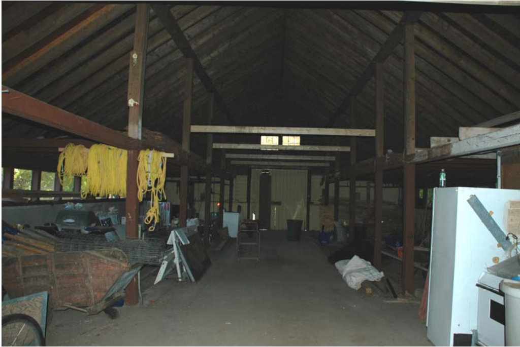
Figure B102-1. Room B-102, looking north toward Door B-3/102 in the center and Doors B-4/102 and B-2/102 on the left and right.
