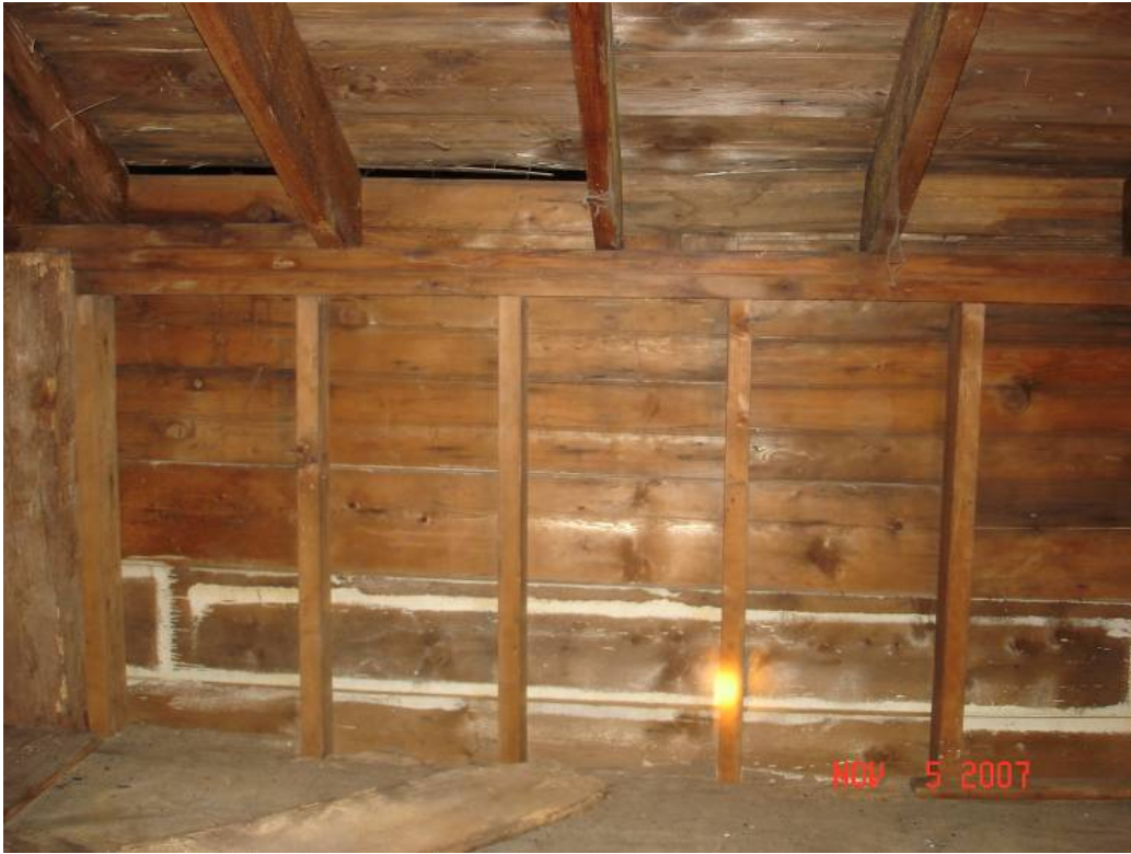
Figure S-13. Framing at north wall of the original 18 th century block.
