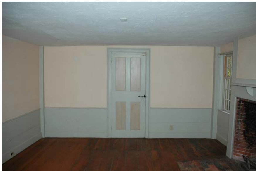
Figure 108-1. East elevation of Room 108 with Door 2/108 that leads to Room 109.
