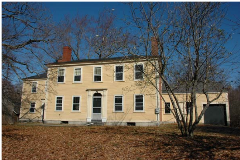
Figure 1.3A-4. South elevation of the John Nelson House.
