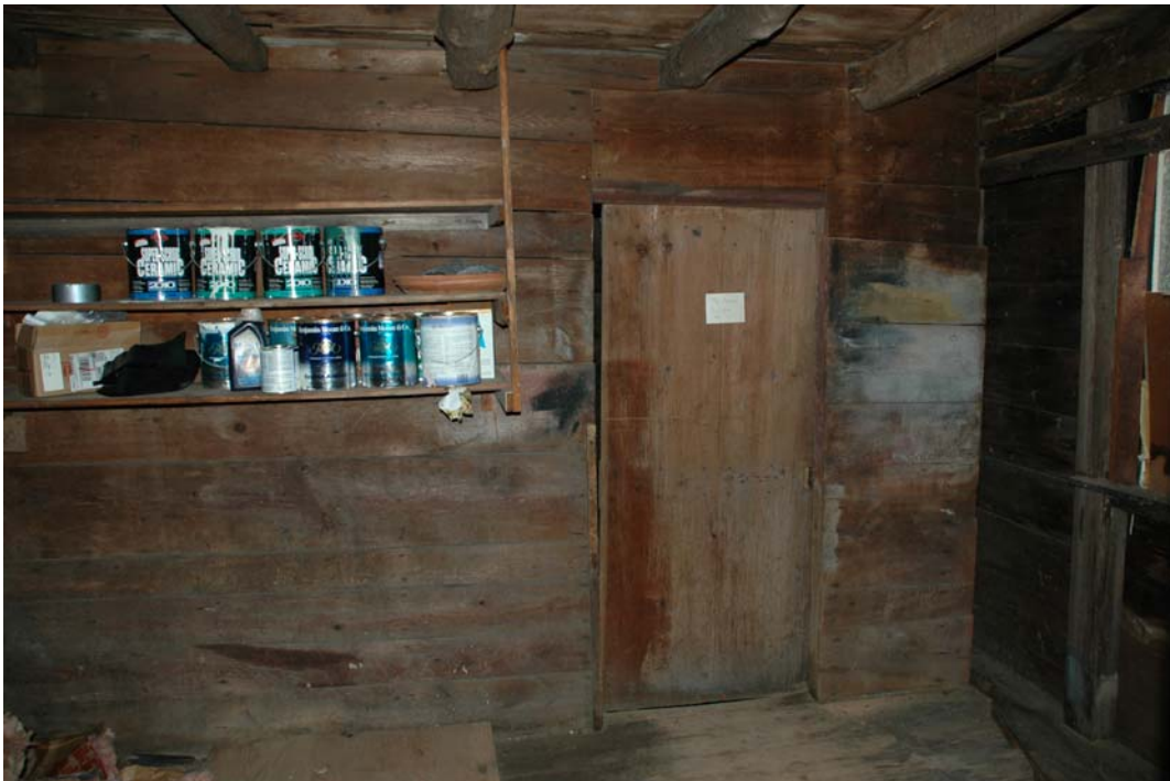
Figure 109-3. Room 109, east elevation with Door 2/110. The room was constructed of what appears to be antique materials salvaged from another building.
