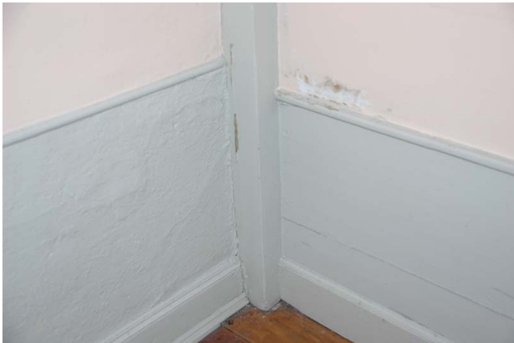
Figure 108-5. Room 108, detail of northwest corner with exposed corner post. The west wall (on the left) is plaster below the chair rail while the north wall (on the right) is horizontal board wainscot. The chair rails do not align and the west wall has a different baseboard and an added shoe molding.
