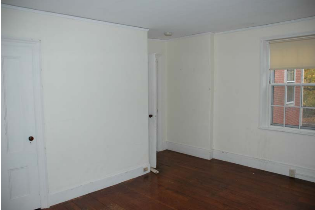
Figure 207-2. Room 207, looking southeast. Door 2/207 on the left leads to a closet and Door 1/207 on the right leads to Room 205. The wall in the southeast corner is boxed out in the vicinity of where the northwest corner of the main block meets the northwest wing, on the other side of the wall.
