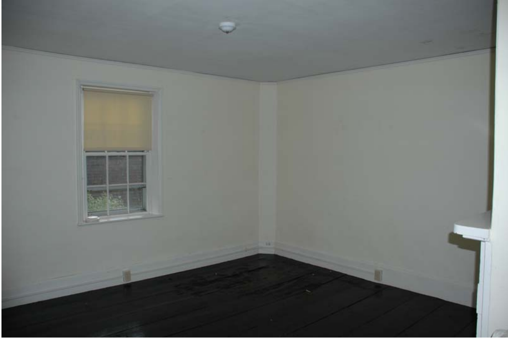
Figure 208-4. Room 208, looking northwest with an angled corner finish, most likely enclosing a corner post. An area of heavily damaged floor boards is near the corner.
