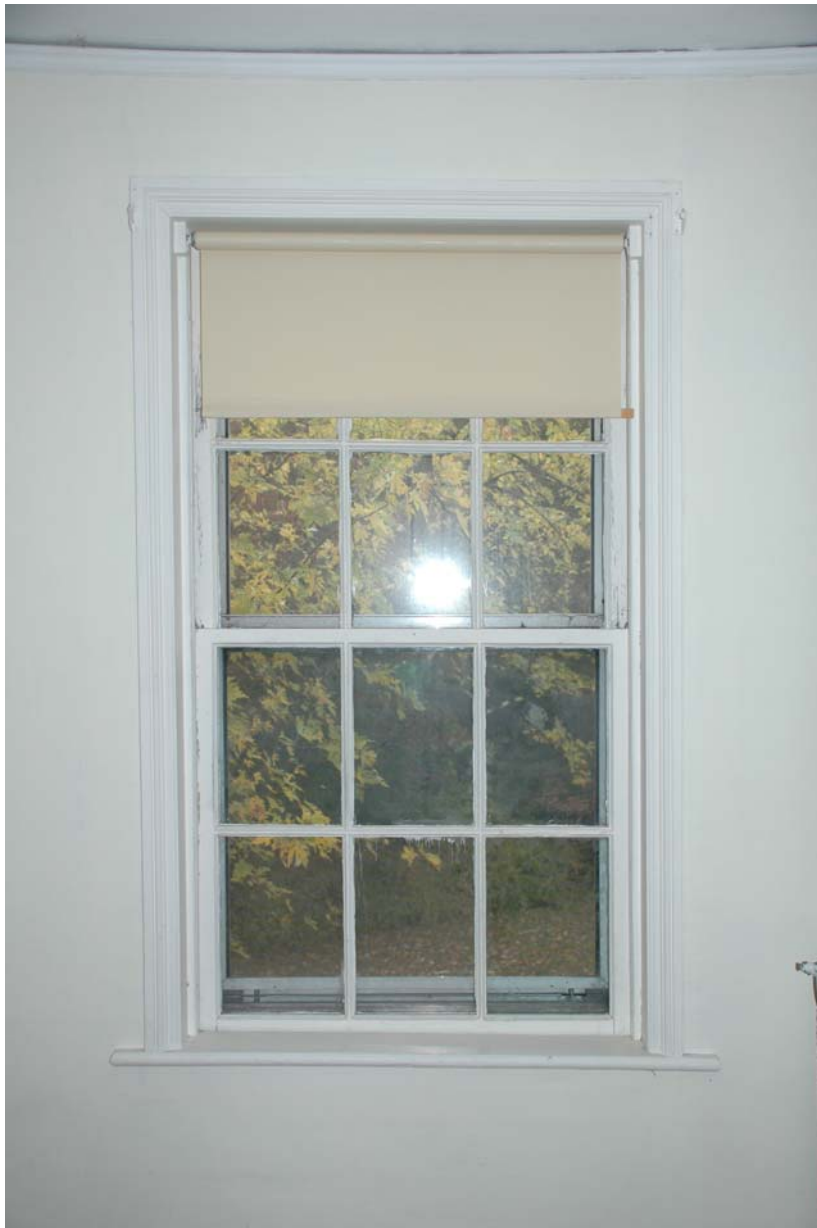
Figure 207-6. Window 216 on the north wall of Room 207.
