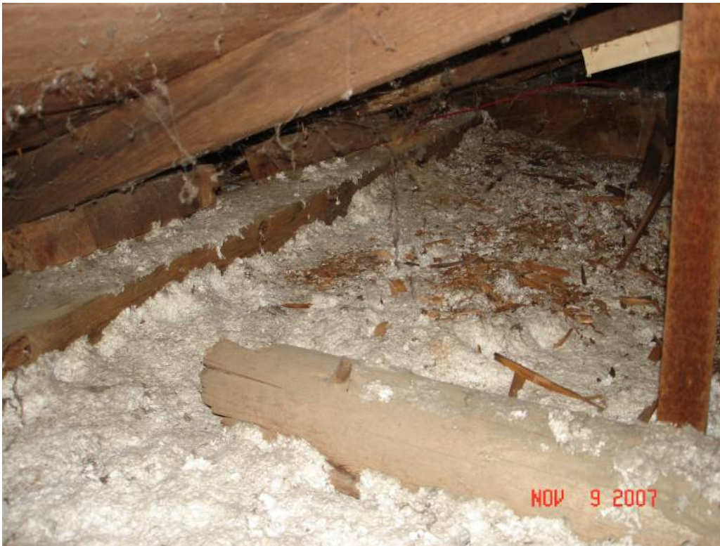
Figure S-3. Half-round joists for ceiling support.
