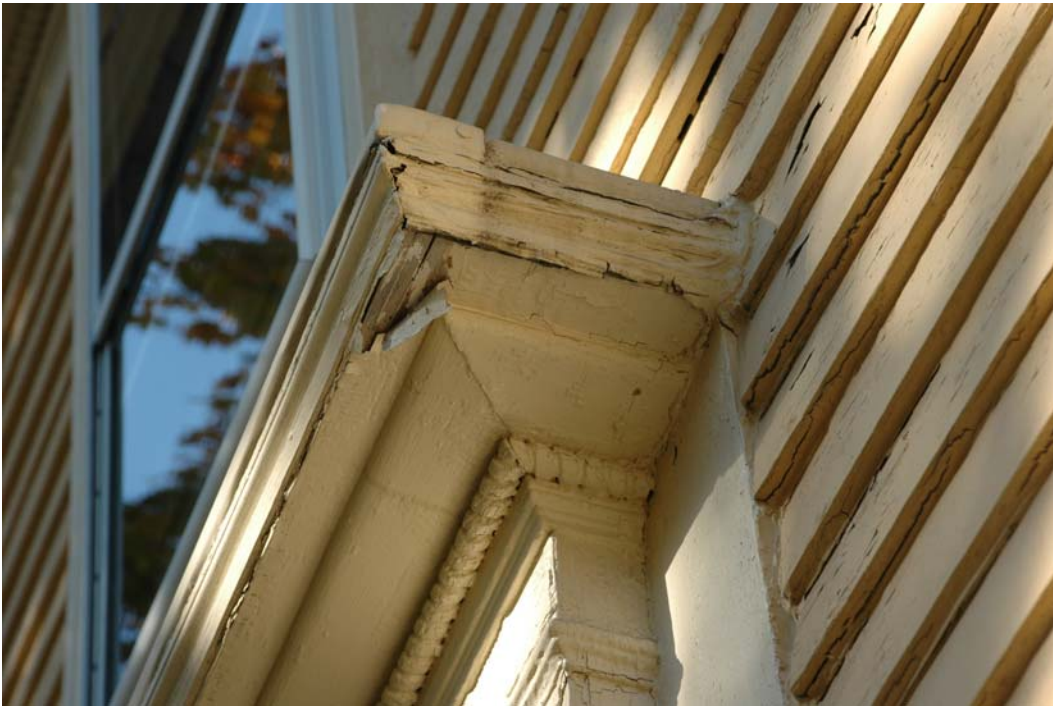
Figure SE-12. Door 1/101: detail of door surround cornice showing condition. Note unique decorative spiral rope molding, also found along the main block roof cornice.
