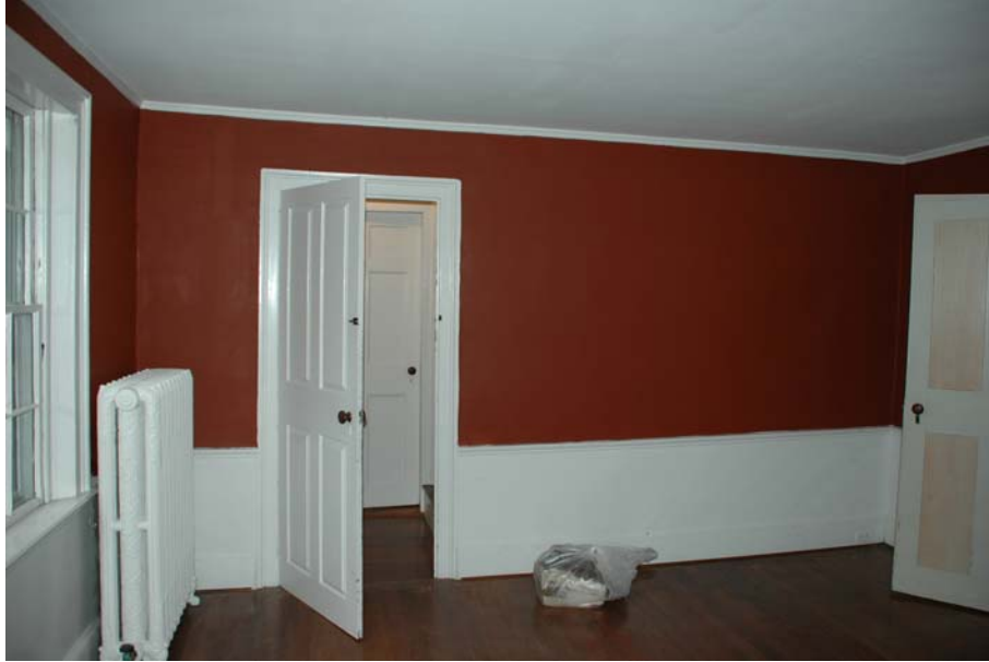
Figure 103-4. West elevation of Room 103 with Door 1/103 leading to Room 101.
