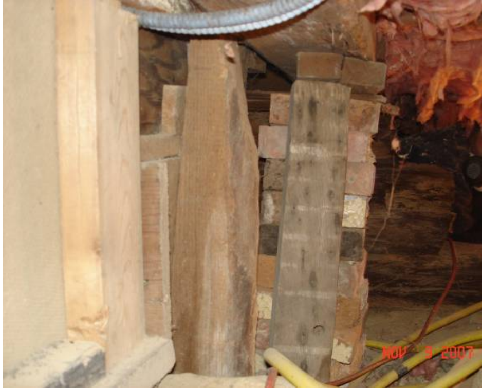
Figure S-5. Shoring of first floor beam.
