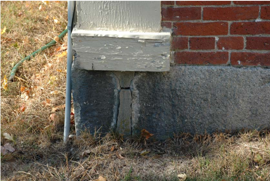
Figure EE-4. Foundation wall at east elevation of main block, with deteriorated corner board and chipped and cracked concrete mortar at foundation wall.
