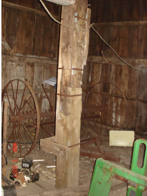
Figure BS-2. Typical barn post.
