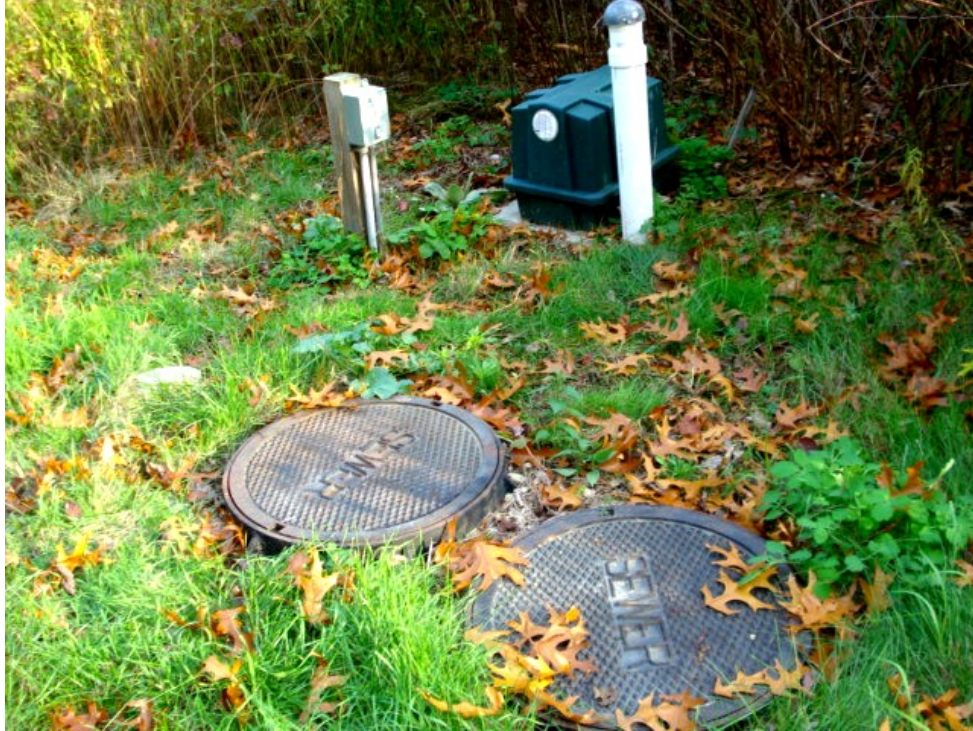
Figure P-6. Sewage Lift Station
