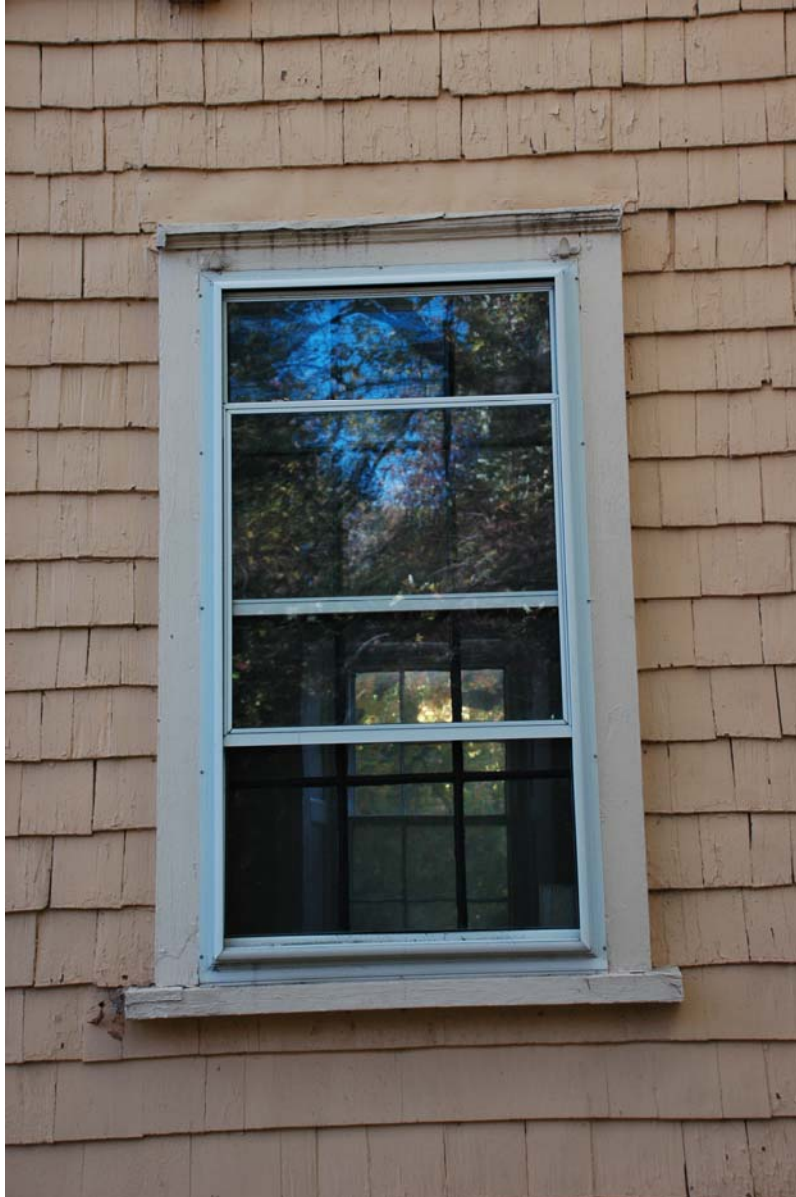
Figure NE-17. Window #115, Type w-A. Lower left portions of frame and sill are rotted and flashed with metal.
