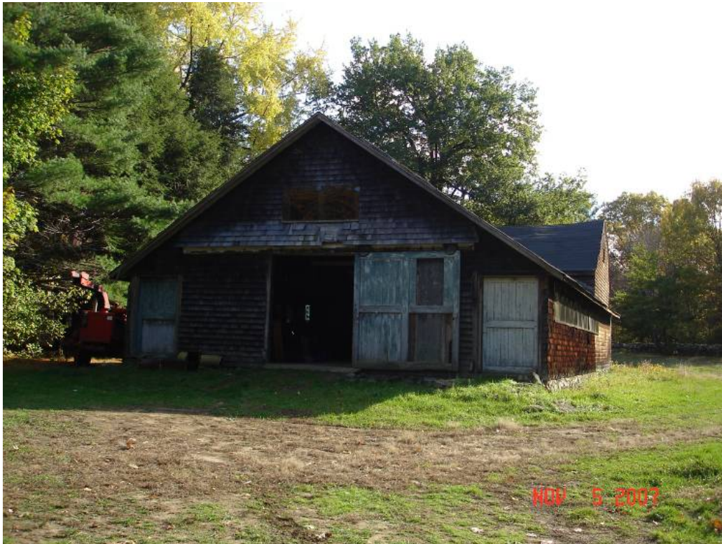
Figure BS-14. North end of north block
