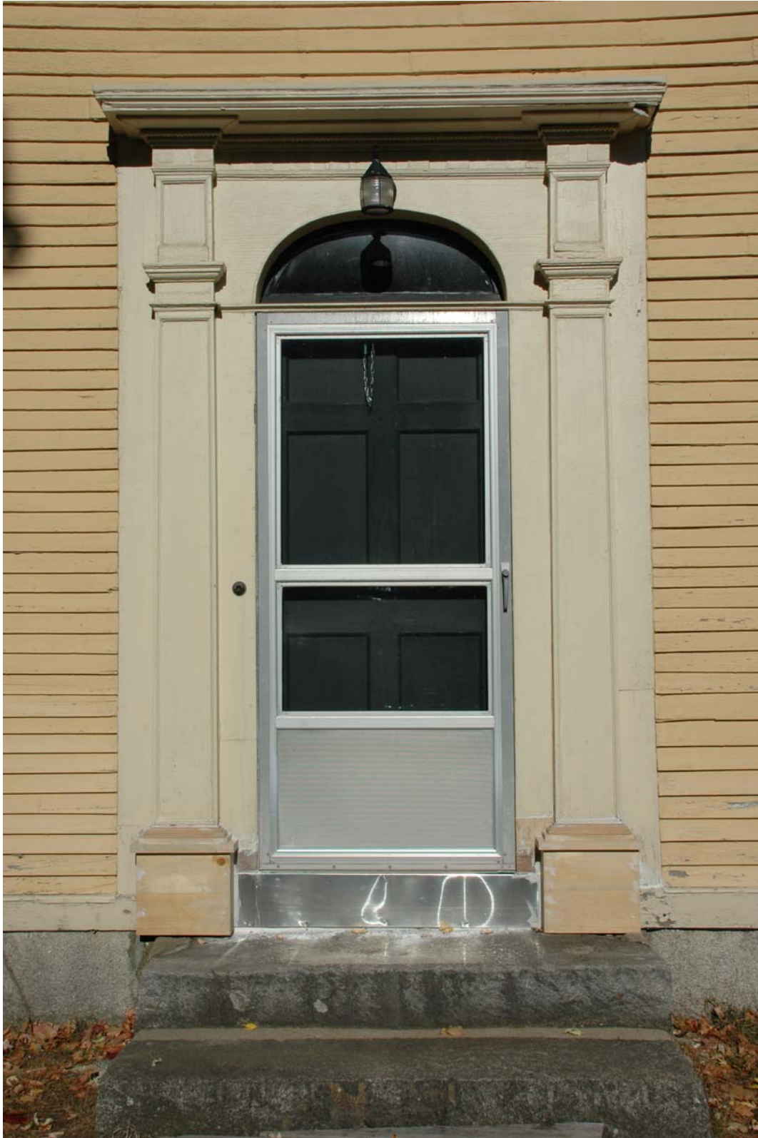
Figure SE-10. Door 1/101 - entrance to the main block. The rotted sill and pilaster bases were replaced by the NPS in October, 2007.
