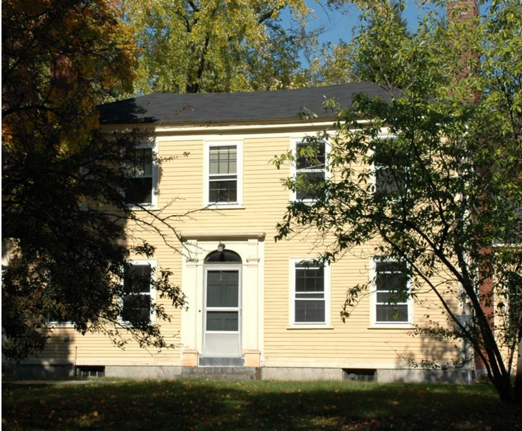
Figure SE-4. South Elevation of main block.
