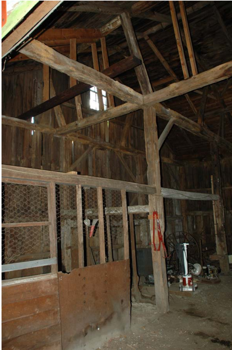
Figure B101-3. Room B-101, looking southeast.
