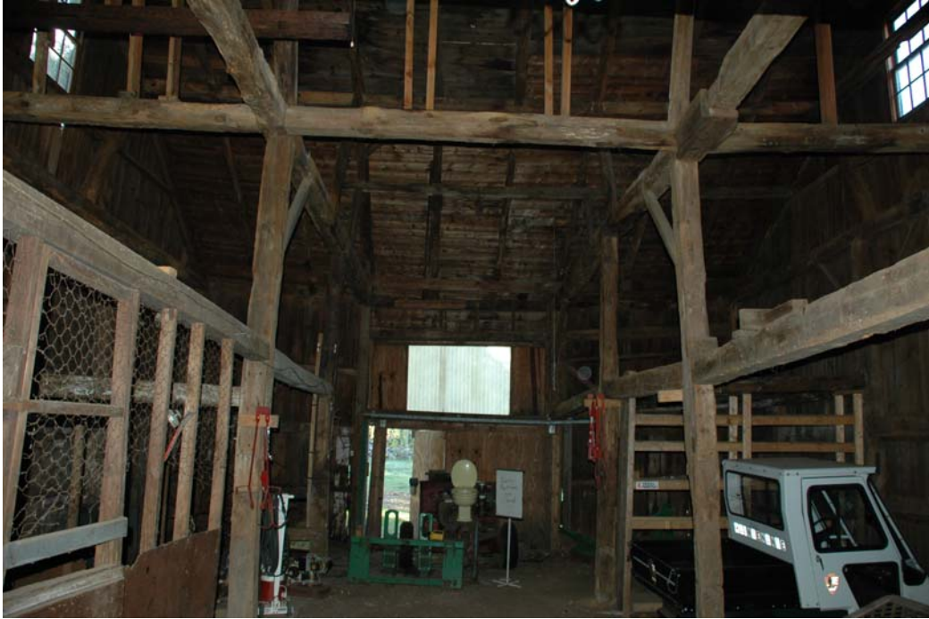
Figure B101-1. Room B-101, looking south. The original barn door opening is infilled with plywood and a corrugated fiberglass panel.
