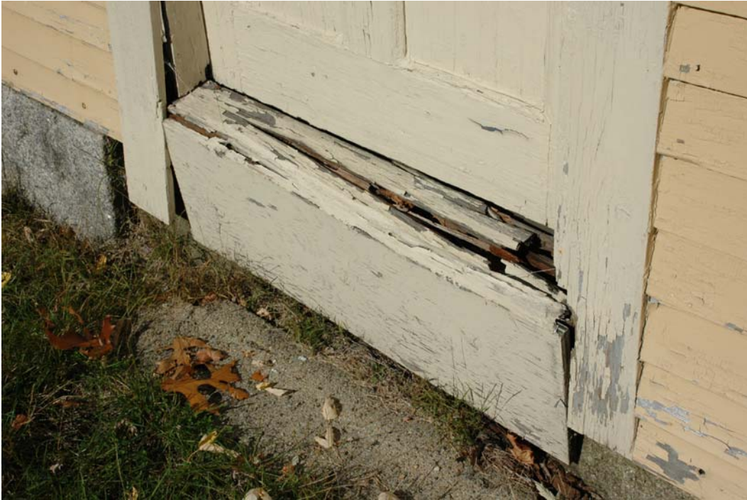
Figure SE-14. Door 1/109: detail of rotted and warped sill.
