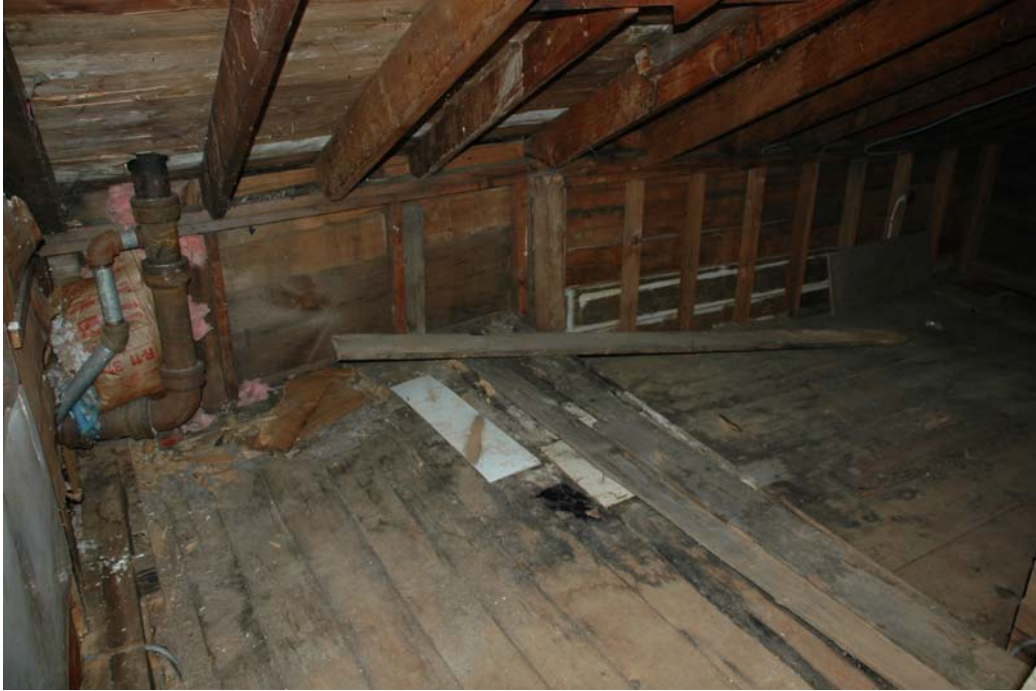
Figure 209-2. Room 209, looking north. The single existing 18 th century structure corner post, since cut down in height, is visible in the center of the wall. The area left of the post is the northwest wing above Room 107 and the area right of the post is the 18 th century block above Room 108.
