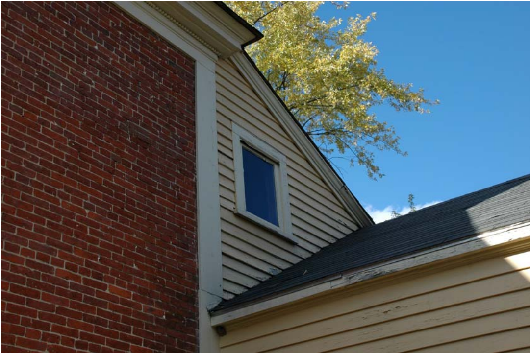
Figure EE-5. East elevation of main block and rear addition. Window #212, Type w-E. The original sash was a 3-light casement as documented in HABS photographs.
