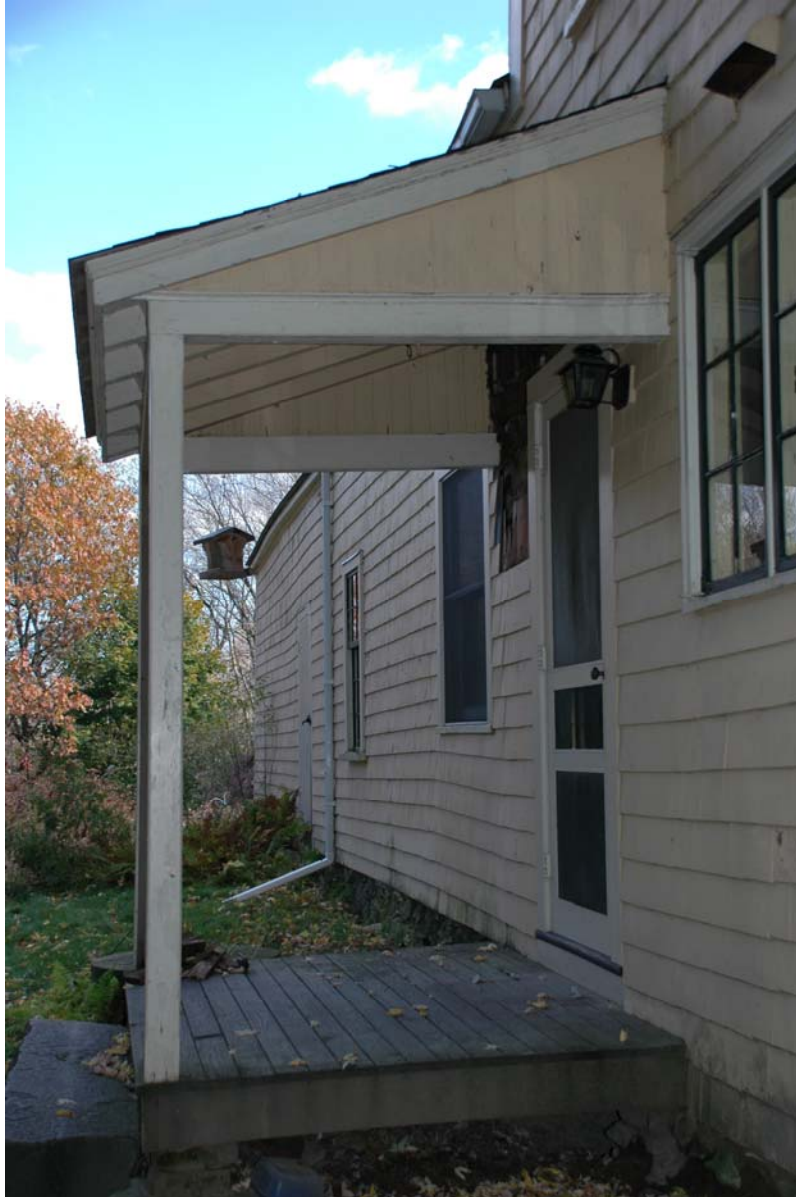
Figure NE-18. Side view of rear porch, looking east.
