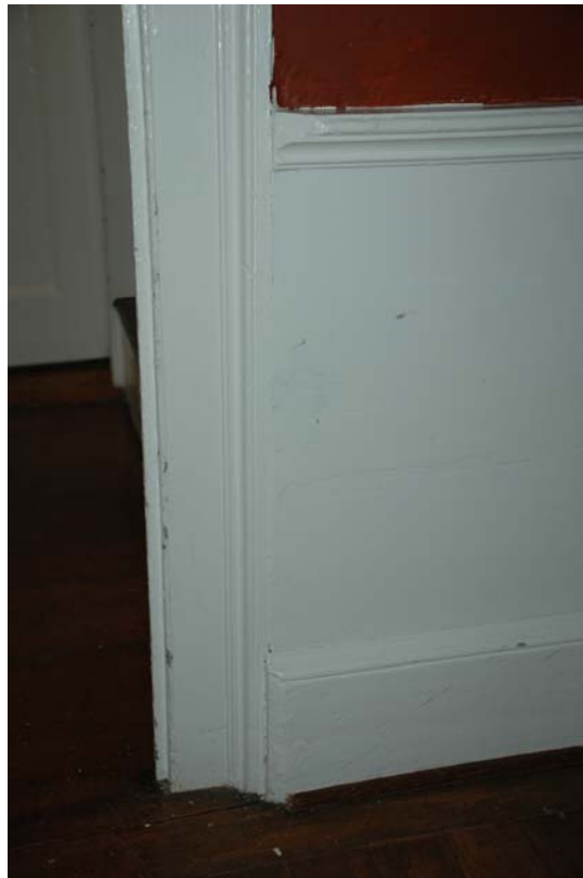
Figure 103-5. Room 103, detail of wood wainscot, chair rail, baseboard, and door casing. The chair rail and baseboard are thicker than the door casing backband and they have been cut at an angle to resolve the difference in depth.
