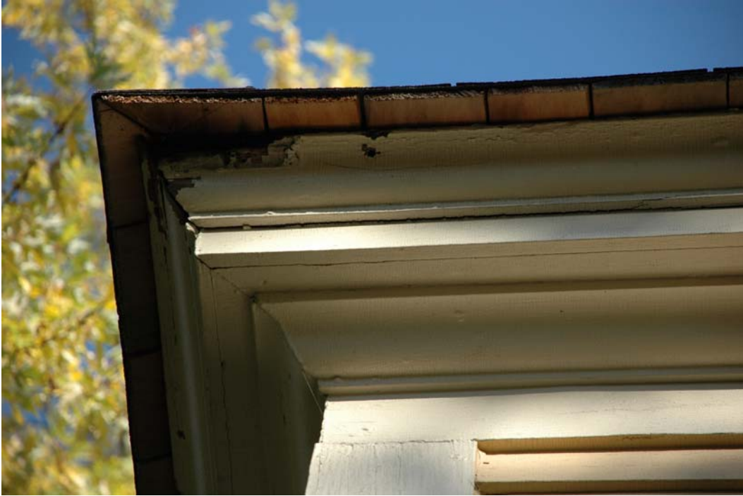
Figure SE-7. Roof cornice condition at southwest corner of northwest wing. Also note wood shingle drip course.
