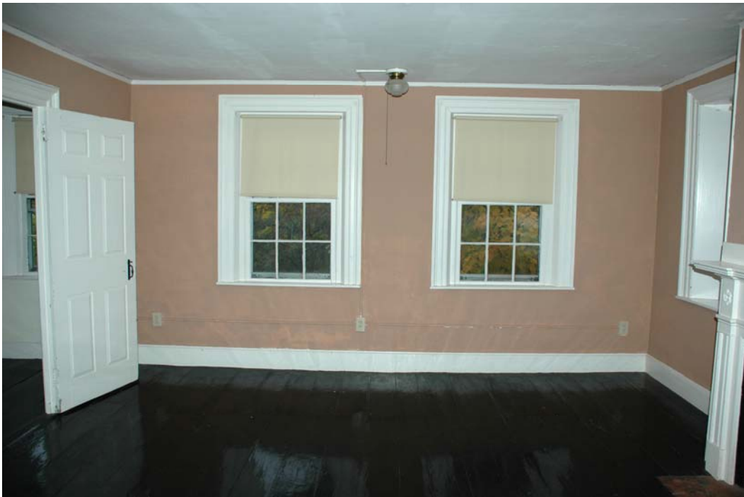
Figure 202-1. South elevation of Room 202 with Windows 207 & 206.
