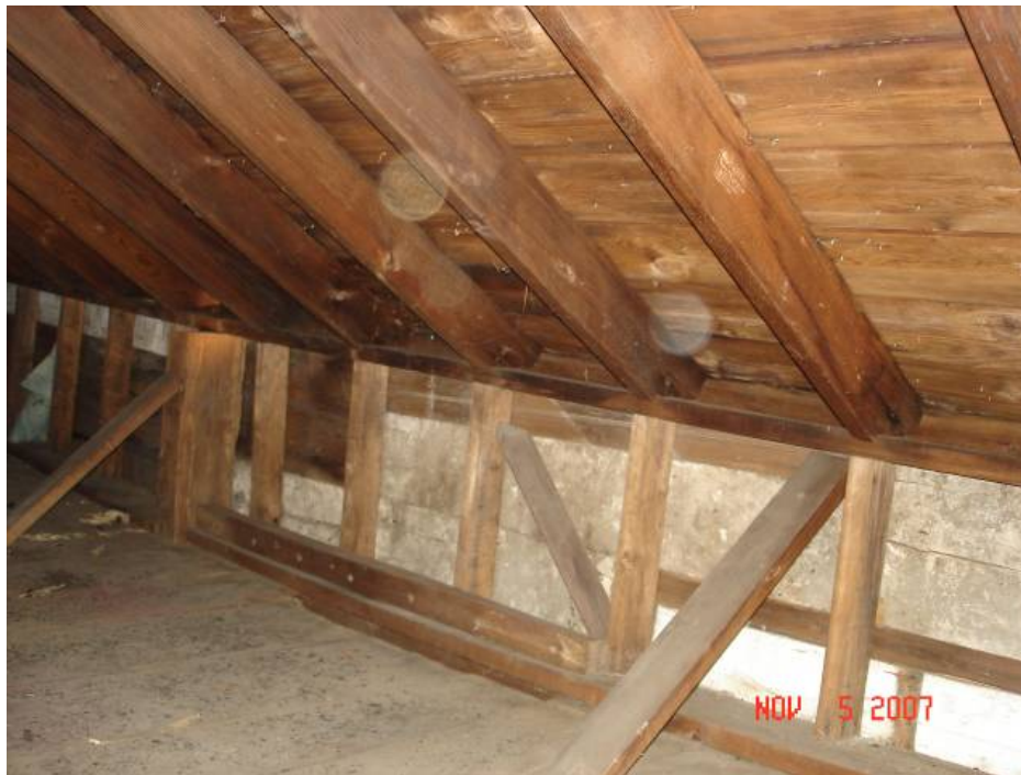
Figures S-17 & 18. Roof framing in the northeast wing.
