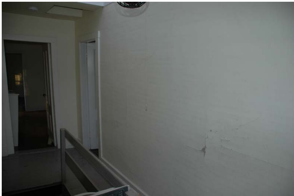
Figure 205-3. North elevation of Room 205. Door 1/207 is on the left and Door 1/206 is on the right.
