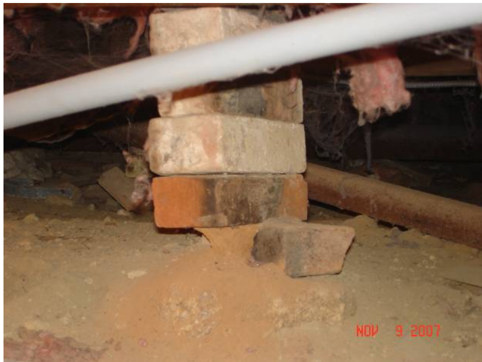
Figure S-4. Shoring of first floor beam.
