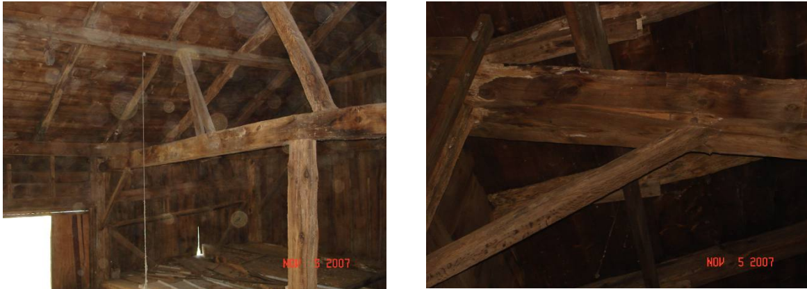
Figure BS-8. Broken tie-beam and ruptured tenon at knee brace
