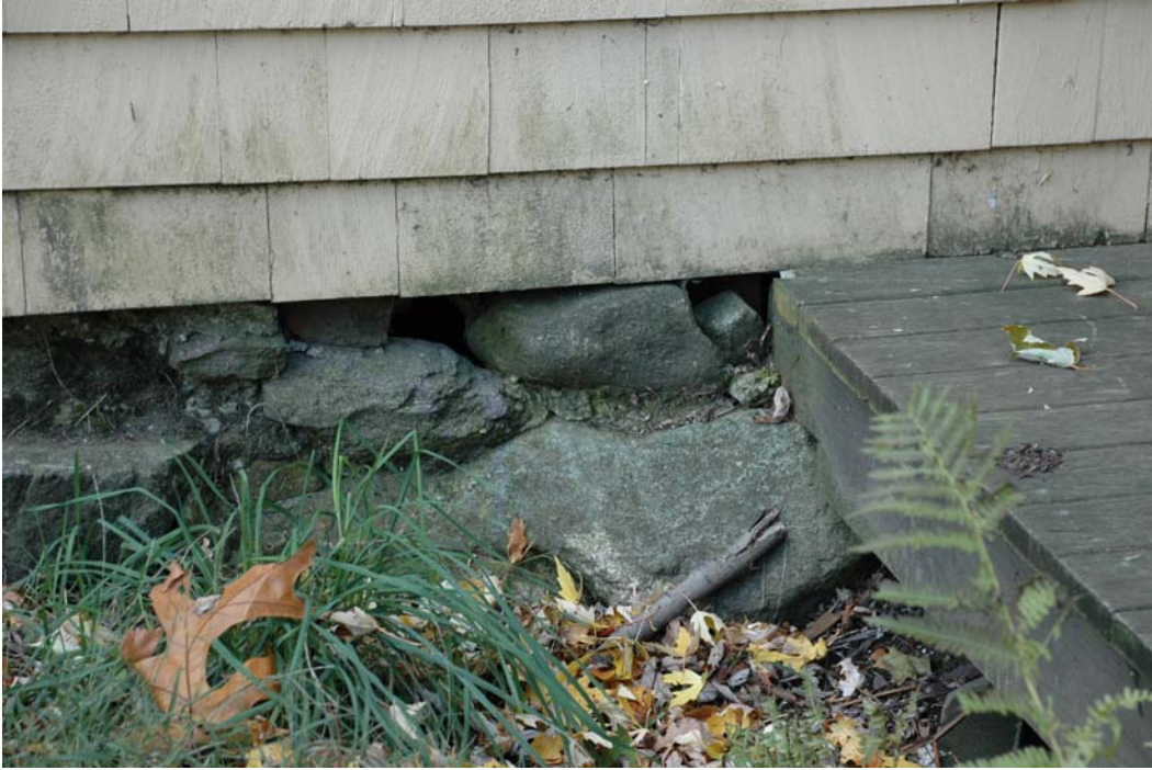
Figure NE-6. Foundation wall near rear porch with areas of missing foundation stones.
