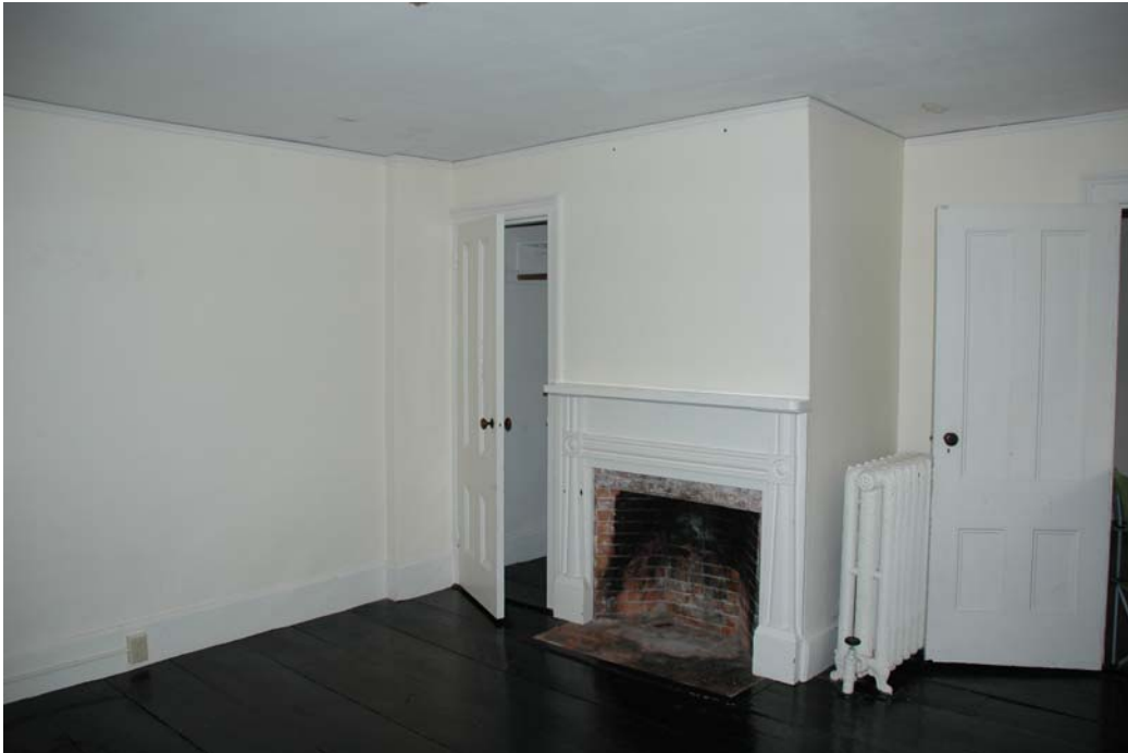
Figure 208-1. Northeast corner of Room 208 with Door 2/208 leading to a closet. The northeast corner is boxed out, possibly concealing a post.
