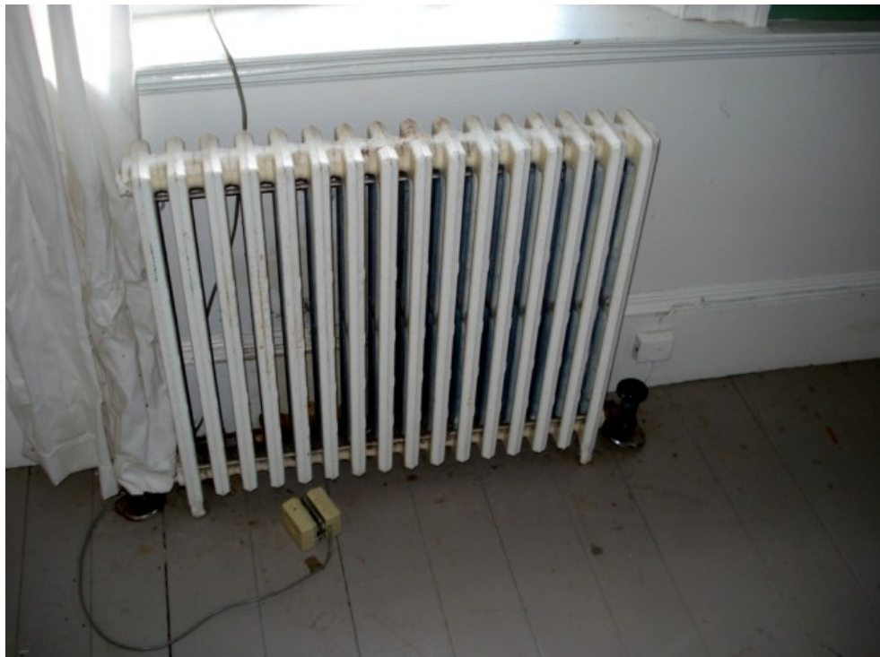
Figure H-5. Typical cast iron radiator.
