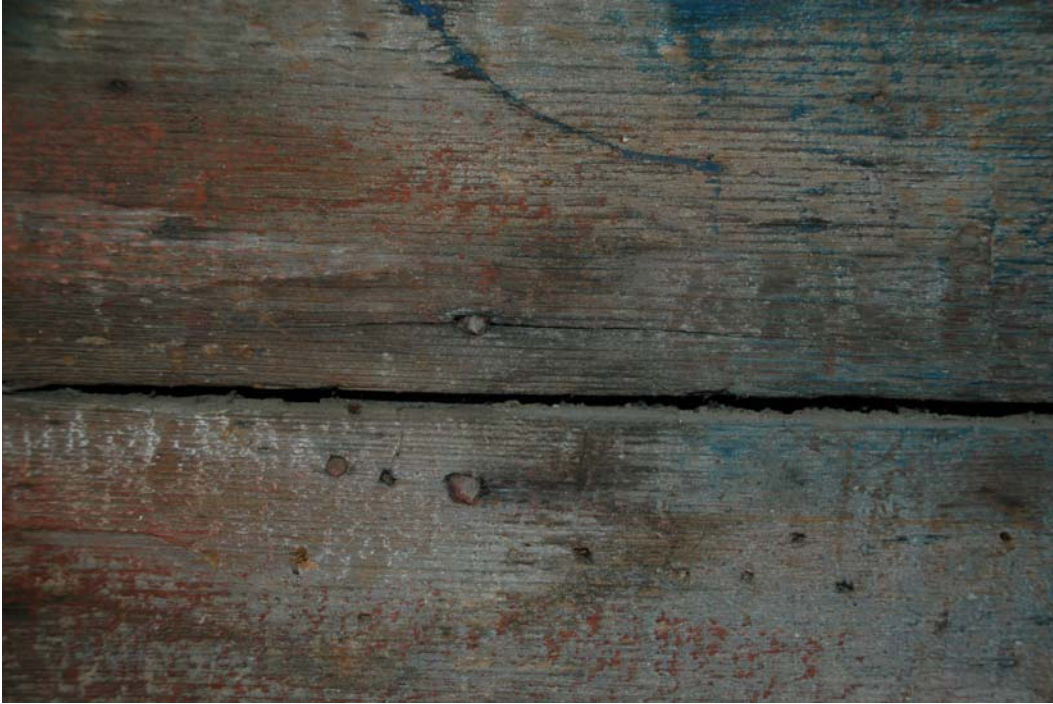
Figure 1.3A-40. Horizontal board wall with hand-wrought and machine-cut nails.
