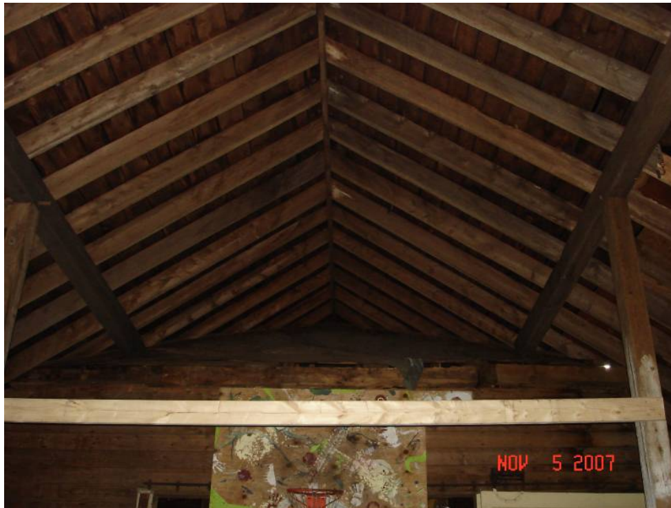
Figure BS-17. North block roof extension over south block roof.
