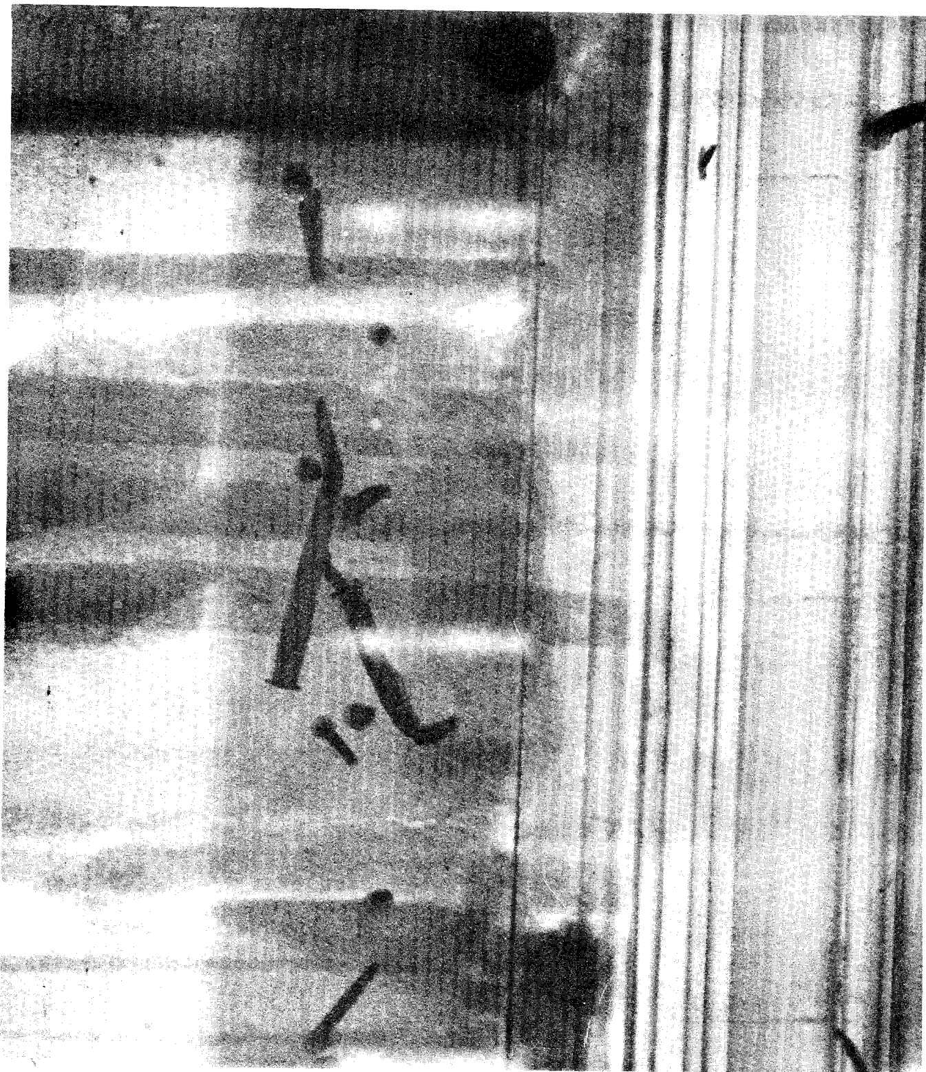
MAVA 01 X010 Room 207, door 202, north jamb, looking east 2'10" above the floor.
