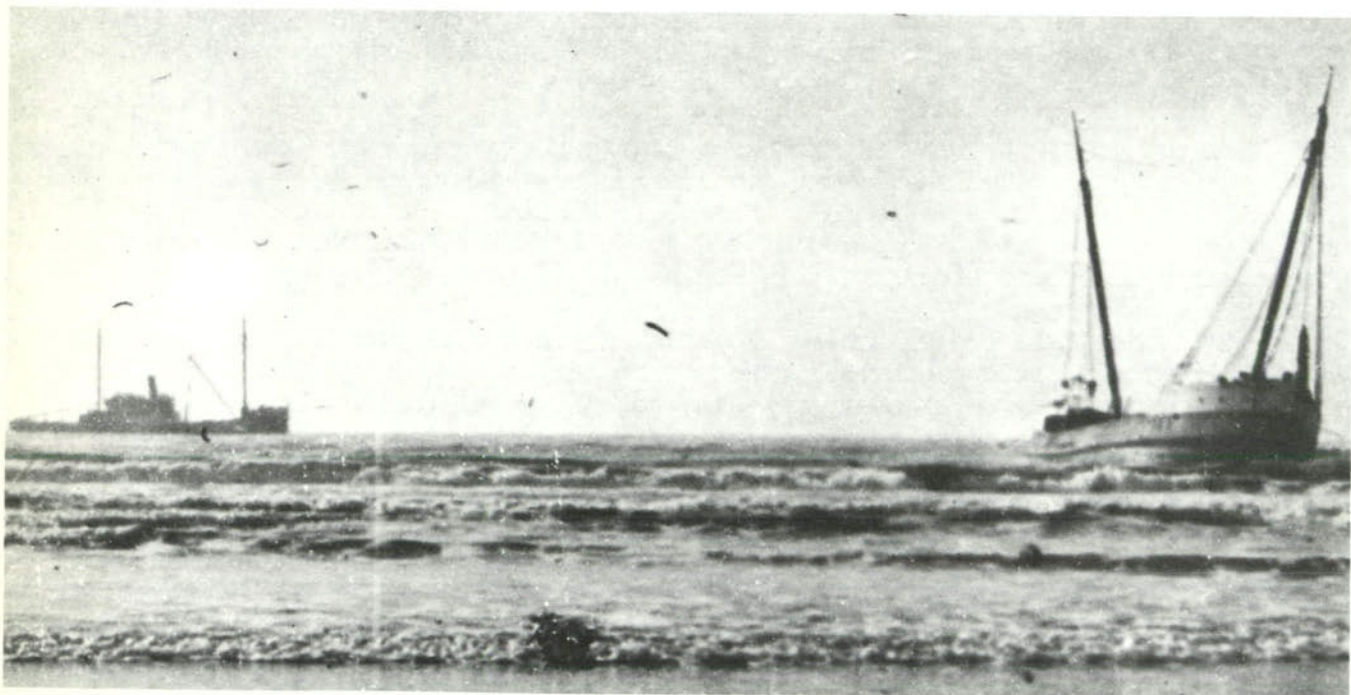
Plate 3. Another view of the Iaquia attempting to salvage Pomo . Note the serious sag in Pomo 's hull and the skewed angle of her masts, both indications of serious damage. Photograph by Clara Marshall, National Maritime Museum, San Francisco.
