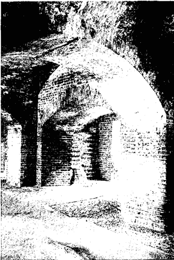
Plate 8.5. Example of second tier brickwork in casemate. NPS photo by Randy Jonsson.
