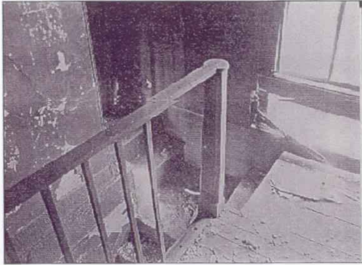
WPTC Pre-Investigation photograph showing stair rail detail.
