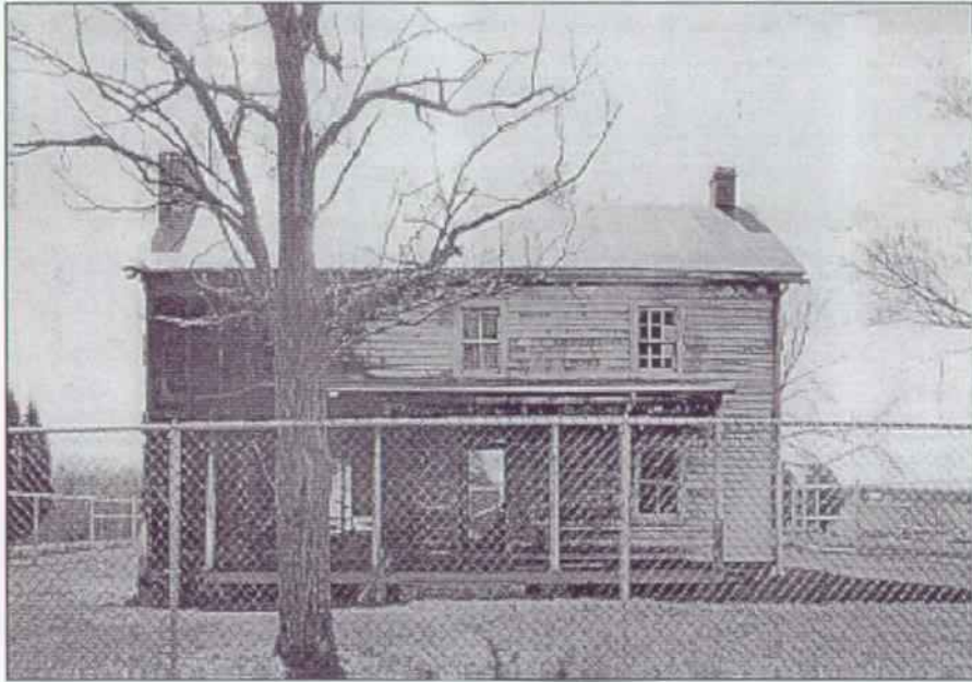
Photograph of the north elevation prior to work.
