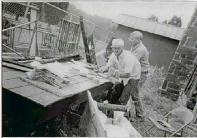
WPTC Photograph #19- cataloging architectural artifacts.
