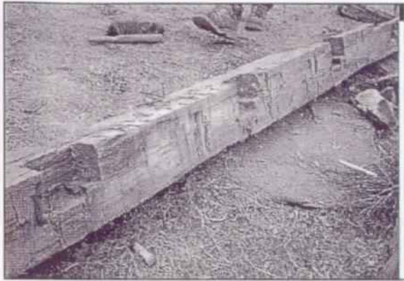
WPTC photographs # 82 (left) and #83 (right), showing sill joinery details.
