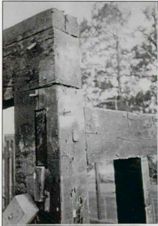
WPTC photograph #55, showing unused mortise pockets.
