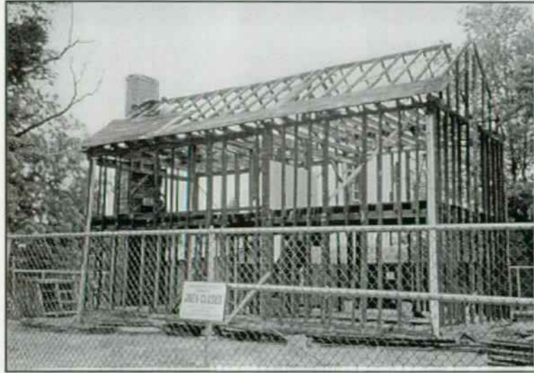
WPTC photograph #56 - view of exposed framing system.
