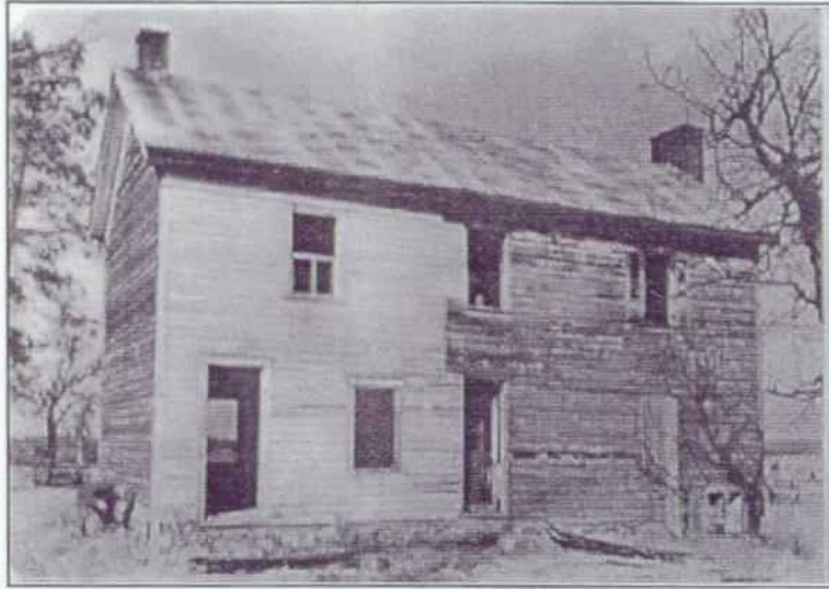
Sheffield photograph #3 / WPTC photograph #95 - north elevation.
