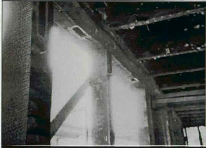
WPTC photograph #55, showing unused mortise pockets.
