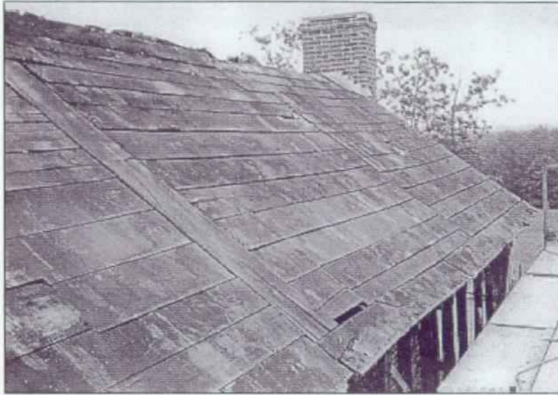
WPTC Photograph #40 showing roof sheathing.
