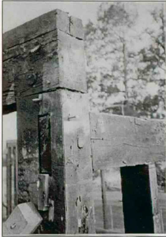
WPTC Photograph #67 showing corner post and top plate detail .
