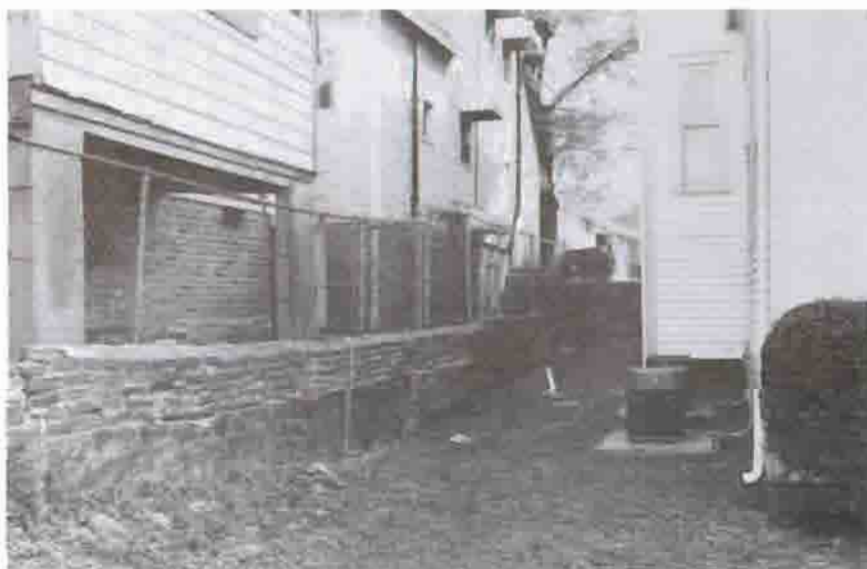
Fig. 11. Typical existing sideyard along the north side of Auburn Avenue. Note wall and steps in background (front corners of 530 and 526 Auburn Avenue), 1994.
