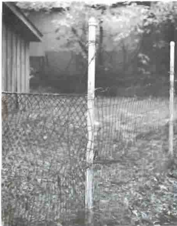
Rolled wire fence at 497 Auburn Avenue.
