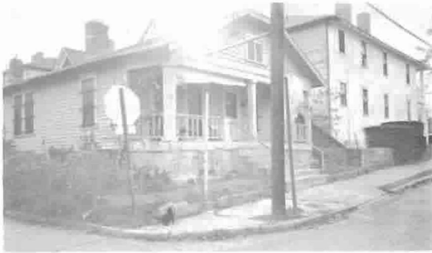
53 Hogue Street. Note rolled wire fence across front yard.
