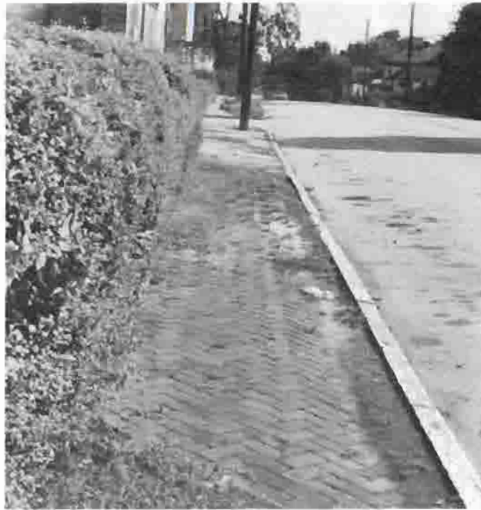
Fig. 7. Existing brick sidewalk on the northwest intersection of Auburn Avenue and Howell Street.
