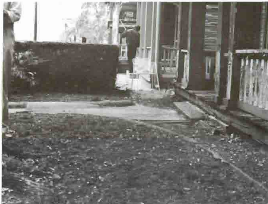
Fig. 10. Historic walk and gutter at 518 Auburn Avenue, 1995.
