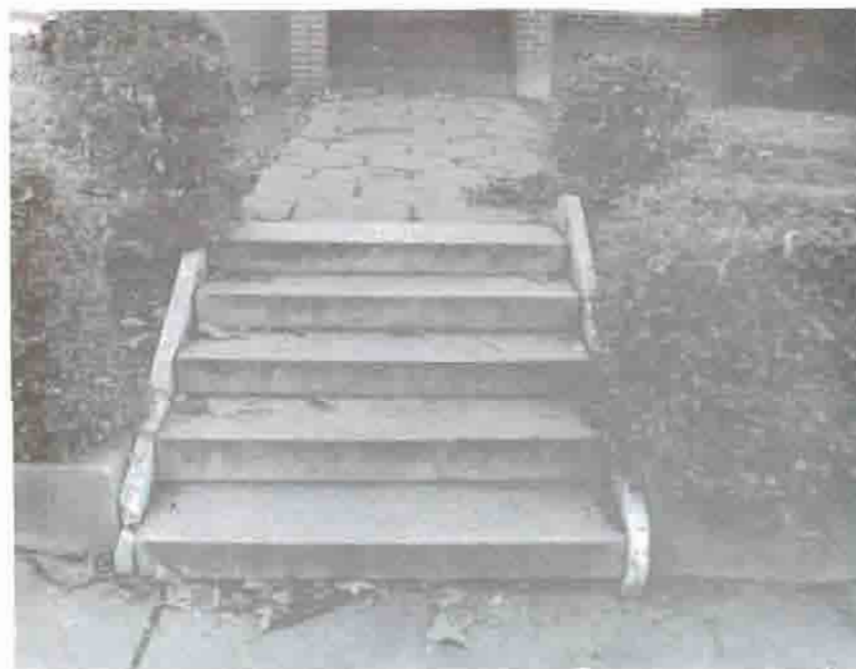
Fig. 51. Detail of front steps at 503 Auburn Avenue, 1995.
