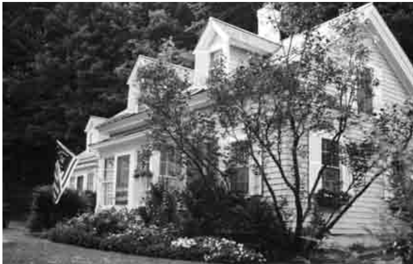
Figure 4.37: Double Cottage foundation shrubs, view northwest showing herbaceous beds (V-37), September 2001. SUNY ESF.
