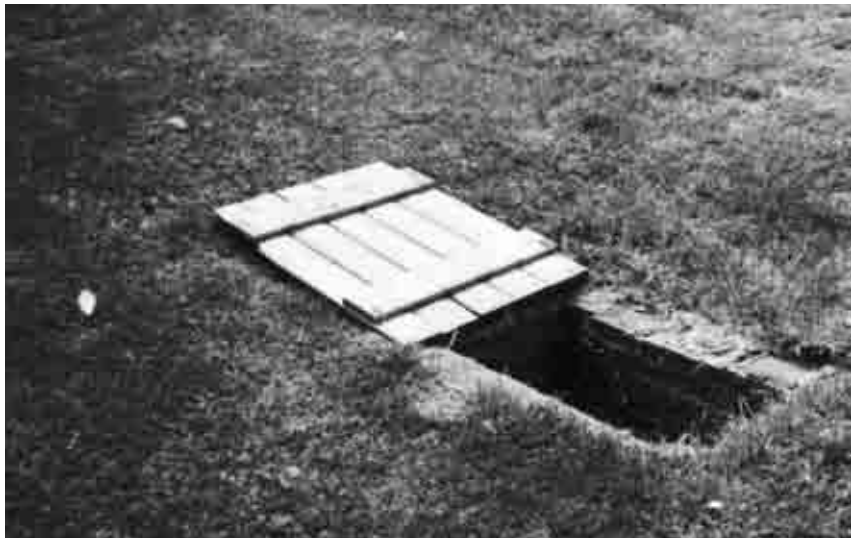
Figure 4.52: Pogue-line valve pit, view west of small one north of the Carriage Barn, September 2001. SUNY ESF.
