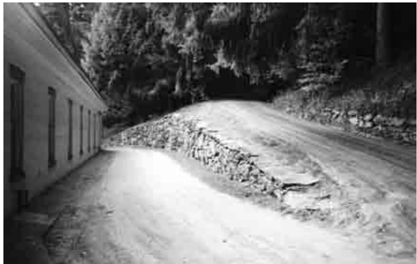
Figure 4.51: Belvedere drive retaining wall, view west with the Bowling Alley (BS-16) to the left and the Upper Meadow road (C-20) to the right, September 2001. SUNY ESF.
