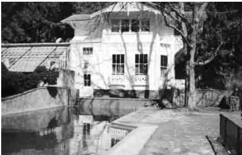
Figure 5.25: The Belvedere, view north with the swimming pool (CWF-1) in the foreground bordered by the pool patio brick walls and barbecue (BS-20), April 2002. SUNY ESF.
