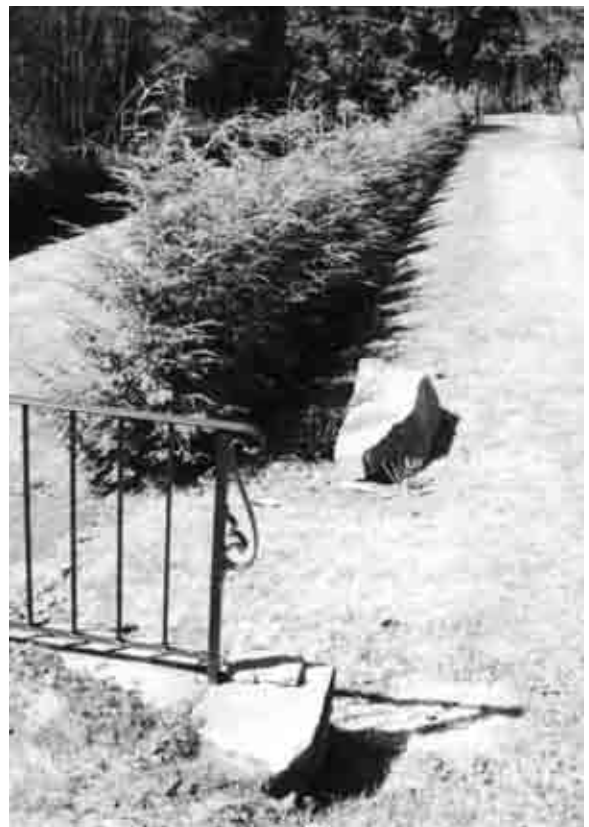
Figure 5.33: Swimming pool terrace railing, detail view of west end, with upper Long Terrace perimeter hedge (V-49) in the background, April 2002. SUNY ESF.
