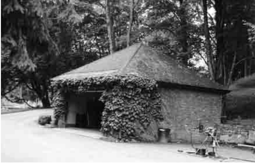
Figure 4.47: The Mansion garage, view southwest, July 2002. SUNY ESF.
