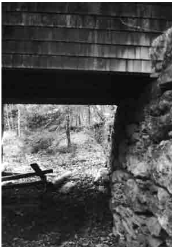
Figure 6.44: Woodshed yard retaining wall, view east beneath the Woodshed along Woodshed access road trace (A5-1), October 2000. SUNY ESF.
