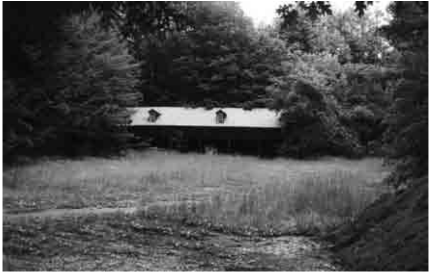
Figure 6.4: Woodshed yard, view west from eastern end to Woodshed (BS-24), July 2002. SUNY ESF. The trace of the lower Woodshed road (C-23) is visible in the foreground..
