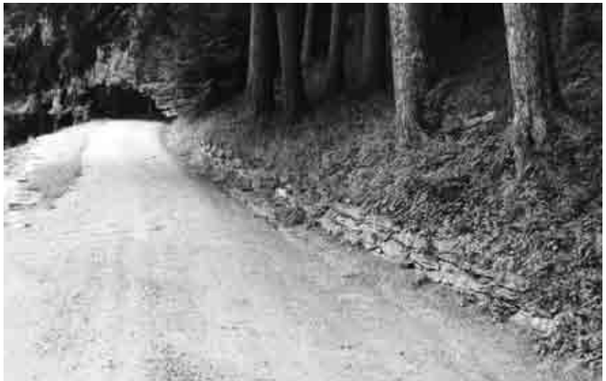
Figure 6.43: Upper Meadow road retaining wall, view west from intersection with Belvedere drive, July 2002. SUNY ESF.
