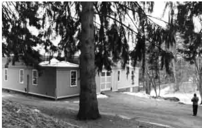
Figure 4.13: The Carriage Barn, view east of entrance and drive prior to construction of walkway, winter 1997. Olmsted Center for Landscape Preservation.
