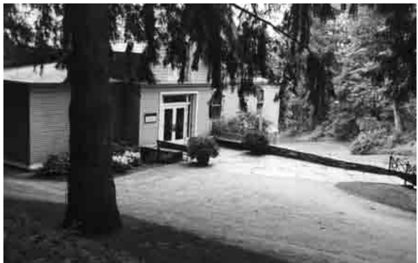
Figure 4.14: The Carriage Barn walkway, view east of stone patio and wall added in 1998–1999, with new beds (V-37) visible along building, July 2002. SUNY ESF.
