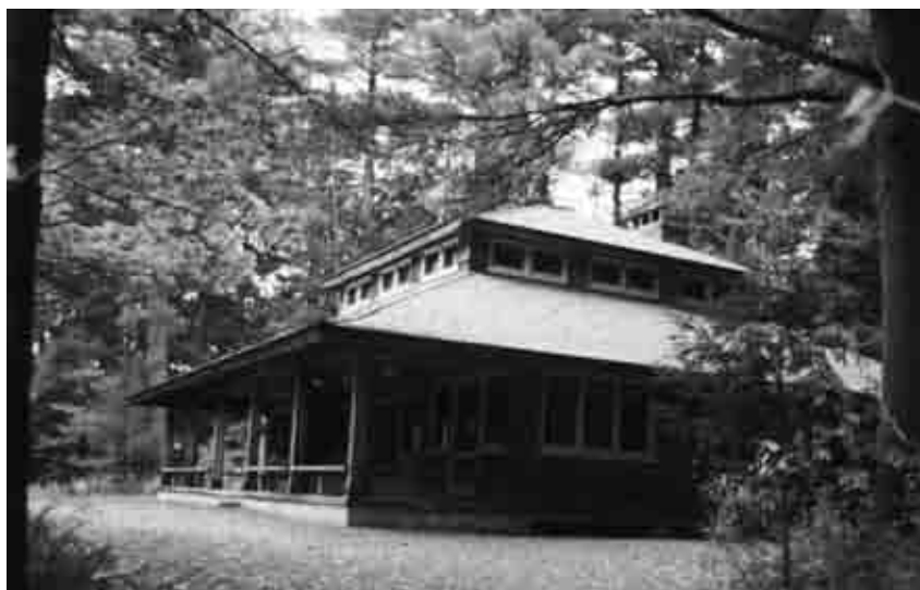
Figure 6.40: The Bungalow, view southeast of front (north side) of building and surrounding white pine plantation, October 2000. SUNY ESF.
