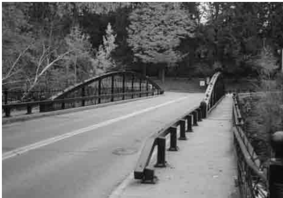
Figure 1.6: The Elm Street Bridge, view north with mature Norway spruce along the perimeter of the Mansion grounds in the background, October 2001. SUNY ESF.
