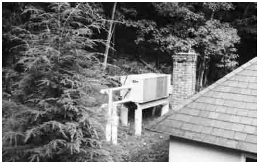
Figure 4.65: Carriage Barn remote air-conditioning unit, view northwest with the Generator Garage to the right, September 2001. SUNY ESF.
