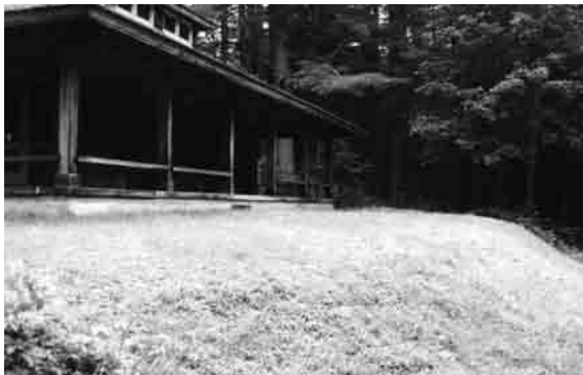
Figure 6.29: Bungalow terrace, view west along north front of the Bungalow, July 2002. SUNY ESF.
