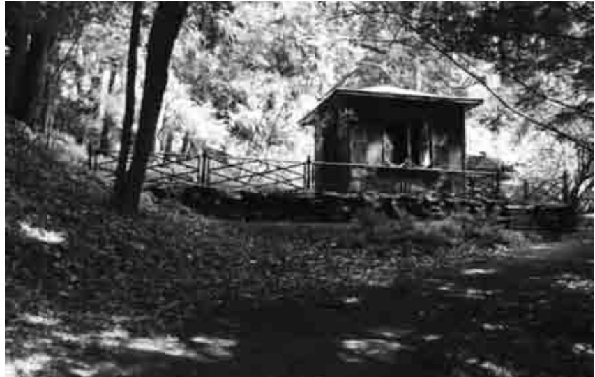
Figure 4.12: The Summerhouses path, view north toward Upper Summerhouse with its stone wall (BS-12) and iron fence (SSF-2), August 2001. SUNY
