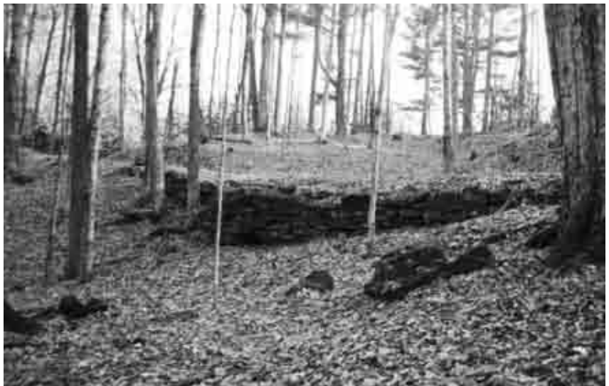
Figure 6.42: Old mountain road retaining wall, view southeast toward Upper Meadow, April 2002. SUNY ESF.
