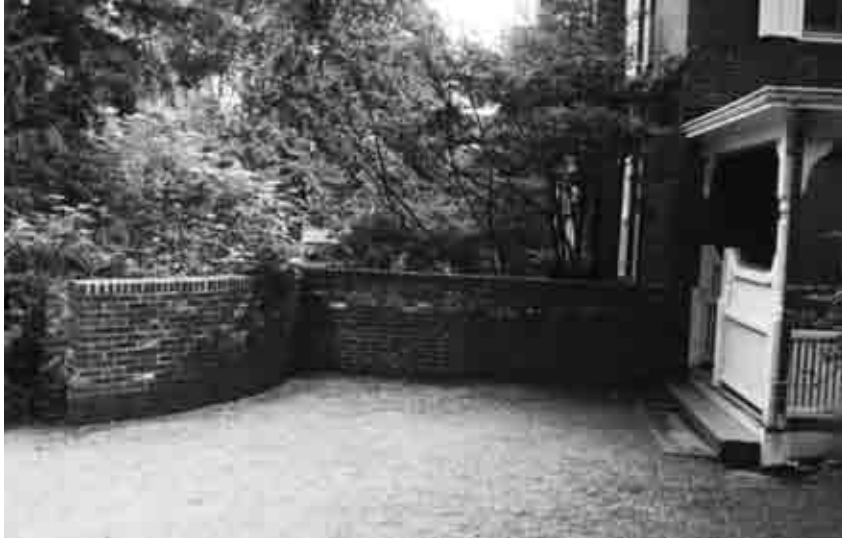
Figure 4.53: The brick retaining wall at the Mansion kitchen entrance, view east illustrating rebuilt sections and ghost of removed garbage enclosure, July 2002. SUNY ESF.
