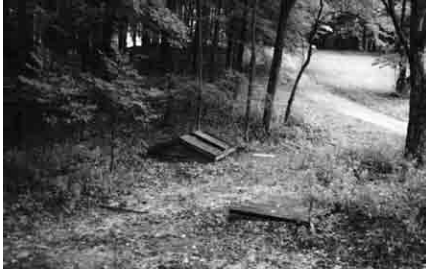
Figure 6.46: Pogue-line valve pit north of Upper Meadow (lower right structure) and Bungalow well house (BS-36, upper left structure), view east with Wood Drive in the background, September 2001. SUNY ESF.
