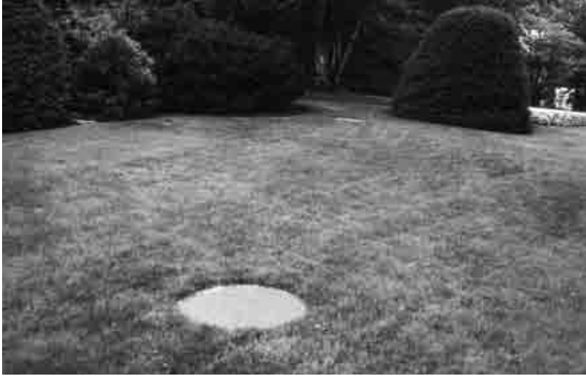
Figure 4.61: Fallout-shelter escape hatches (manholes) in the Mansion lawn, view north with the Mansion foundation shrubs at left, July 2002. SUNY ESF.
