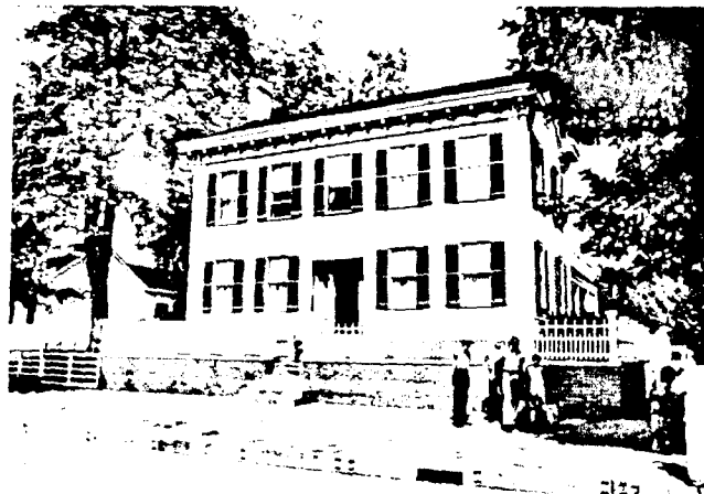
1. West Elevation (unless otherwise noted, all photographs are of the Lincoln Home, and were made in July 1979 or April 1980).
