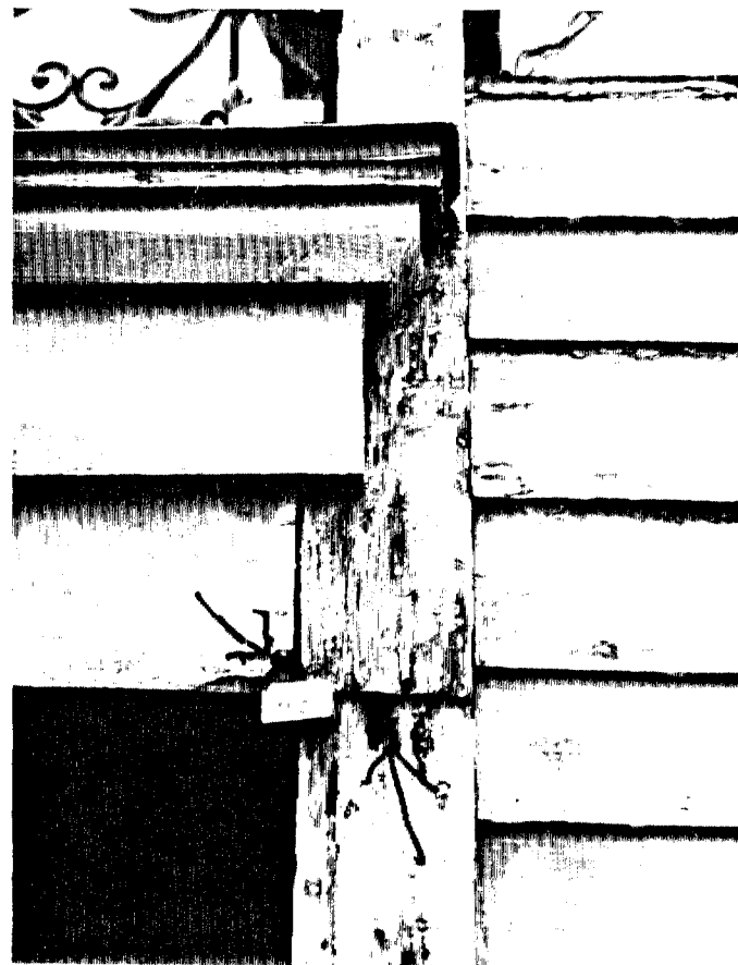
Photo showing some of the deteriorated areas in the materials trim and siding. Arrow shows these areas.
