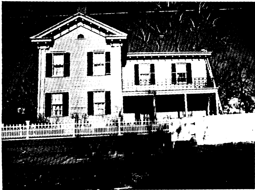
Photo showing completed paint job on south side of home.
