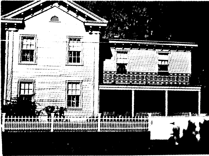
Photo showing first coat exterior wood paint, south side.
