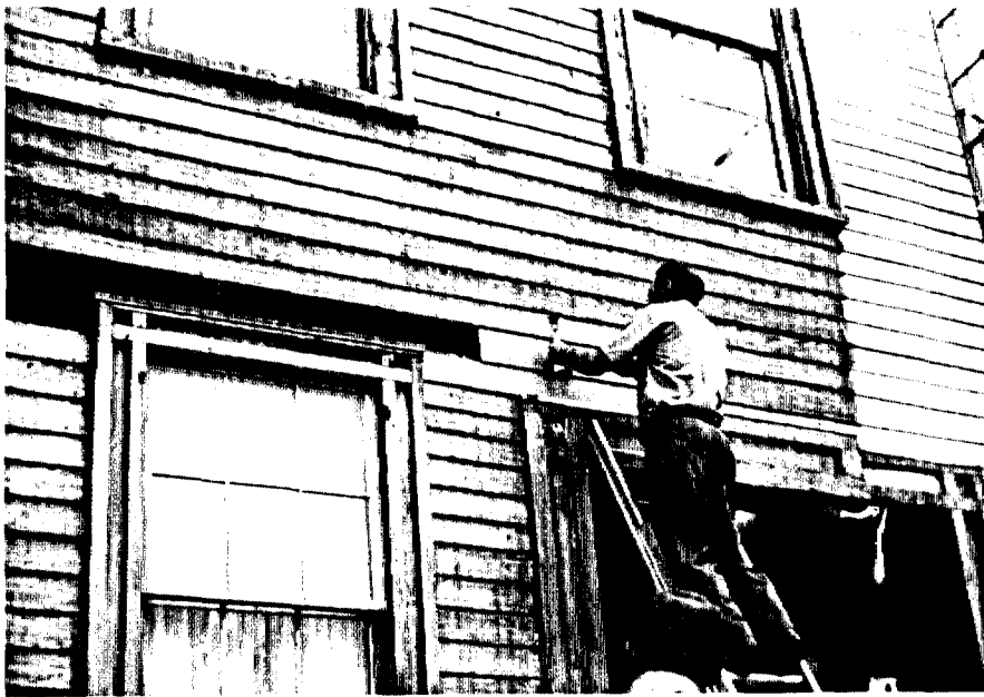
Photo showing workman replacing deteriorated siding board with nonhistoric old materials. Arrow showing board.
