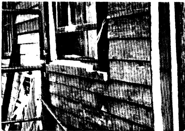
Photo showing deteriorated areas removed from sill.
