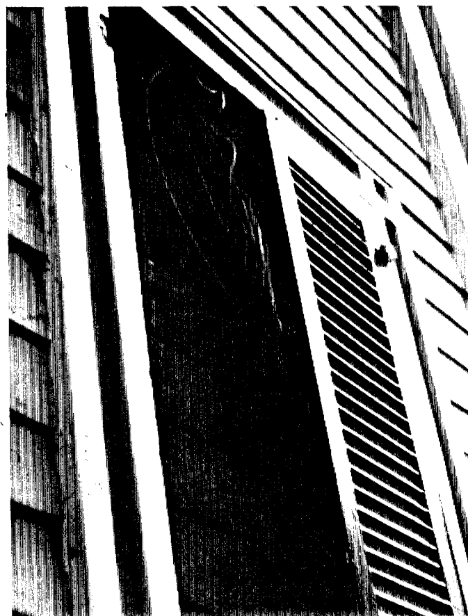
Photo showing closed-in window (boarded) by Mr. Lincoln when he added top part to house, north side of bottom floor.
