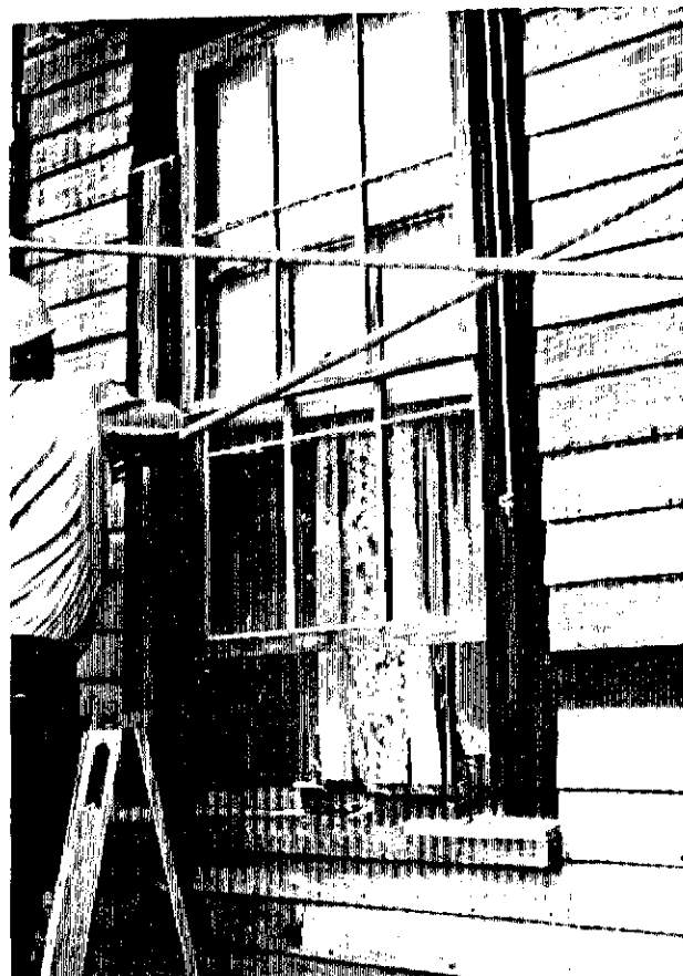
Photo showing part of deteriorated window trim cut off lower window in front, (arrow) southwest end. Also showing patched sill.
