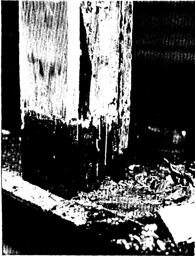
Photo showing deteriorated porch column before treatment, on south side.
