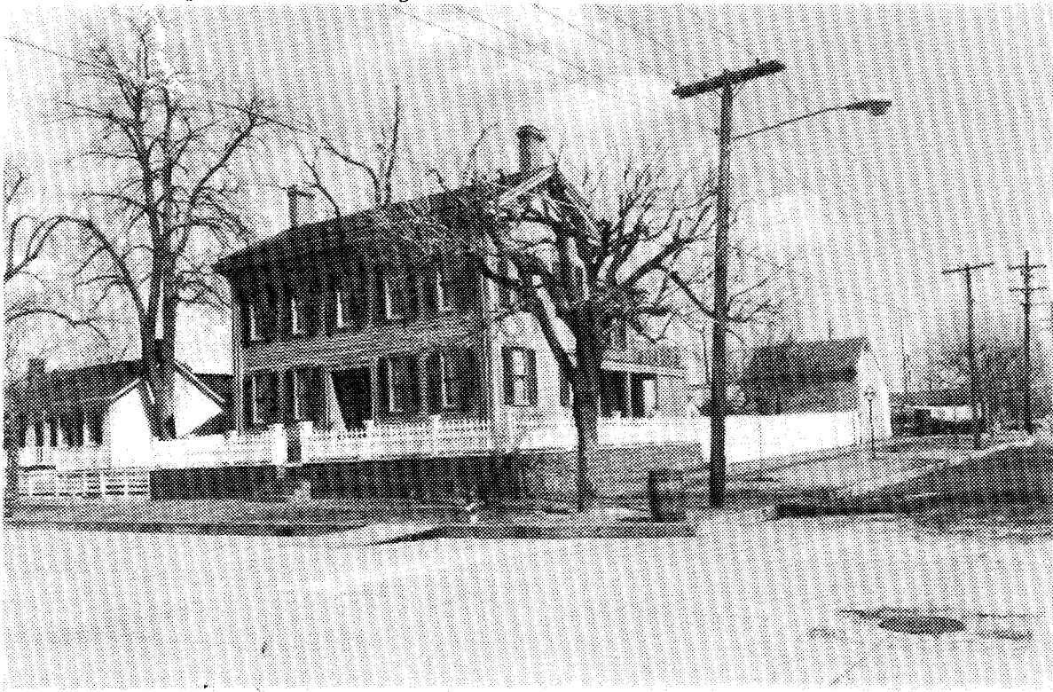
Fig. VI-26. View of Lincoln Home from the southwest showing problems caused by modern utility lines.
