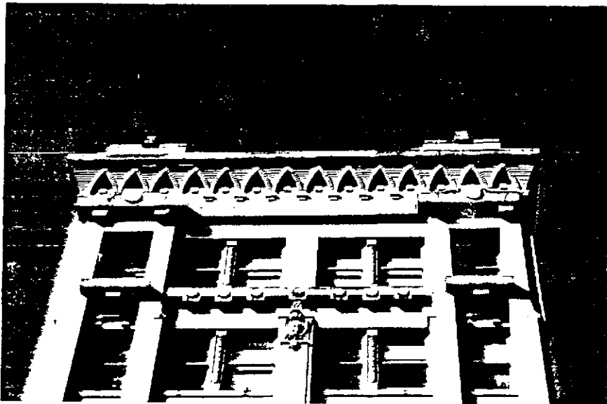
Springfield Architectural Survey (Lincoln Center Survey)
