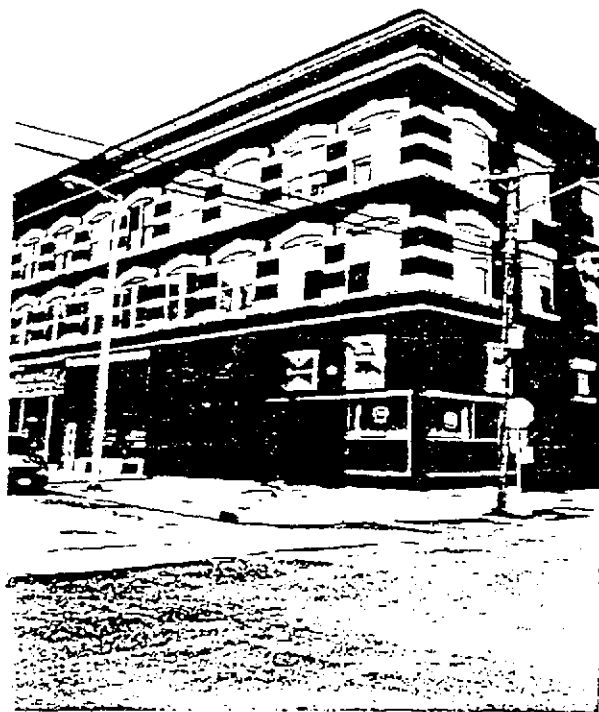
Springfield Architectural Survey (Lincoln Center Survey)
