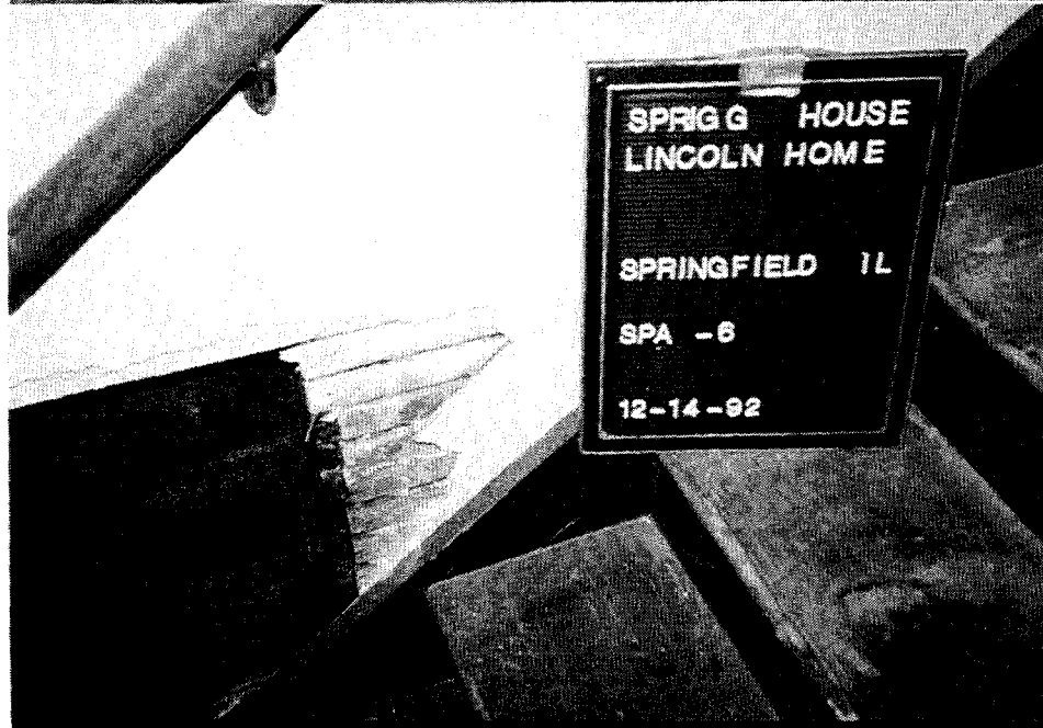
Photo SPA-6 1922 Plaster Stair S1-Wall
