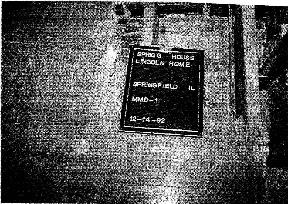
Photo MMD-1 Blown-in Insulation Room 202
