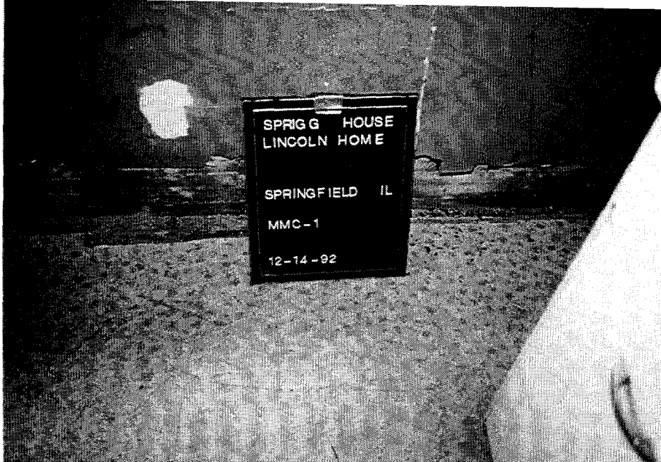
Photo MMC-1 Fibrous Wall Board Room 208
