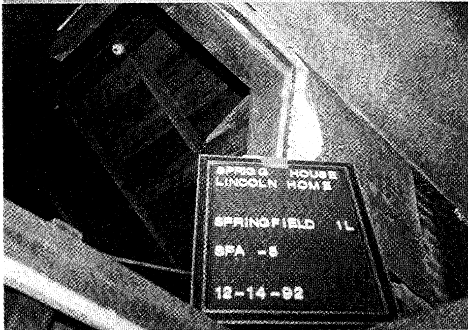
Photo SPA-5 1922 Plaster Hall 201D-Ceiling
