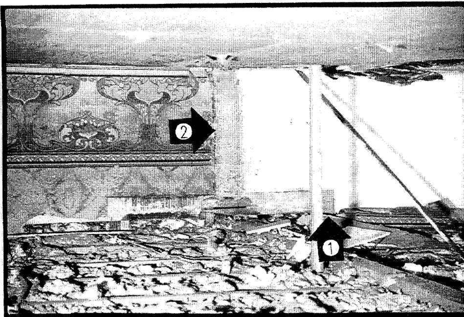
FIGURE 3.62 EVIDENCE OF WINDOW LOCATION IN THE 1874/1879 ADDITION
