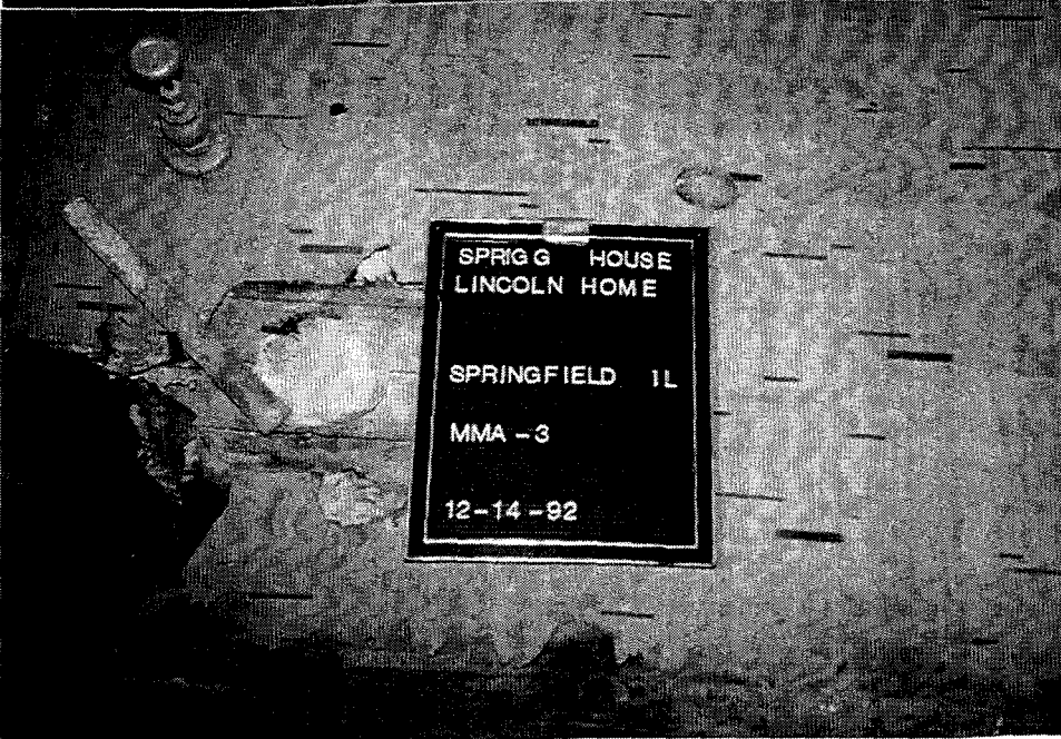
Photo MMA-3 Mastic Under Sheet Flooring Bathroom 201A
