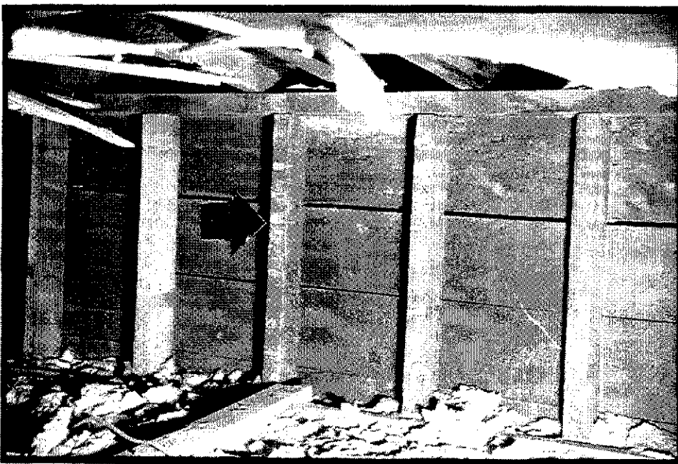
FIGURE 3.64 EVIDENCE OF CHIMNEY STACK LOCATION IN THE 1874/1879 ADDITION
