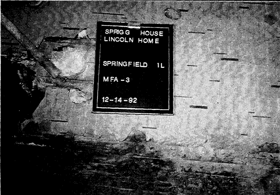
Photo MFA-3 Sheet Flooring-Linoleum Bathroom 201A
