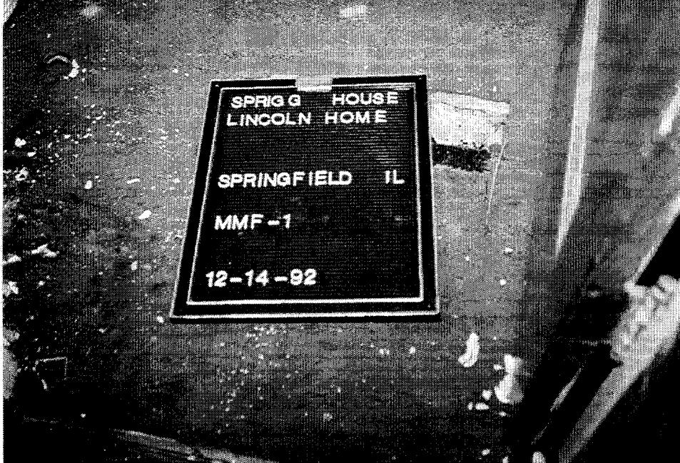
Photo MMF-1 Mastic Under Carpet Room 207D
