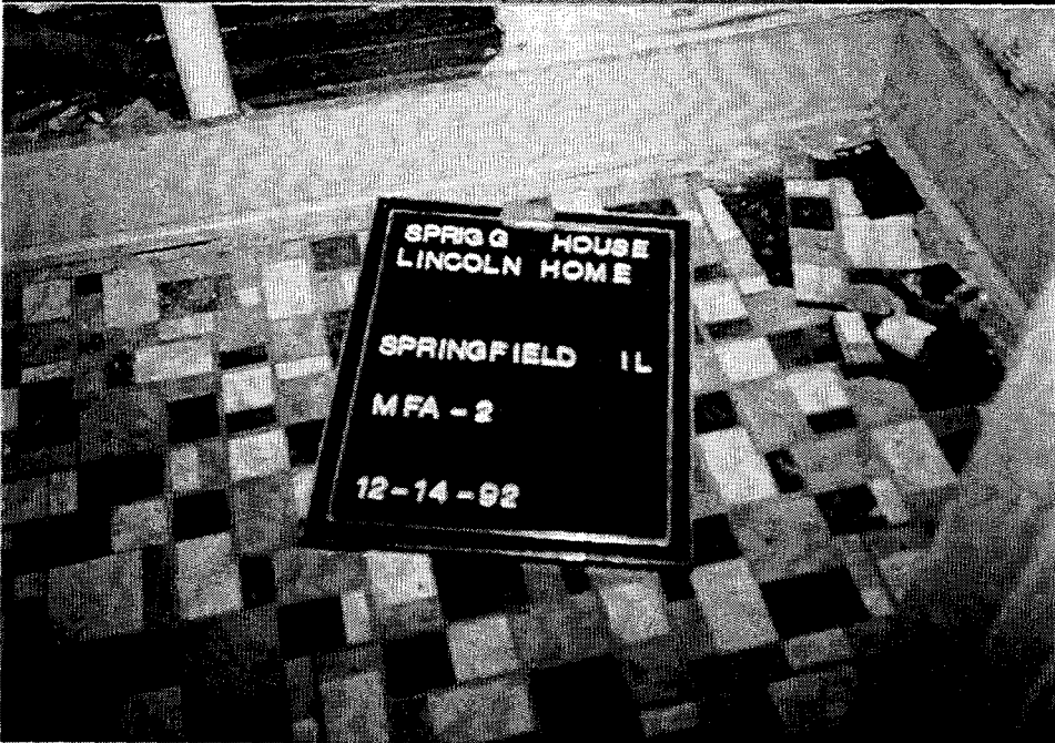
Photo MFA-2 Sheet Flooring-Linoleum Closet 207B
