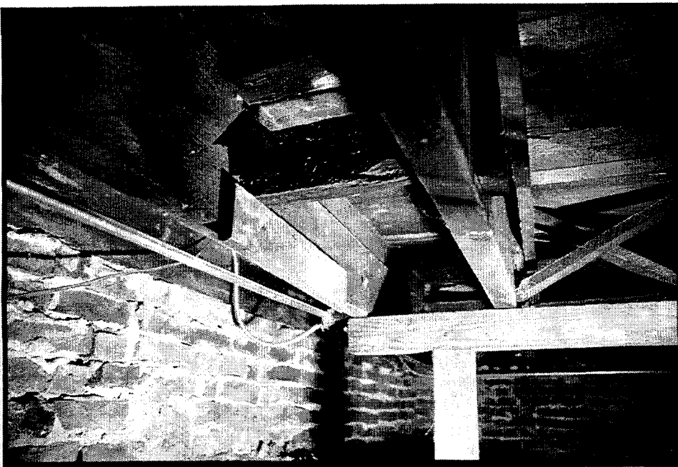
FIGURE 3.25 LOCA- TION OF THE CHIM- NEY STACK AND HEARTH
