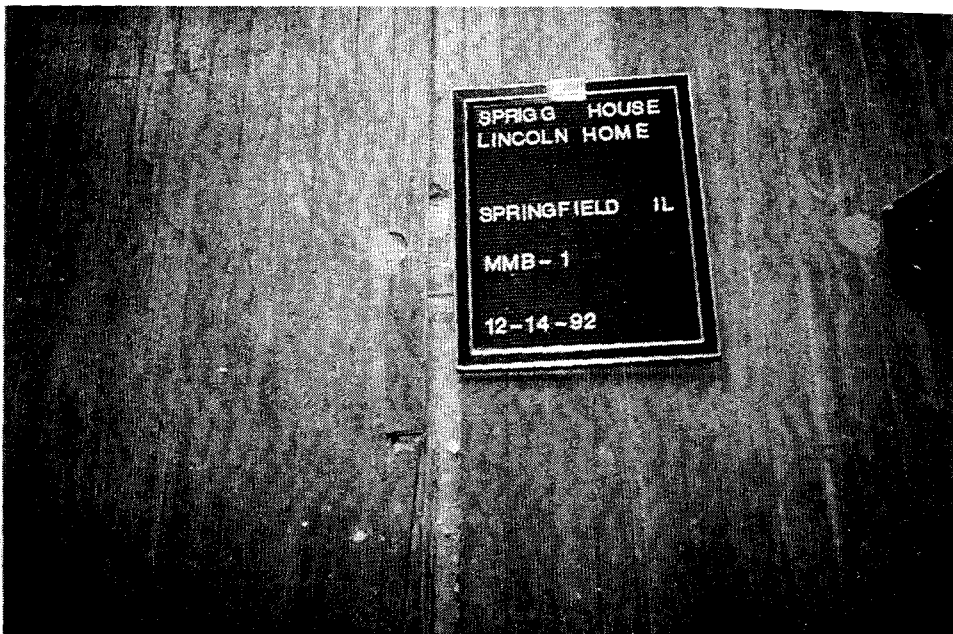
Photo MMB-1 Felt Paper Under Wood Floor Room 204
