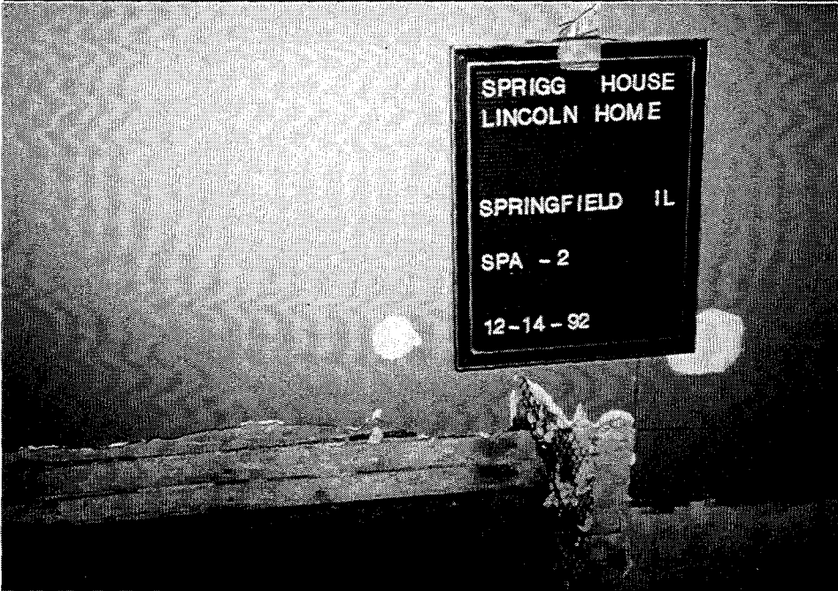
Photo SPA-2 1922 Plaster Room 208-Wall
